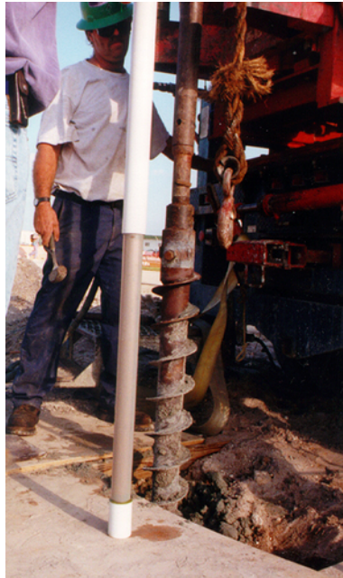
Figure 4. Installation of ISPF with adjacent hollow-stem auger at OU 1.
