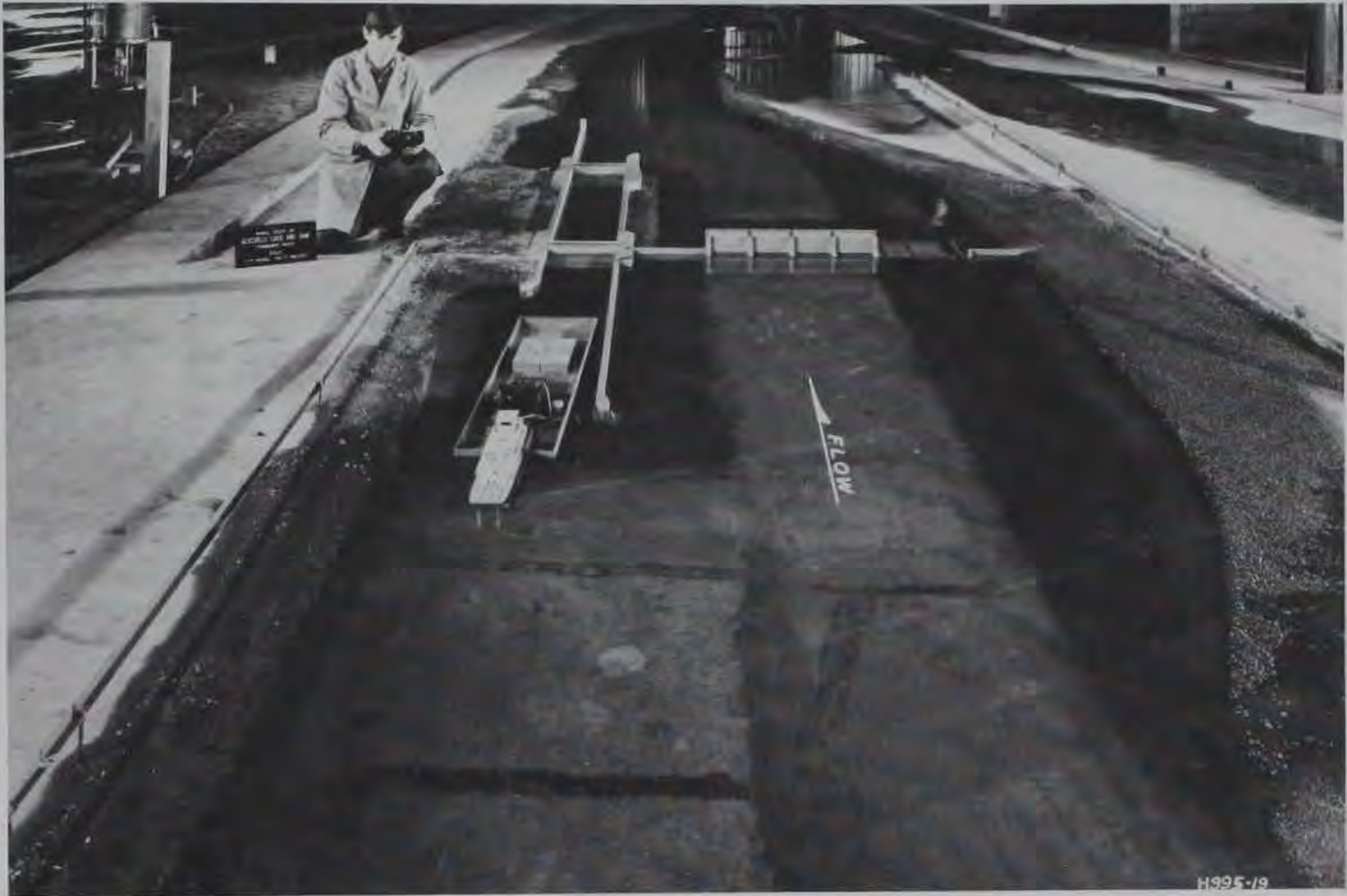
Figure 5. Remote-controlled towboat and tow in the upper lock approach
