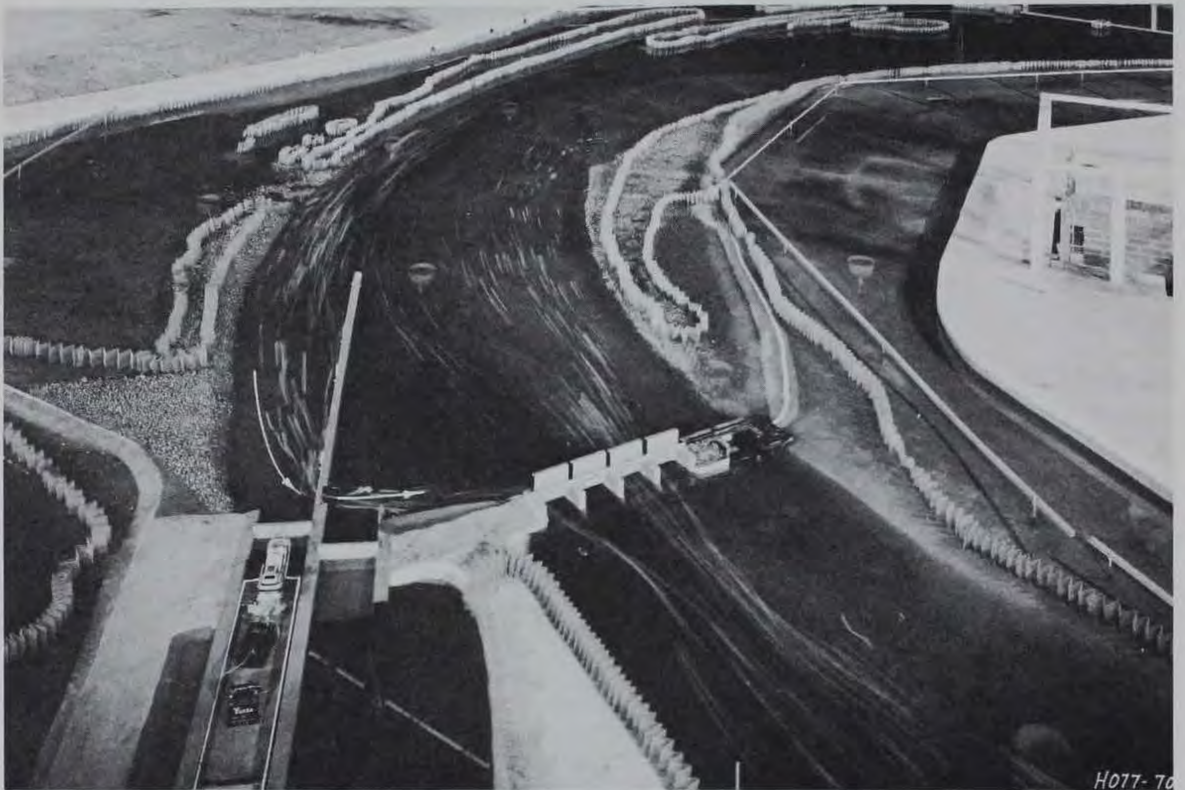
Photo 3. Plan A-modified; discharge 36,000 cfs, upper pool el 674.0. Surface currents in approaches to lock and dam. Note flow through the ice gap in upper guard wall
