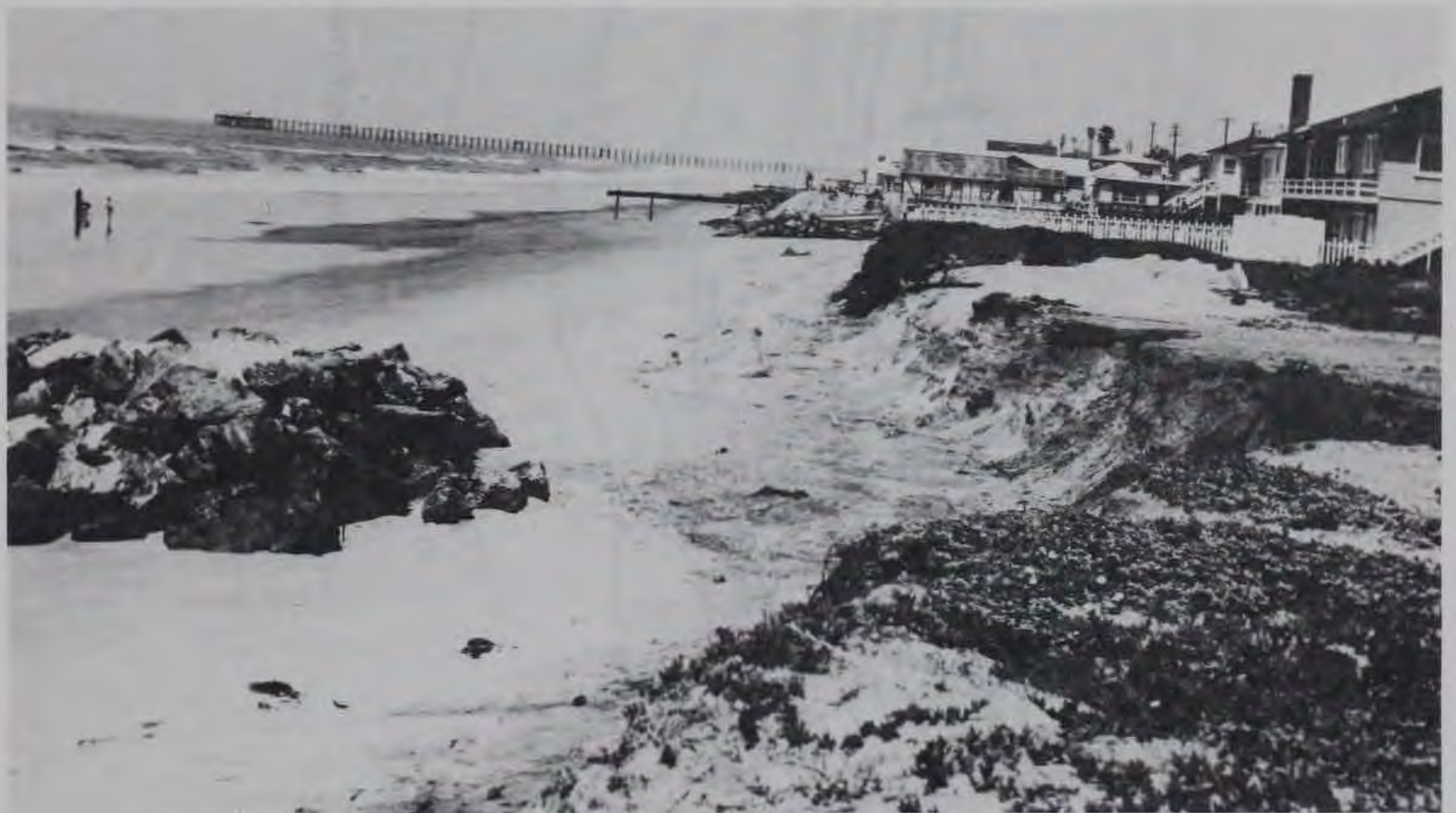
Figure 3. Typical beach erosion at Oceanside
