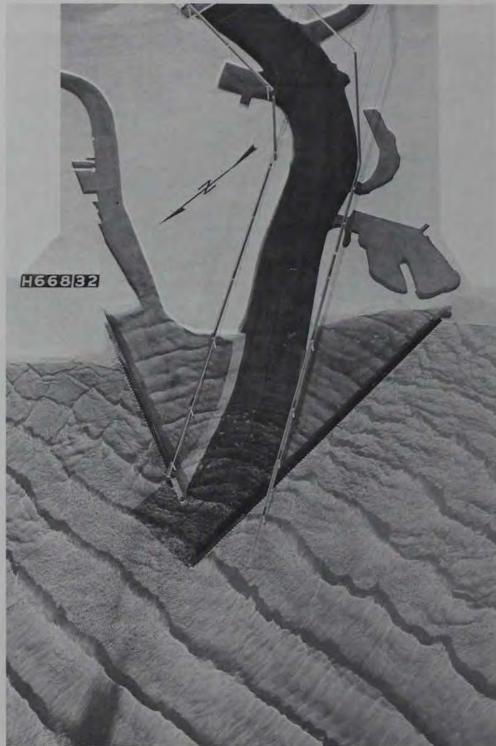
Photograph 7. Plan 3; 9-sec, 10-ft waves from north 06^{\circ} east
