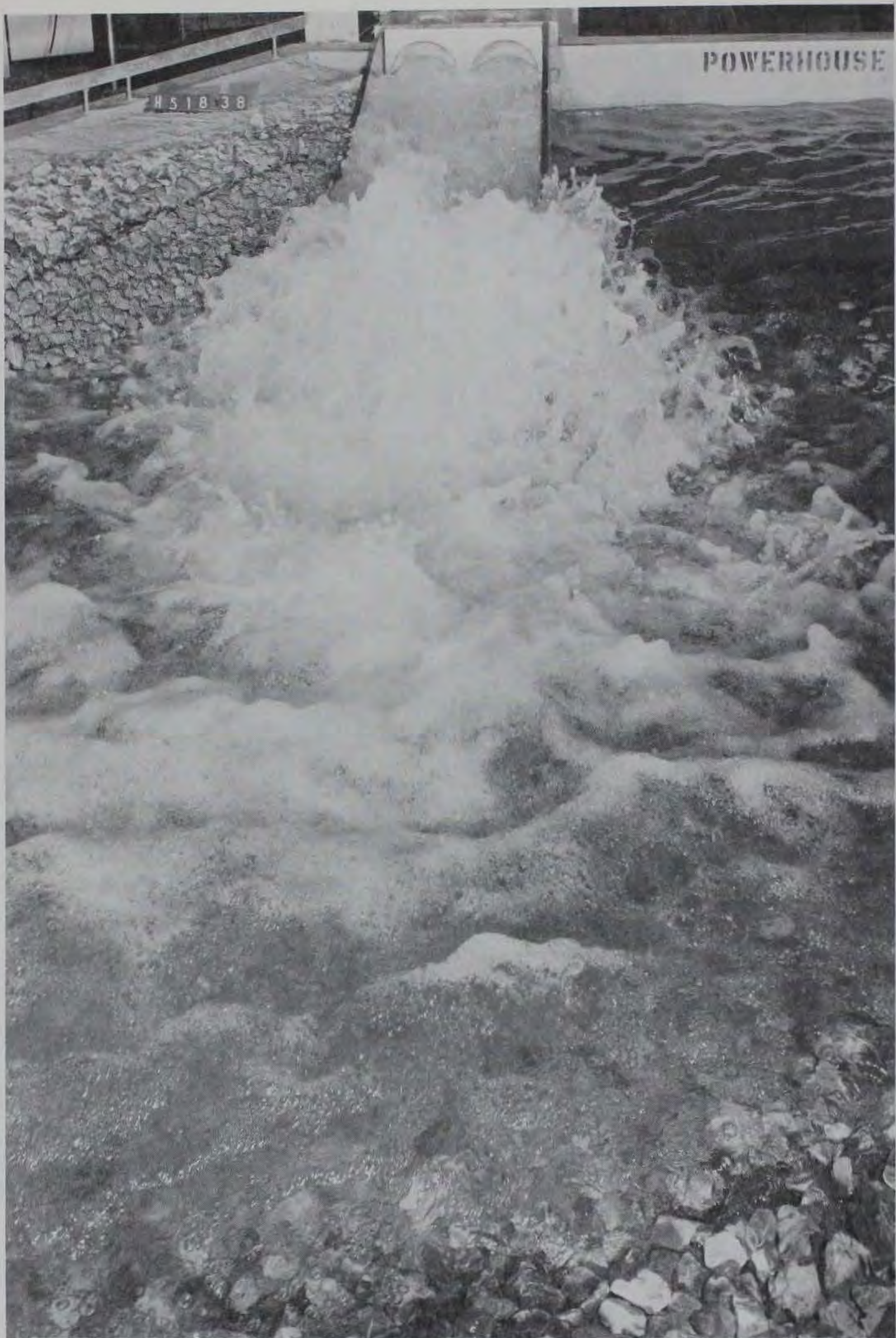
Photo 8. Recommended deflector plate design. Flow at pool el 1048, 28.1-in. sleeve travel, tailwater el 503, view from opposite bank showing attack on bank adjacent to tailrace
