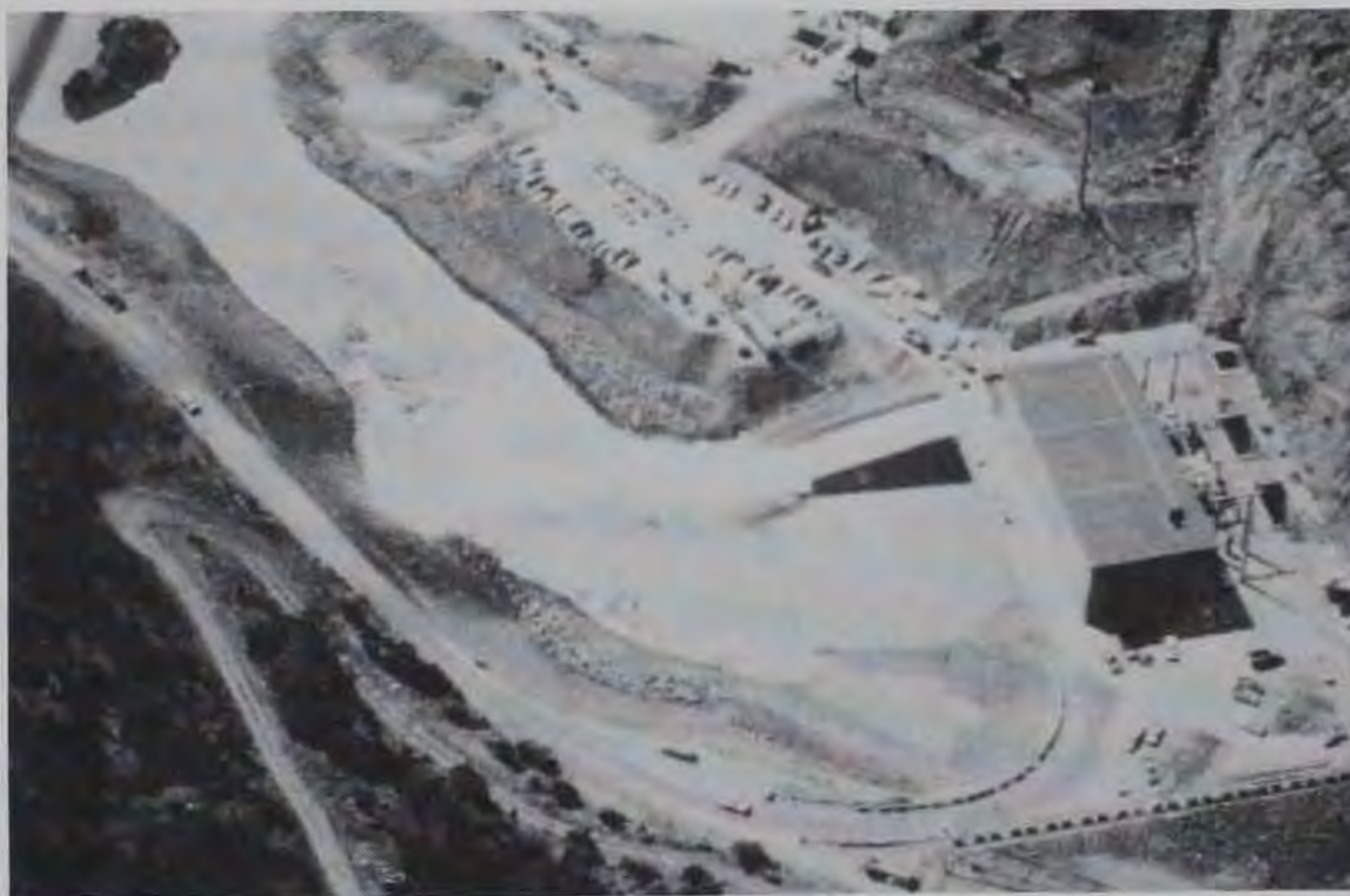
b. Aerial view of failure of opposite bank
