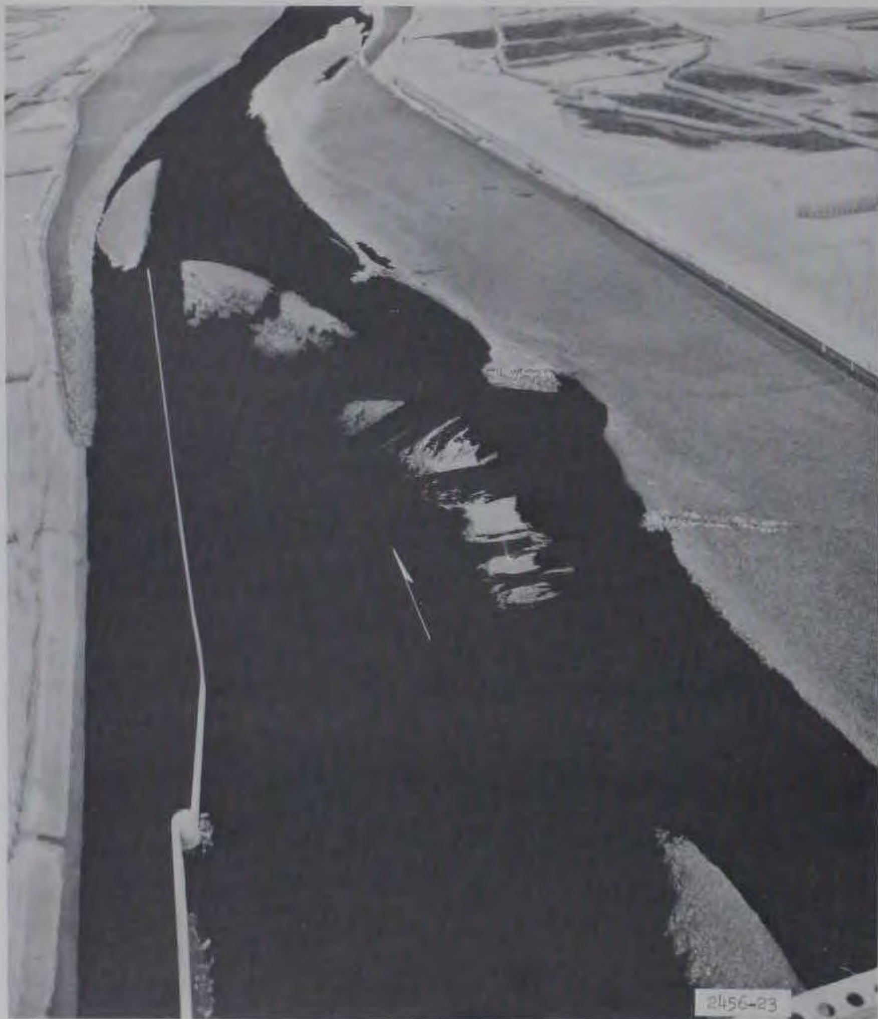
Photograph 9. Plan A-6, run 1, pool el 166.1. Note shoal area in the approach channel downstream of the end of the guard wall extension
