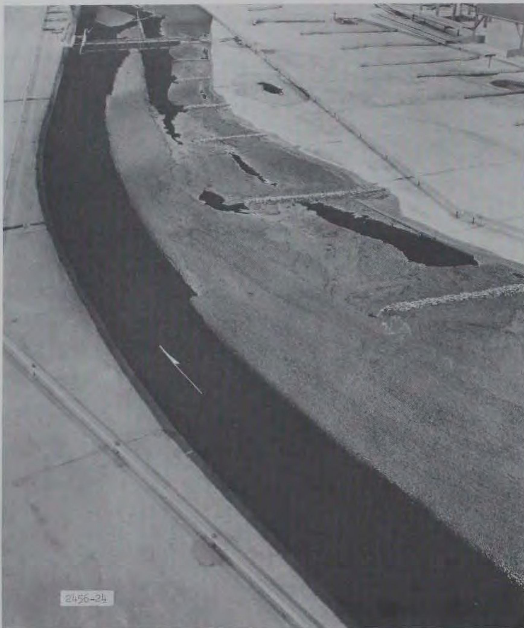
Photograph 7. Plan A-5, run 4, water surface lowered to el 168.0. Note bar formation opposite ends of right bank dikes
