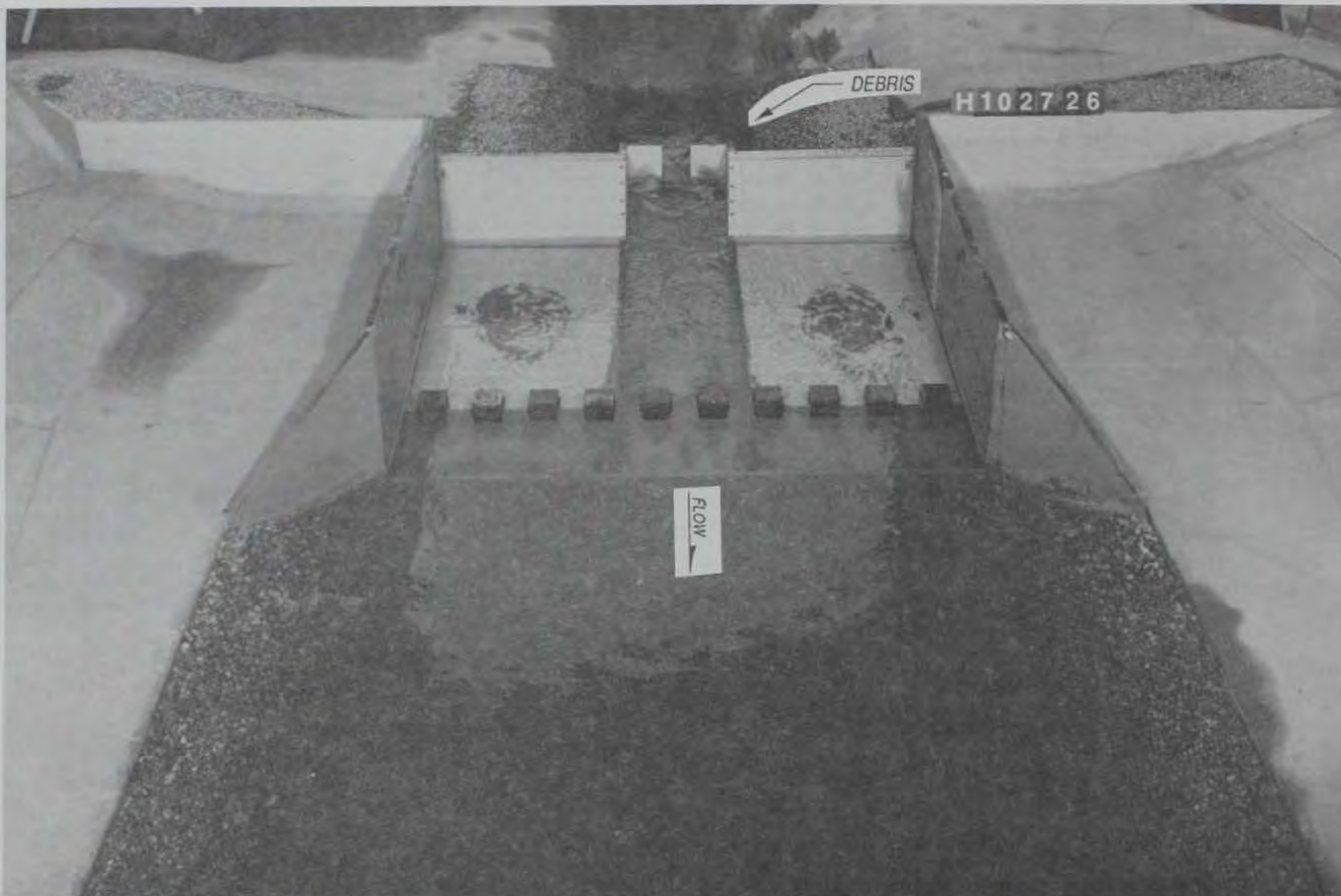
Photo 10. Type 2 debris deflectors, debris passage looking upstream, discharge 28 cu m/sec (1,000 cfs), tailwater el 735.54
