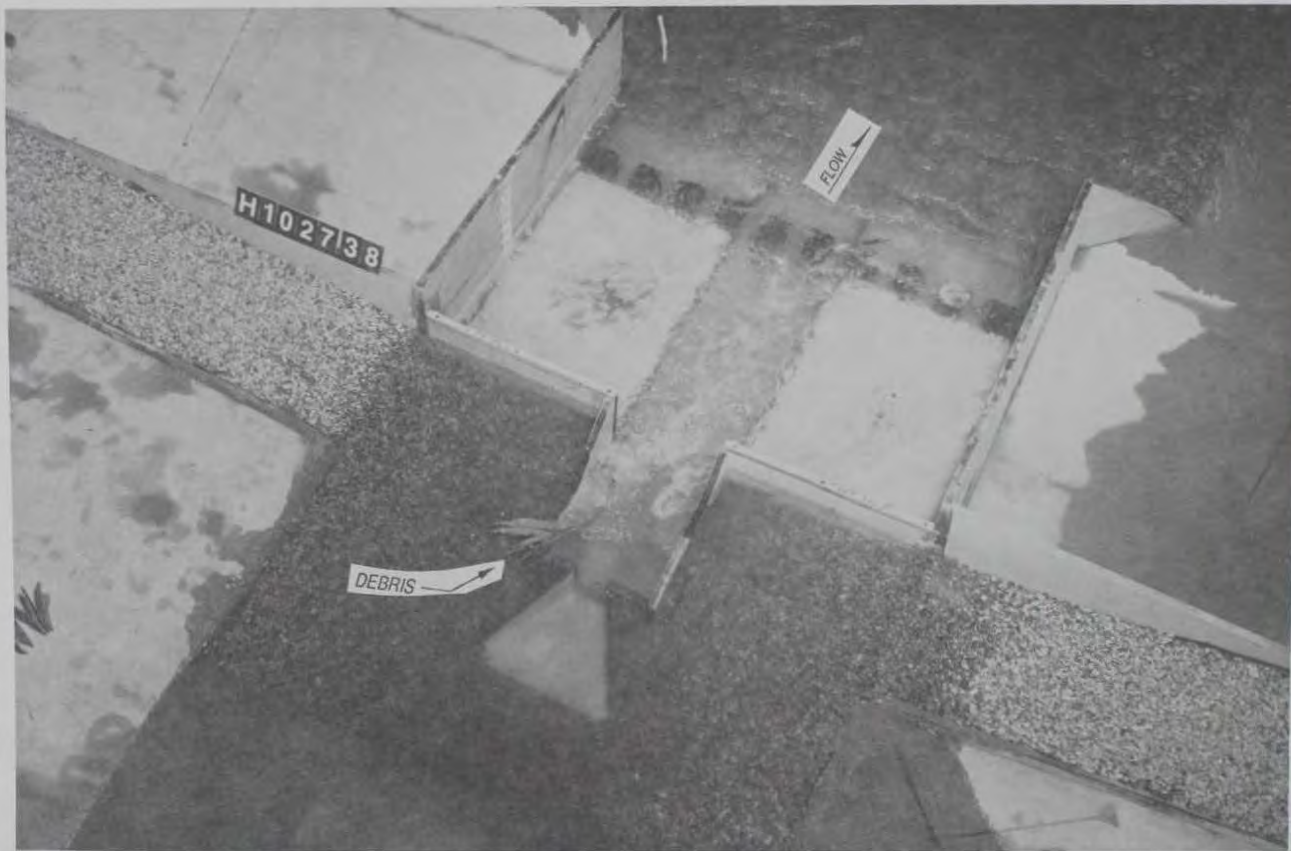
Photo 15. Type 2 debris deflectors, debris passage looking downstream, discharge 283 cu m/sec (10,000 cfs), tailwater el 747.01
