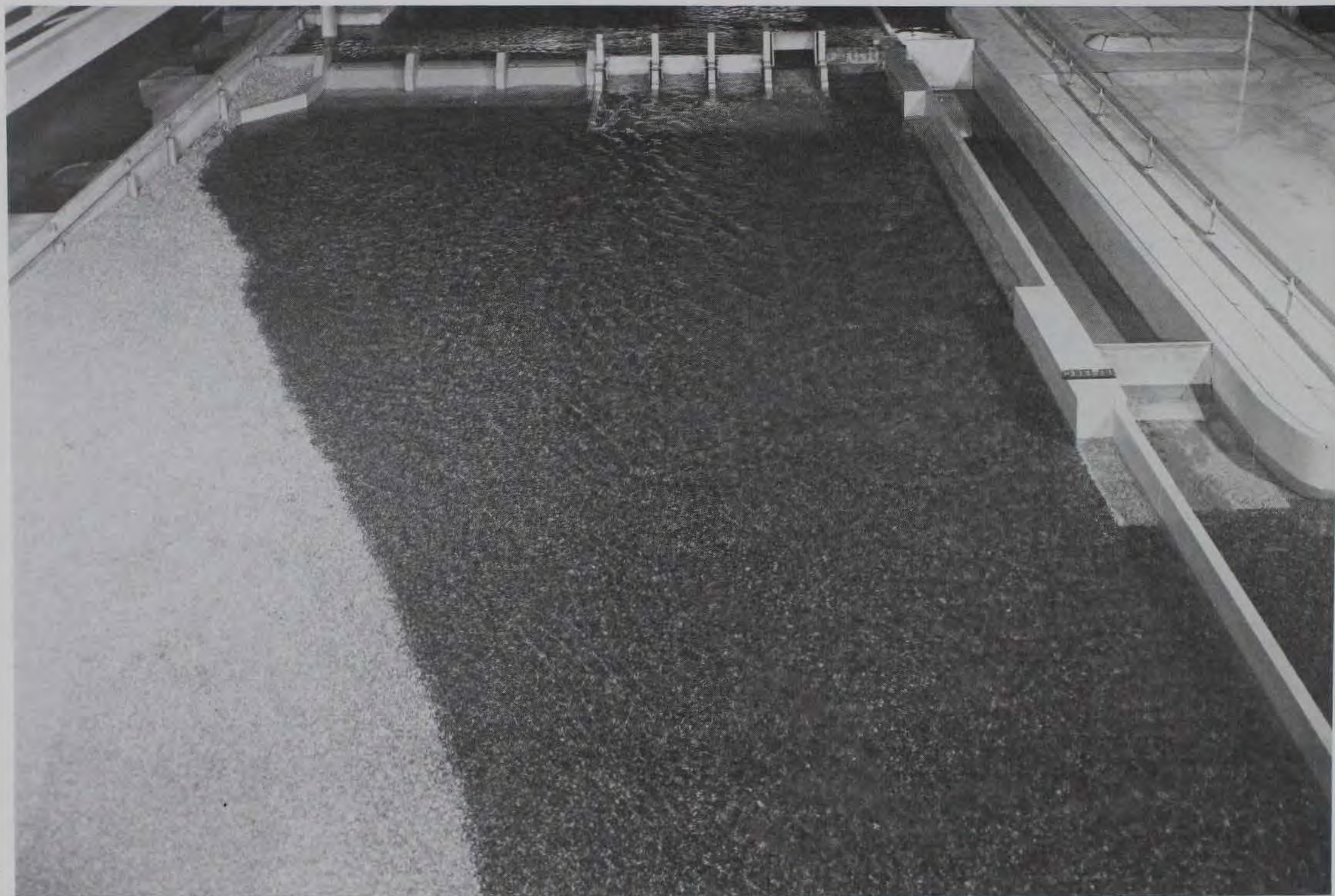
Photo 5. One tainter gate fully open; pool el 122; tailwater el 95; looking upstream
