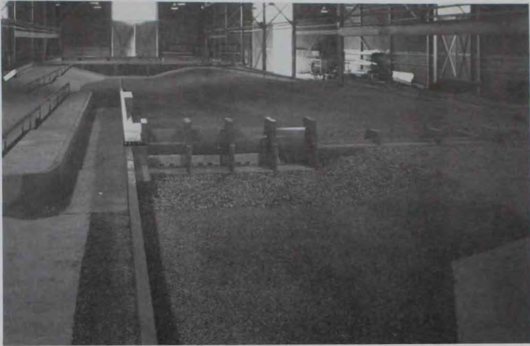
a. Looking downstream
