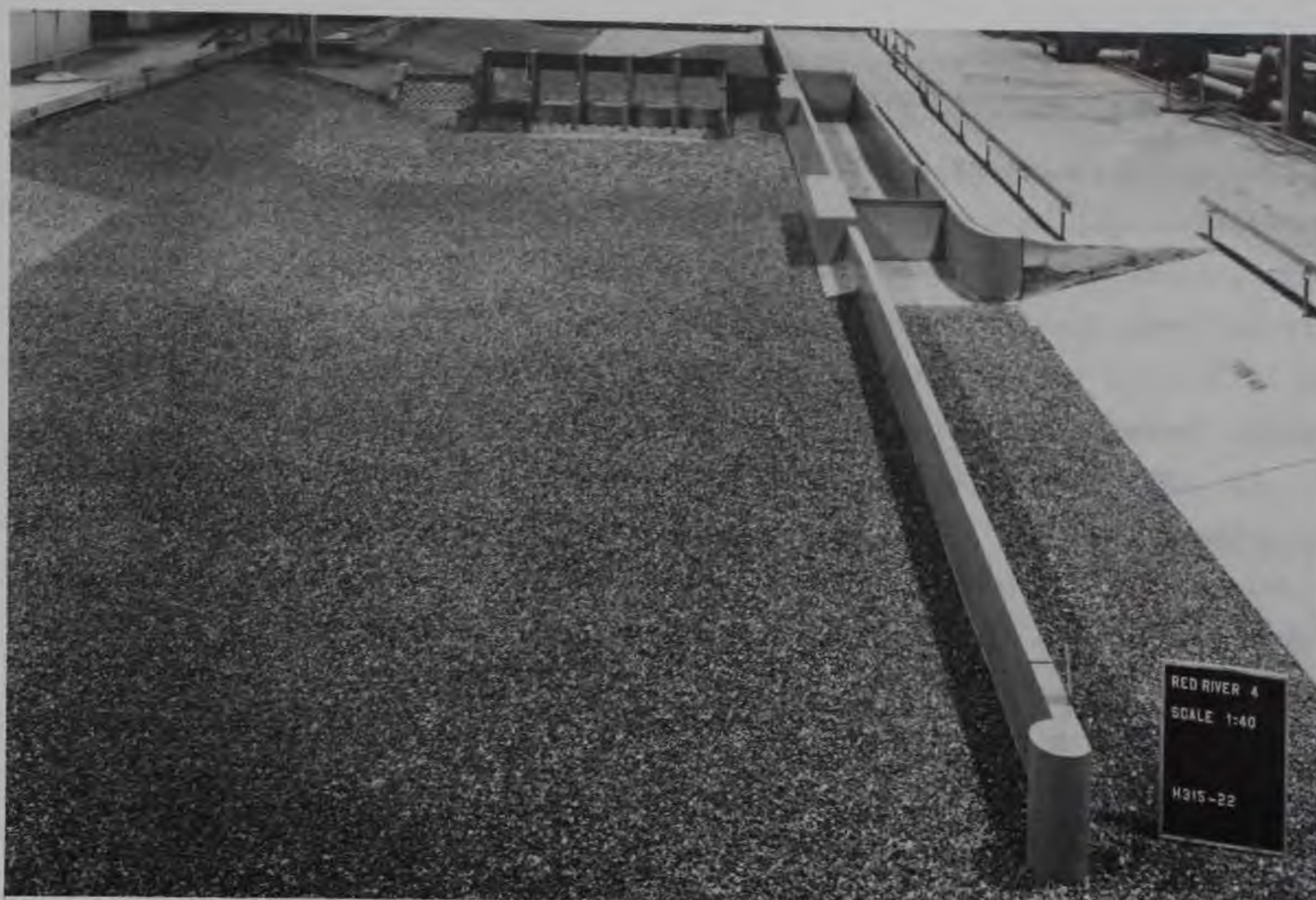
Figure 7. Overall view of downstream channel looking upstream
