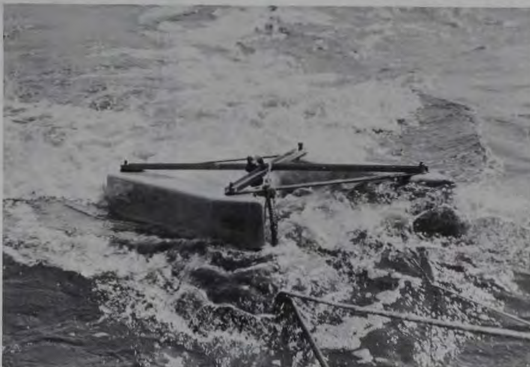
Fig. 16. Boomer transducer mounted on catamaran trailing the survey boat
