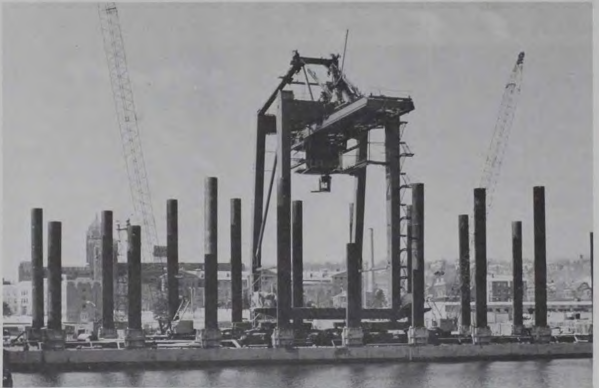
Fig. 70. DeLong barges supporting gantry cranes at Cam Rahn Bay
