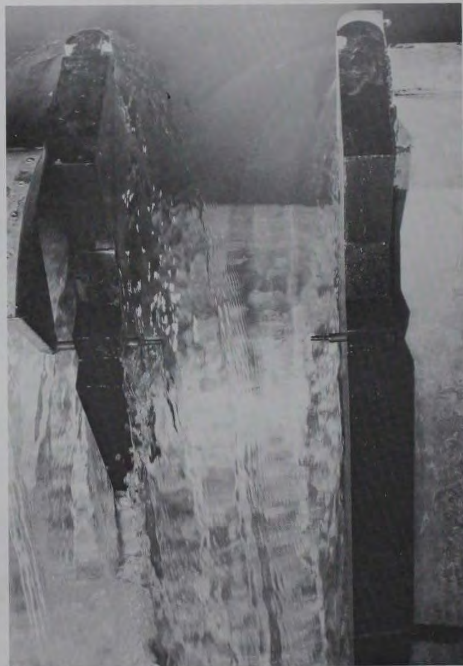
b. Type 2 left abutment
