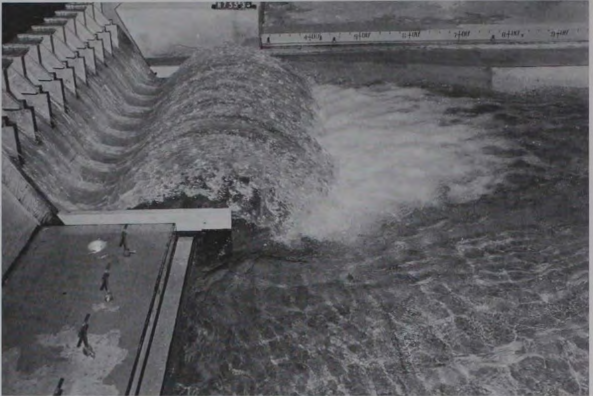
c. Discharge 200,000 cfs, pool el 484.0, tailwater el 337.0
