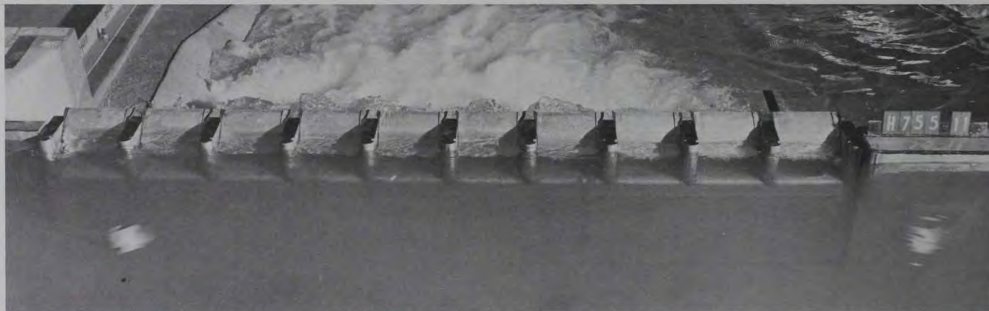
b. Discharge 528,000 cfs, pool el 485.0, all gates open 30.6 ft
