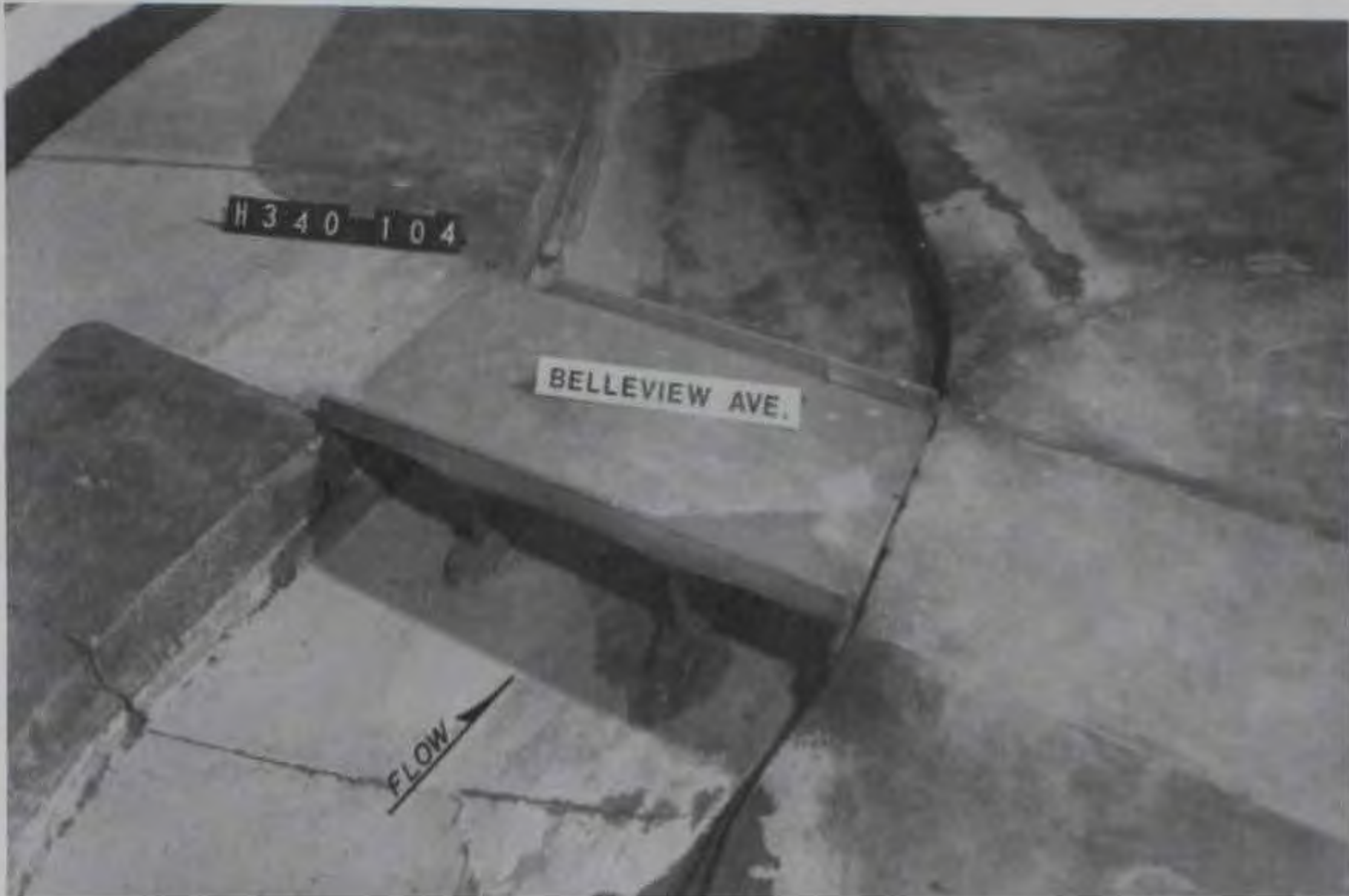
a. Belleview Avenue Bridge
