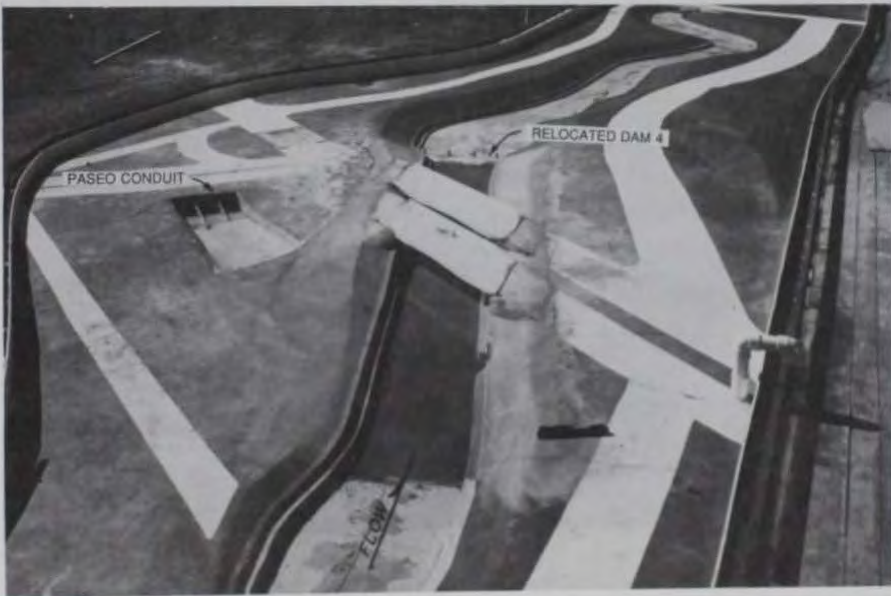
Photo 59. Paseo realignment, sta 123+00 to sta 147+00
