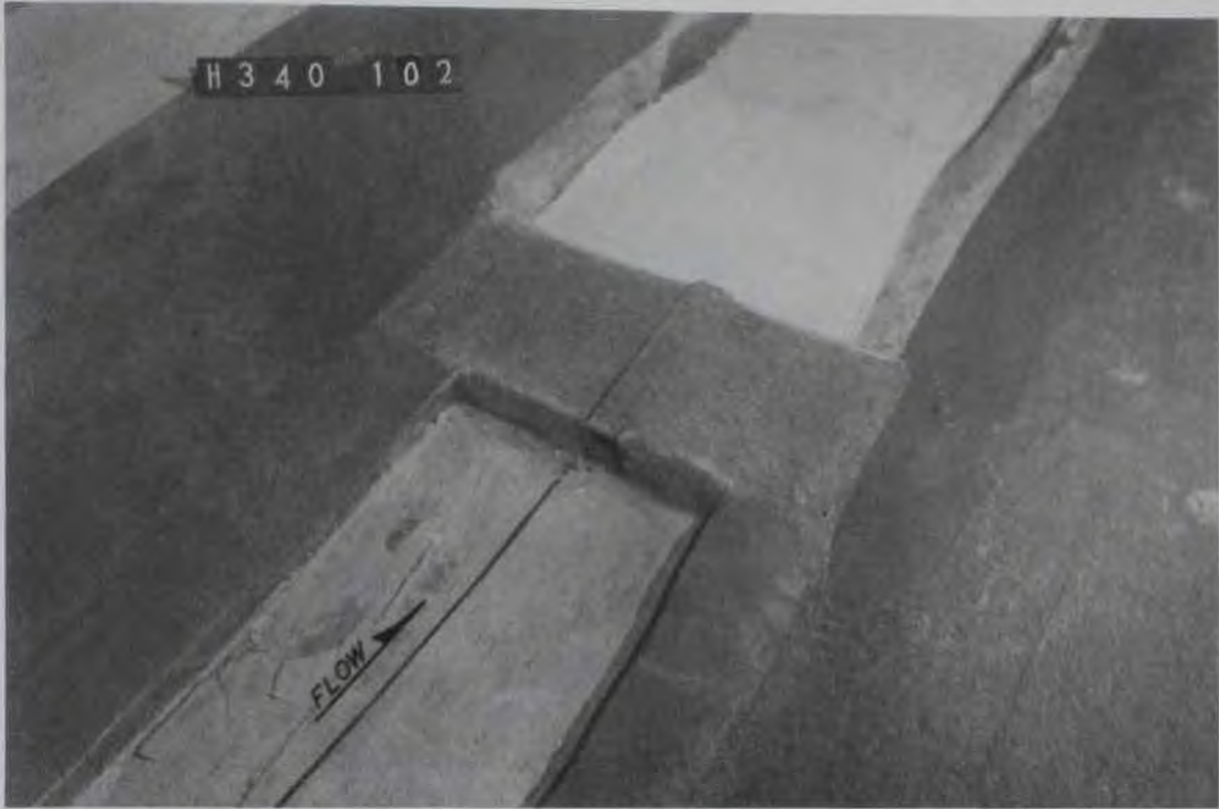
Photo 41. Modification at low-water crossing (51st Street)
