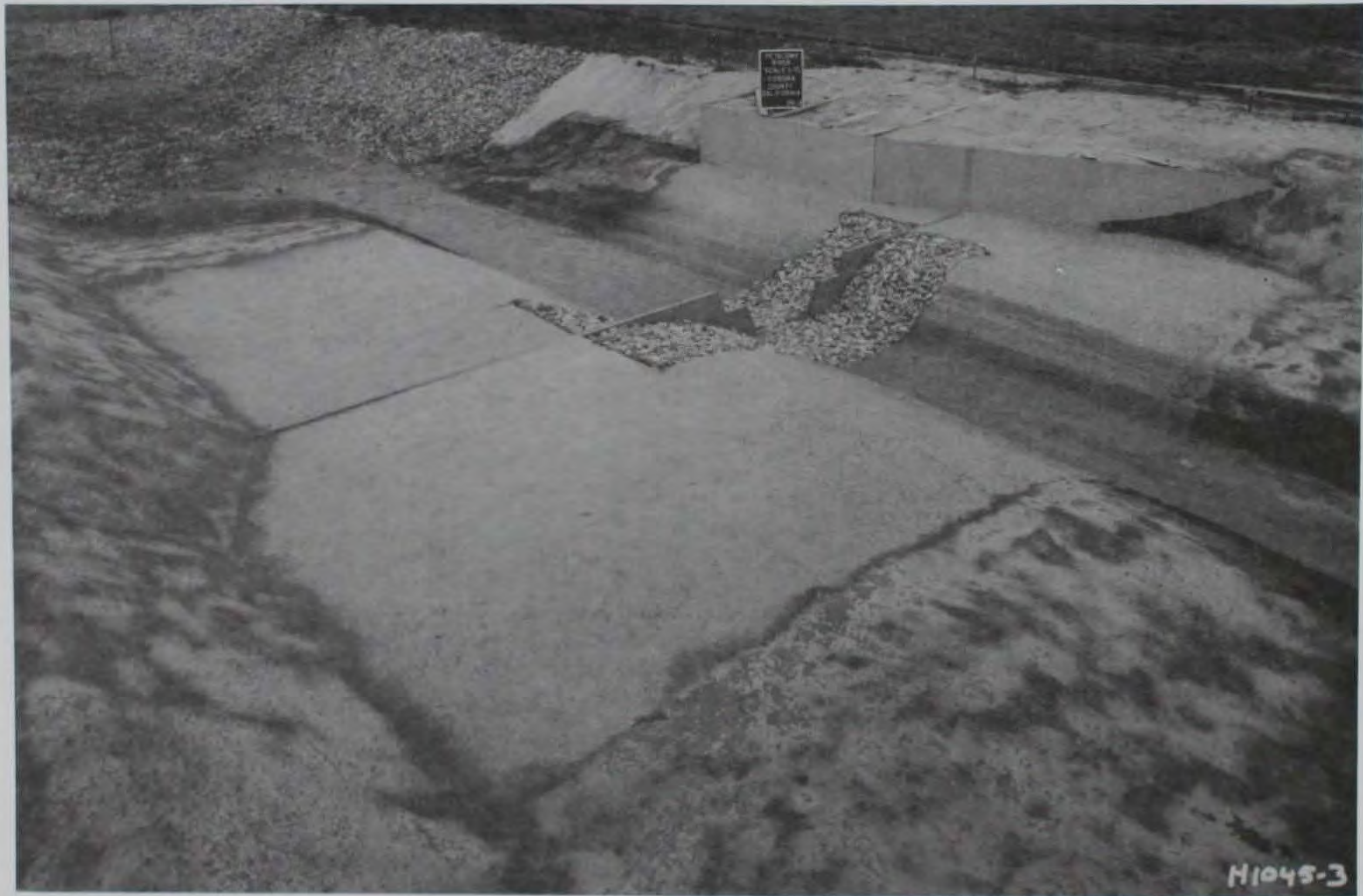
Figure 5. Side view of weir
