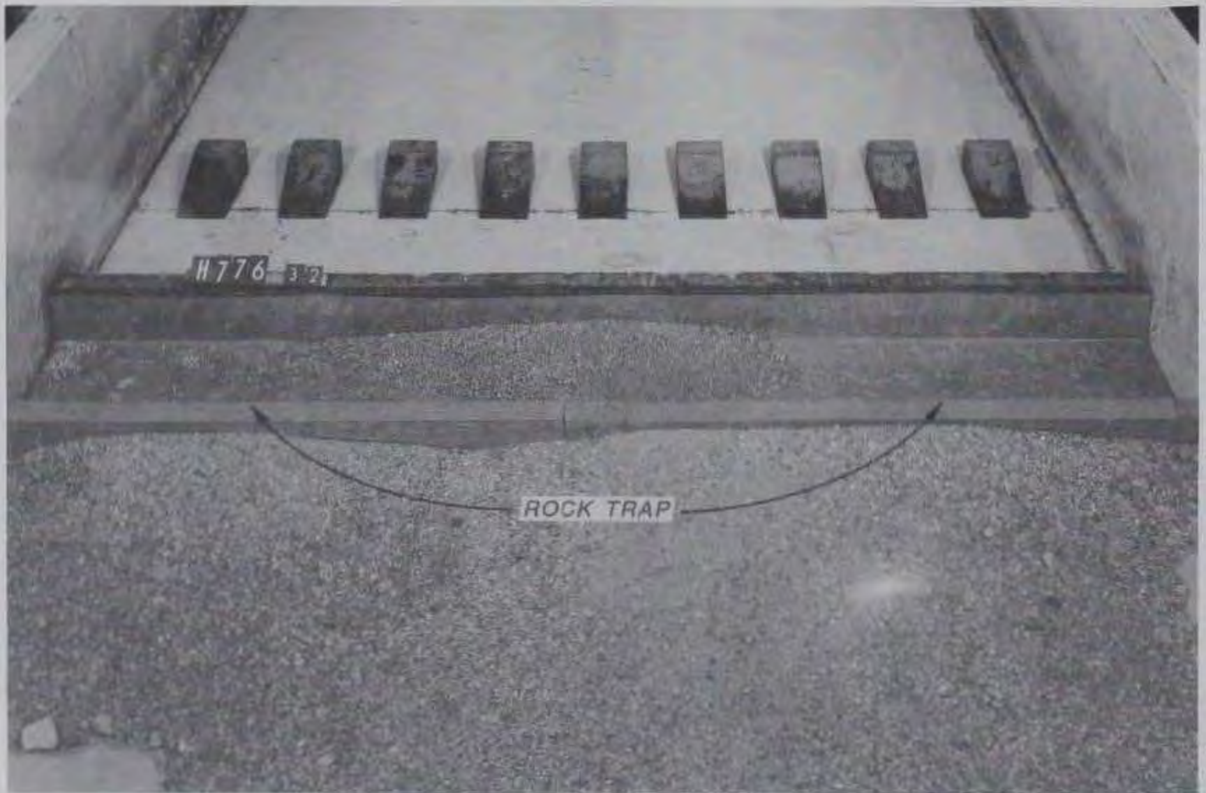
b. Dry bed view of rock trap
