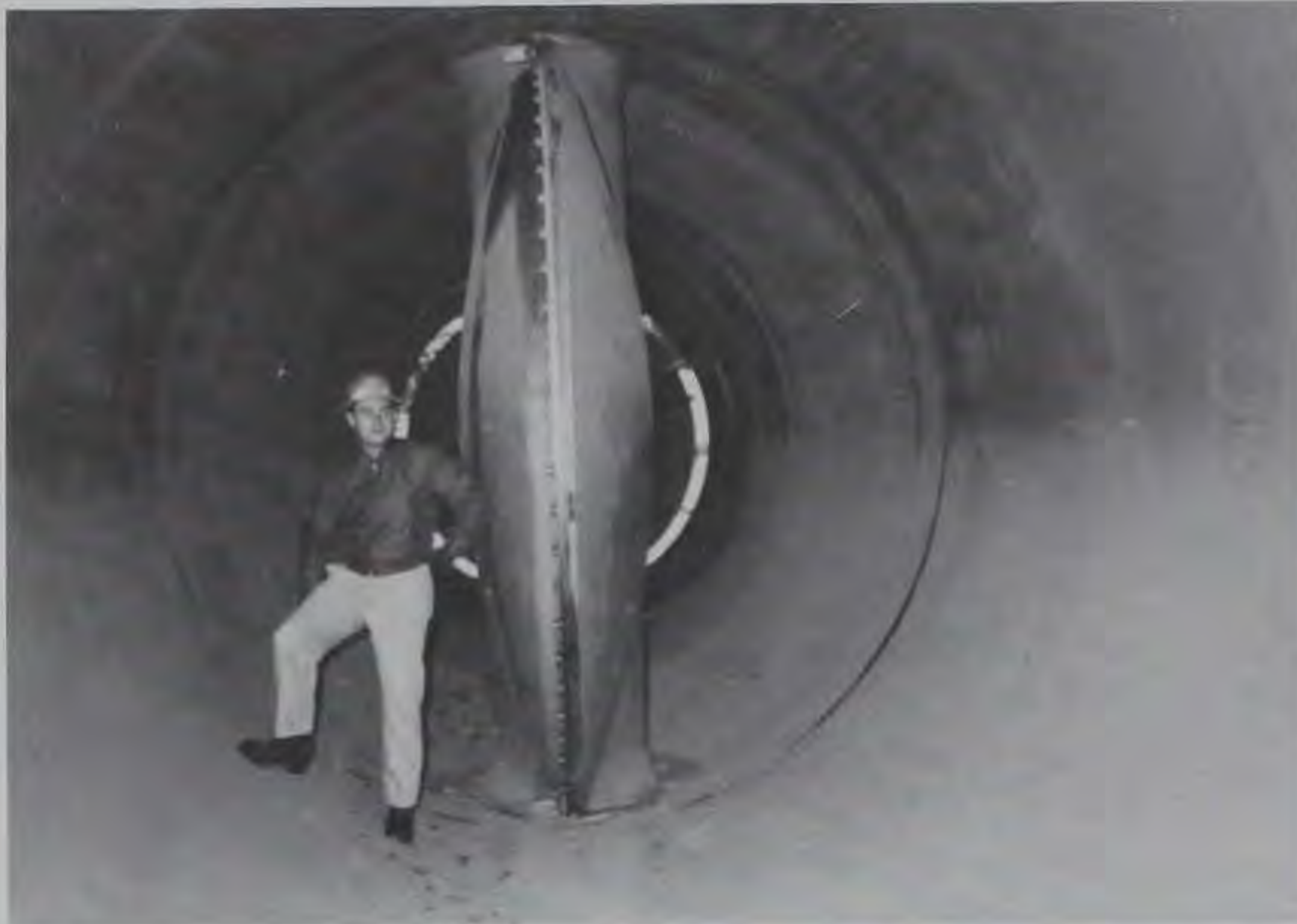
Fig. 6. Looking downstream at the fully open butterfly valve. Note the original 108-in.-diam Howell-Bunger valve in the background
