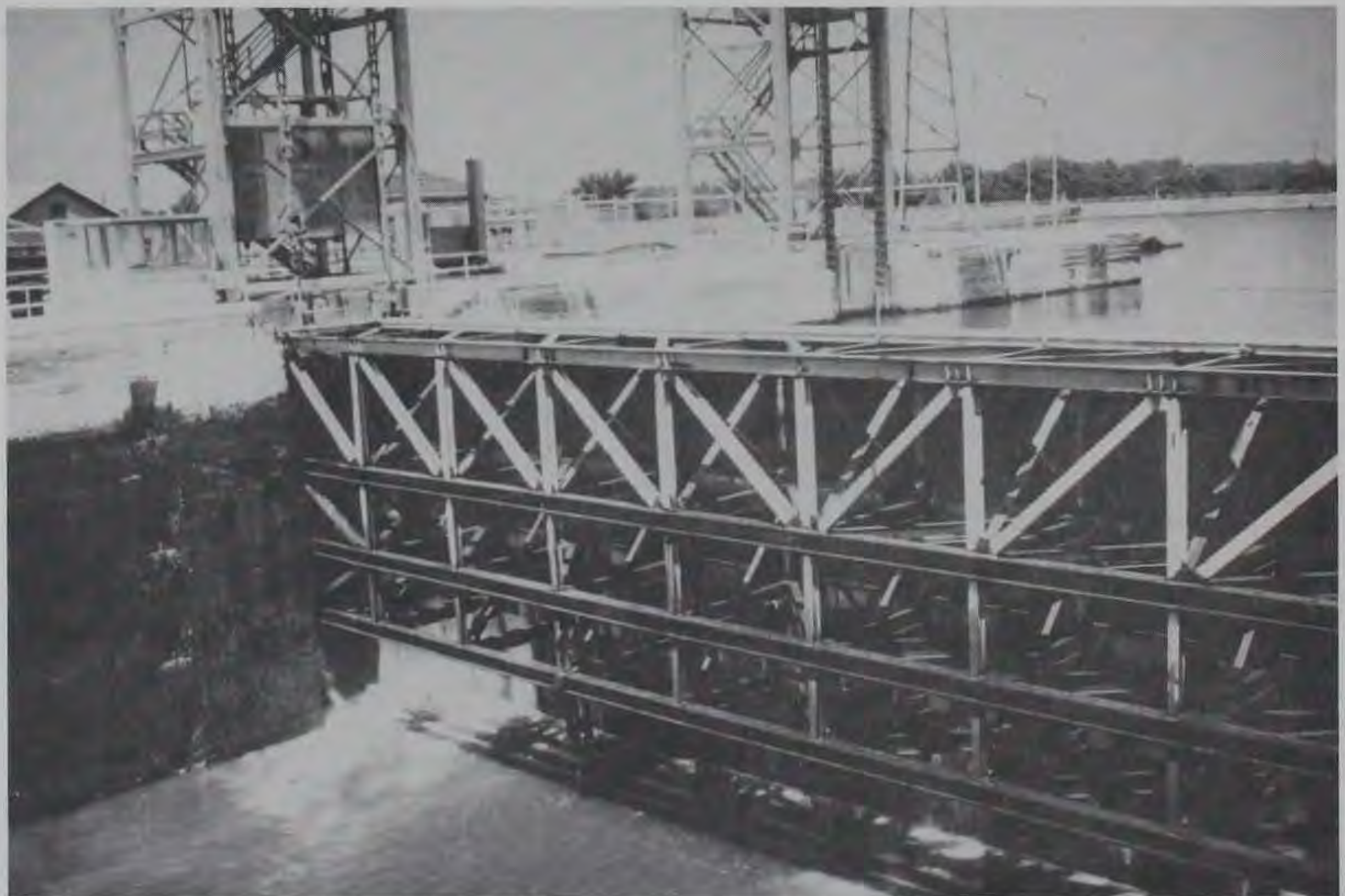
Figure 2. Lockport Lock lift gate
