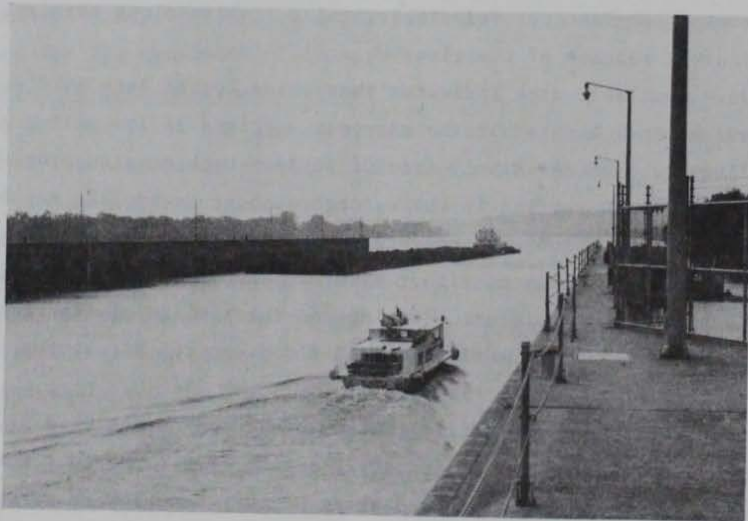
Figure 108. Survey boat used in support of Ohio River acoustic profiling survey, shown leaving the Greenup Locks and Dam
