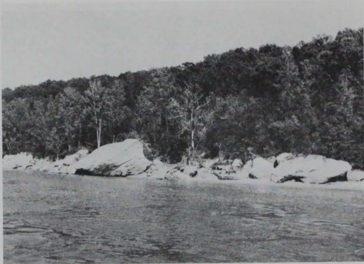
Figure 83. Large, detached pieces of rock along bank line at the base of Fountain Bluff at about RM 82.6 upstream from Grand Tower, Ill.
