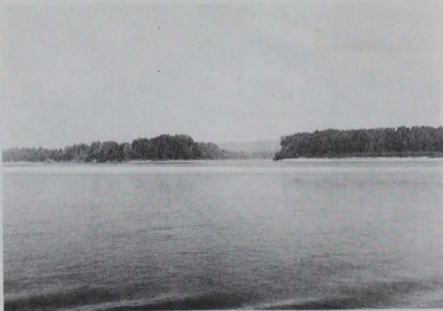
Figure 84. Side channel closure caused by sandbar development resulting from dike placement upstream of mouth of chute
