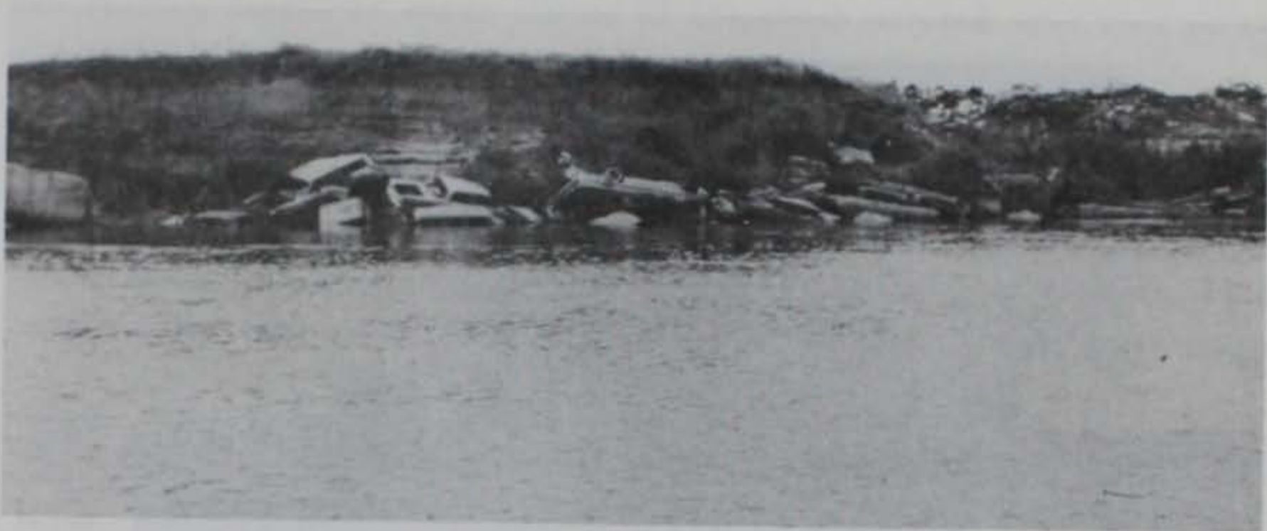
Figure 50. Bank-line protection measures undertaken by local interests along a portion of the east bank of the White River just downstream of Augusta, Ark.
