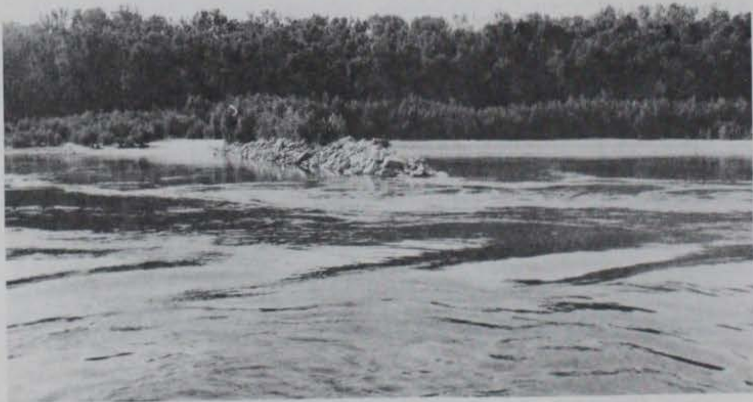
Figure 78. Stone training dike of type used along Middle Mississippi River by the CE
