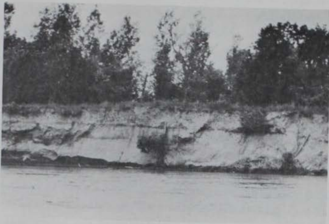
Figure 94. Section of actively caving bank line on the Missouri River bank composed of heterogenous mixture of materials of dredged spoil material
