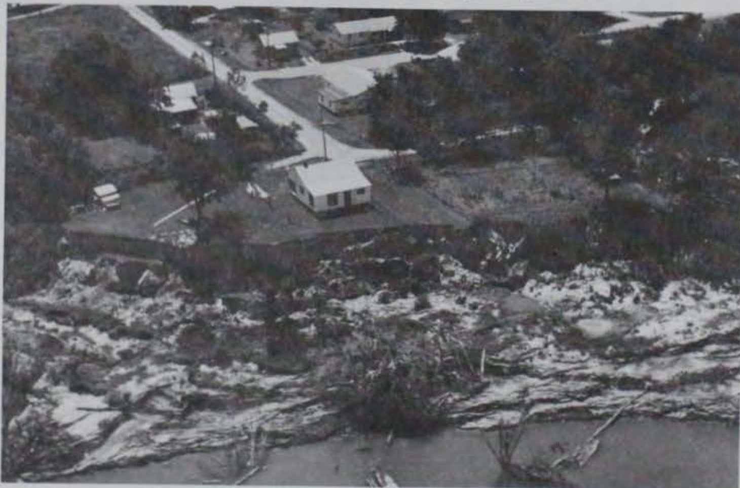
Figure 46. Aerial view of bank-line failure at a point along west bank line of White River at Des Arc, Ark., view to the east (from Memphis District, CE)
