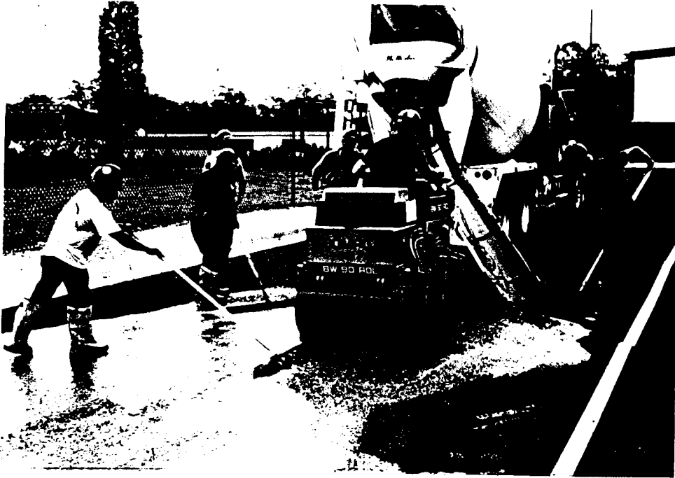
Figure 1.3: Typical view of applying grout to open-graded asphalt concrete surface
