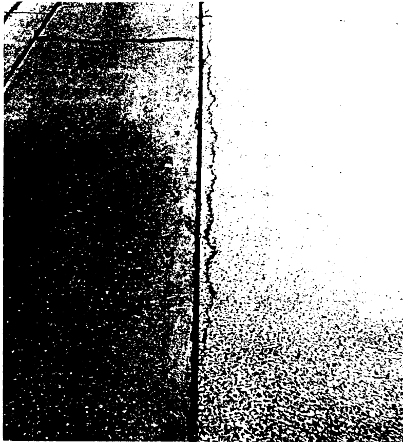
Figure 3.10: Cracking near RMP/PCC interface on Operations Apron
