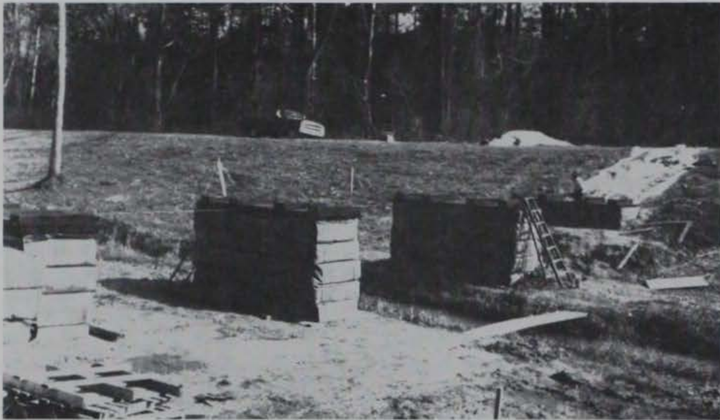
Photo 17. Bearing pads above supports
