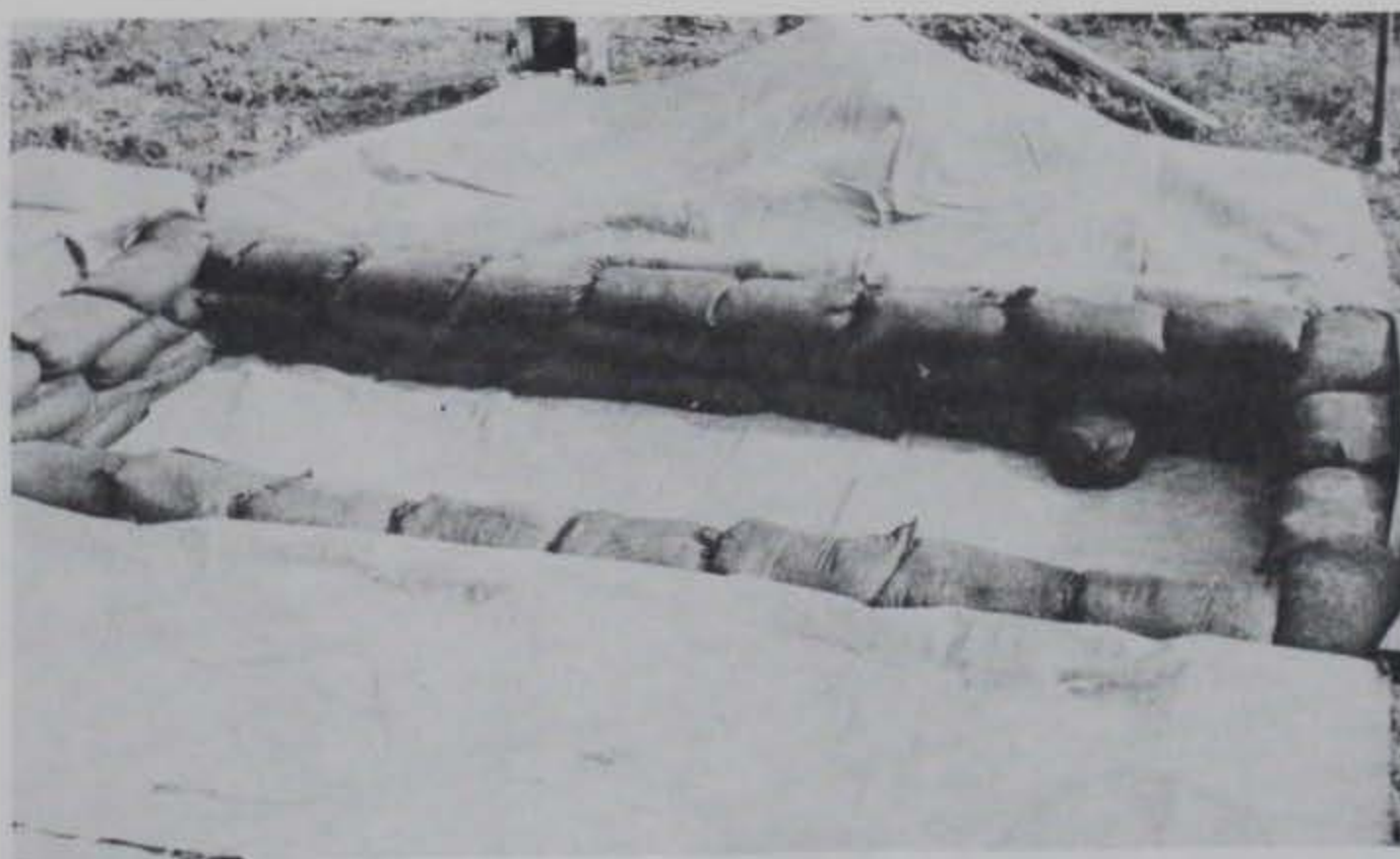
Photo 8. Typical first support layer showing sandbag form (note membrane flaps)
