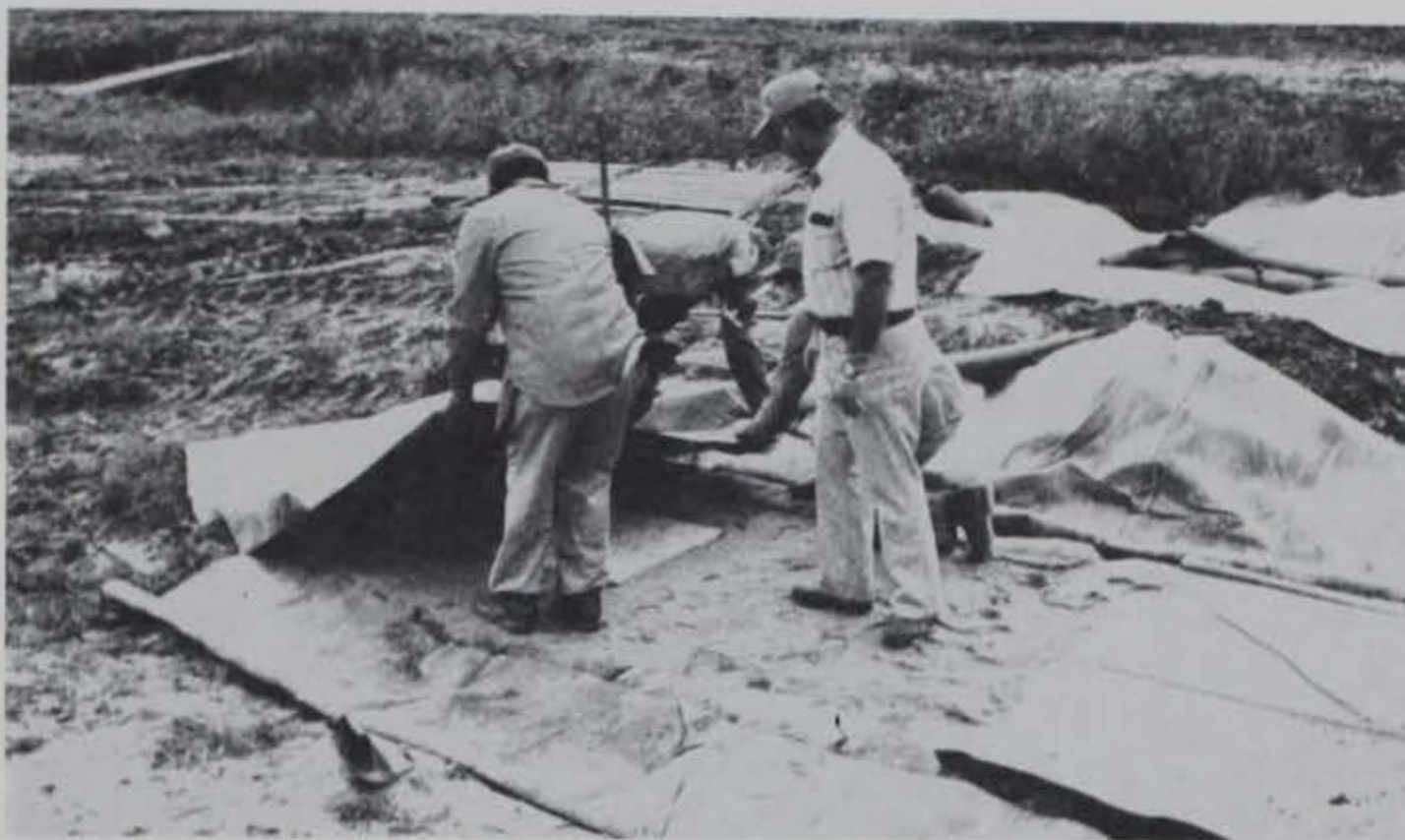
Photo 11. Closing flaps of membrane support layer (note plywood board)
