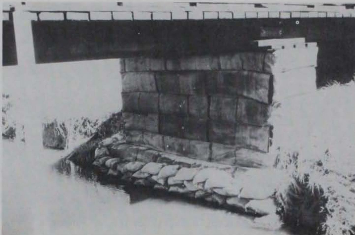
Photo 29. Scour protection at support 2 (March 1981)
