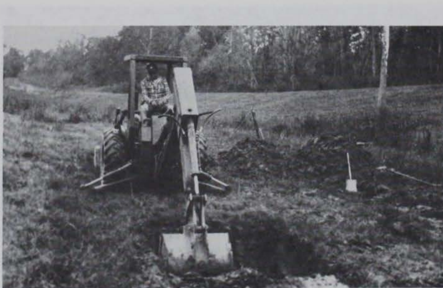
Photo 4. Excavating for layered support
