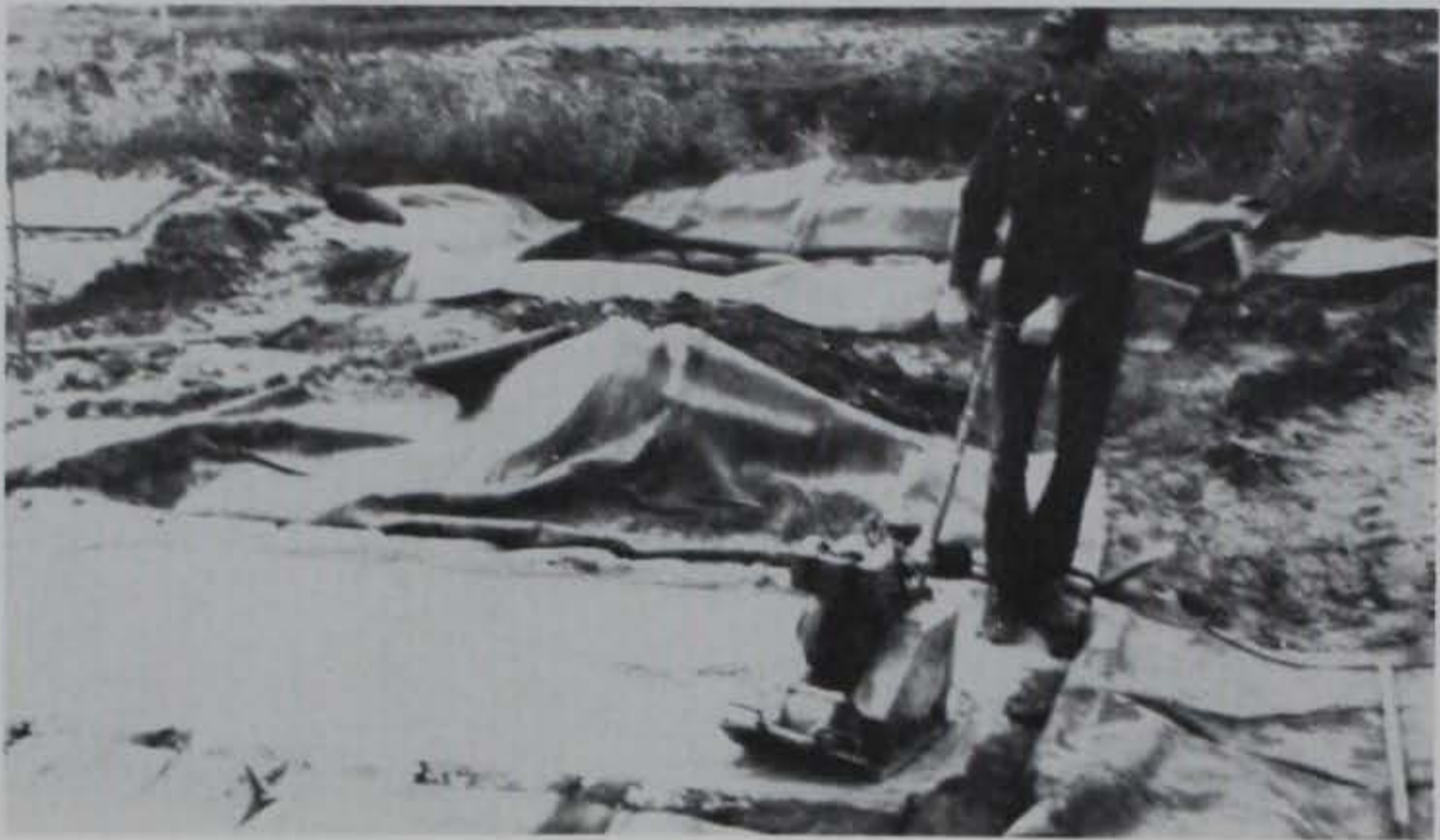
Photo 9. Compacting sand inside layer (mechanical compaction)
