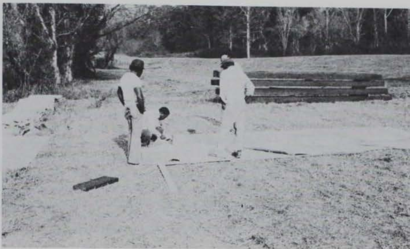
Photo 3. Cutting membrane pattern
