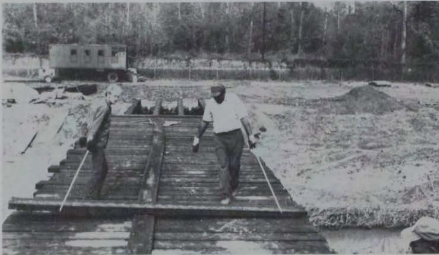
Photo 21. Placing decking on stringers
