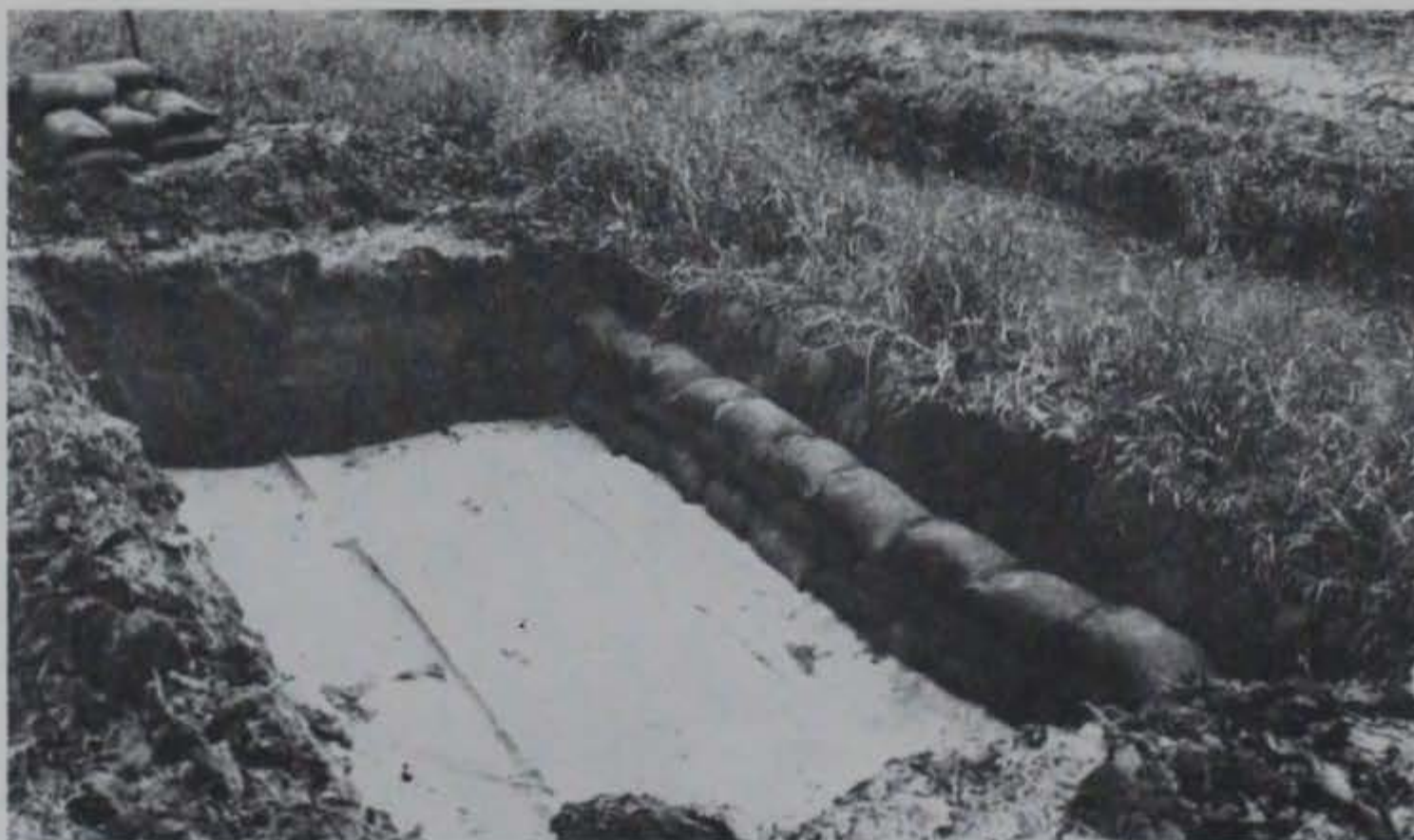
Photo 6. Excavation with bottom membrane and sandbags toward creek
