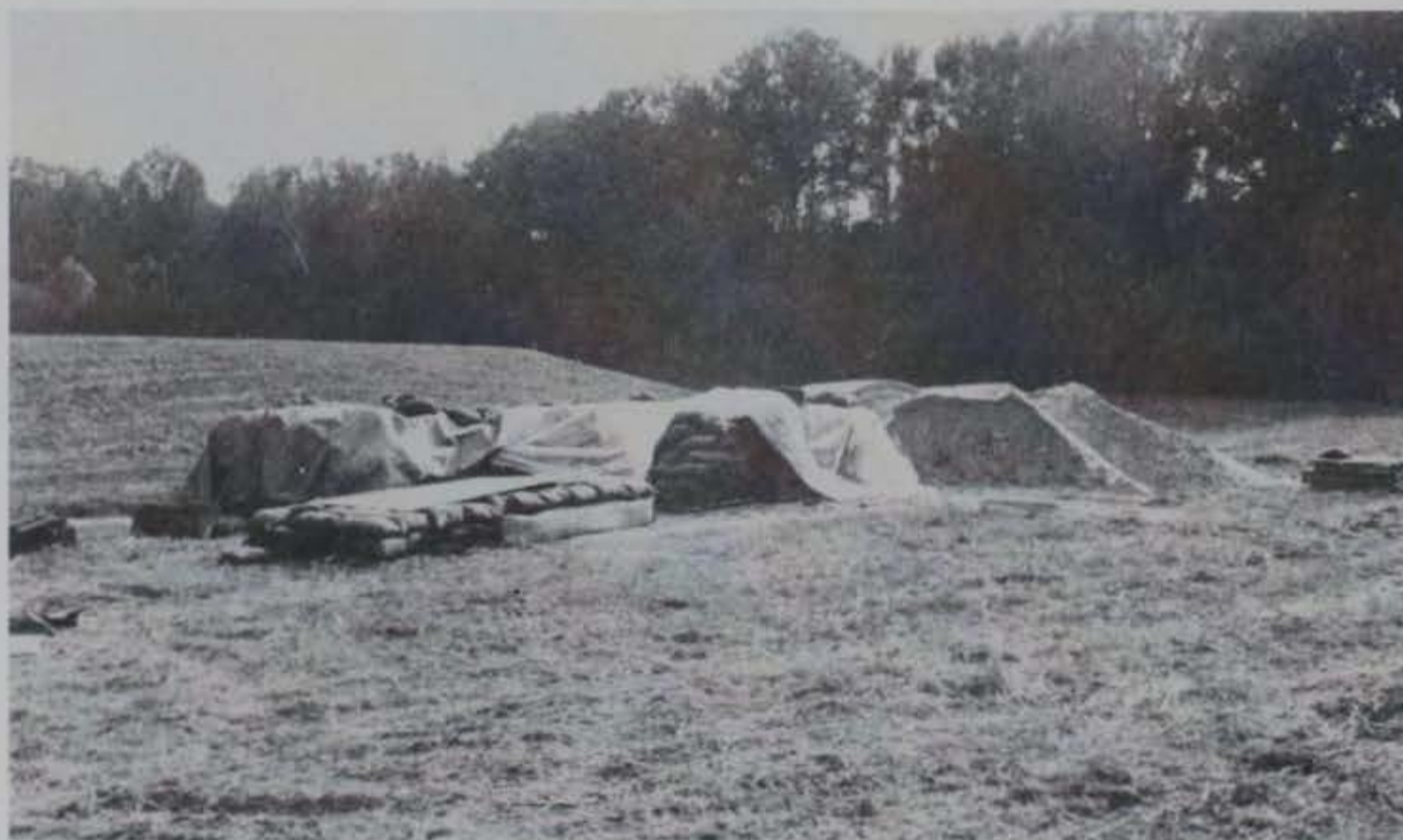
Photo 2. Sand stockpile and filled sandbags
