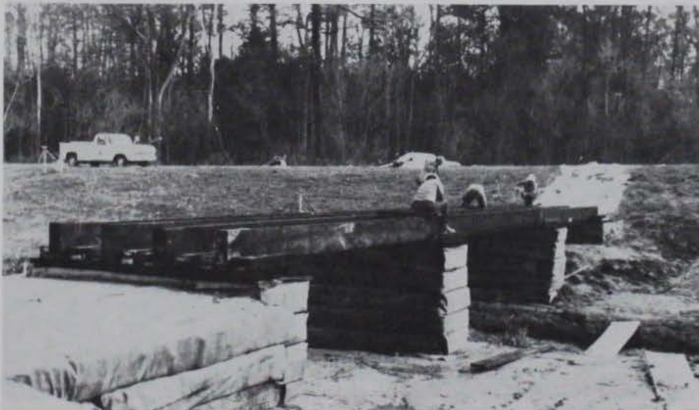
Photo 20. Stringers in place on supports
