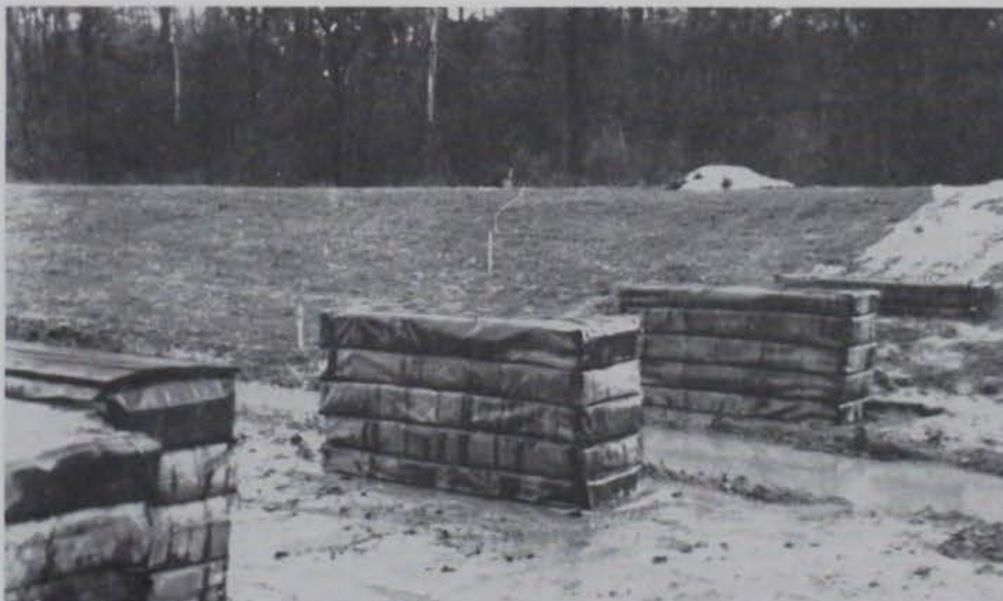
Photo 16. Completed layered supports
