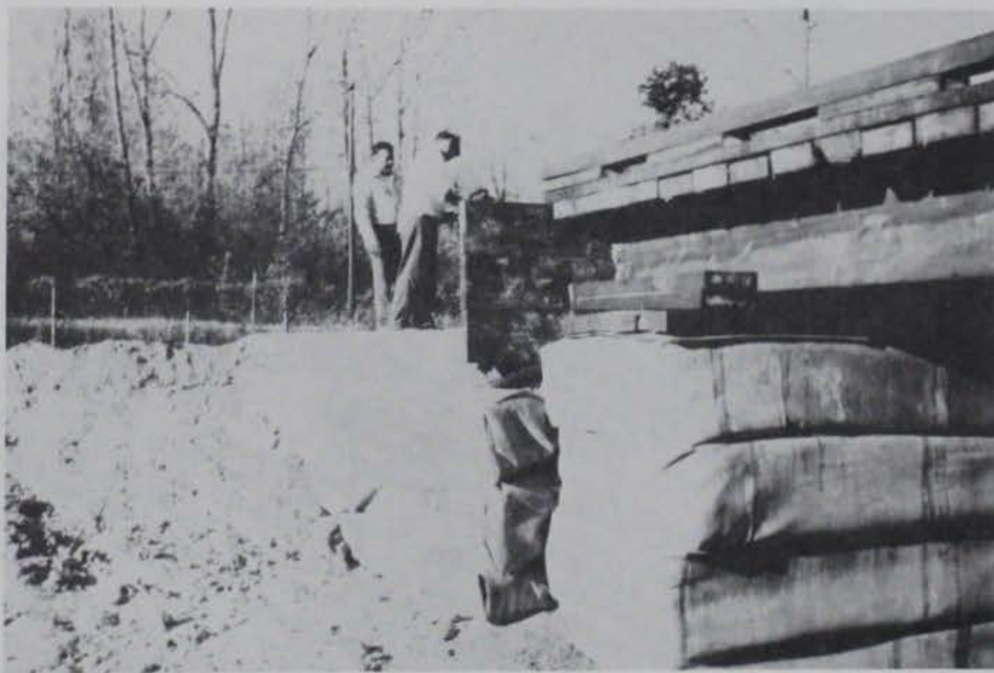
Photo 24. Layered approach construction north of support 4
