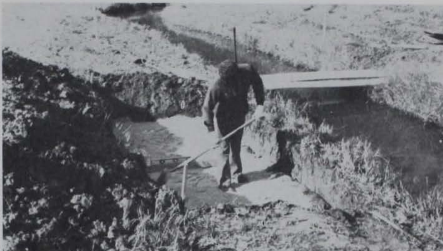
Photo 7. Leveling sand in excavation
