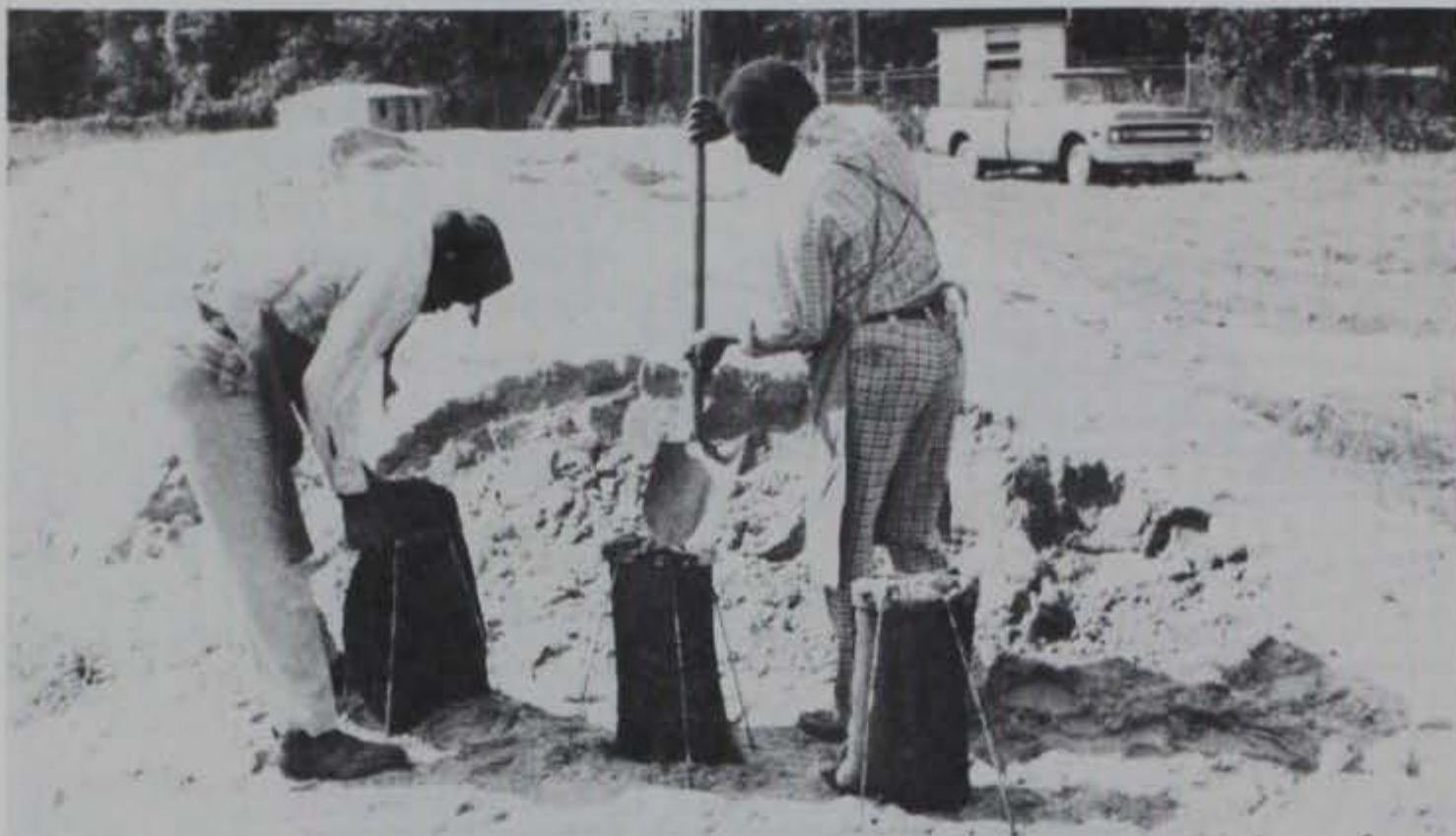
Photo 1. Filling sandbags
