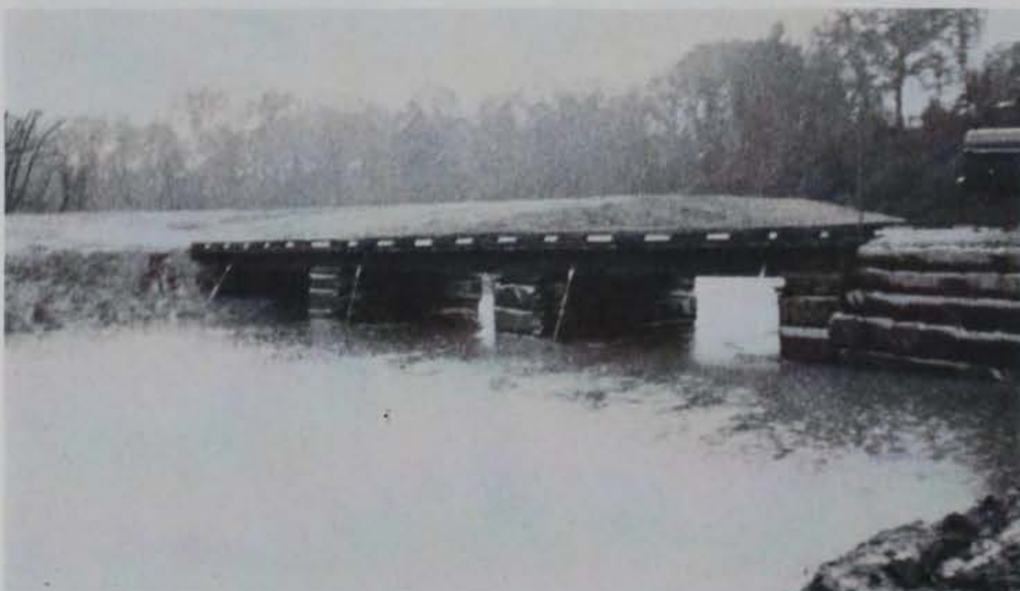
Photo 26. Completed bridge showing upstream cables
