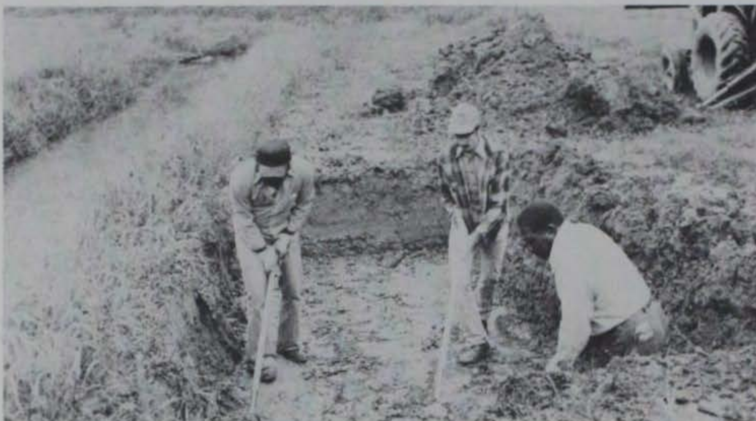
Photo 5. Finishing bottom of excavation
