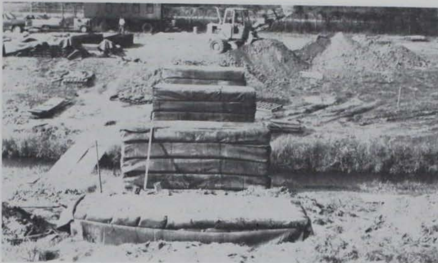
Photo 15. Partially built supports (support 1 open)
