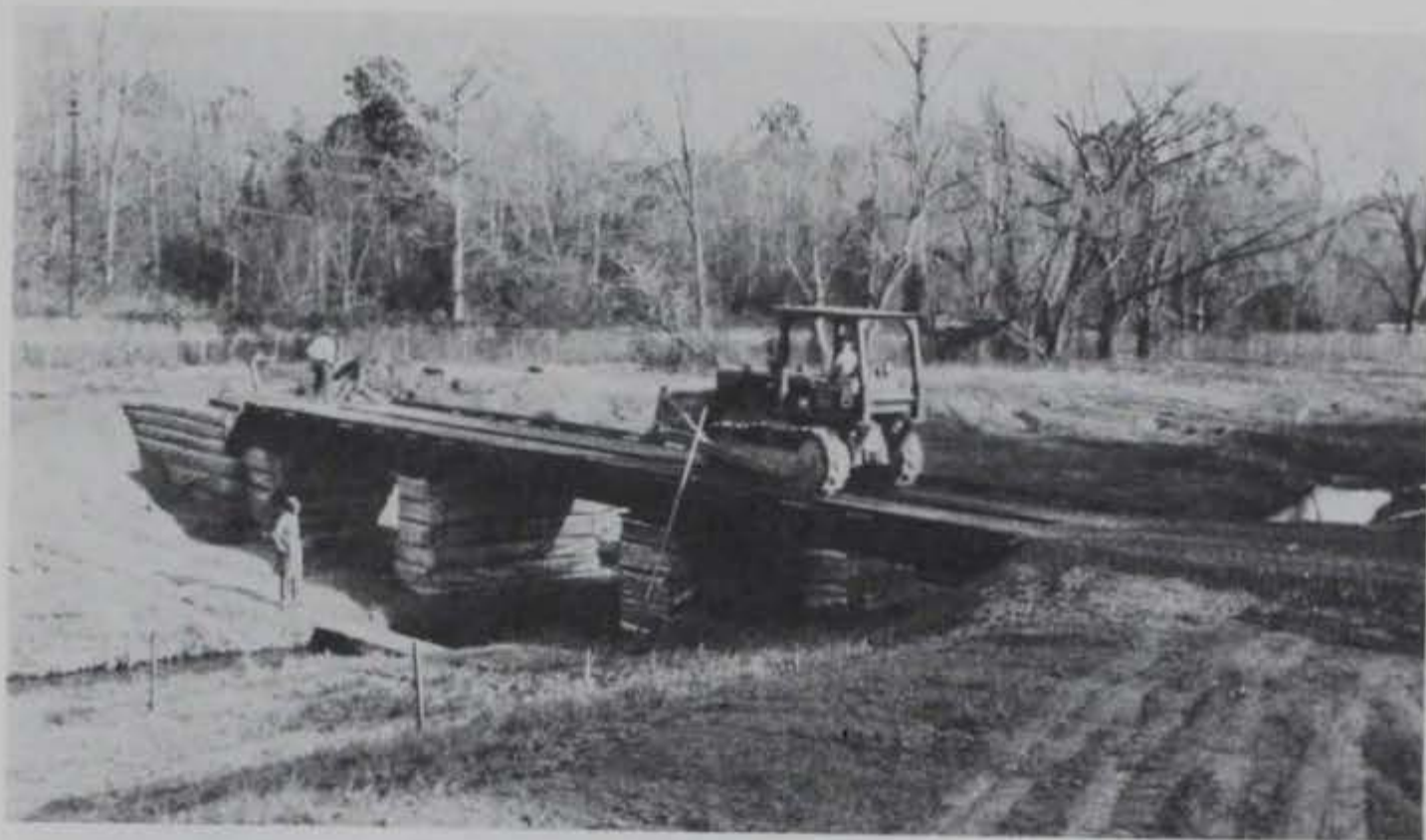
Photo 27. Seating superstructure on supports
