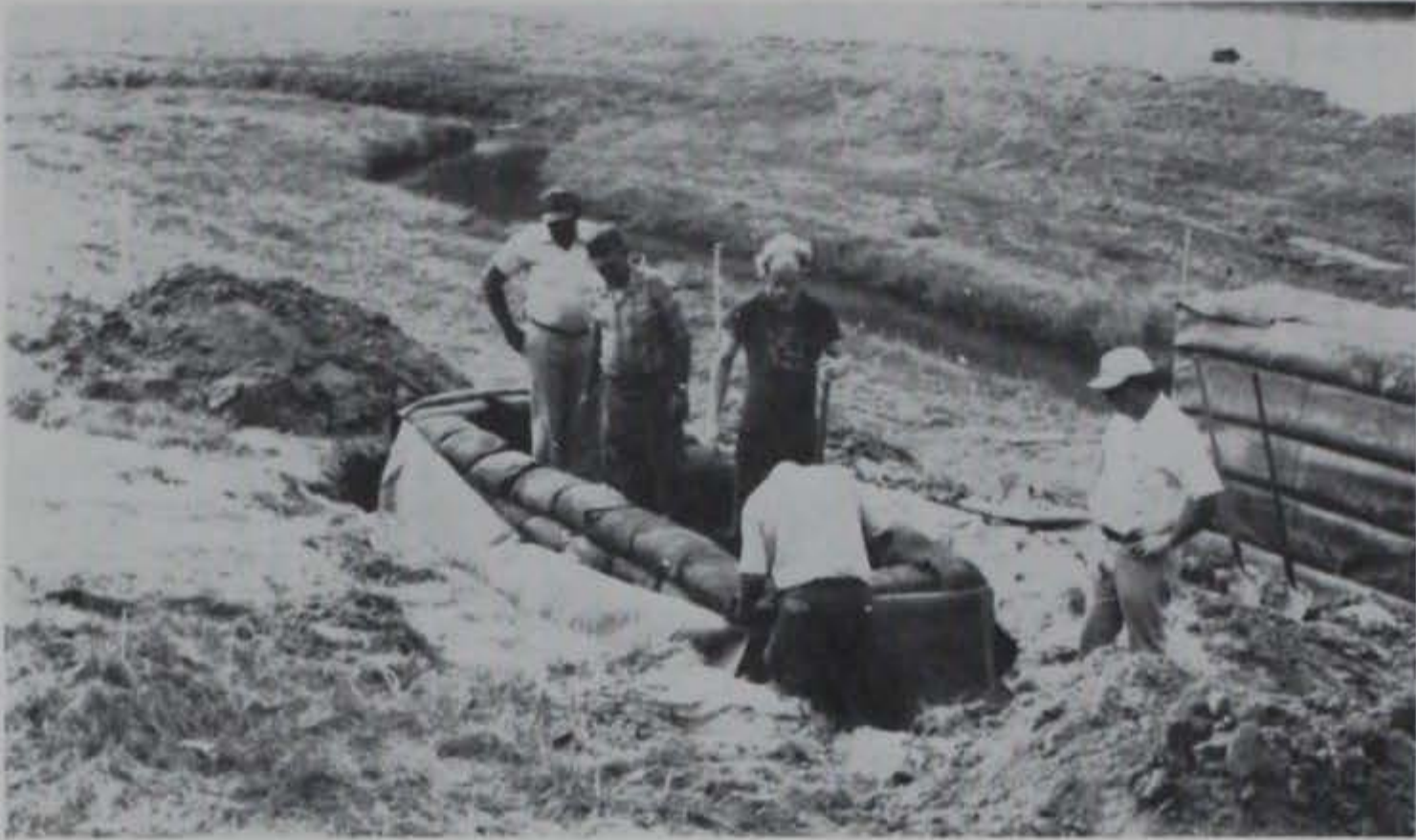
Photo 13. Upper support layer with sandbag form in place
