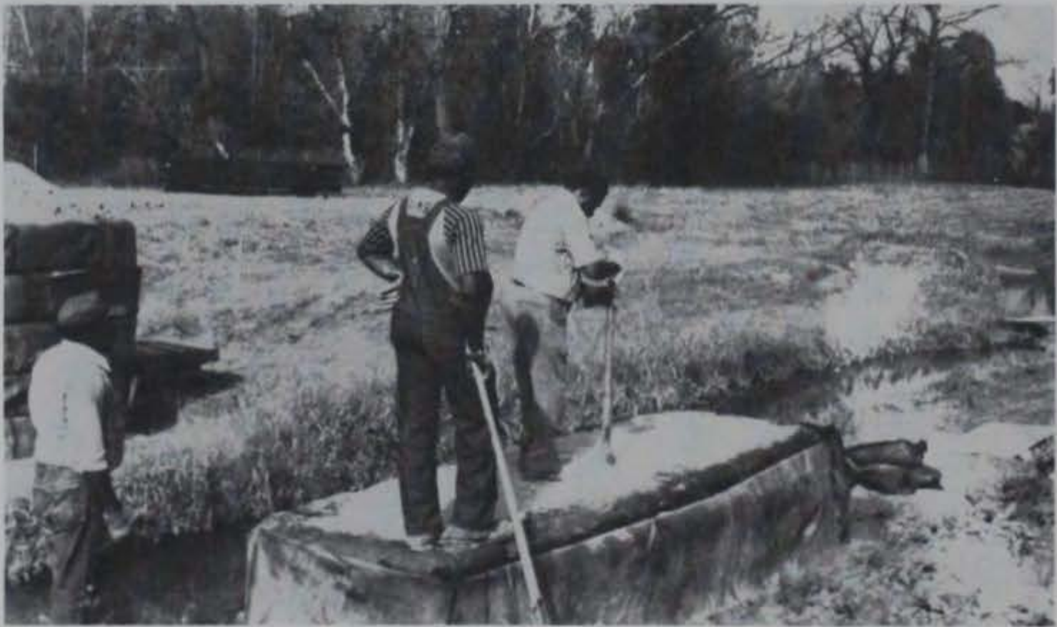
Photo 14. Hand compaction in upper layer
