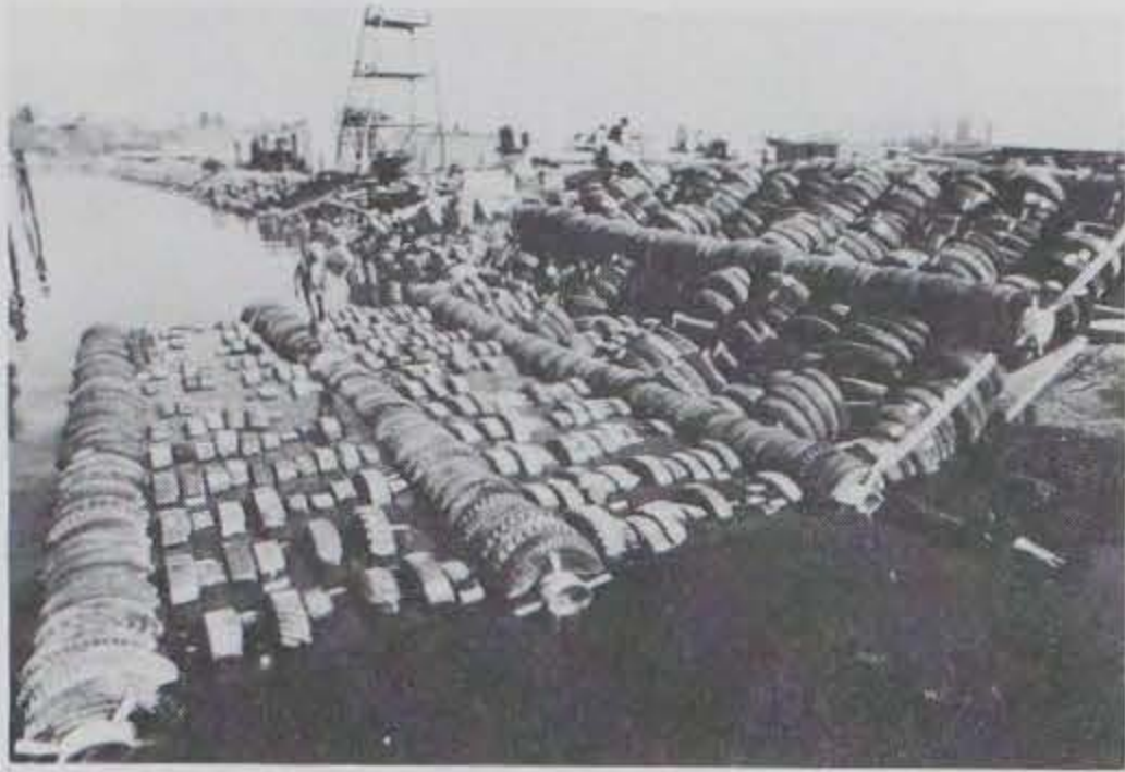
Photo 7. Assembling pipe-tire breakwater (Four modules are complete).
