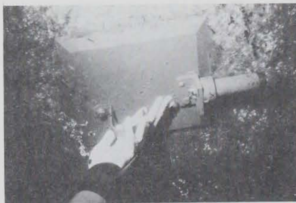
Photo F-6. Photo depicting pressure sensor on bottom of float.
