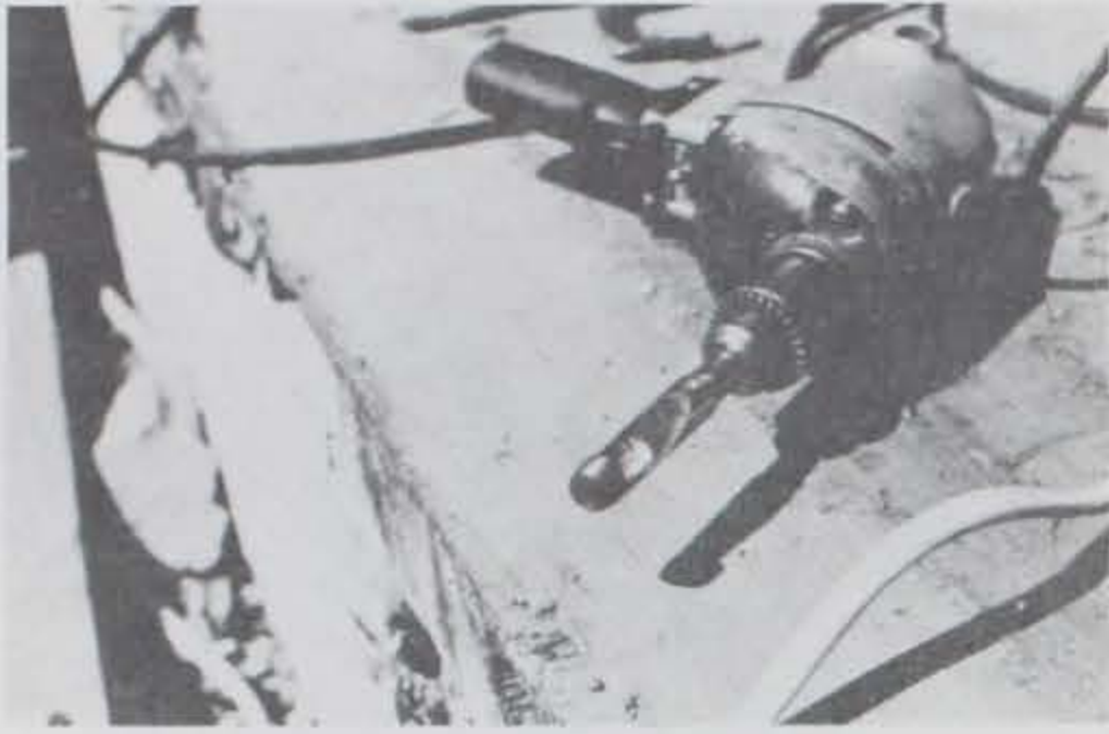
Photo B-13. Closeup showing a punch-shaped bit used to make holes in the tires and belting.
