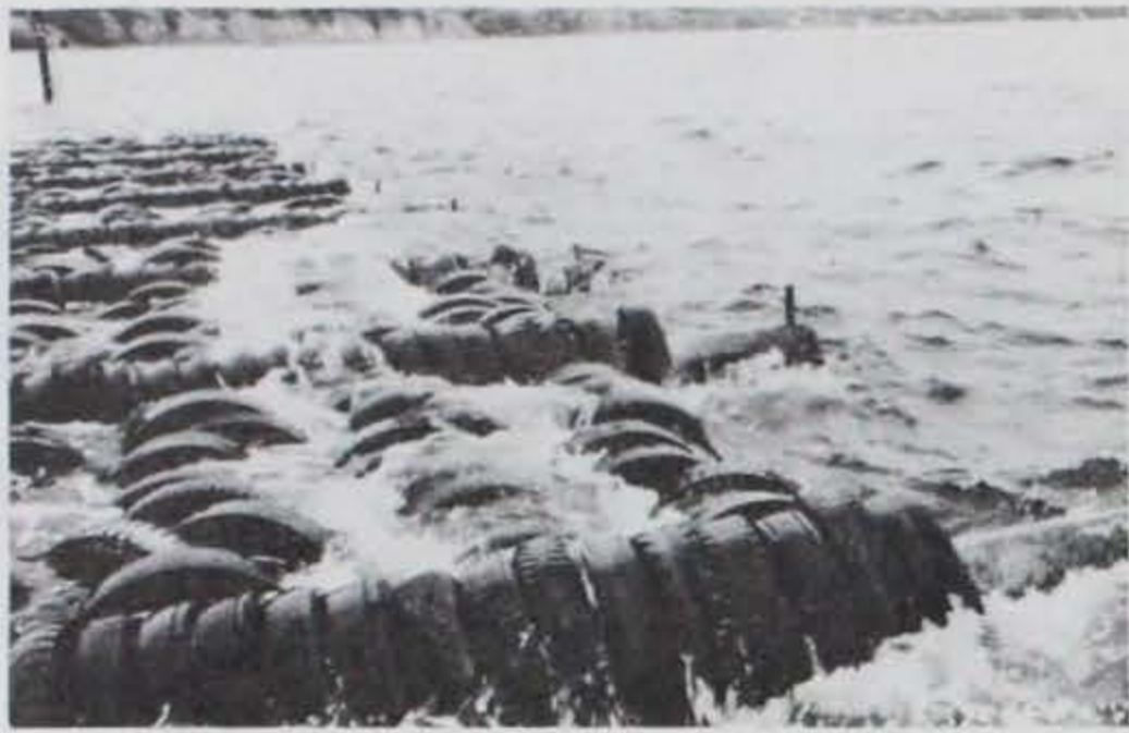
Photo B-25. Wave action compressing the tires on the pipes.
