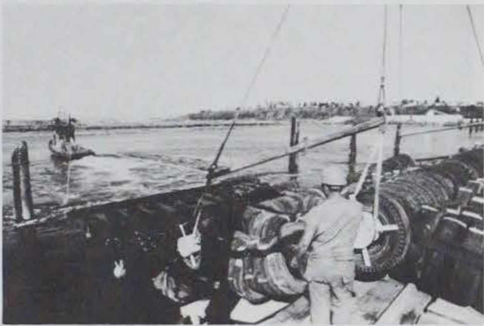
Photo B-21. Launching of completed pipe-tire breakwater.
