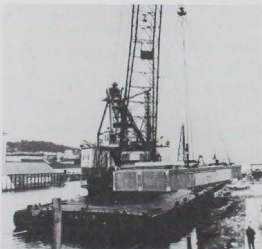
Photo 5. Launching of concrete breakwater.
