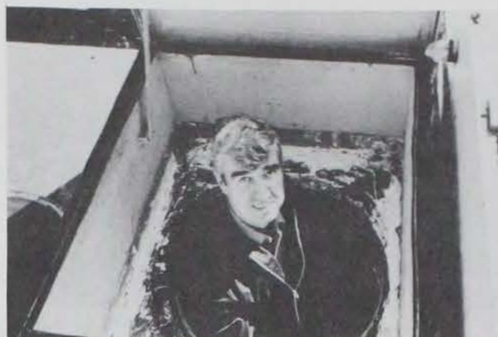
Photo F-14. Photo showing secondary hatch to keep waves from washing into the equipment compartment.
