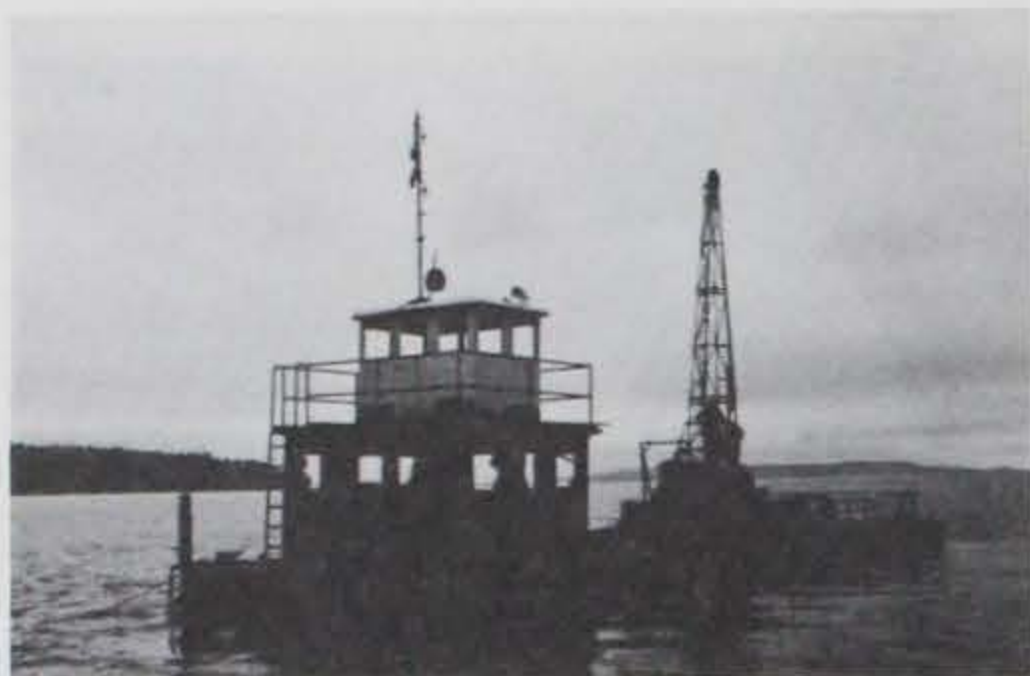
Photo C-7. Drill barge taking bore samples at the test site.
