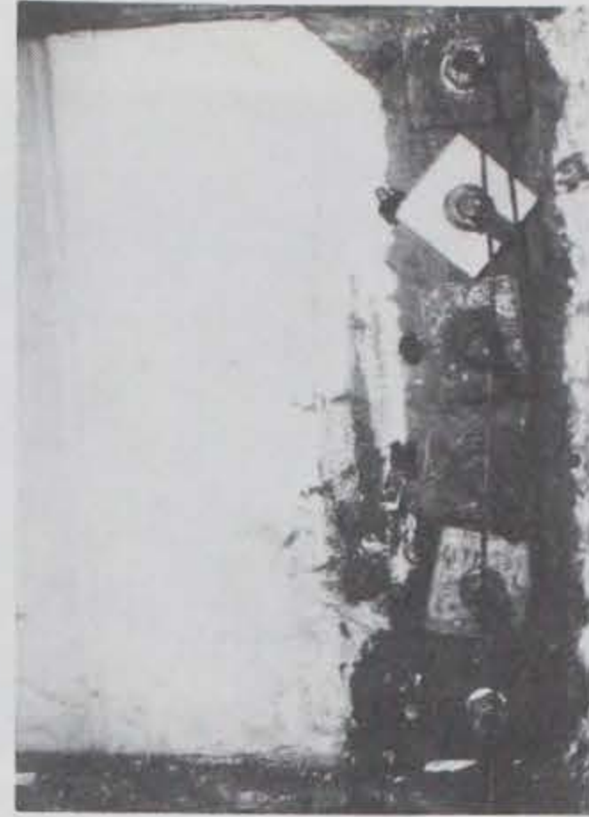
Photo D-20. Photo depicting inside of float with six tensioned bars near sidewall.
