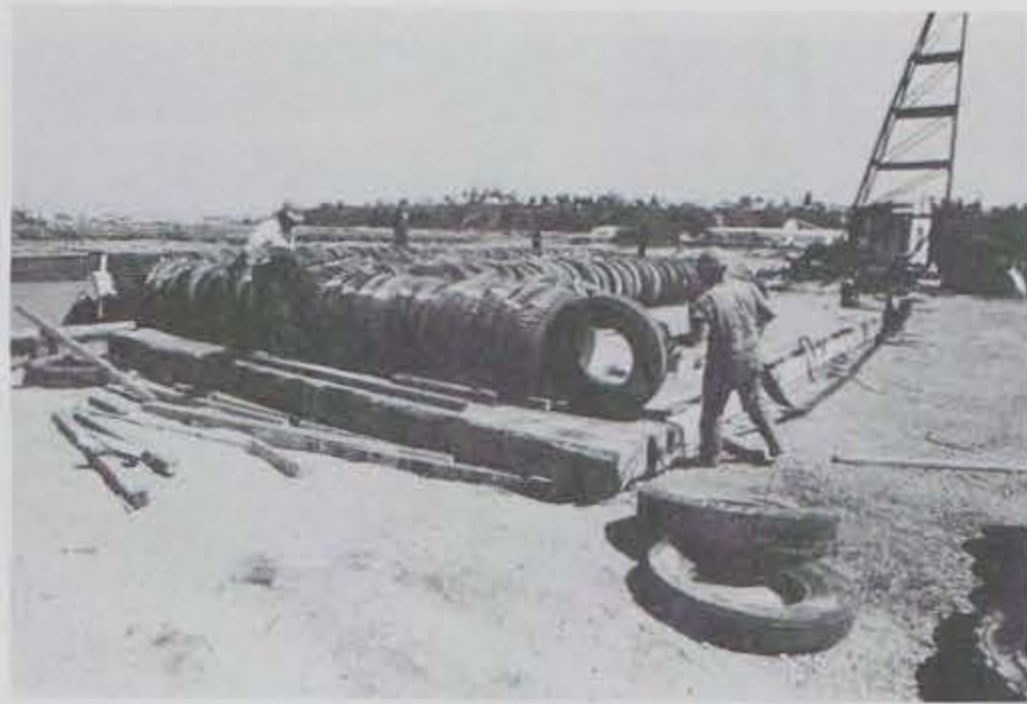
Photo 8. Assembling a module.
