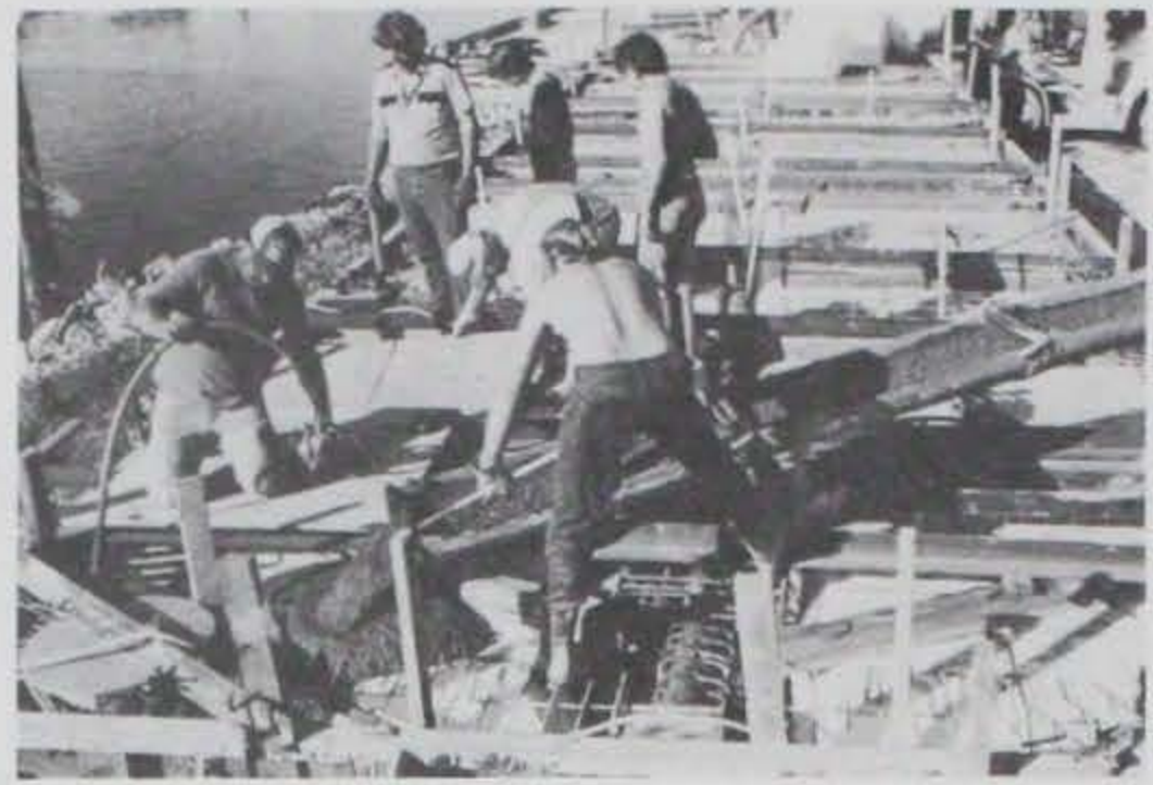
Photo 2. Placing concrete in sides and internal walls.
