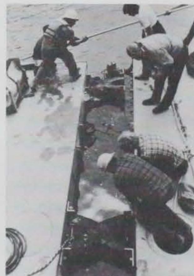
Photo 6. Joining units with flexible connectors.
