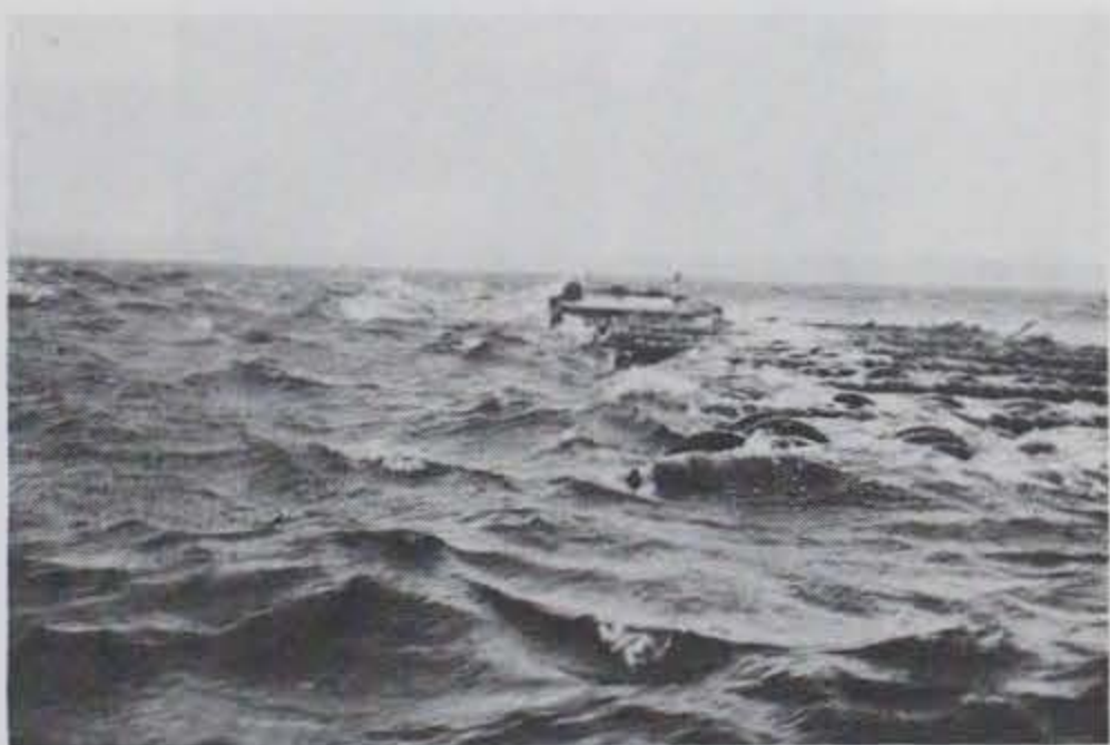
Photo B-23. 1.5-ft-high waves washing onto the pipe-tire wave breakwater.
