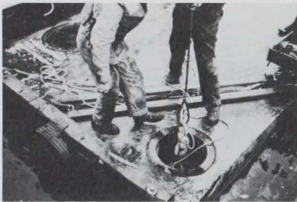
Photo C-33. A quick-release hook being used for the third and final unanchoring.
