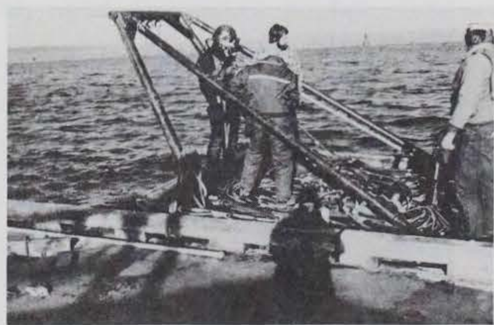
Photo C-30. Utilizing divers to simplify the second reanchoring.
