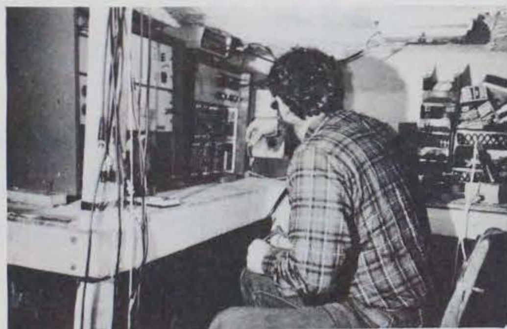
Photo F-17. Working under adverse conditions inside the float.
