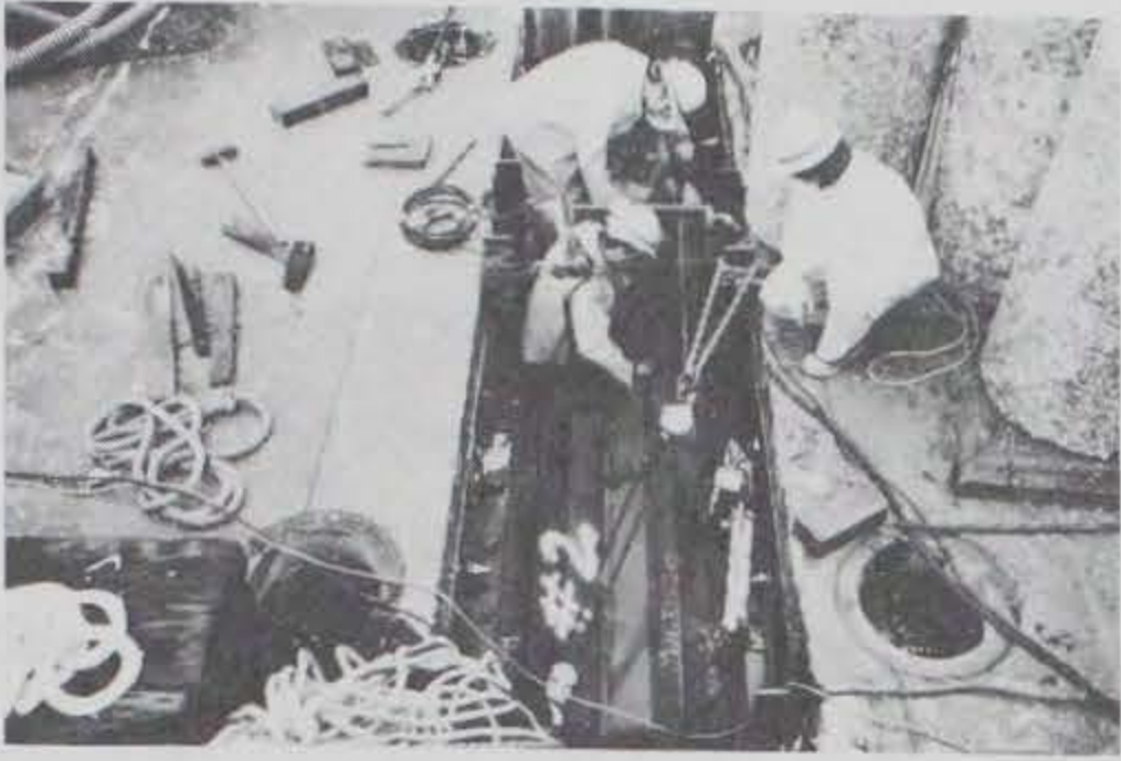
Photo D-31. New flexible connectors being "coaxed" into position.
