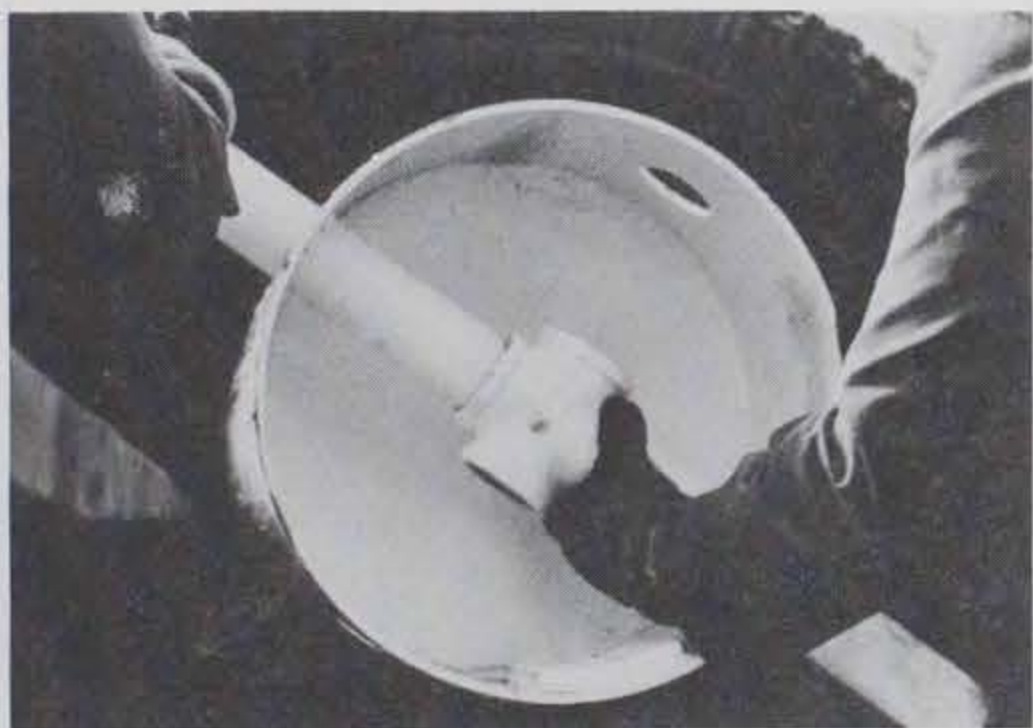
Photo 11. Keeper pipes being secured (welding of keepers required to prevent loosening).
