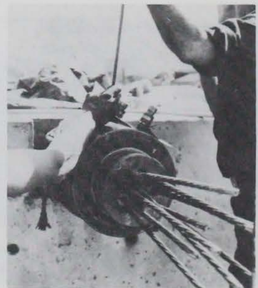
Photo A-12. Preparing for post-tensioning.
