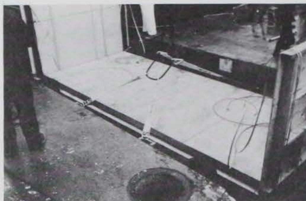
Photo D-14. Cofferdam being lowered between the floats.
