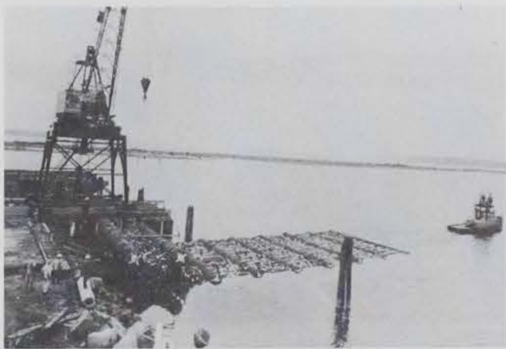
Photo 12. Launching of pipe-tire breakwater.
