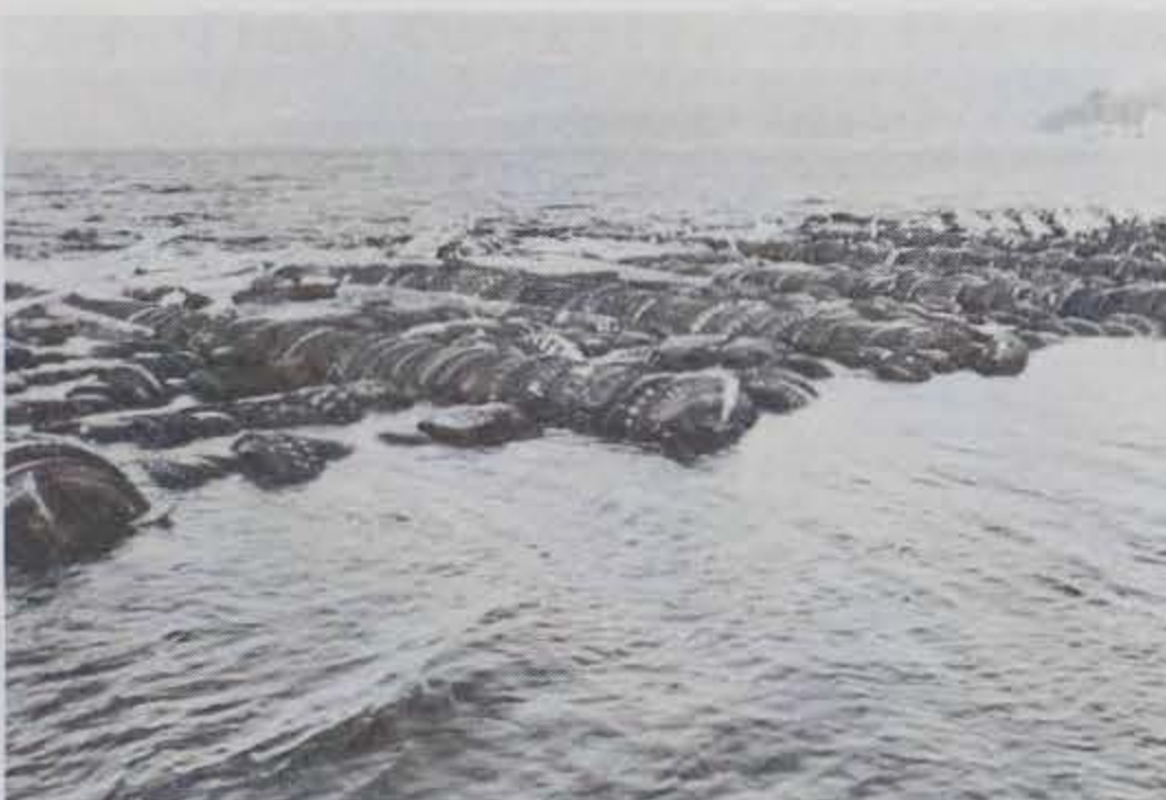
Photo 23. Pipe-tire breakwater after having weathered numerous storms.
