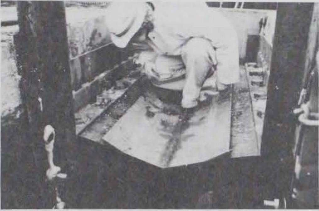
Photo D-33. Horizontal flexible connector being inspected.
