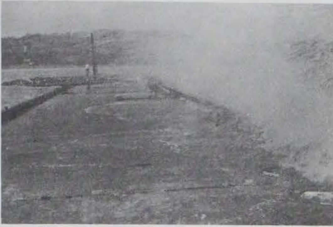
Photo 19. 1.5-ft waves overtopping the concrete breakwaters.
