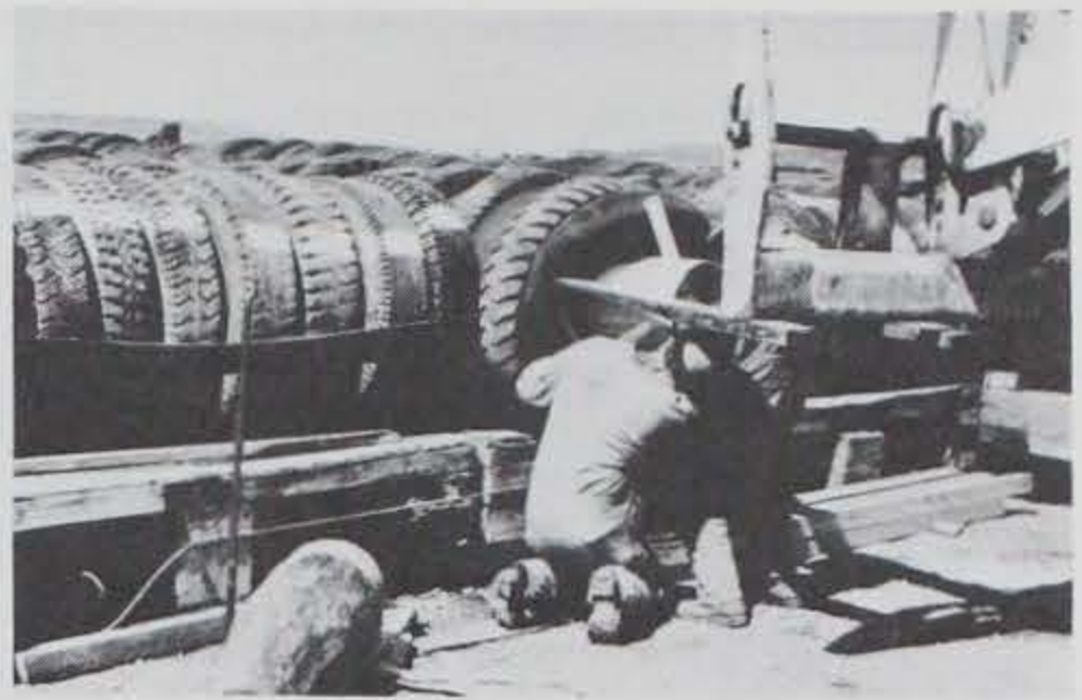
Photo B-20 Securing the keeper pipes.
