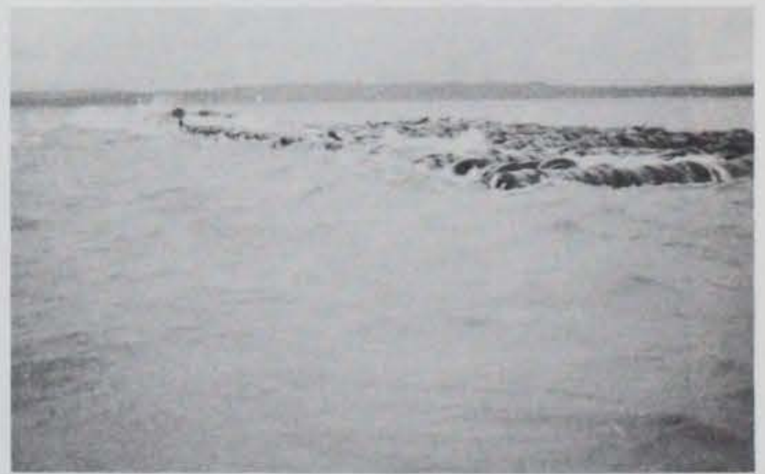
Photo 18. Waves reflecting from windward side of concrete float.
