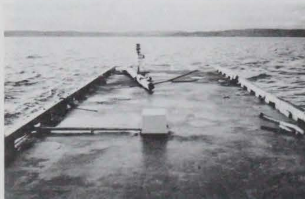
Photo A-24. Photo showing type of debris which washed across the deck.
