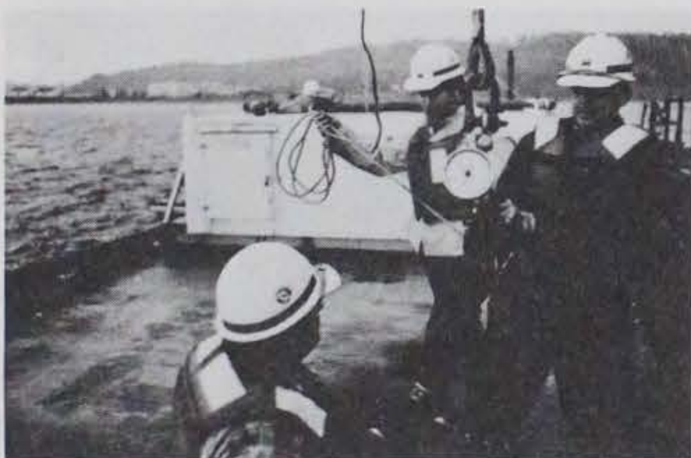
Photo C-29. Anchor line tension being measured during the unanchoring procedure.
