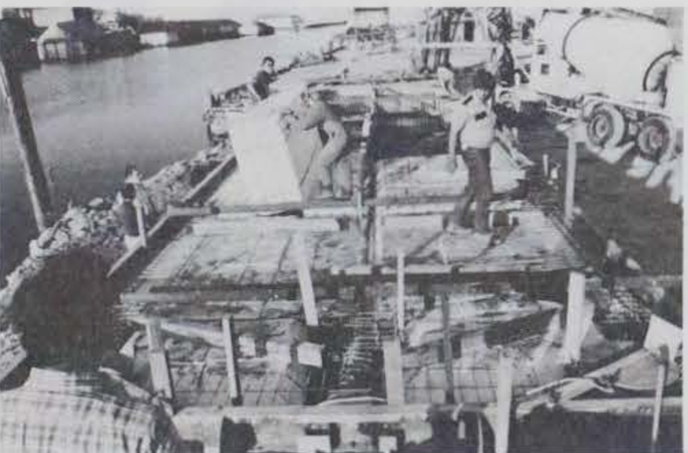
Photo A-5. Styrofoam being lowered after bottom of float was placed.
