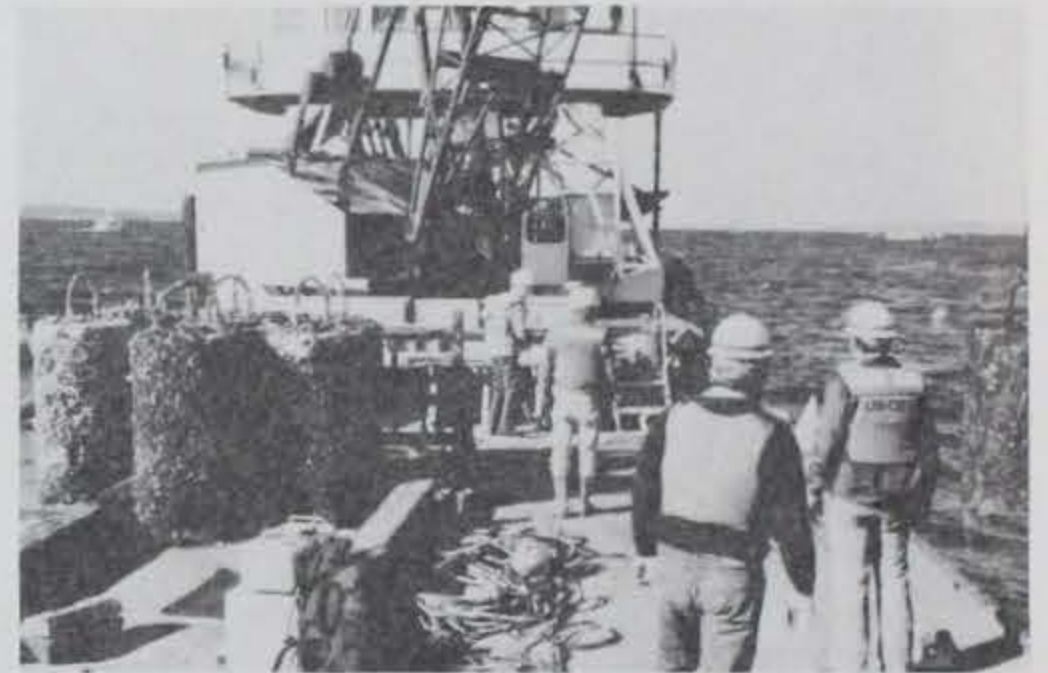
Photo C-22. Removing clump weights (note numerous marine organisms attached to the weights).
