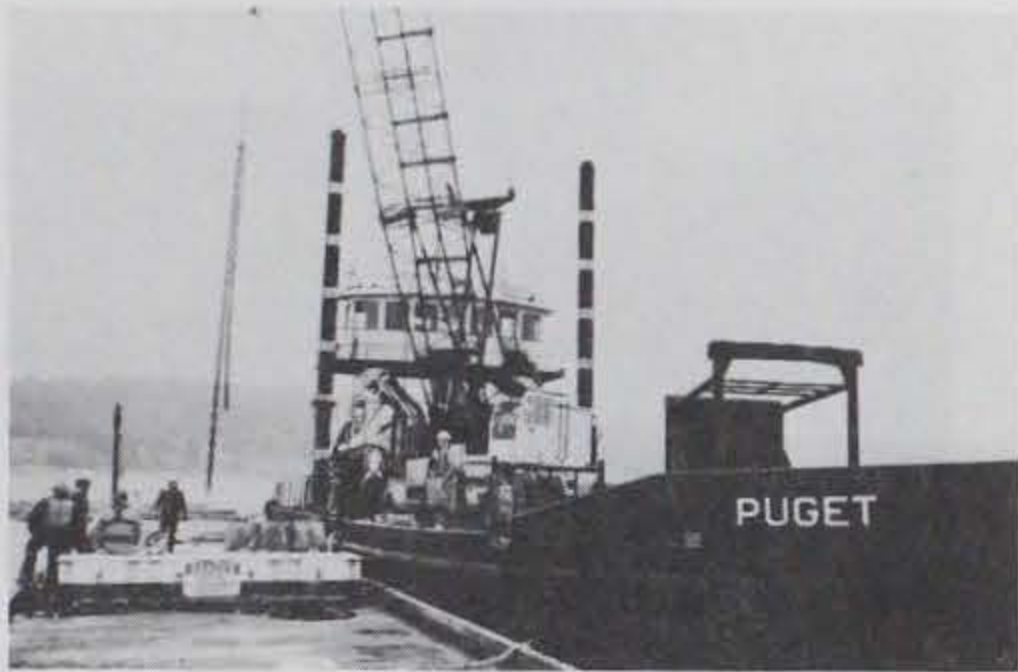
Photo C-15. A new anchor chain being readied for installation.
