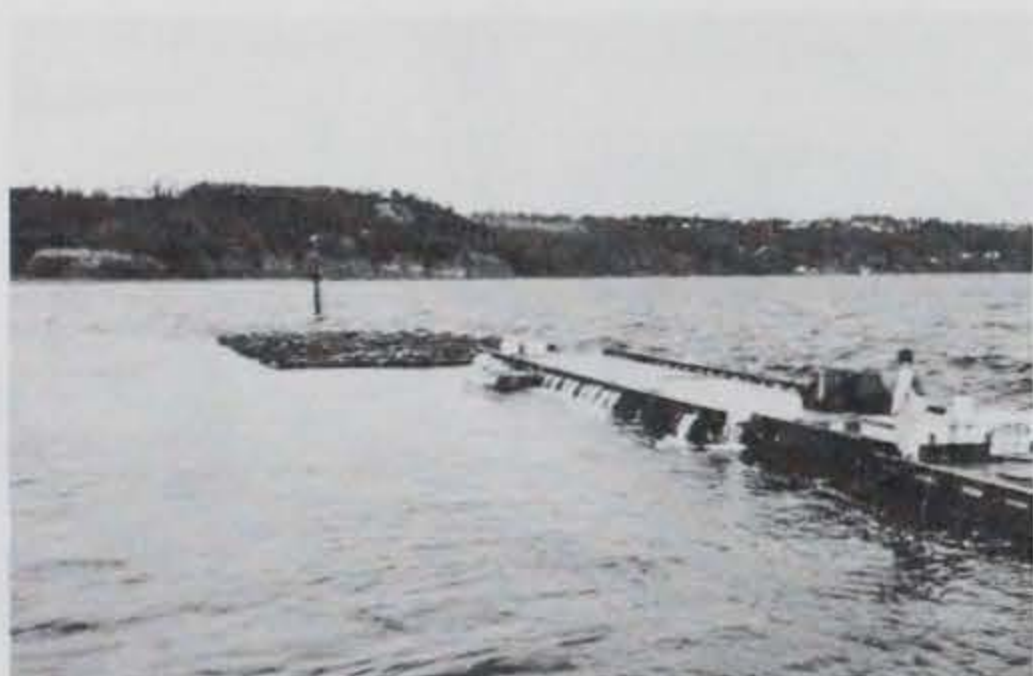
Photo A-21. Overtopping waves swamping a work skiff.
