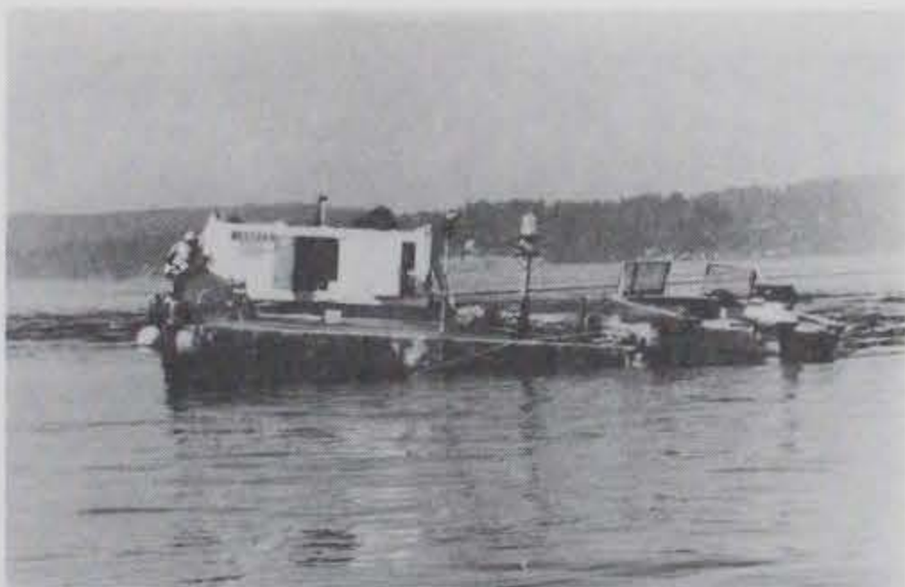
Photo C-17. The concrete breakwater tipping in response to the tug's pull.
