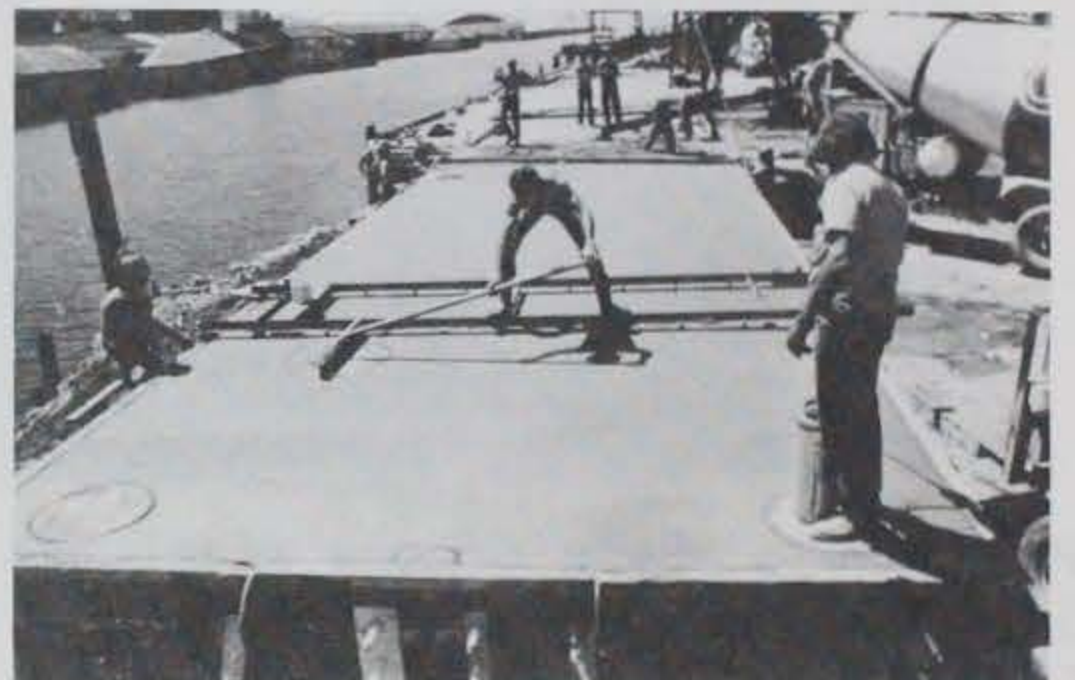
Photo A-10. Using a broom to create a nonskid surface.
