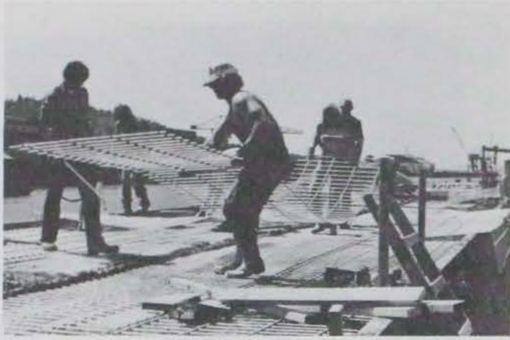
Photo A-7. 3/8-in. welded wire fabric being laid on the deck.
