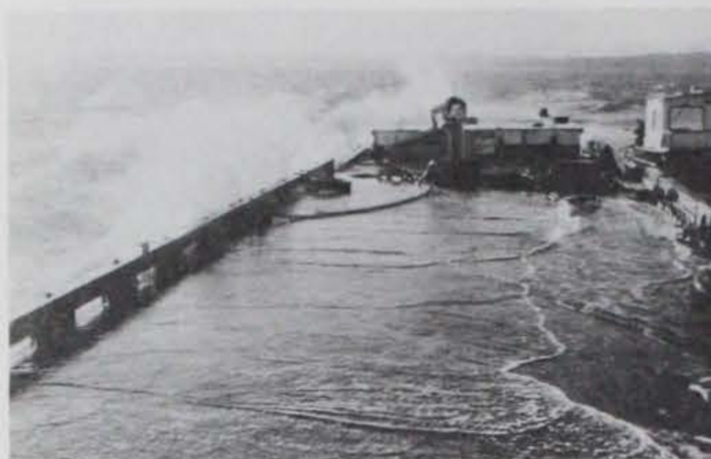
Photo A-20. Work continuing cautiously on the slippery, rolling deck.
