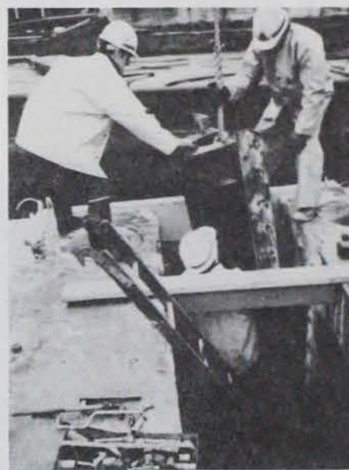
Photo D-16. Fender system hardware being removed.
