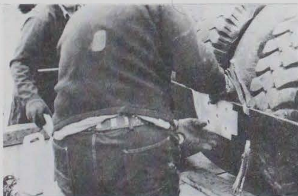
Photo B-11. Marking the hole pattern on the belting.
