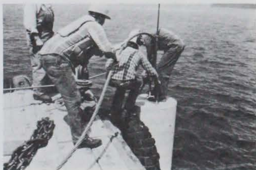
Photo C-11. Attaching clump weights to the concrete breakwater's anchor lines.
