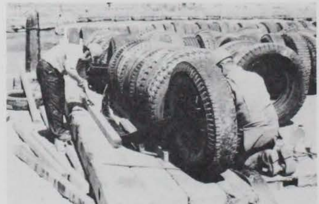
Photo B-6. Belting being placed around the first row of tires.
