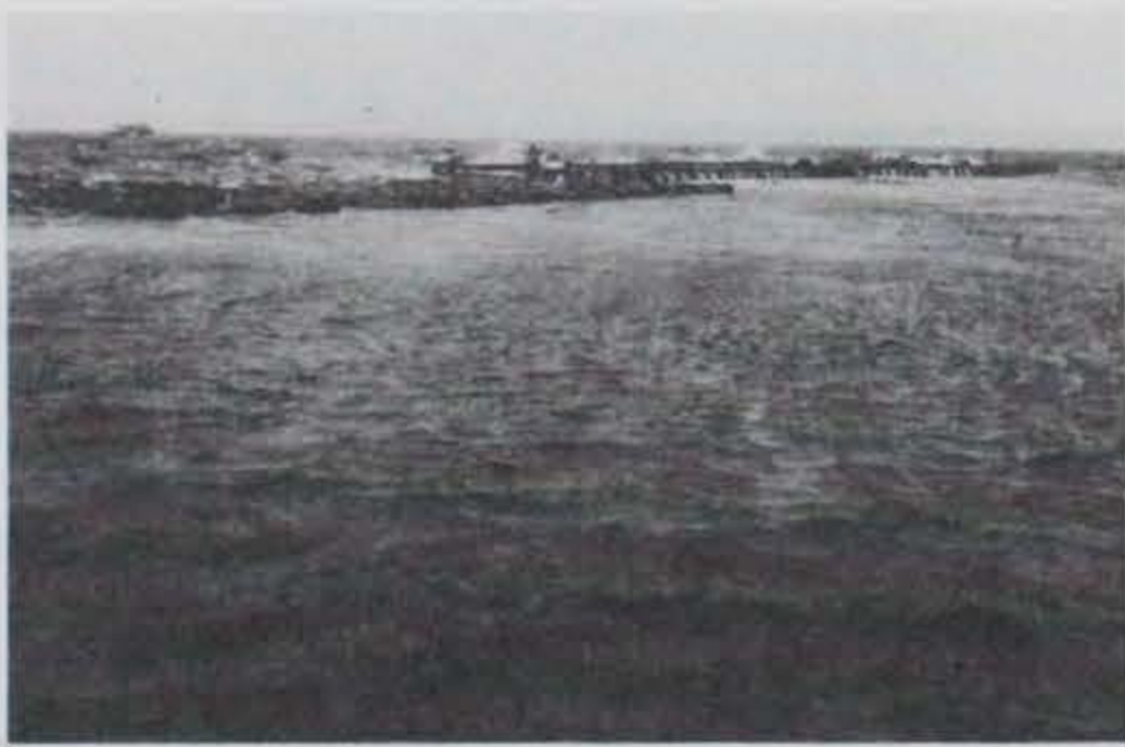
Photo 17. Example of both breakwaters providing good protection from storm waves.
