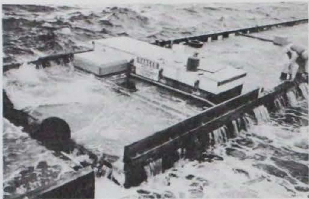
Photo A-19. Waves overtopping the low deck (13-in.) freeboard allowing considerable wave overtopping.
