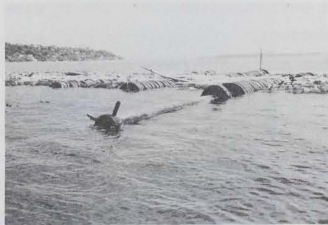
Photo 24. A broken longitudinal pipe pulling out of the tires.
