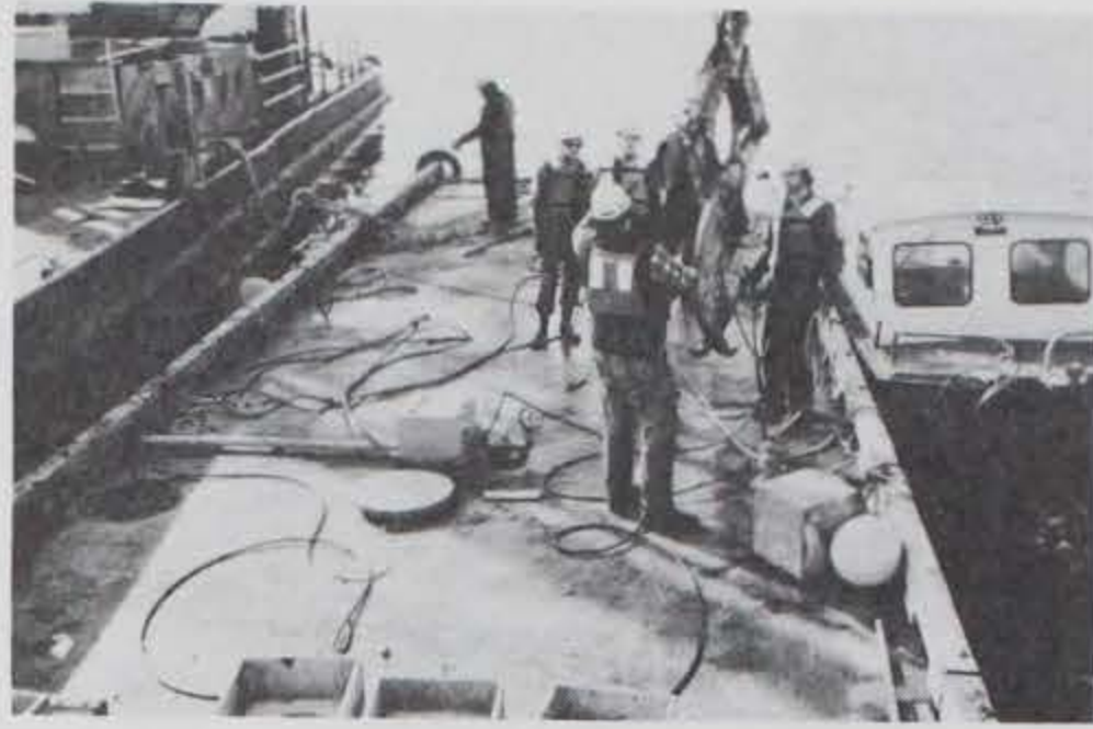
Photo C-26. Encountering some difficulties during the first reanchoring operation.
