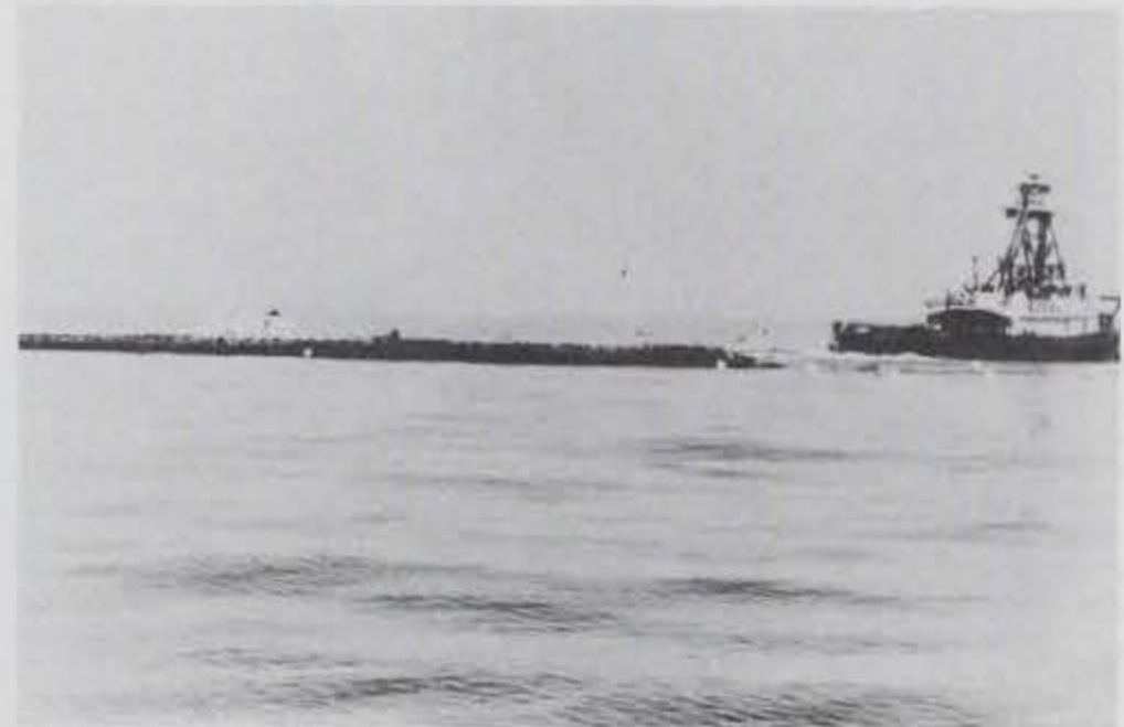
Photo C-16. Tugboat pulling to determine anchor line stiffness.
