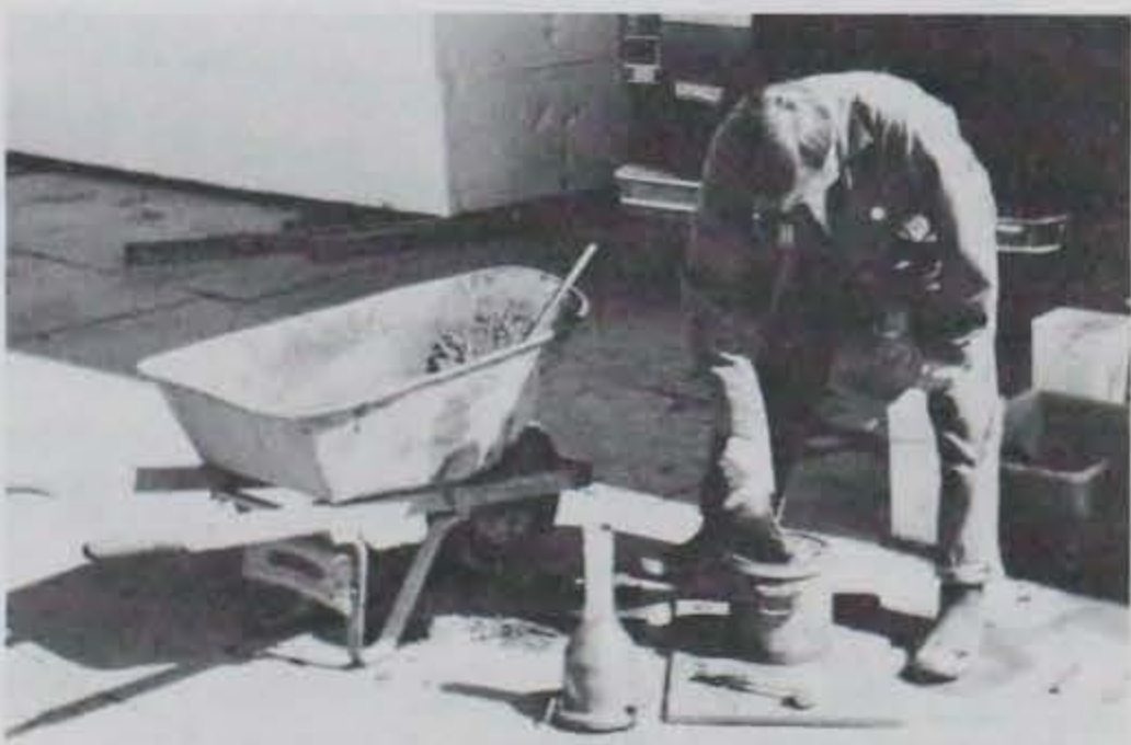
Photo A-11. Taking concrete samples (done throughout the placement).
