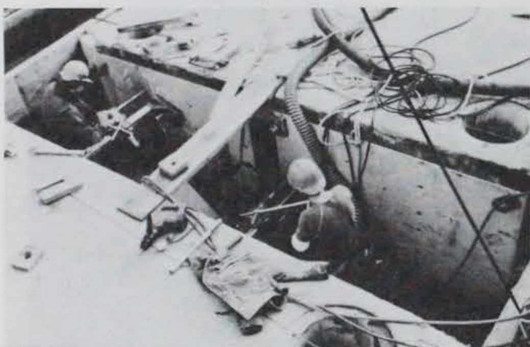
Photo D-27. Additional bolt holes being drilled in floats.
