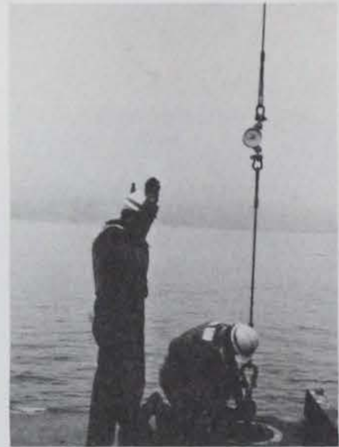
Photo C-34. Removing the keeper plate prior to dropping the anchor line.
