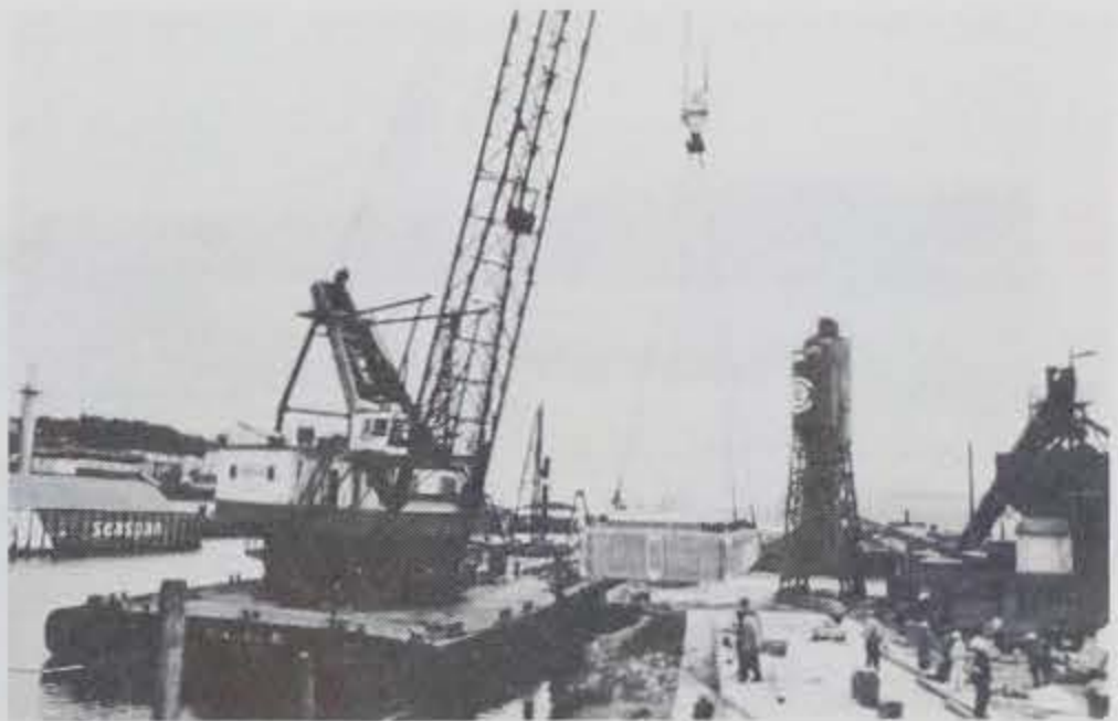
Photo A-16. A large derrick lifting one of the 140-ton floats.
