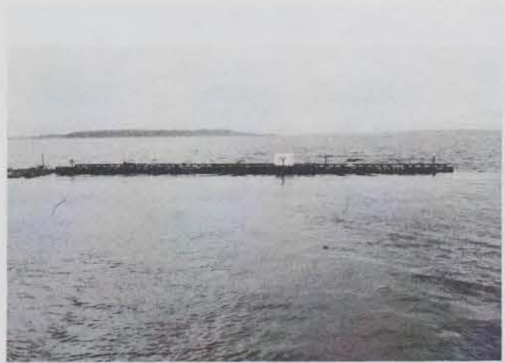
Photo D-24. Resuming monitoring of rigidly connected breakwater.
