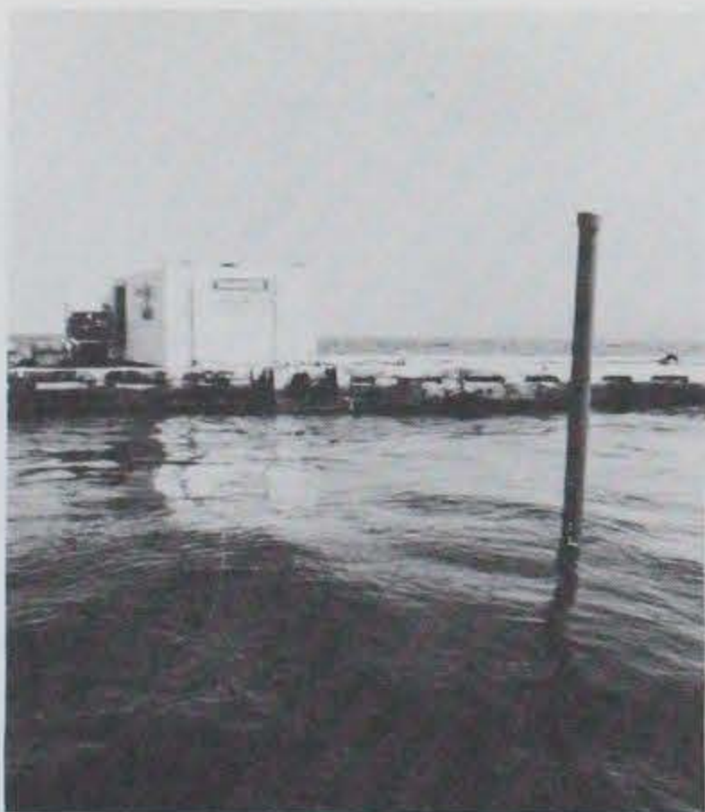
Photo 29. Photo showing the deckhouse that protected equipment from the elements (wave buoy in foreground).
