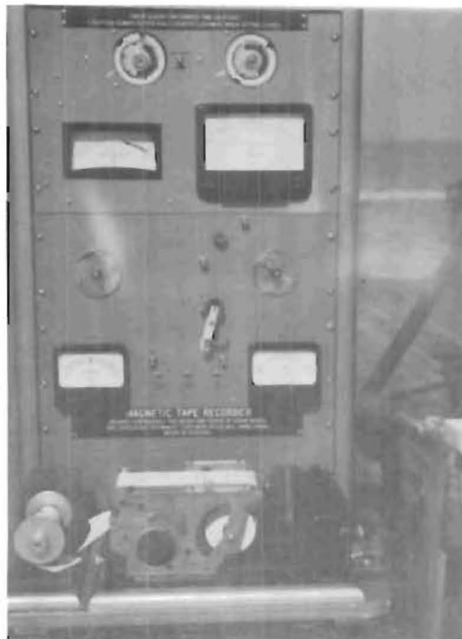
Figure 5 - Cabinet Containing Both Paper Tape and Magnetic Tape Recorders
