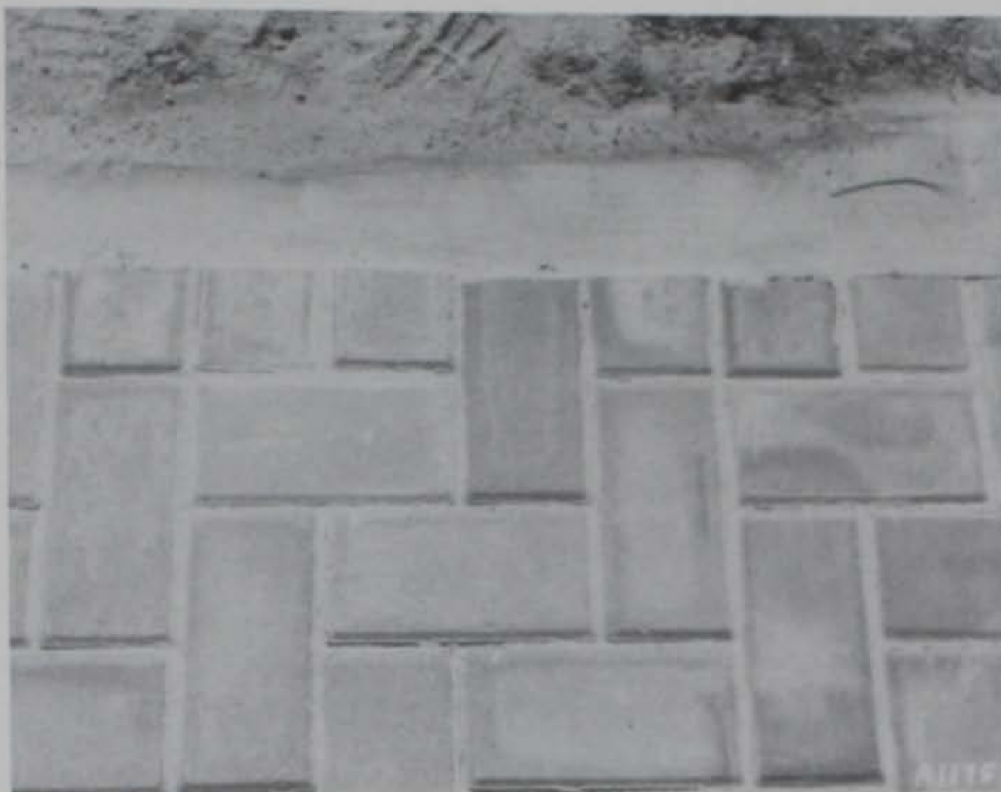
Figure 23. Trimmed edge of block pavement with jointing sand
