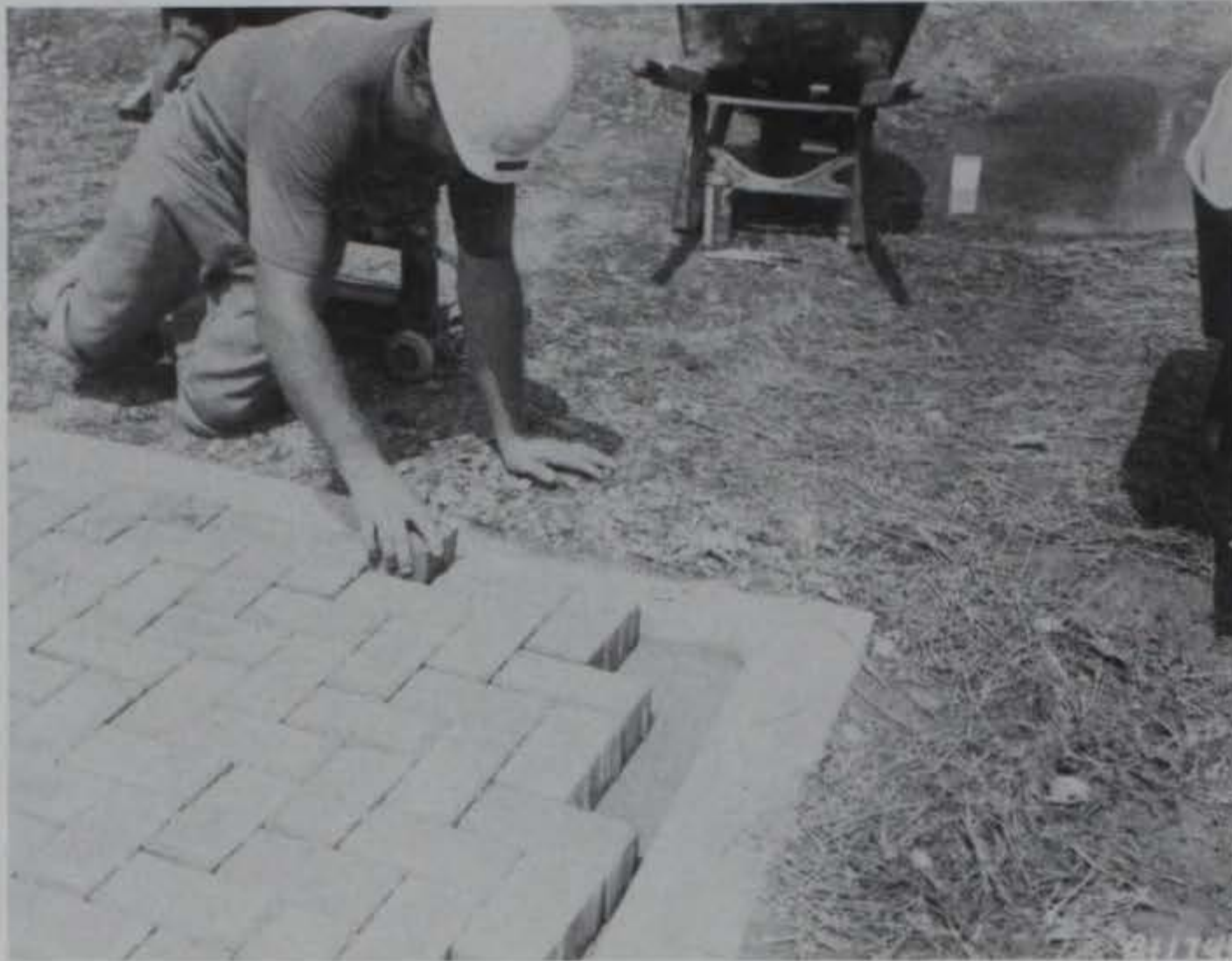
Figure 21. Trimming in pavement edge with cut block
