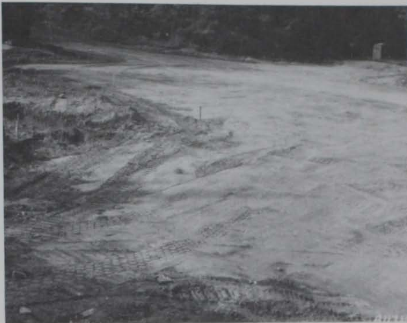
Figure 7. Compacted subgrade
