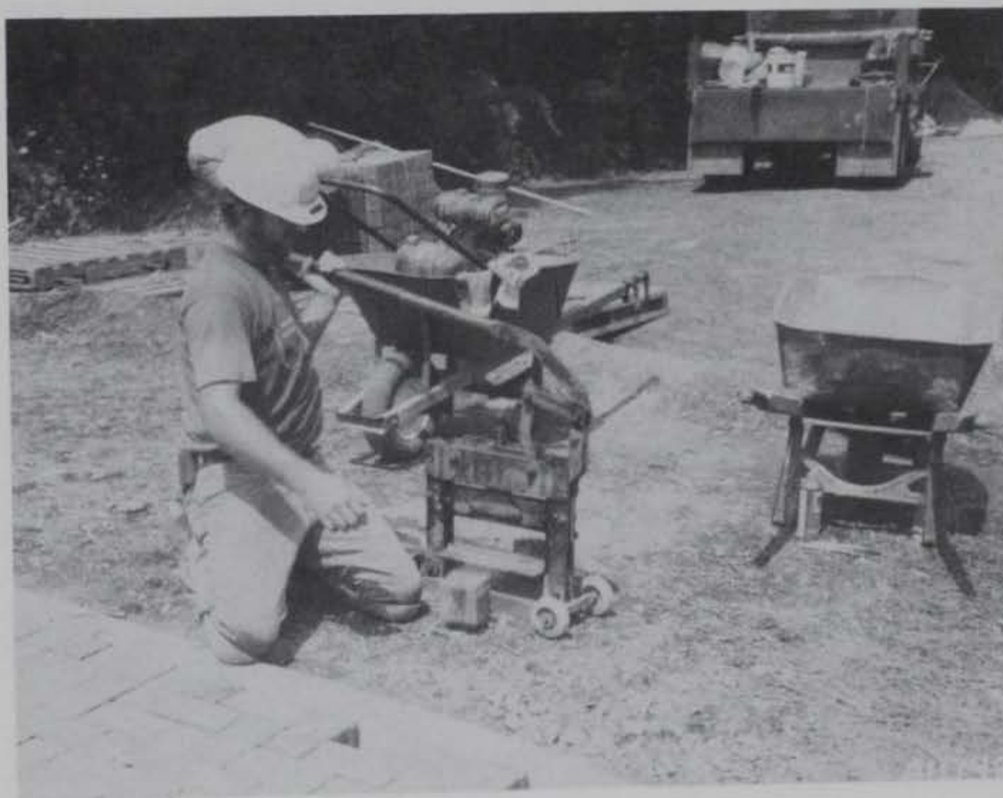
Figure 20. Cutting paving block with hand splitter
