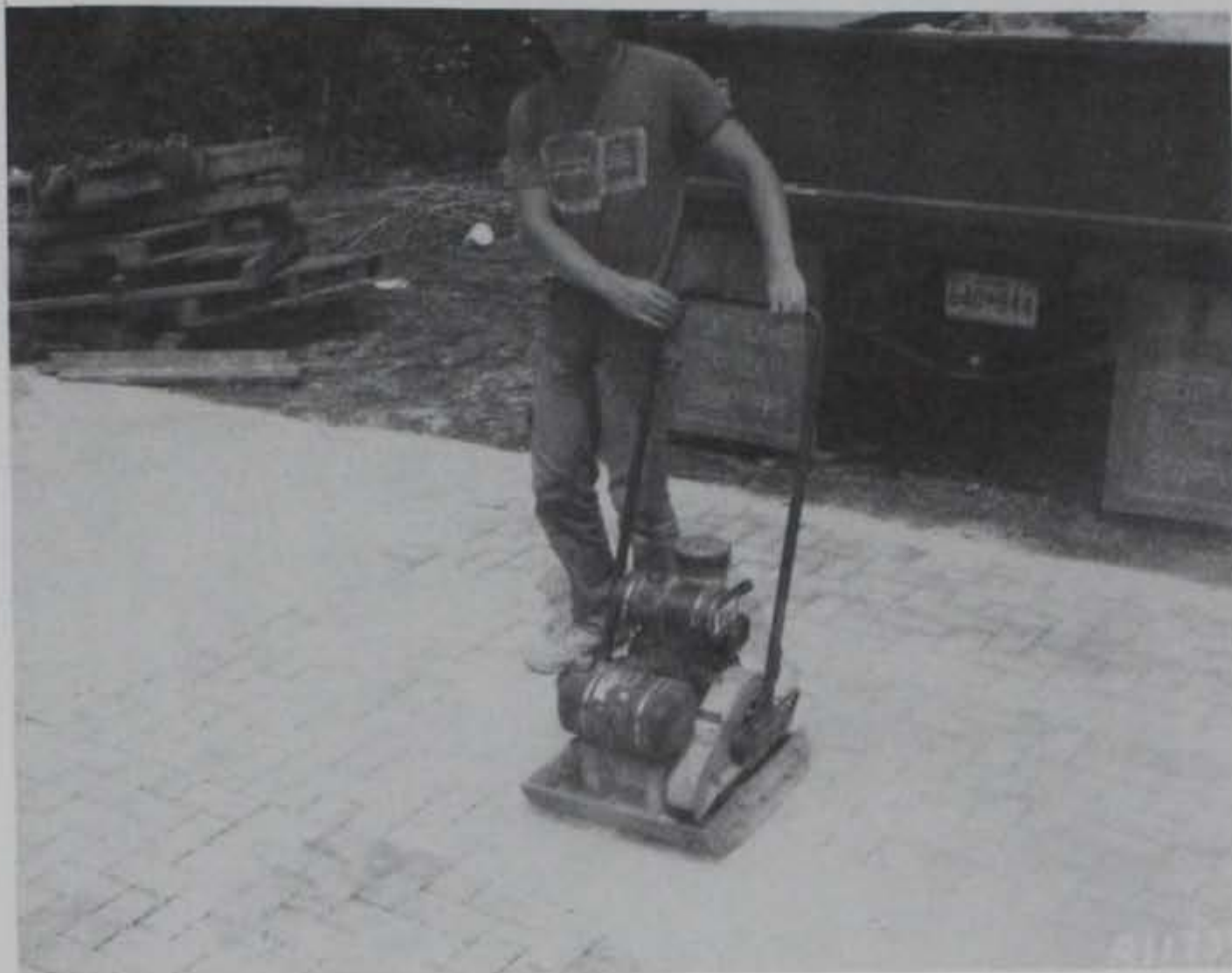
Figure 19. Vibrating jointing sand into paving block joints
