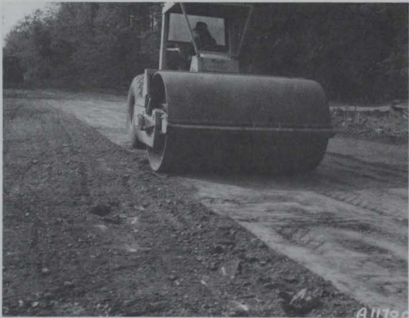
Figure 10. Recompactng select-fill subbase
