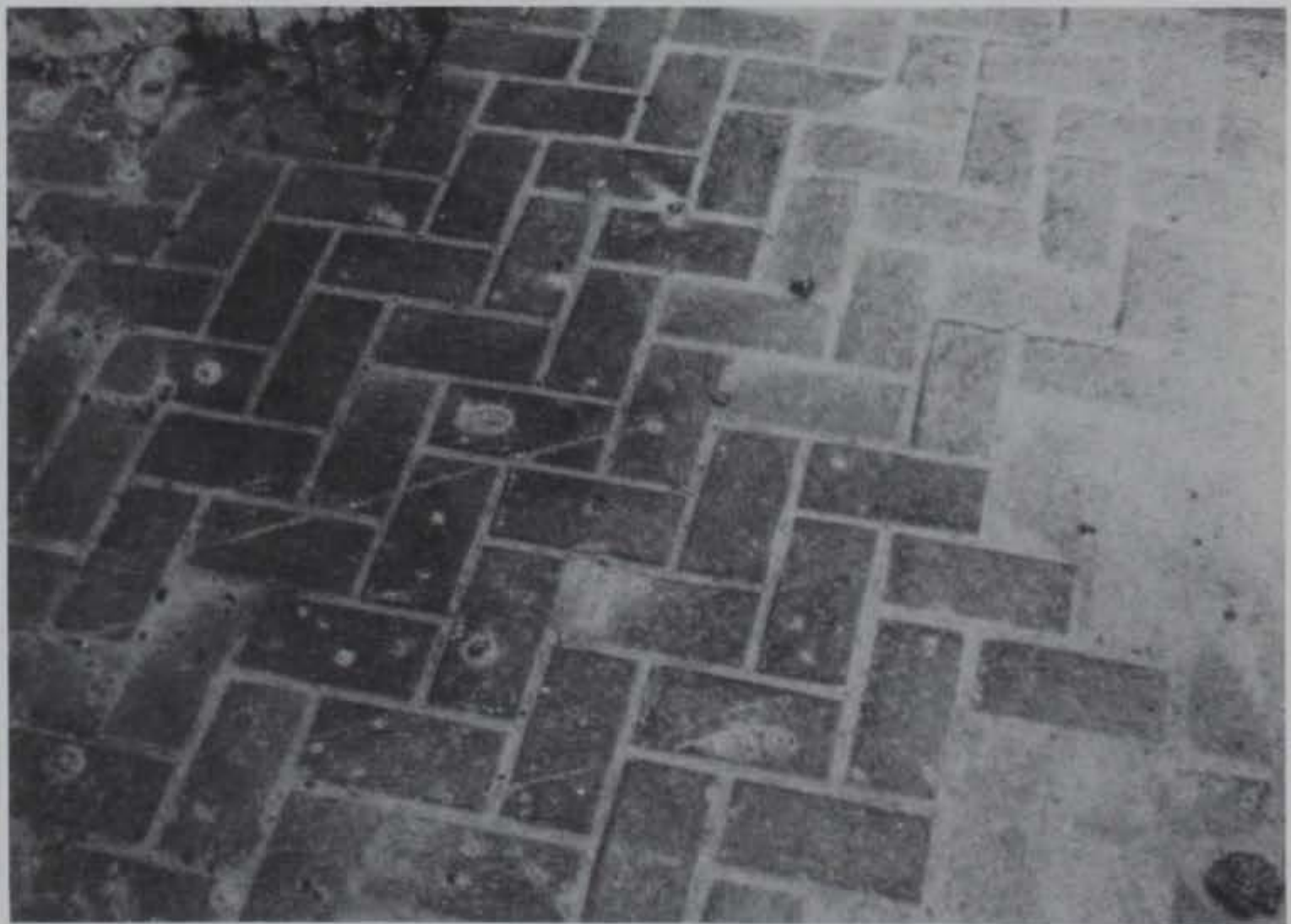
Figure 30. Close-up of block pavement after 1 year of service
