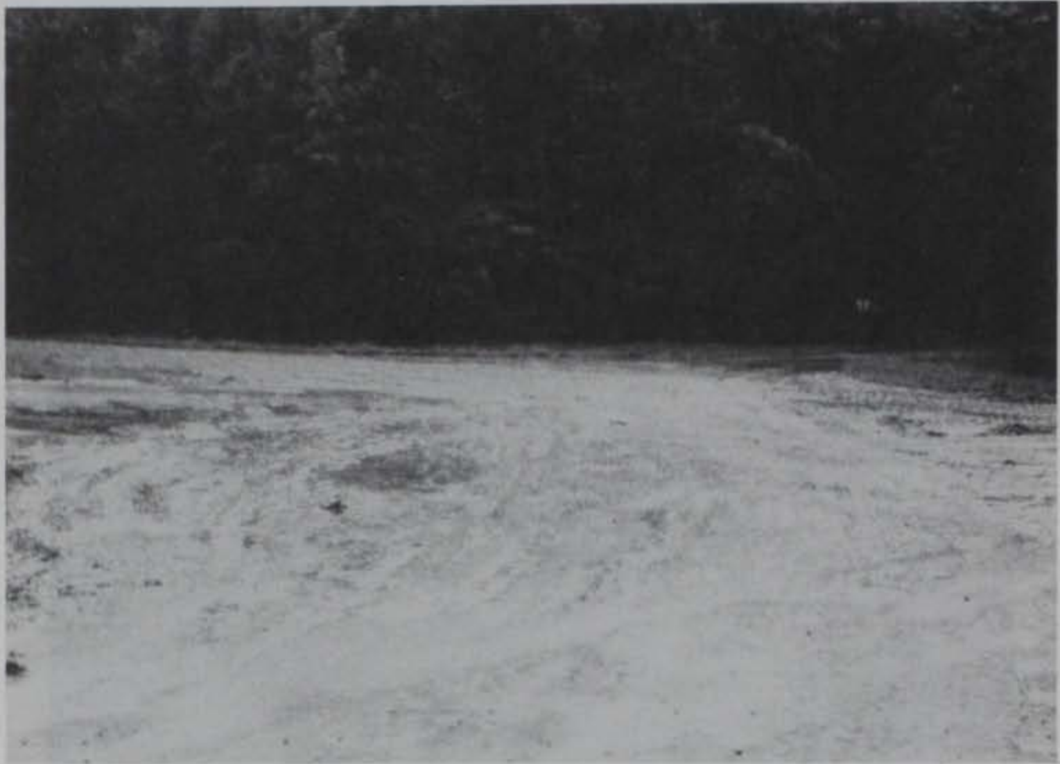
Figure 29. Mud covered block pavement after 1 year of service
