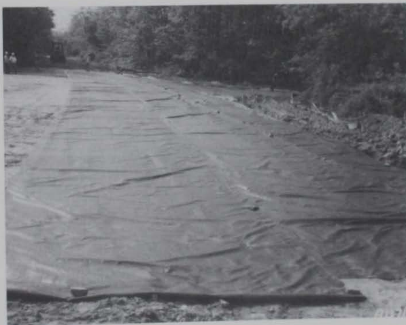
Figure 8. Geotextile on top of recompact subgrade
