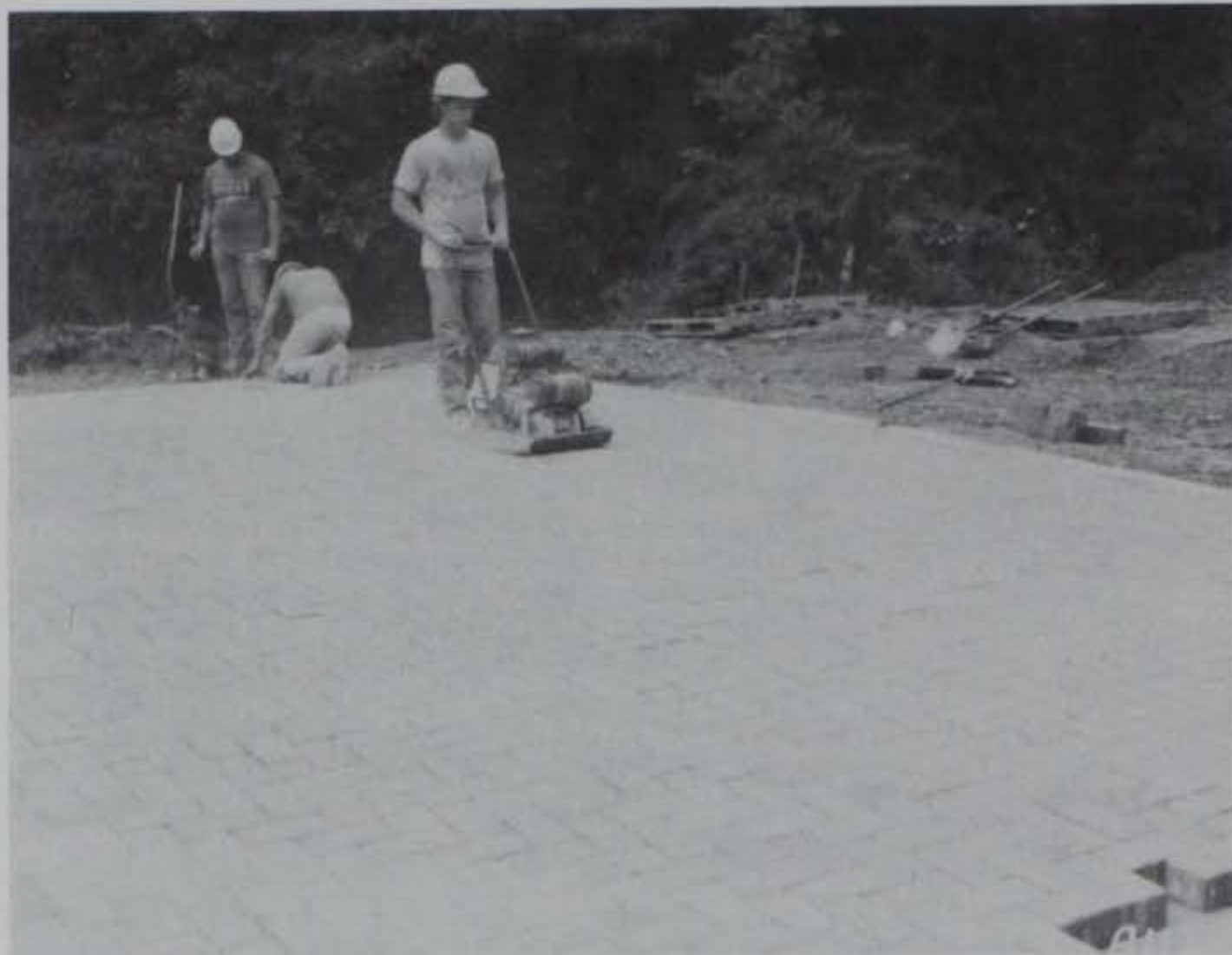
Figure 17. Initial compacting of paving blocks
