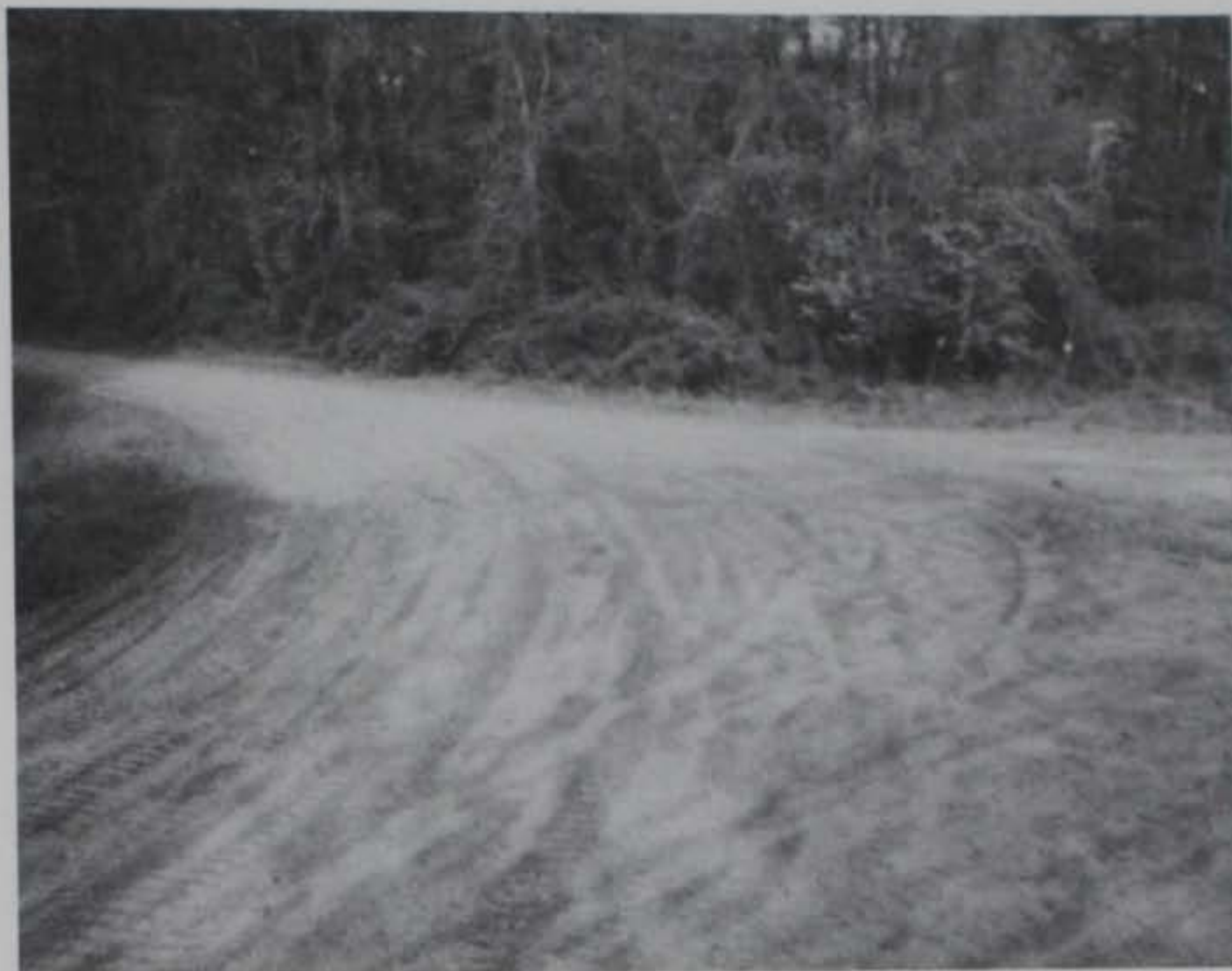
Figure 11. A 4-in.-thick crushed stone base course
