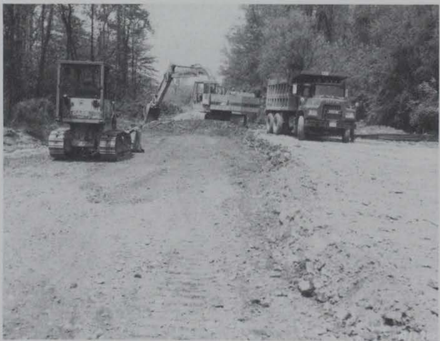
Figure 6. Removing 27 in. of existing soil
