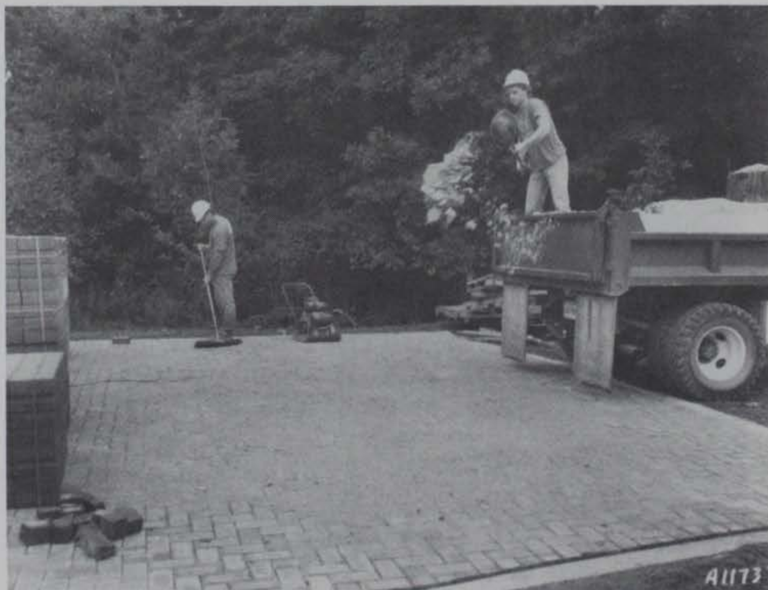
Figure 18. Spreading jointing sand over compacted paving blocks
