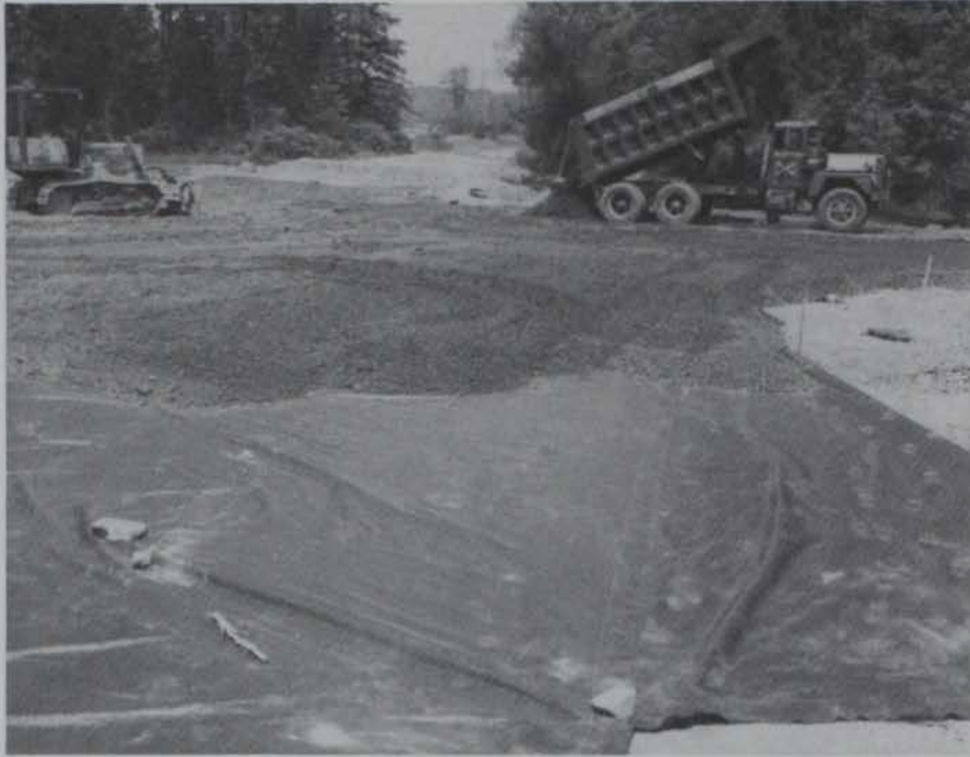
Figure 9. Select-fill subbase material being spread over geotextile
