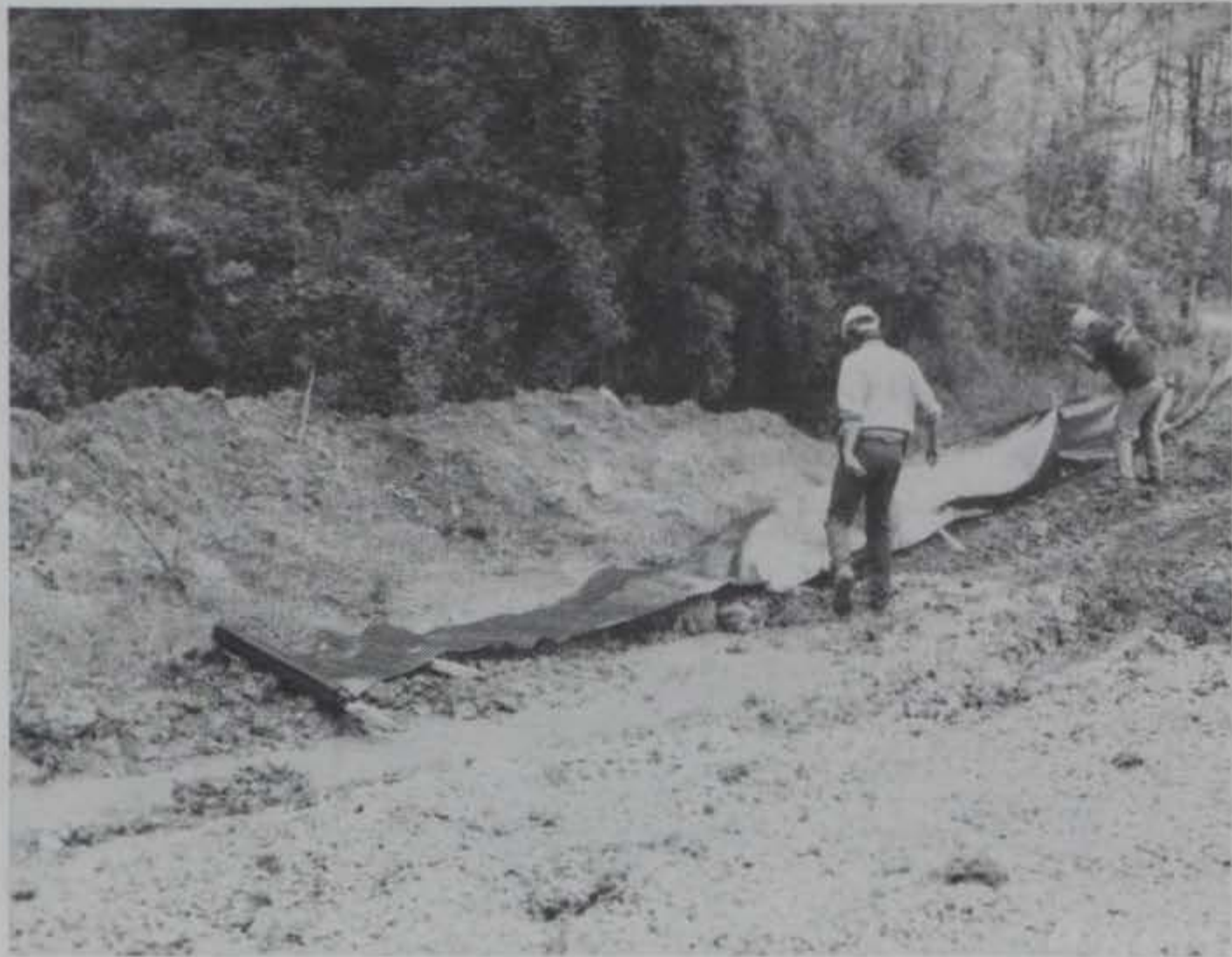
Figure 5. Erecting silt fence barriers
