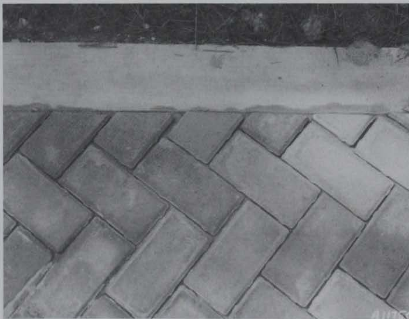
Figure 22. Trimmed edge of block pavement without jointing sand
