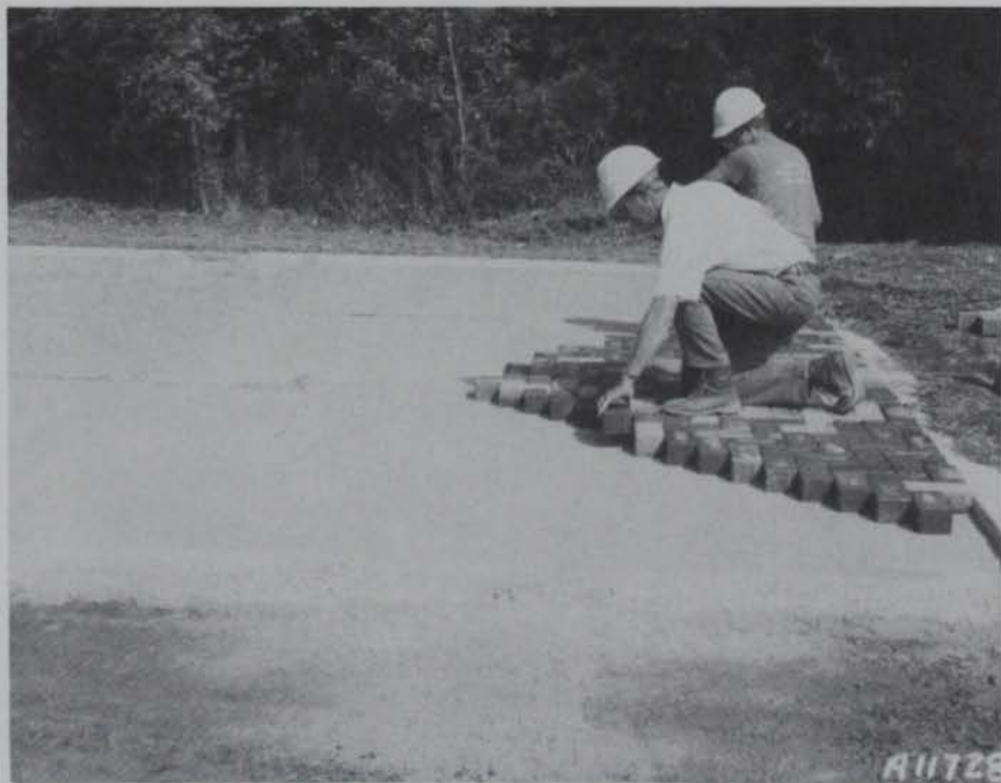
Figure 14. Hand placing concrete paving blocks
