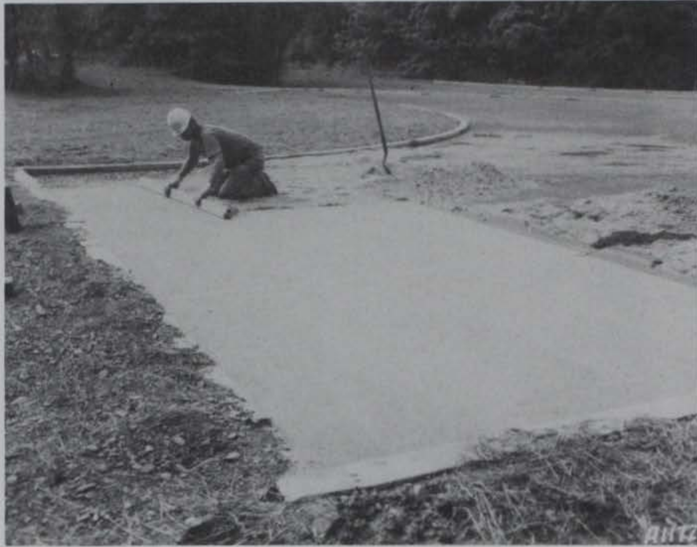
Figure 13. Screeding 1-in.-thick bedding sand layer
