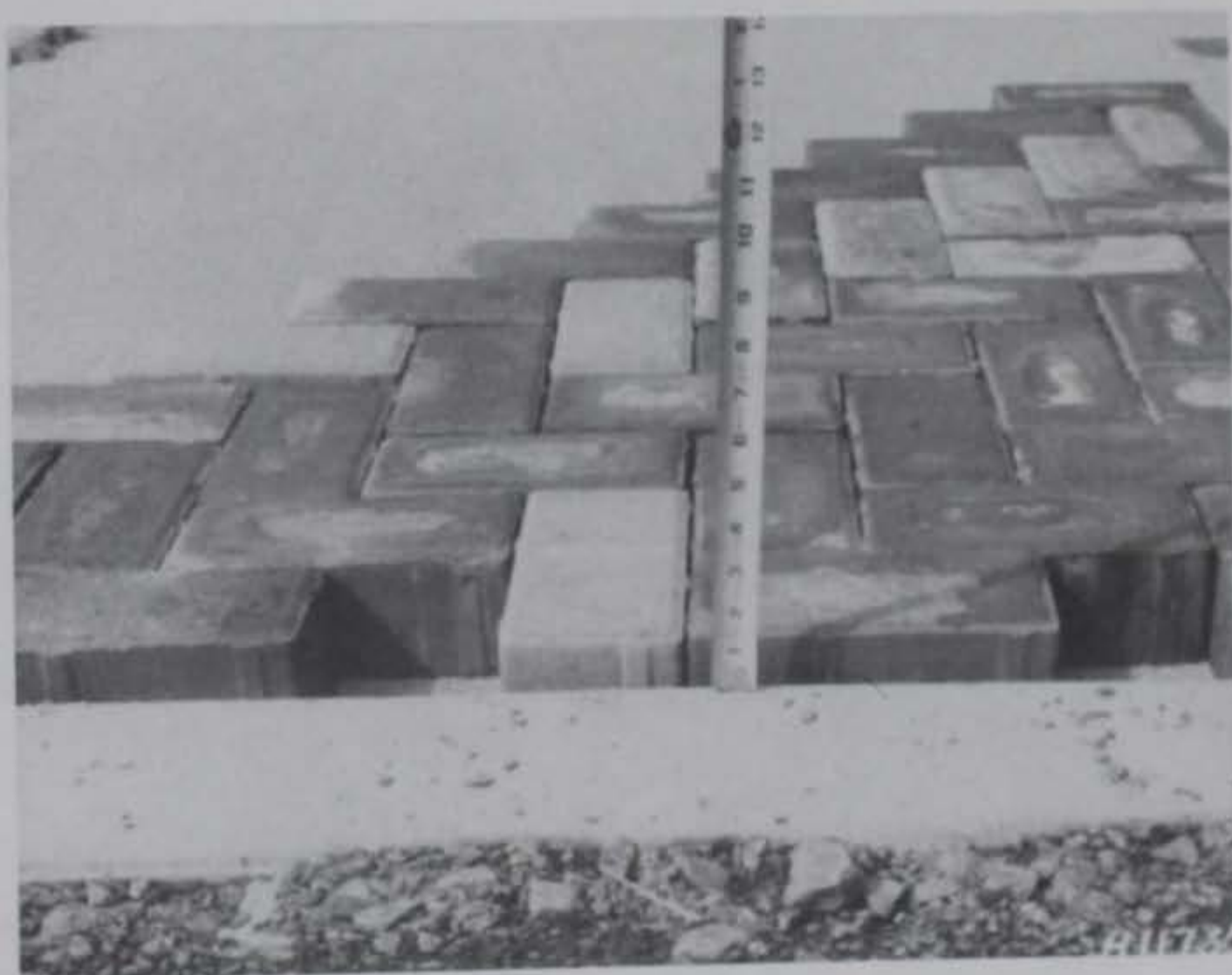
Figure 16. A 3/4-in.-height differential to allow for compaction and settlement
