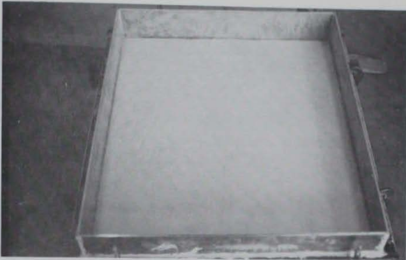
Photo 3. Six-inch-deep collar clamped in position
