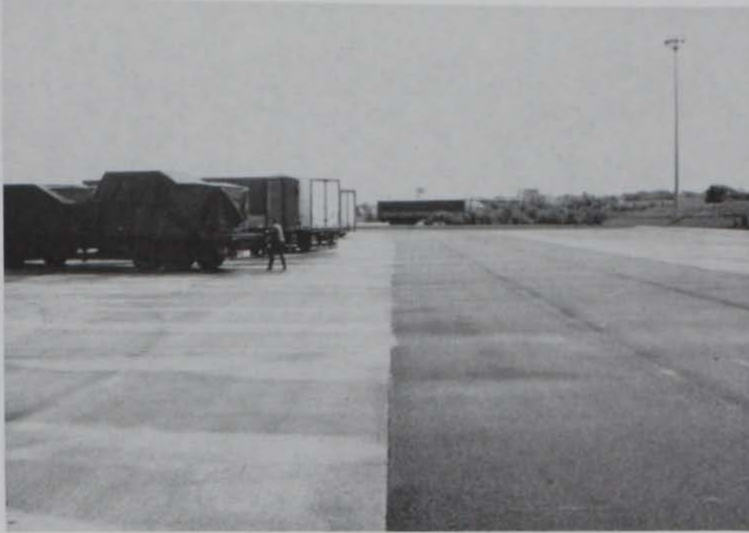
Photo 1. Commercial parking facility - Niort, France
