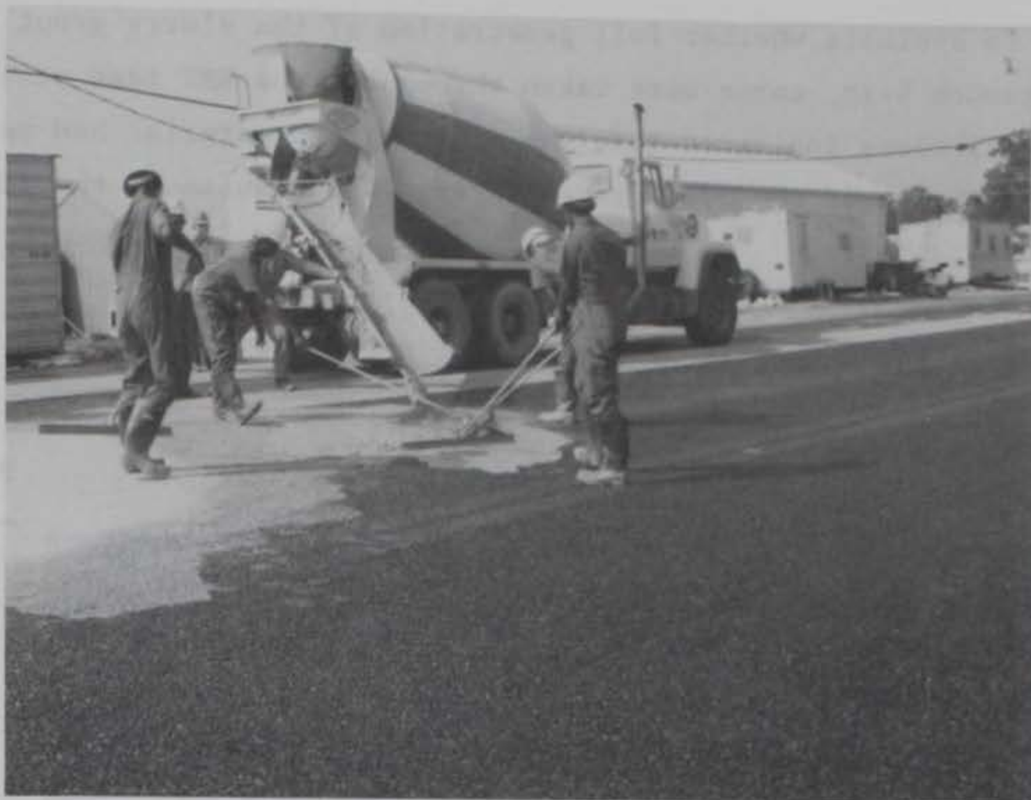
Figure 9. Resin modified slurry grout being applied to open-graded asphalt mixture
