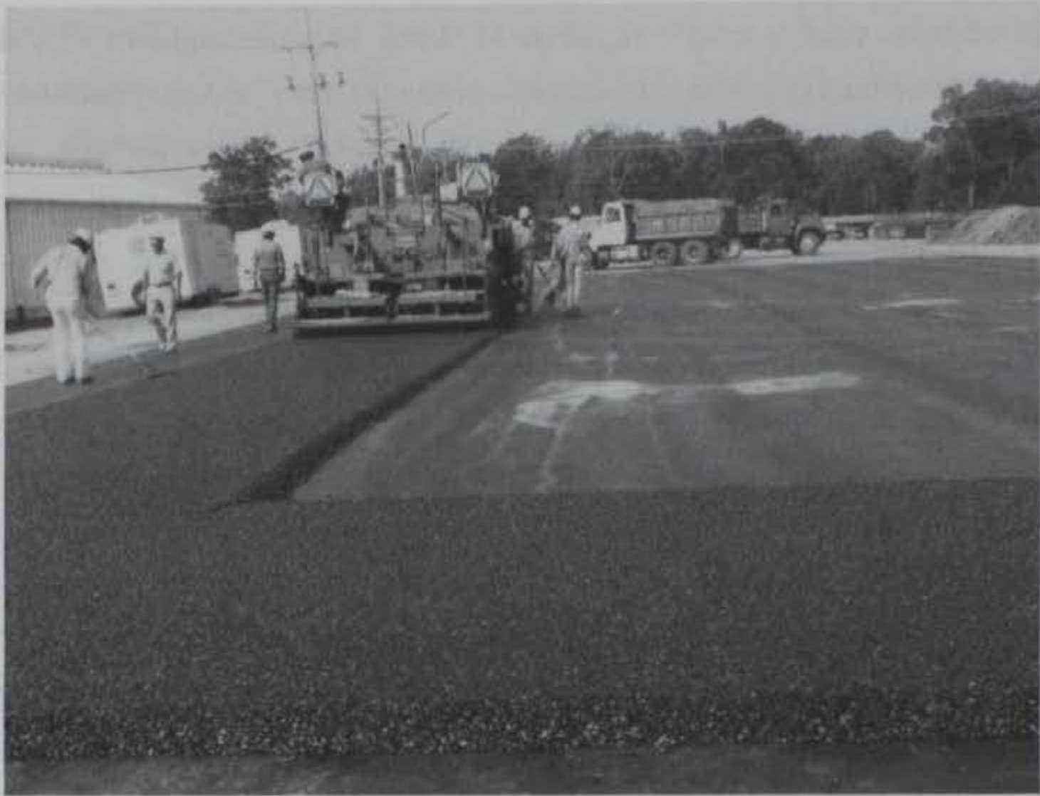
Figure 6. Placing open-graded asphalt material
