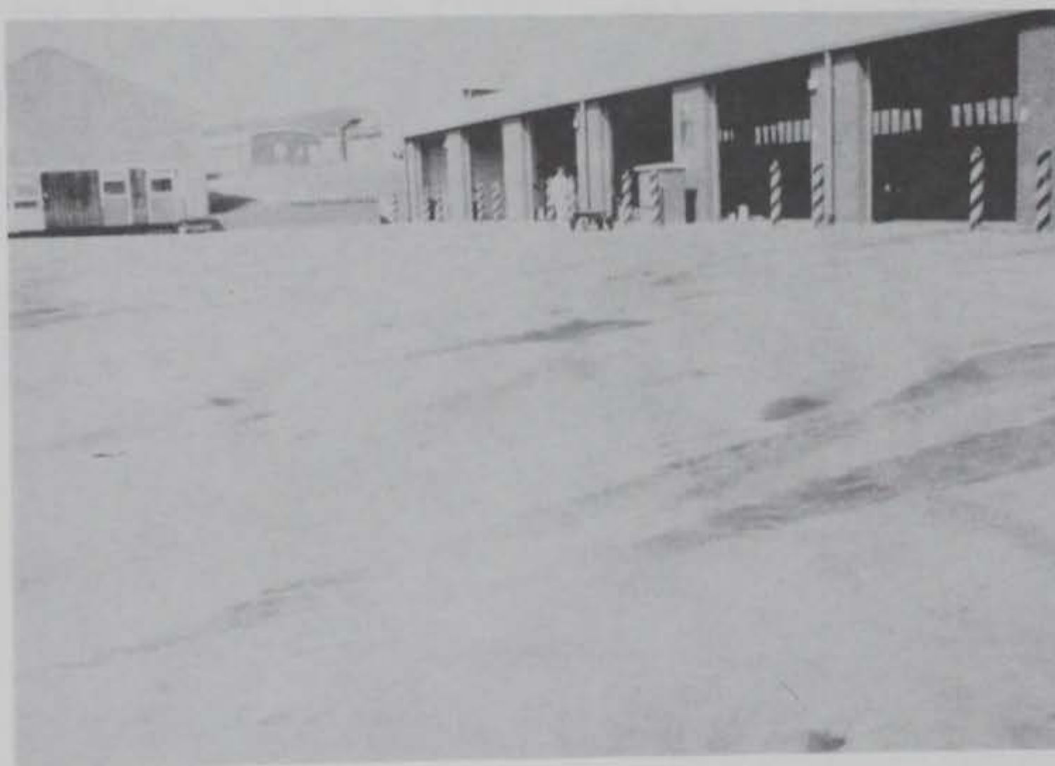
Photo 26. Tank maintenance and staging area, Lulworth, England
