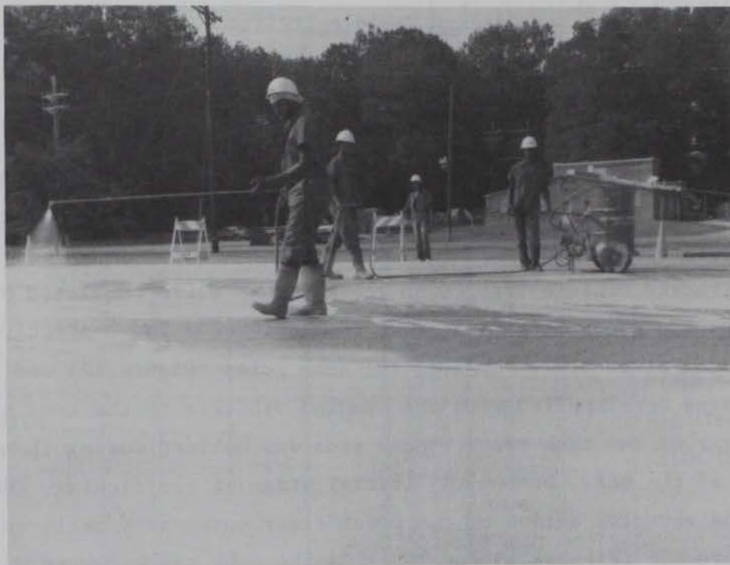
Figure 10. Applying curing compound
