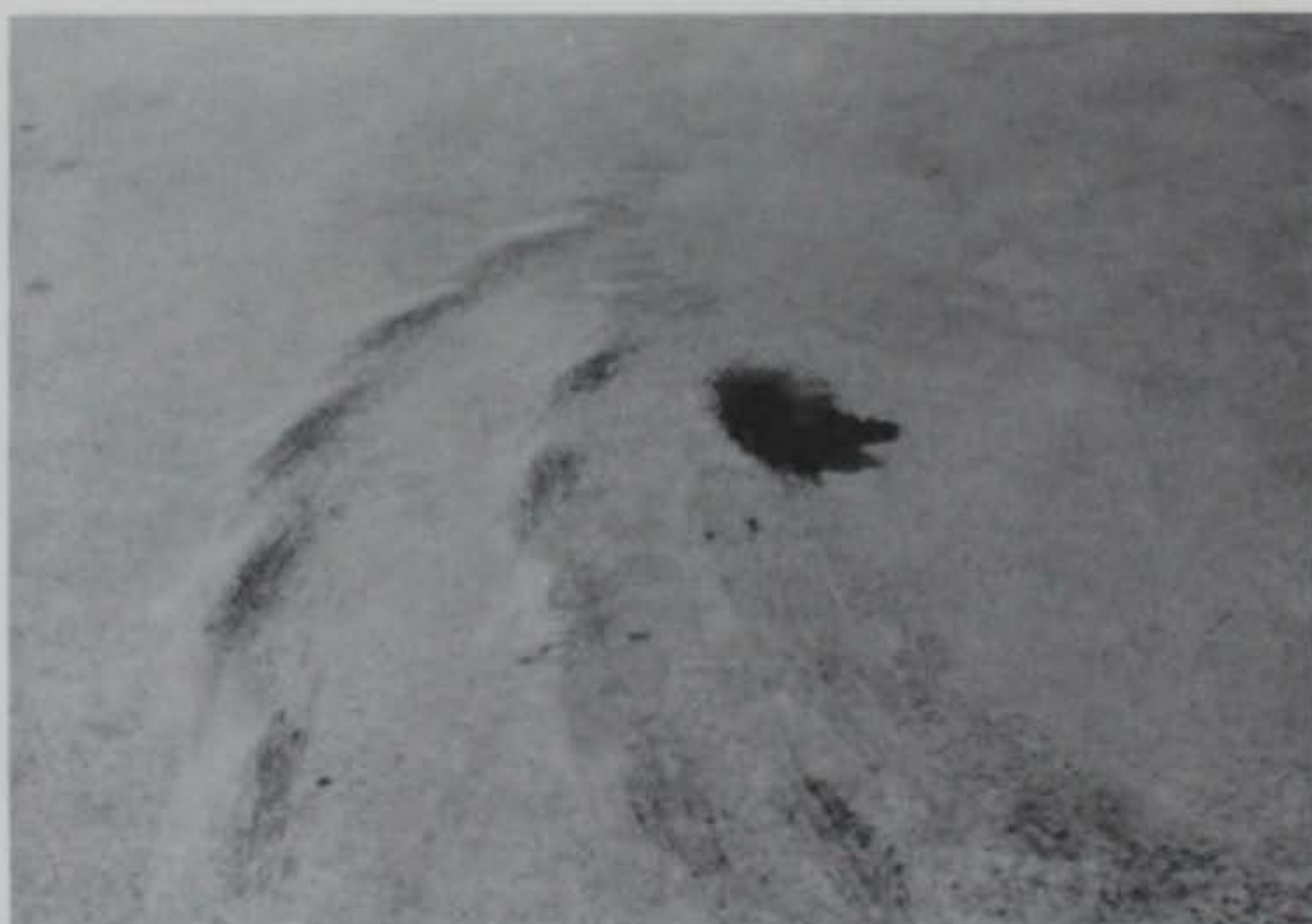
Photo 28. Abrasions caused by locked wheel turns
