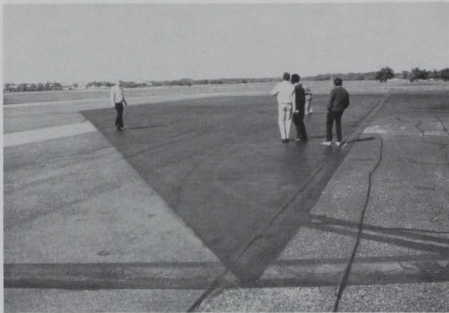
Photo 11. Asphalt concrete pavement that was sealed with Promak
