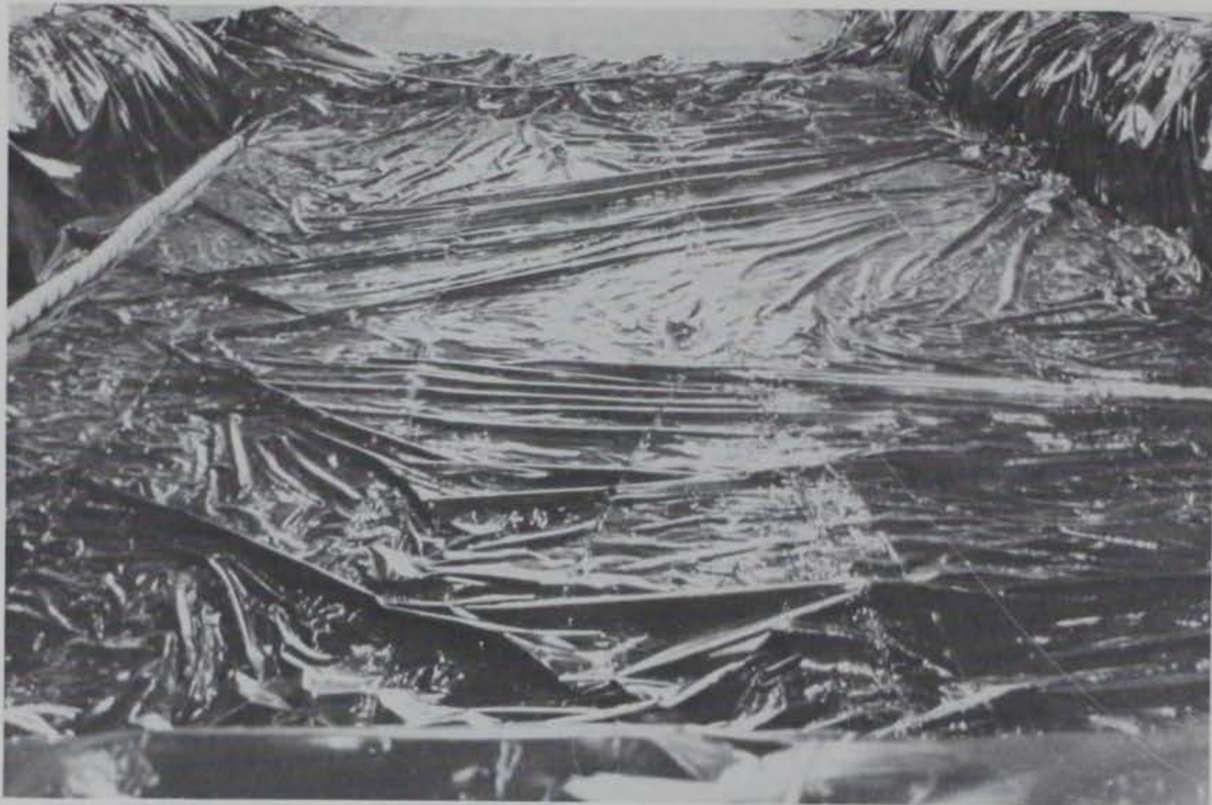
Photo 11. Test Section No. 2 trench lined with waterproof membrane
