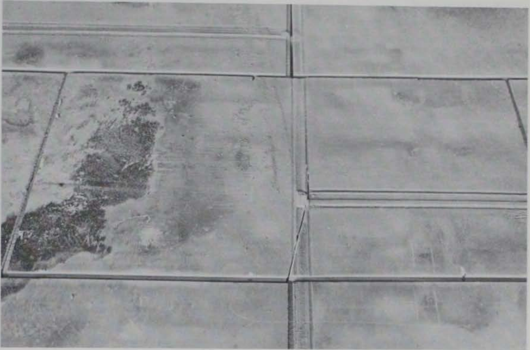
Photo 9. Closeup view of insulation in Test Section No. 1, item 1, after traffic
