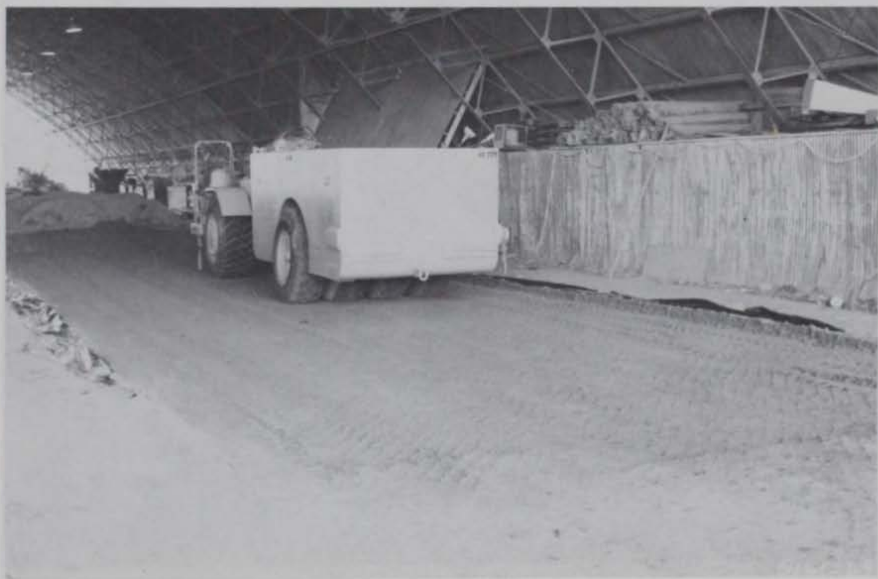
Photo 66. Compacting gravel subbase with 50-ton pneumatic roller
