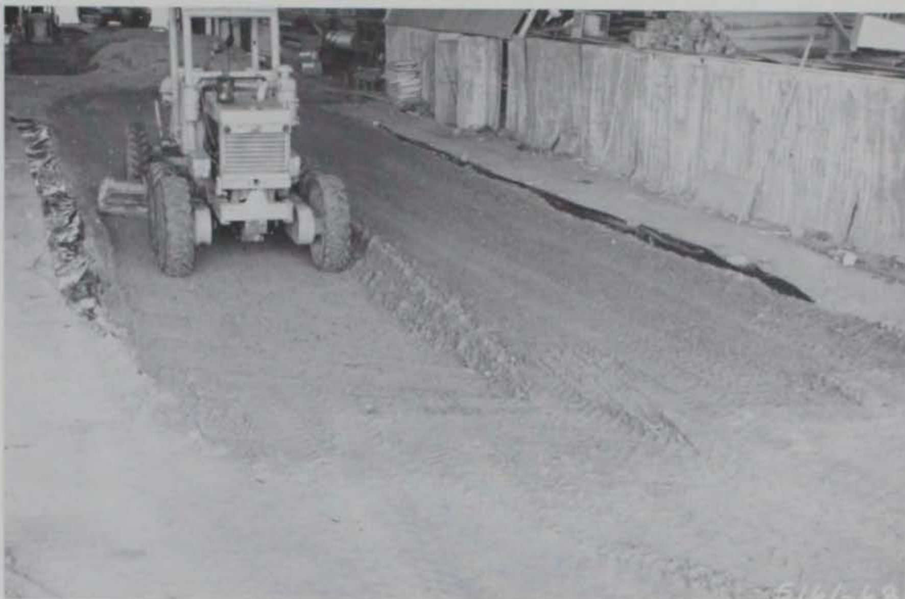
Photo 65. Grading gravel to desired thickness over Styrofoam
