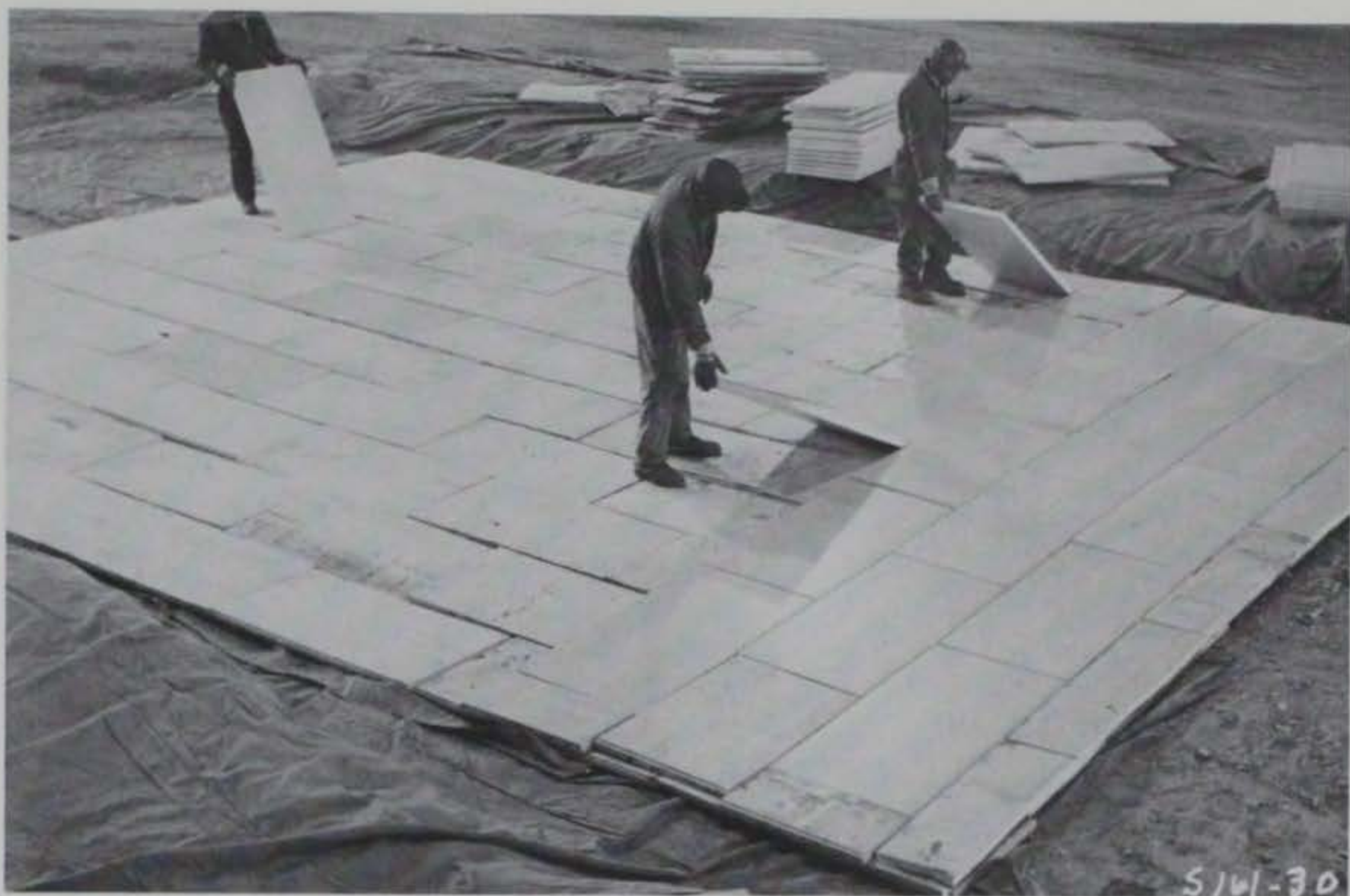
Photo 33. Placing insulation over membrane
