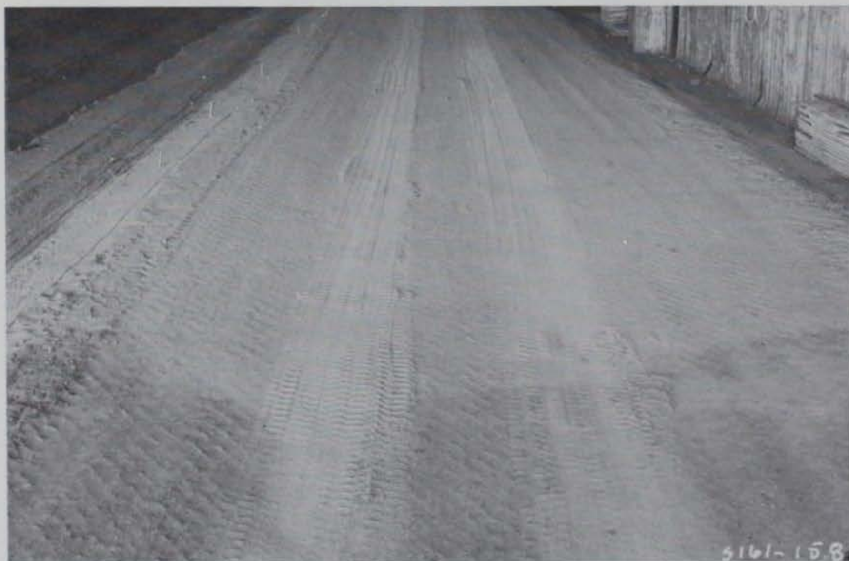
Photo 88. General view of Test Section No. 5 after traffic
