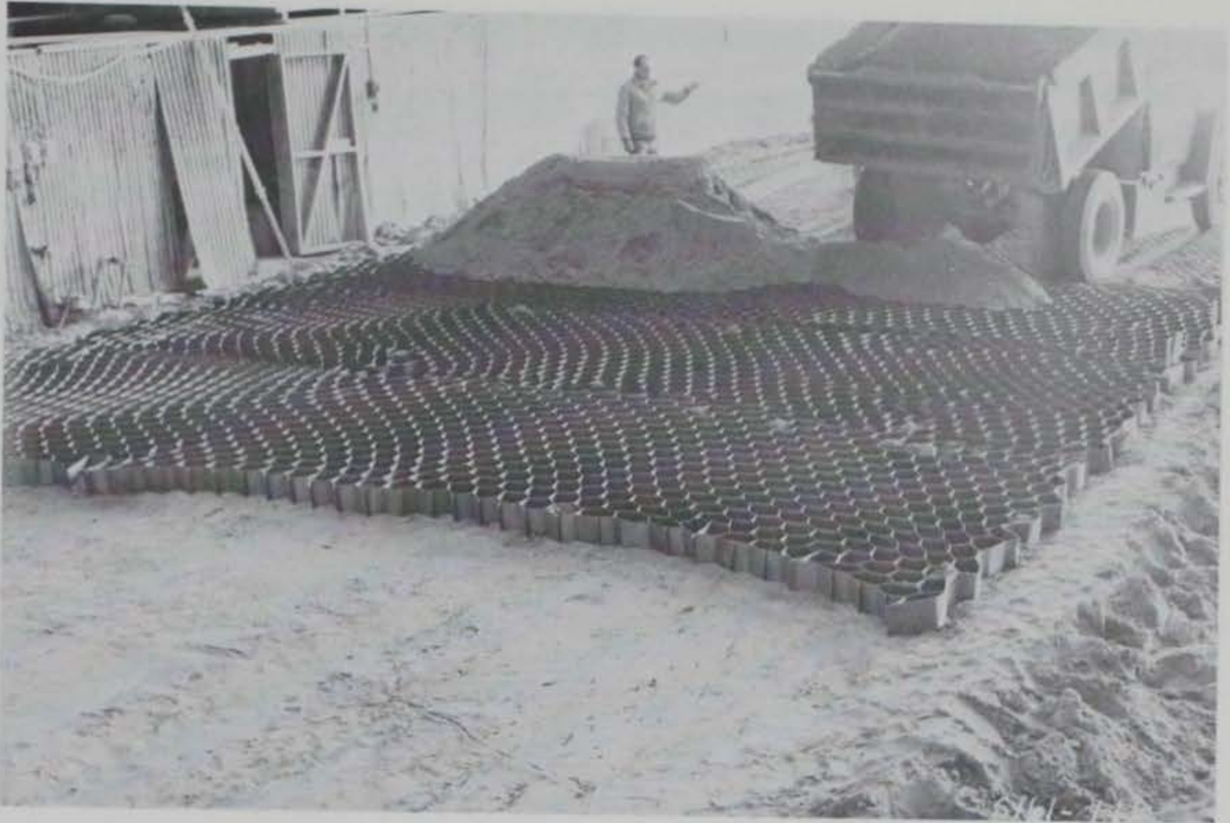
Photo 81. Dumping sand into 6-in. paper grid
