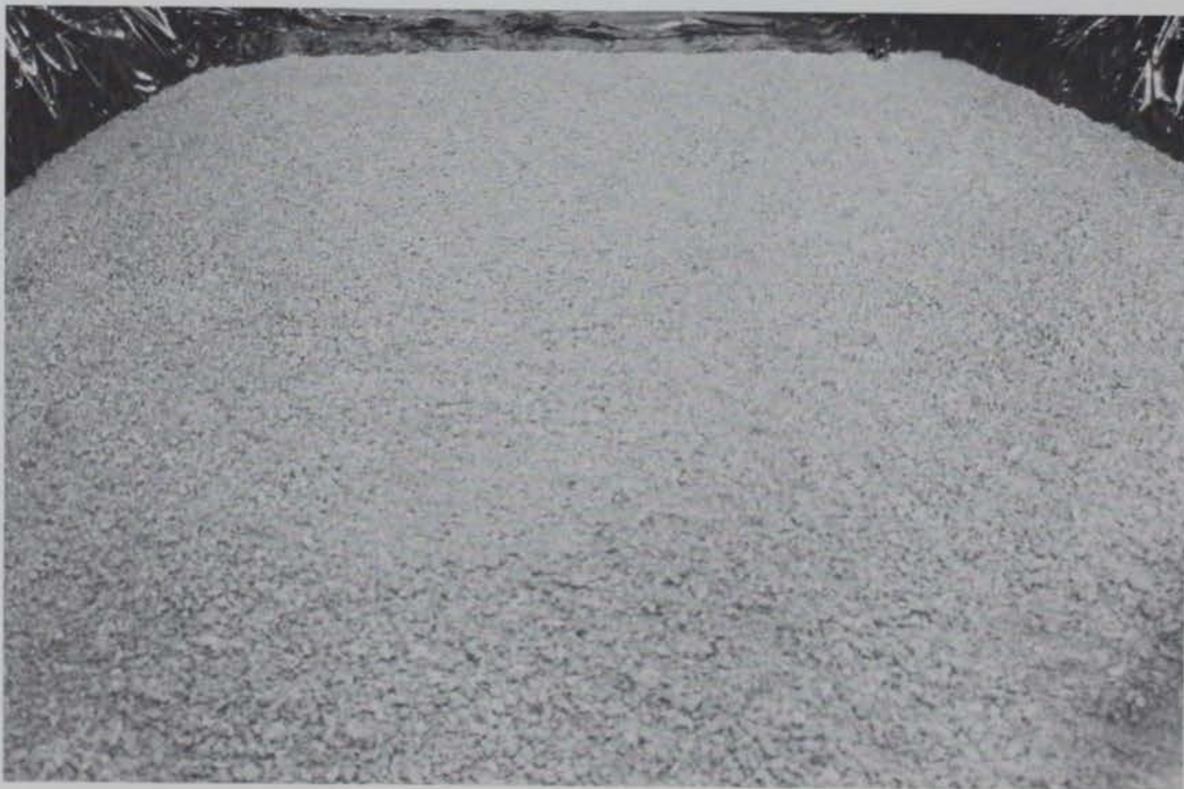
Photo 12. General view of finished gravel blanket
