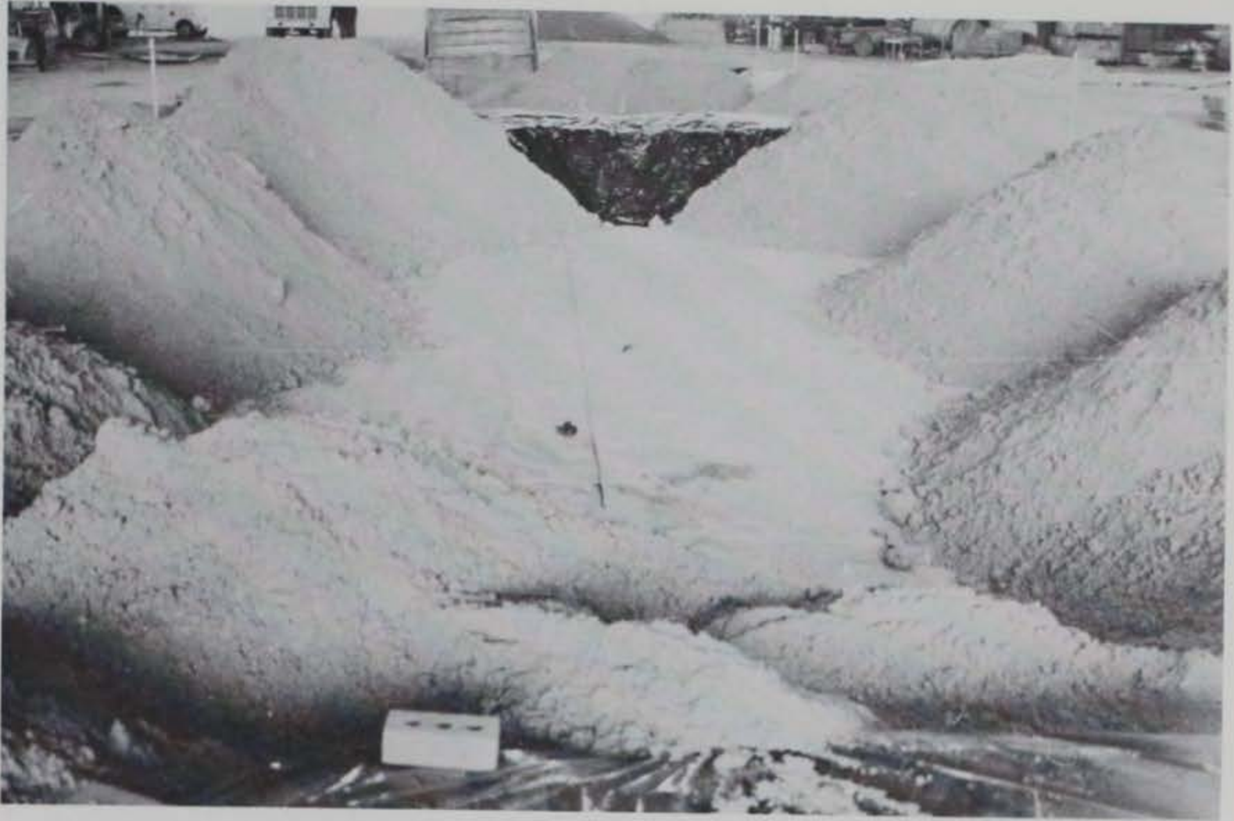
Photo 13. Sand end dumped on top of filter cloth
