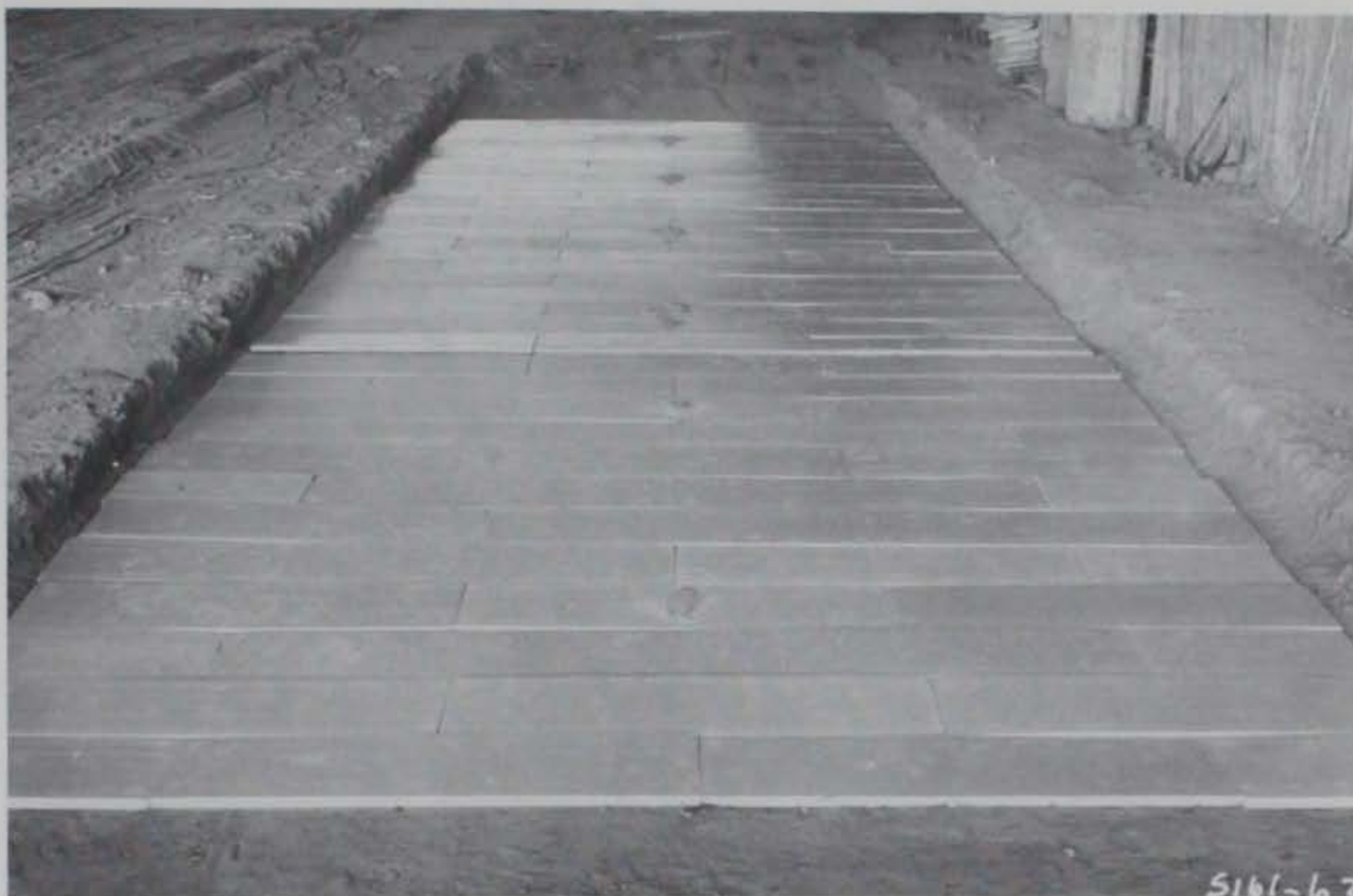
Photo 61. Styrofoam HI 60-psi panels in place on subgrade
