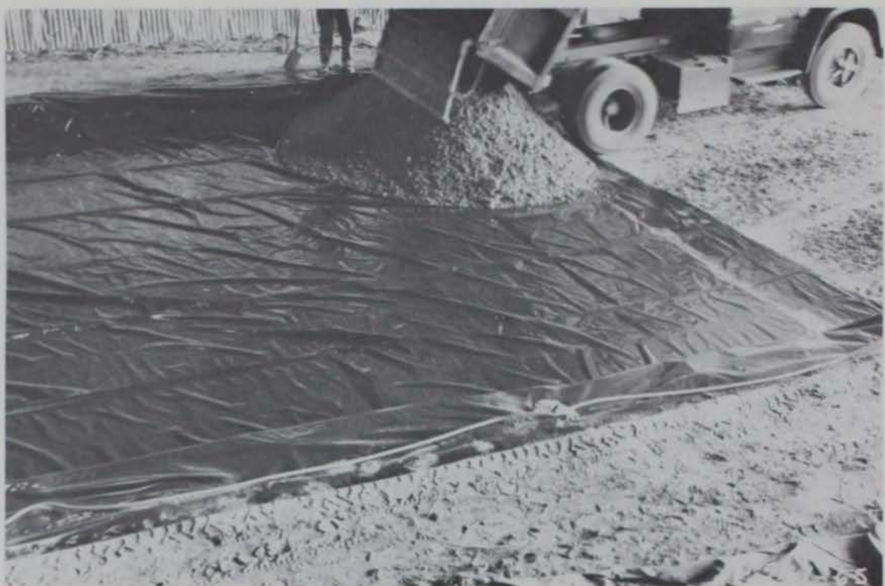
Photo 63. End dumping gravel on Styrofoam
