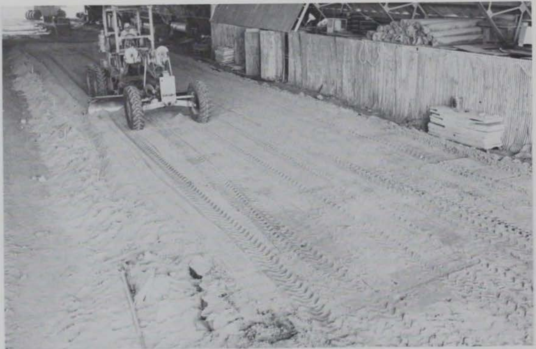
Photo 84. Grading excess sand from top of grid leaving 1-1/2- to 2-in. cover
