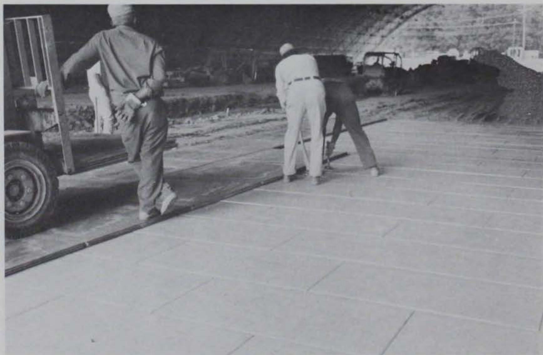
Photo 4. Placing XML9 landing mat over insulation
