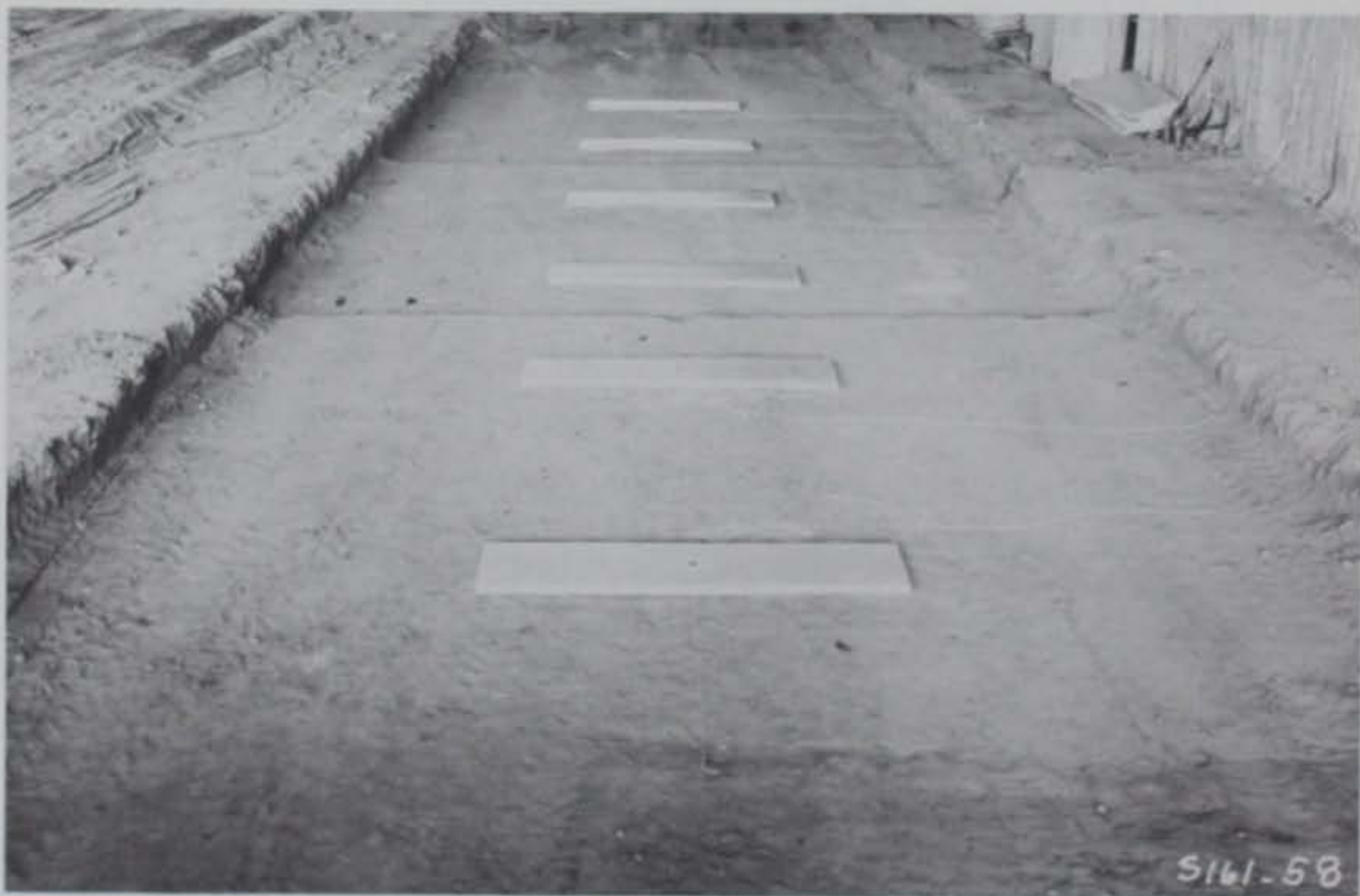
Photo 60. Instrumented Styrofoam panels in place on subgrade
