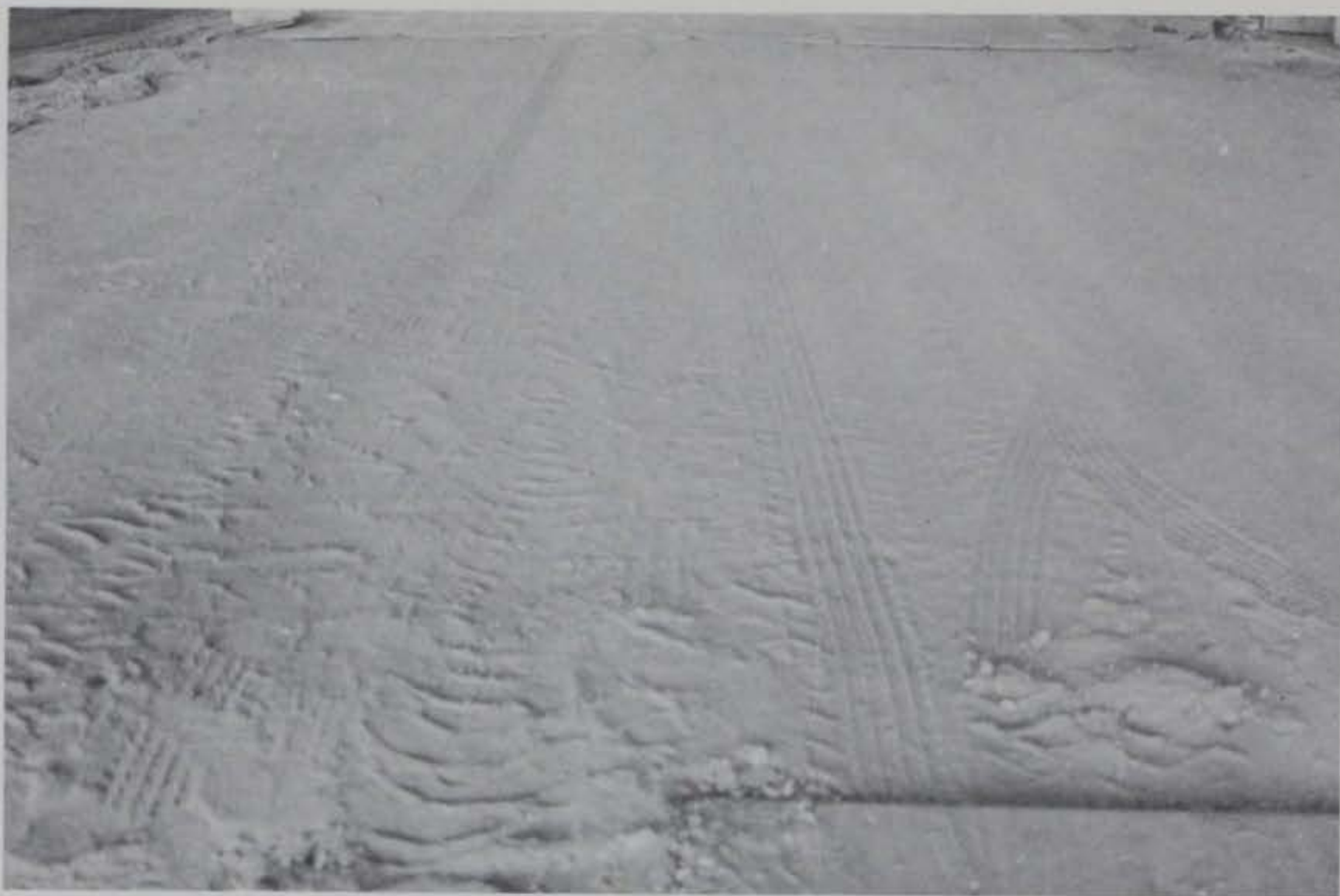
Photo 7. General view of base course, Test Section No. 1, item 2, after traffic
