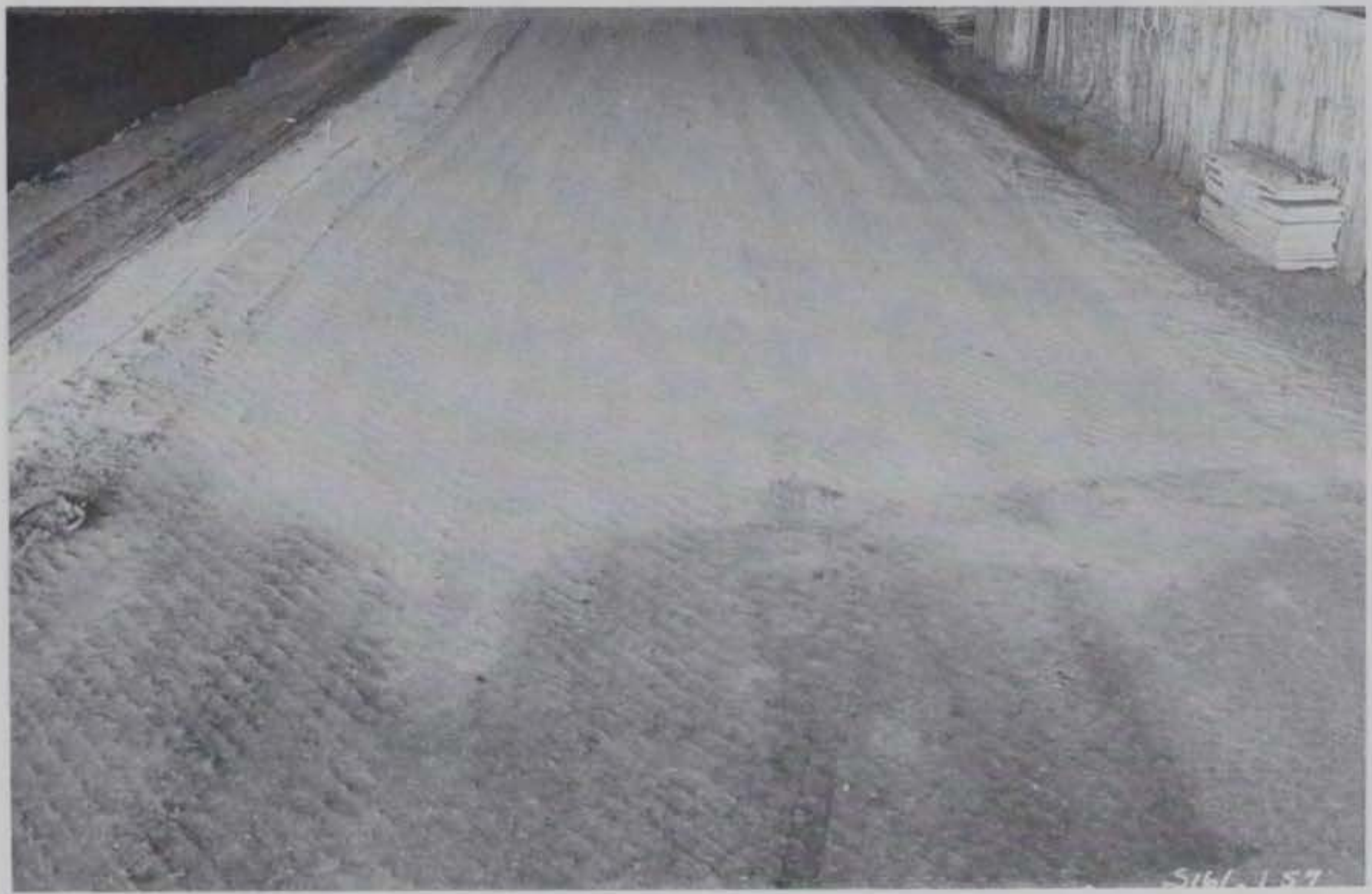
Photo 86. General view of Test Section No. 5 prior to traffic
