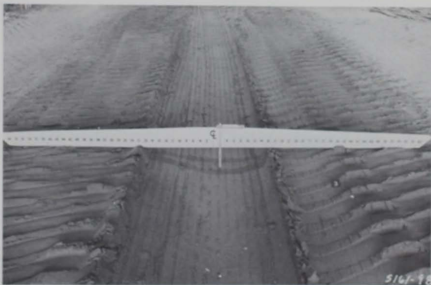
Photo 46. Test Section No. 3, item 3, after 100 coverages of C-130 loading
