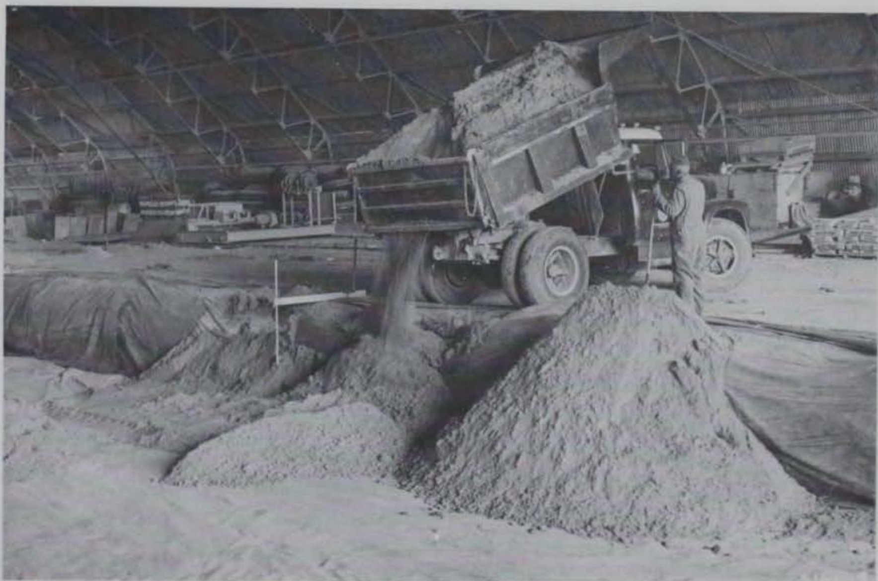
Photo 26. End dumping sand into Test Section No. 3 trench
