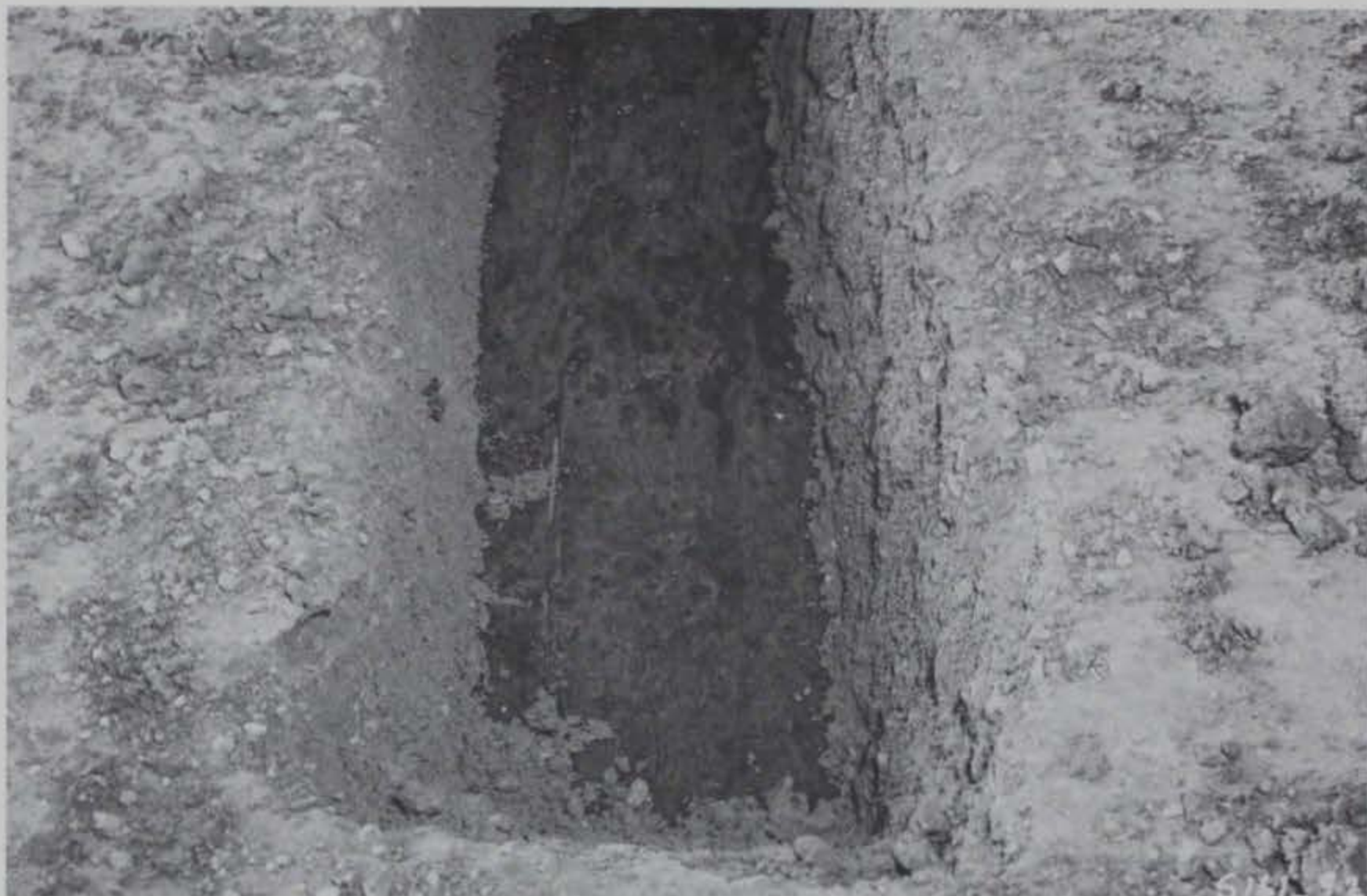
Photo 71. Trench in Test Section No. 4, item 1, showing condition of membrane after 480 passes
