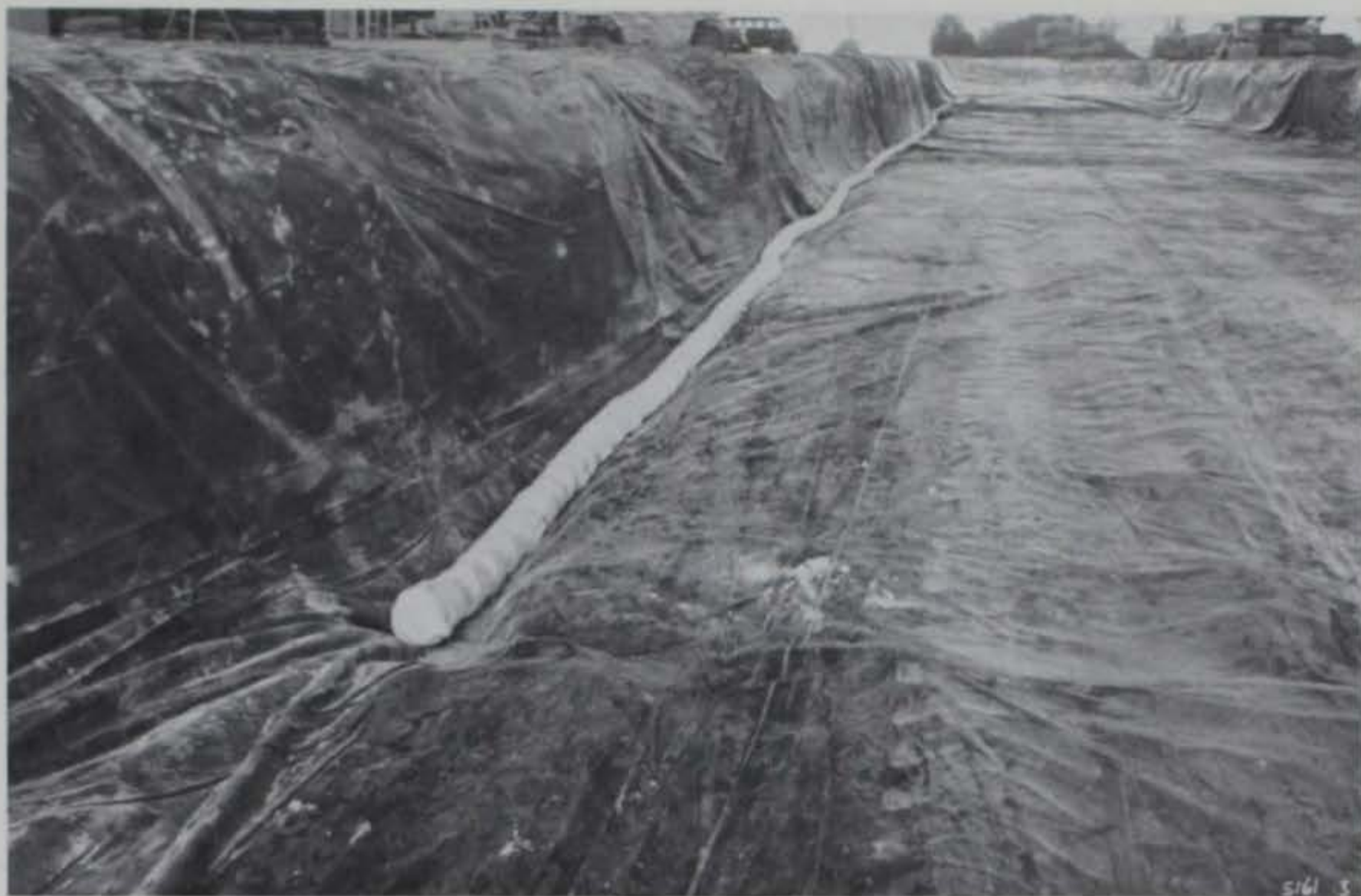
Photo 21. Membrane-lined Test Section No. 3 trench
