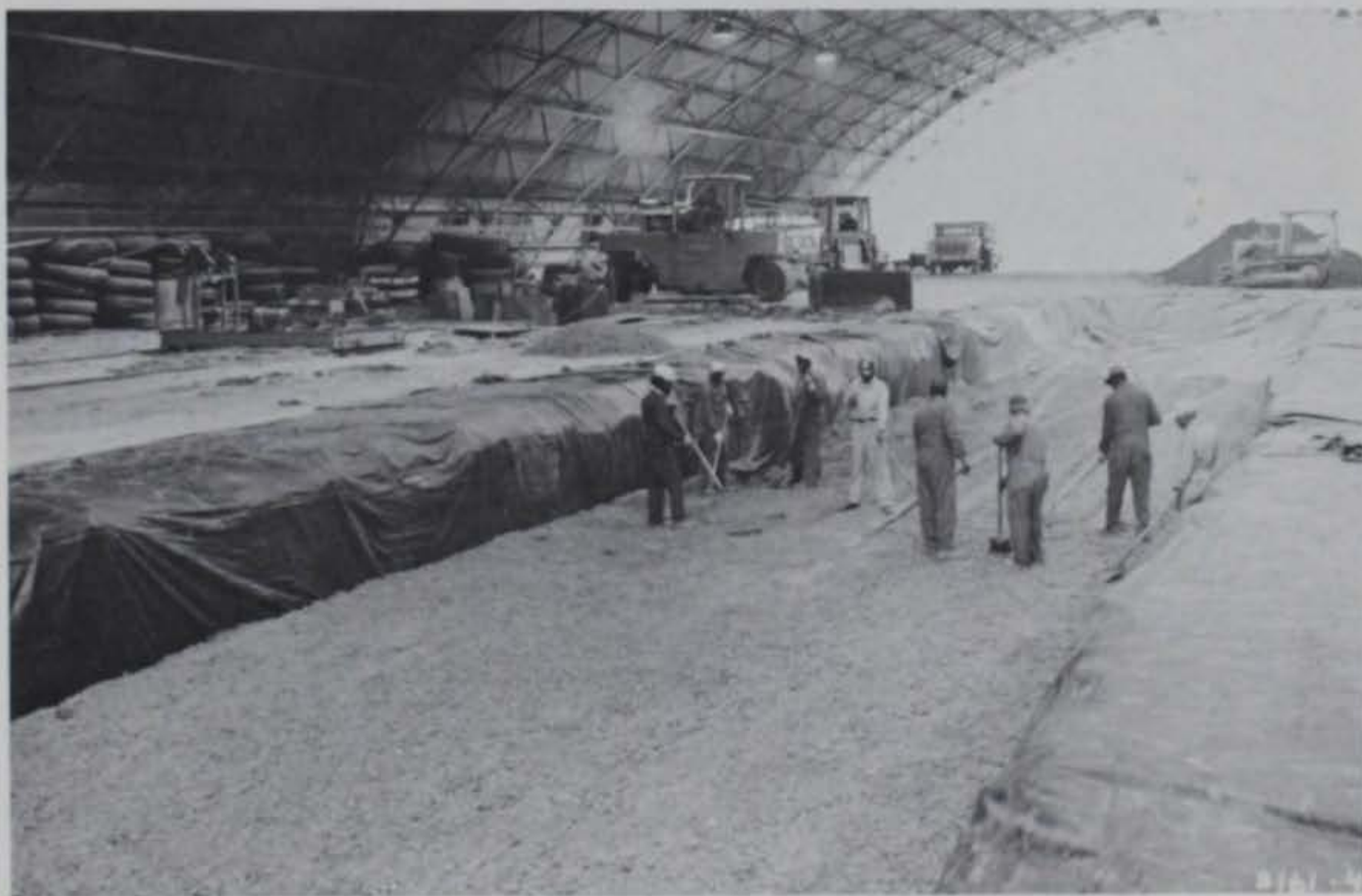
Photo 22. Hand leveling washed gravel
