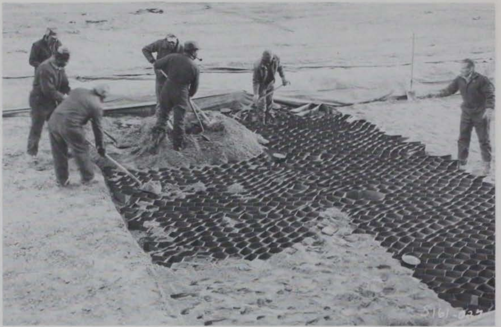
Photo 31. Filling grids with hand shovels
