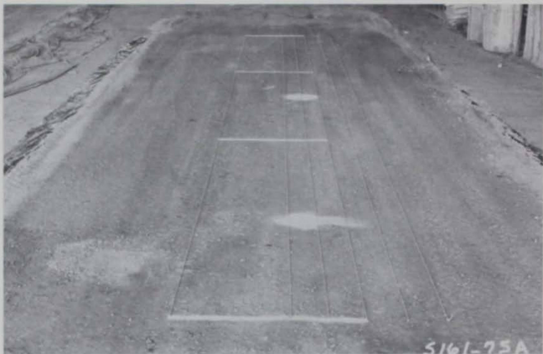
Photo 67. General view of completed Test Section No. 4 prior to traffic
