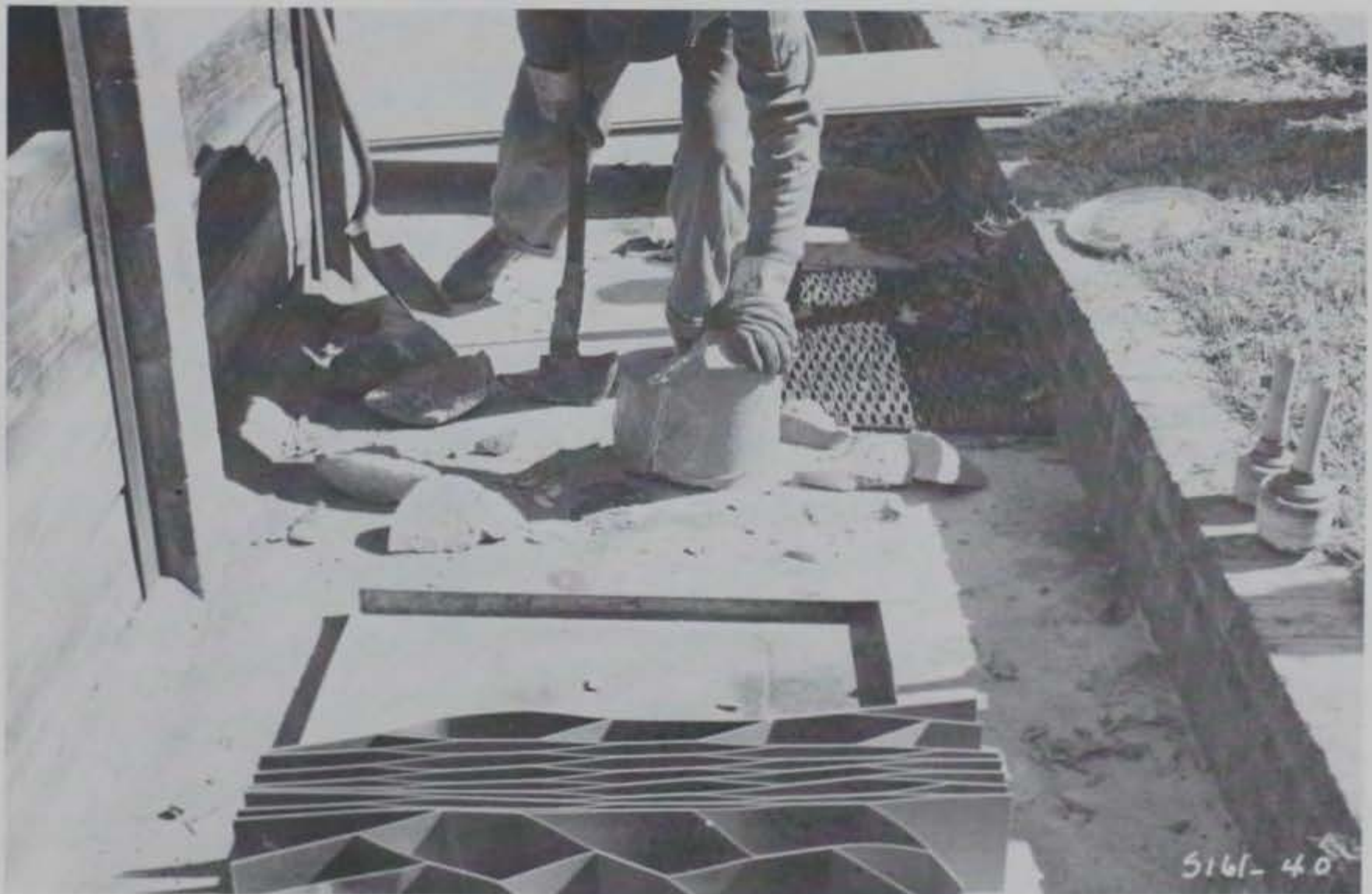
Photo 54. Breaking up frozen sand with ax
