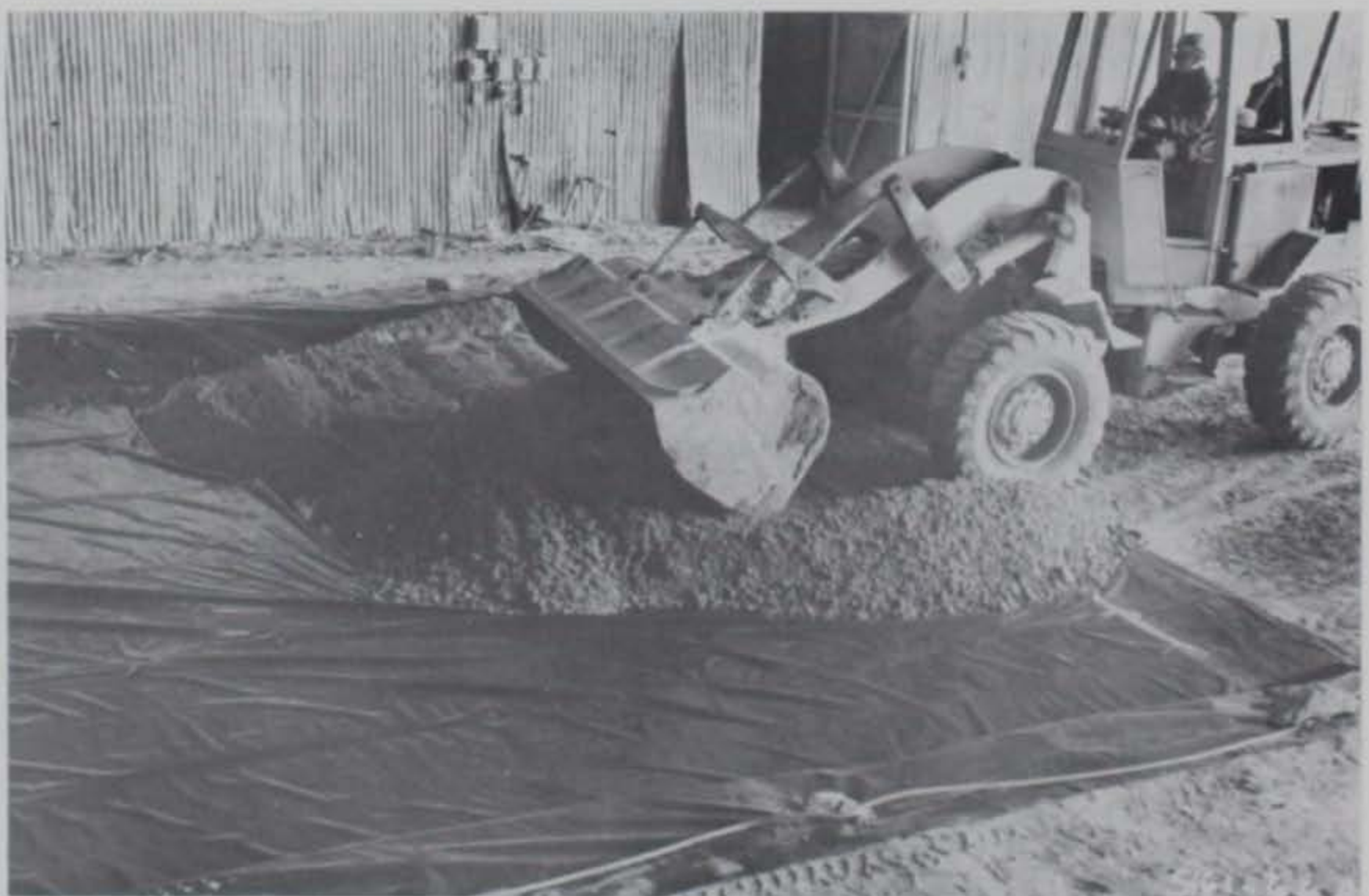
Photo 64. Spreading gravel over Styrofoam with front-end loader
