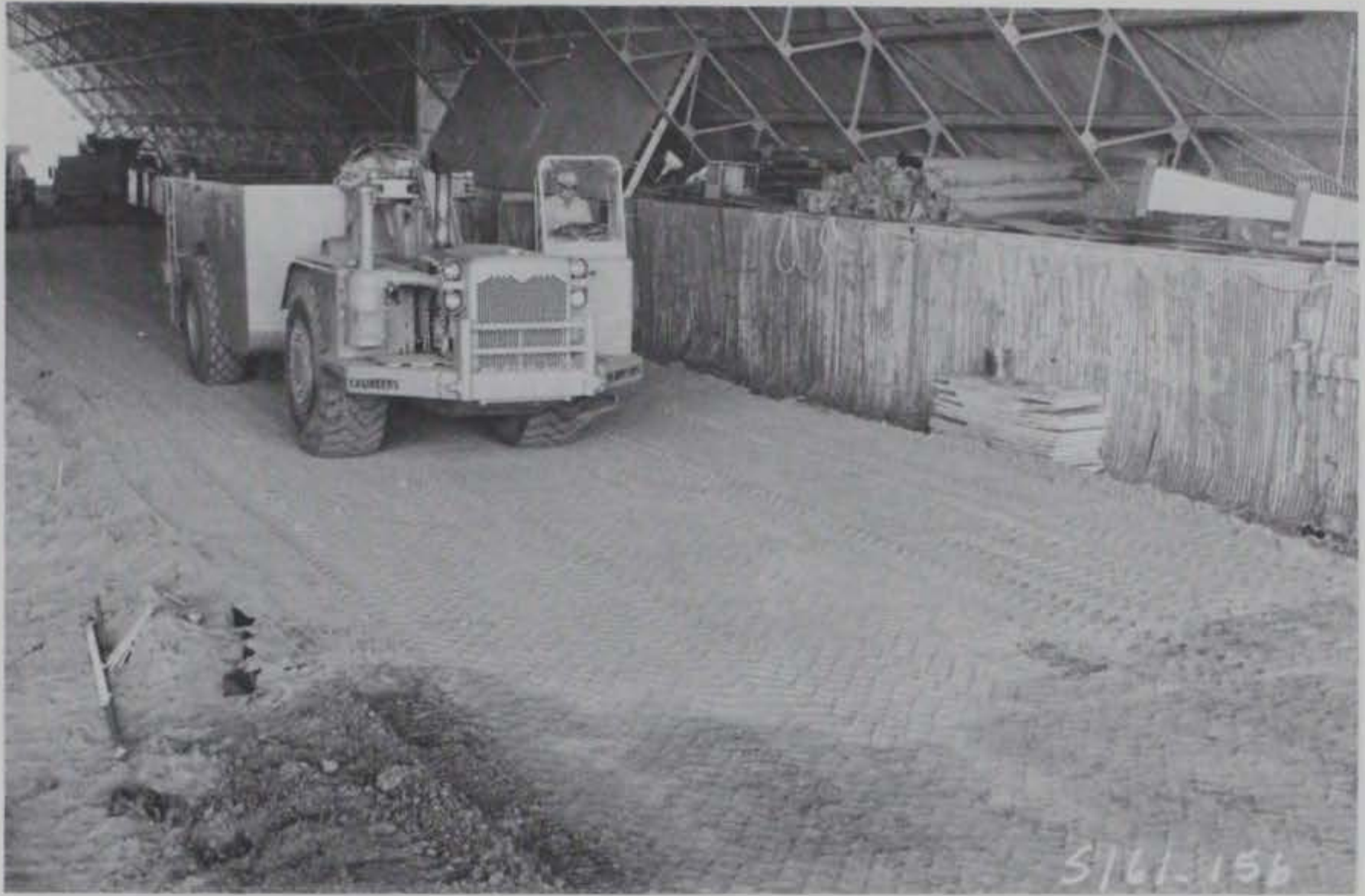
Photo 85. Compacting sand into grid with 50-ton pneumatic roller
