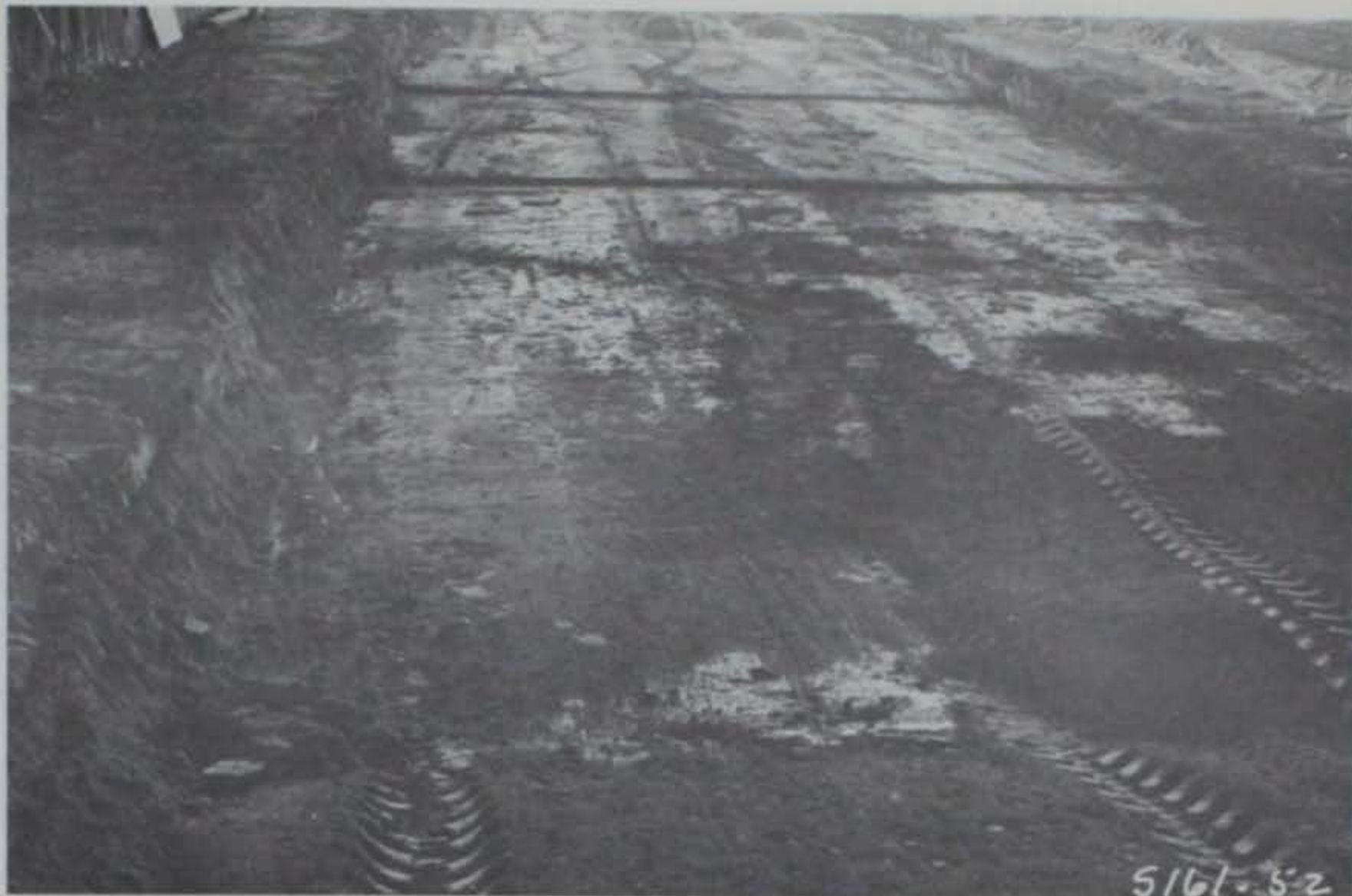
Photo 57. General view of prepared subgrade
