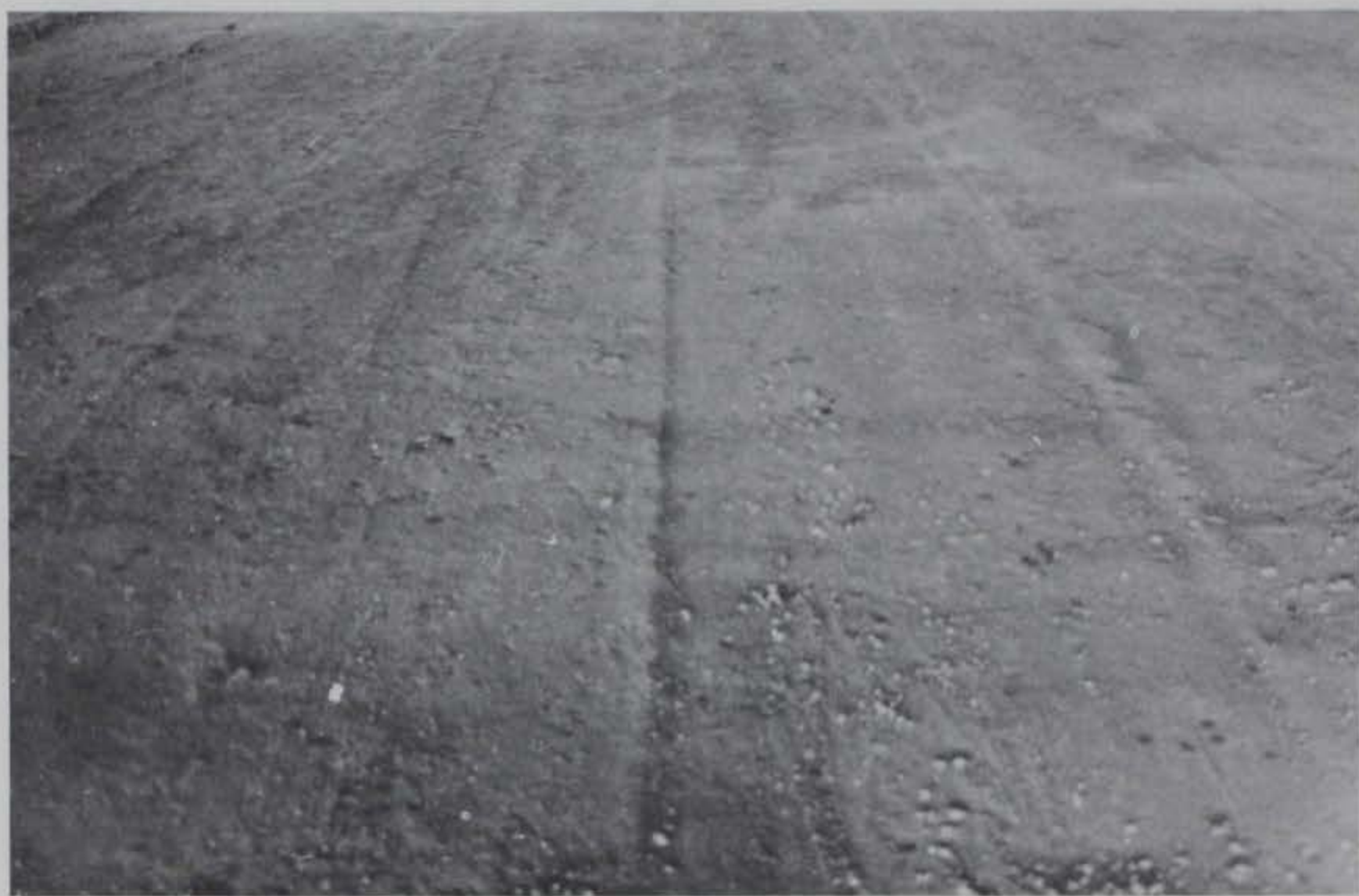
Photo 3. Gravel base over insulation
