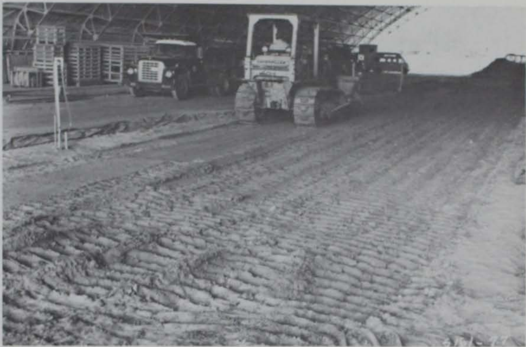
Photo 41. Compaction with D-4 tractor
