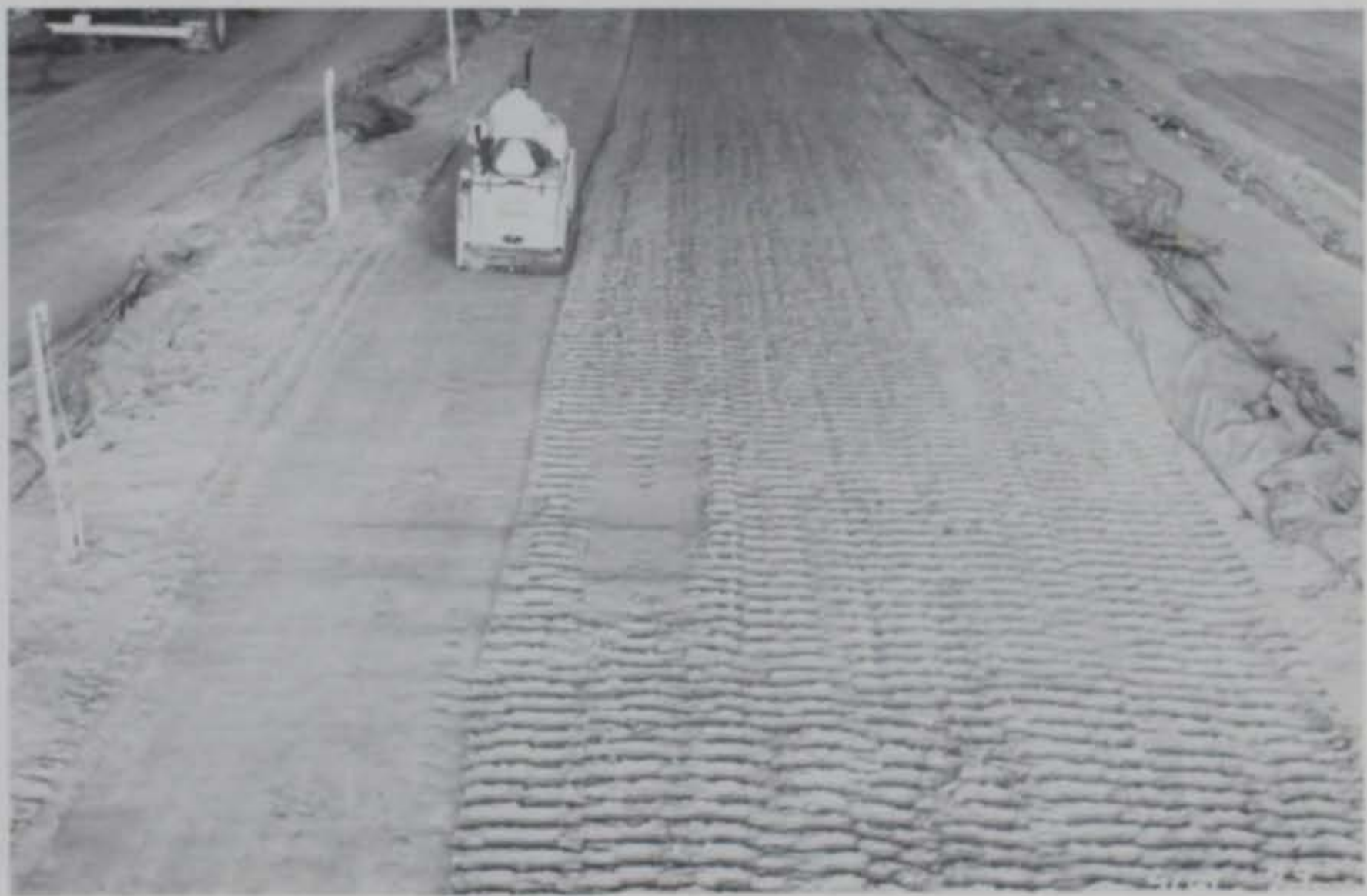
Photo 42. Compaction with vibratory roller
