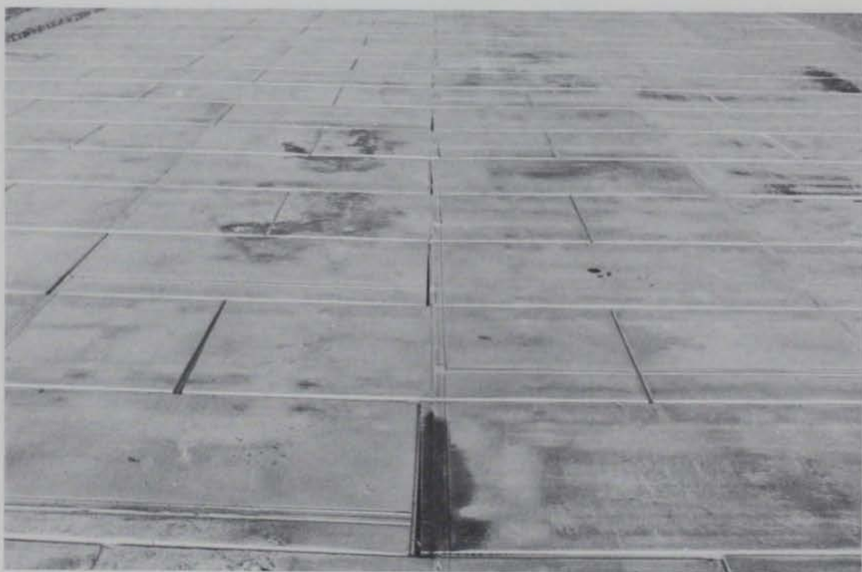
Photo 8. General view of insulation in Test Section No. 1, item 1, after traffic
