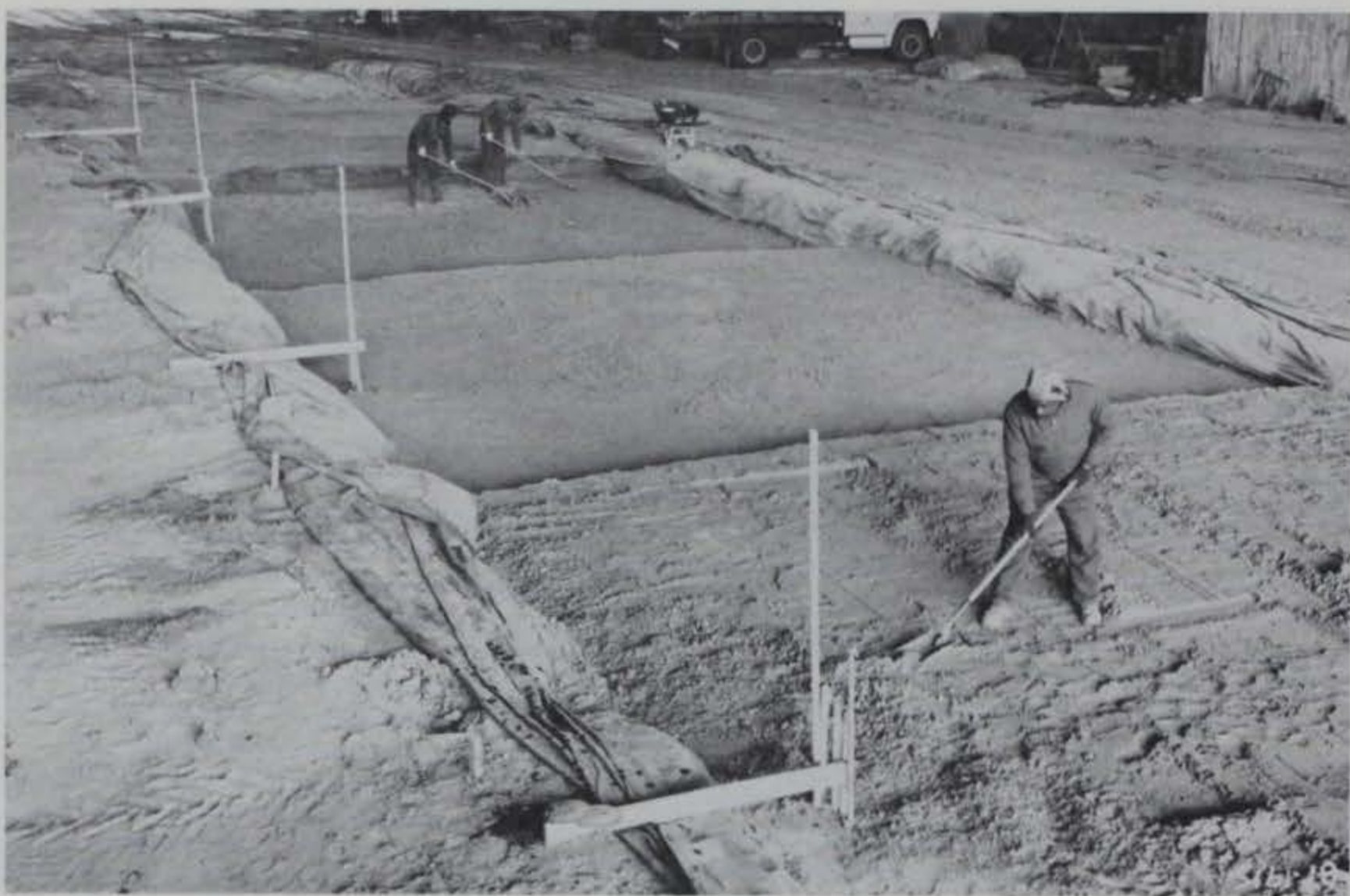
Photo 27. Hand leveling of sand surface prior to placing grids
