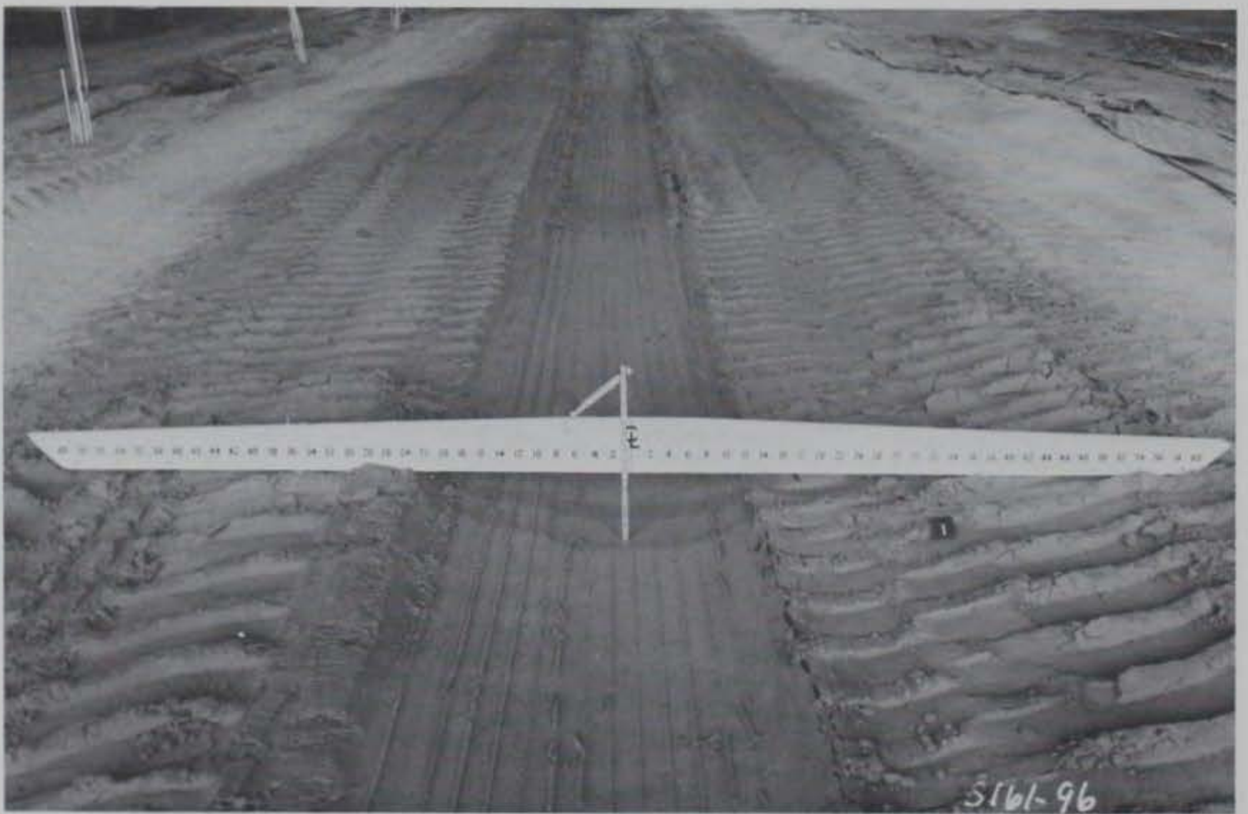
Photo 44. Test Section No. 3, item 1, after 100 coverages of C-130 loading
