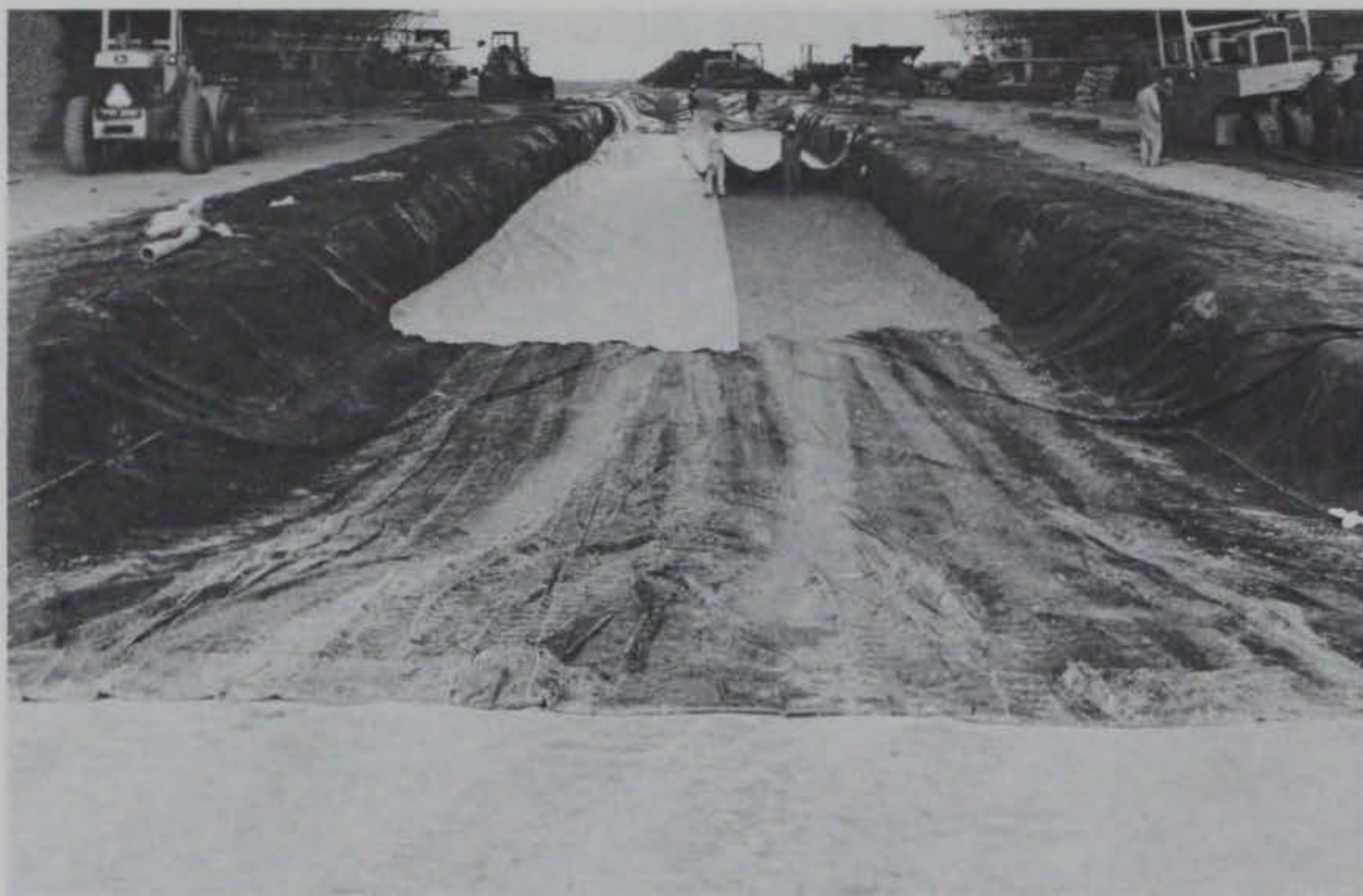
Photo 23. Placing filter cloth over gravel
