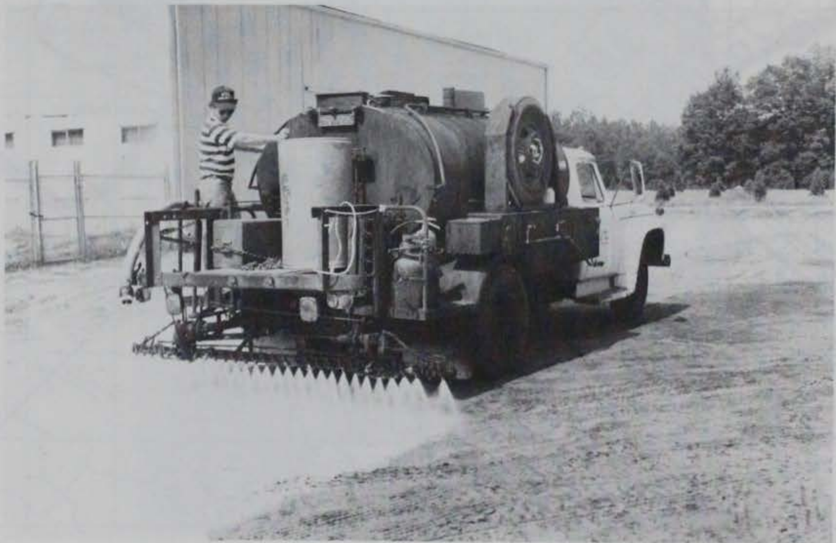
b. Applying PVA, Fort Stewart, Ga.
