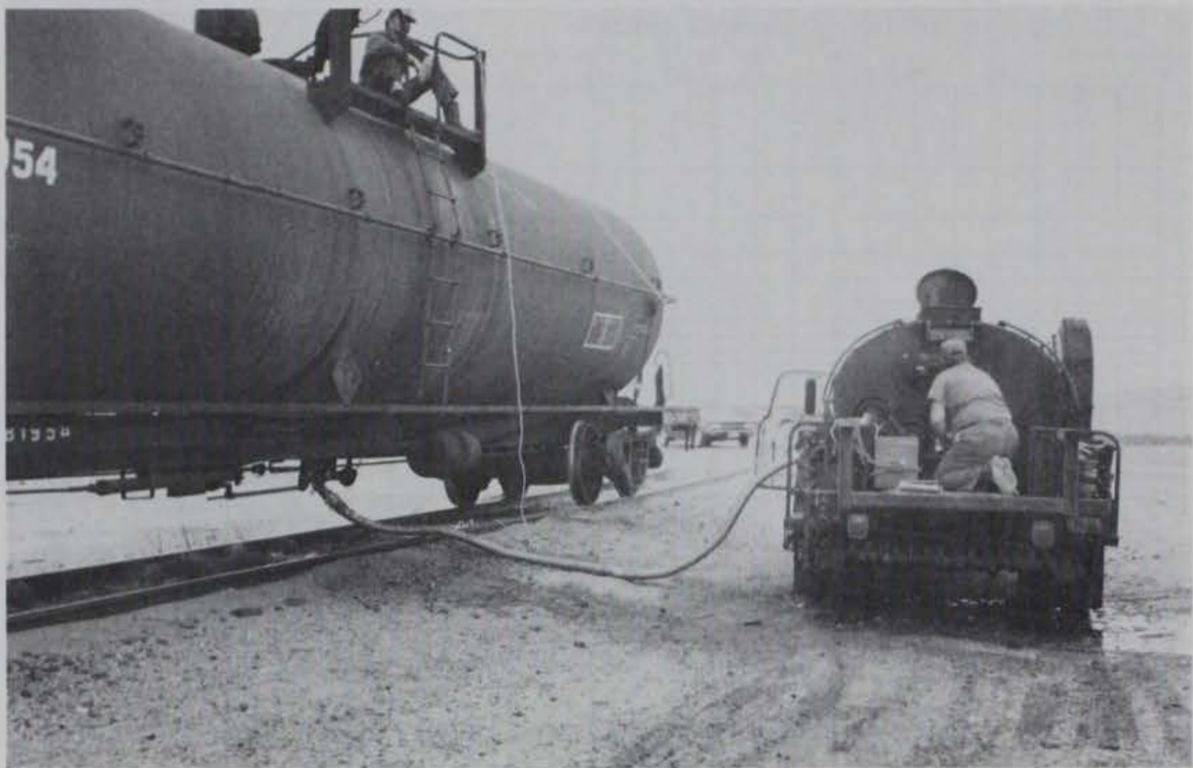
Figure 9. Loading product MgCl_2 from railroad tank car
