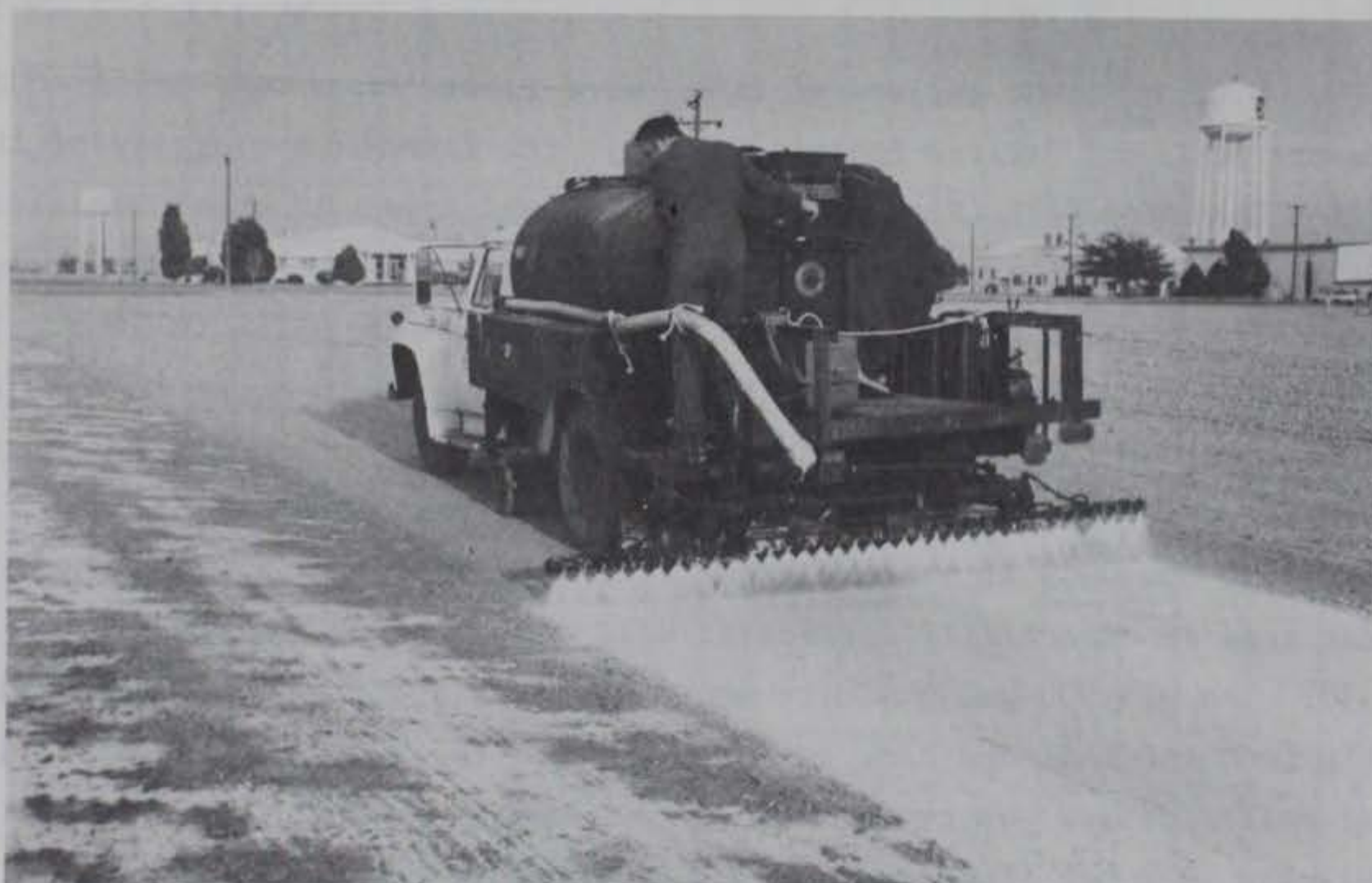
Figure 6. Applying PVA at Fort Bliss, Tex.
