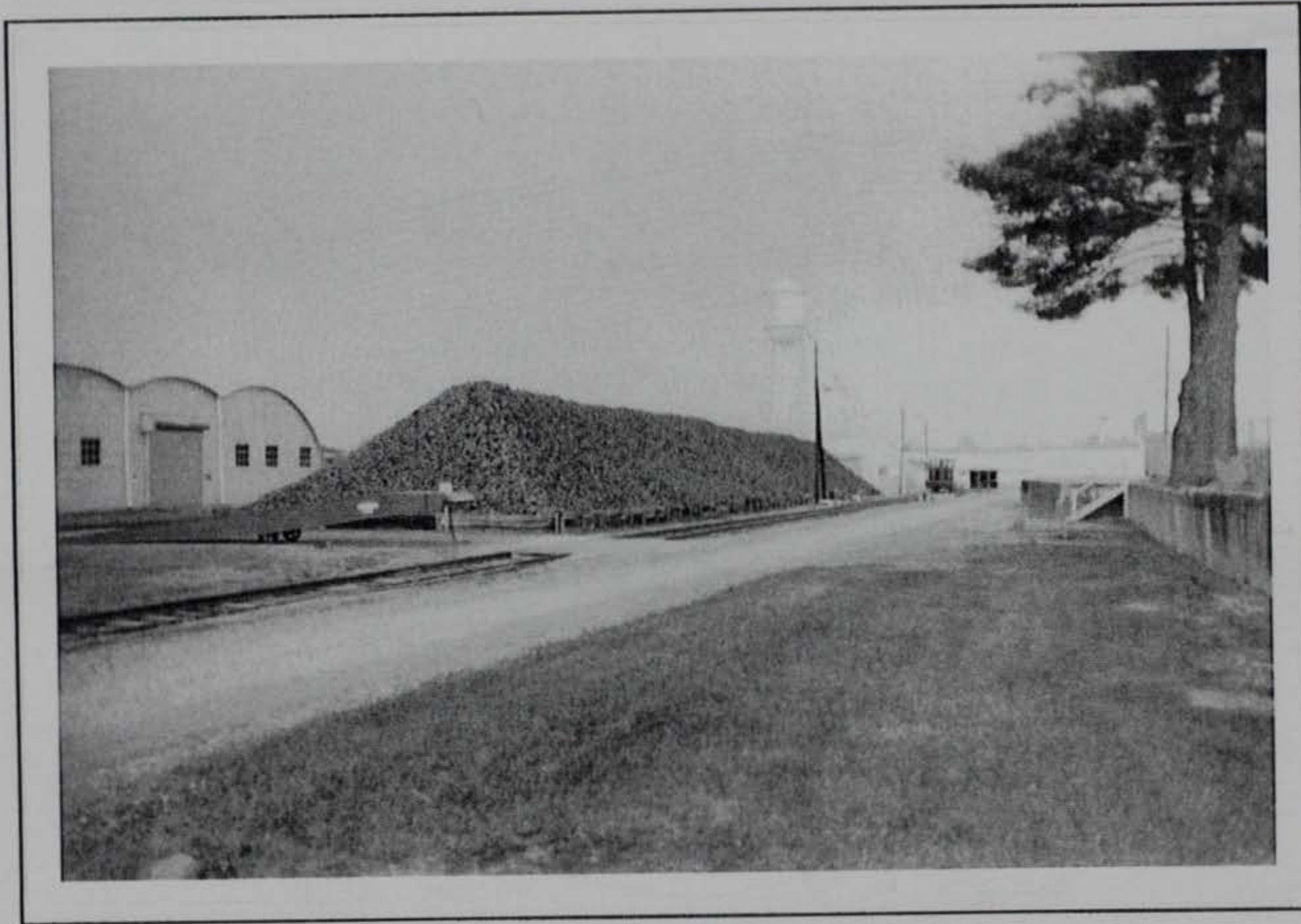
Figure E-9. Pile #59, Point Pleasant Depot, WV
