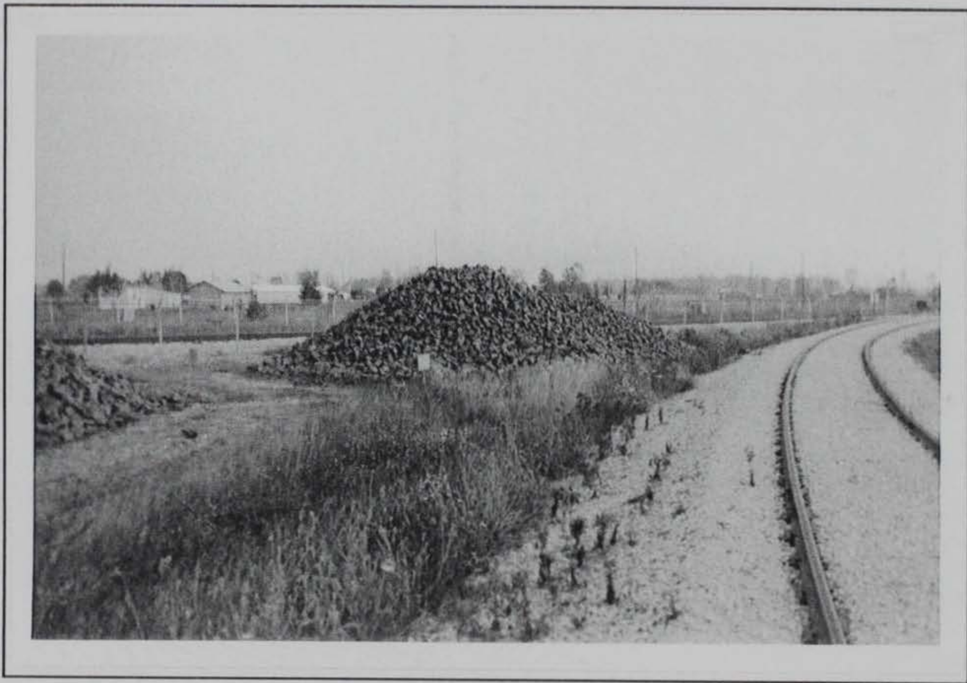
Figure B-37. Pile #38, New Haven Depot, IN
