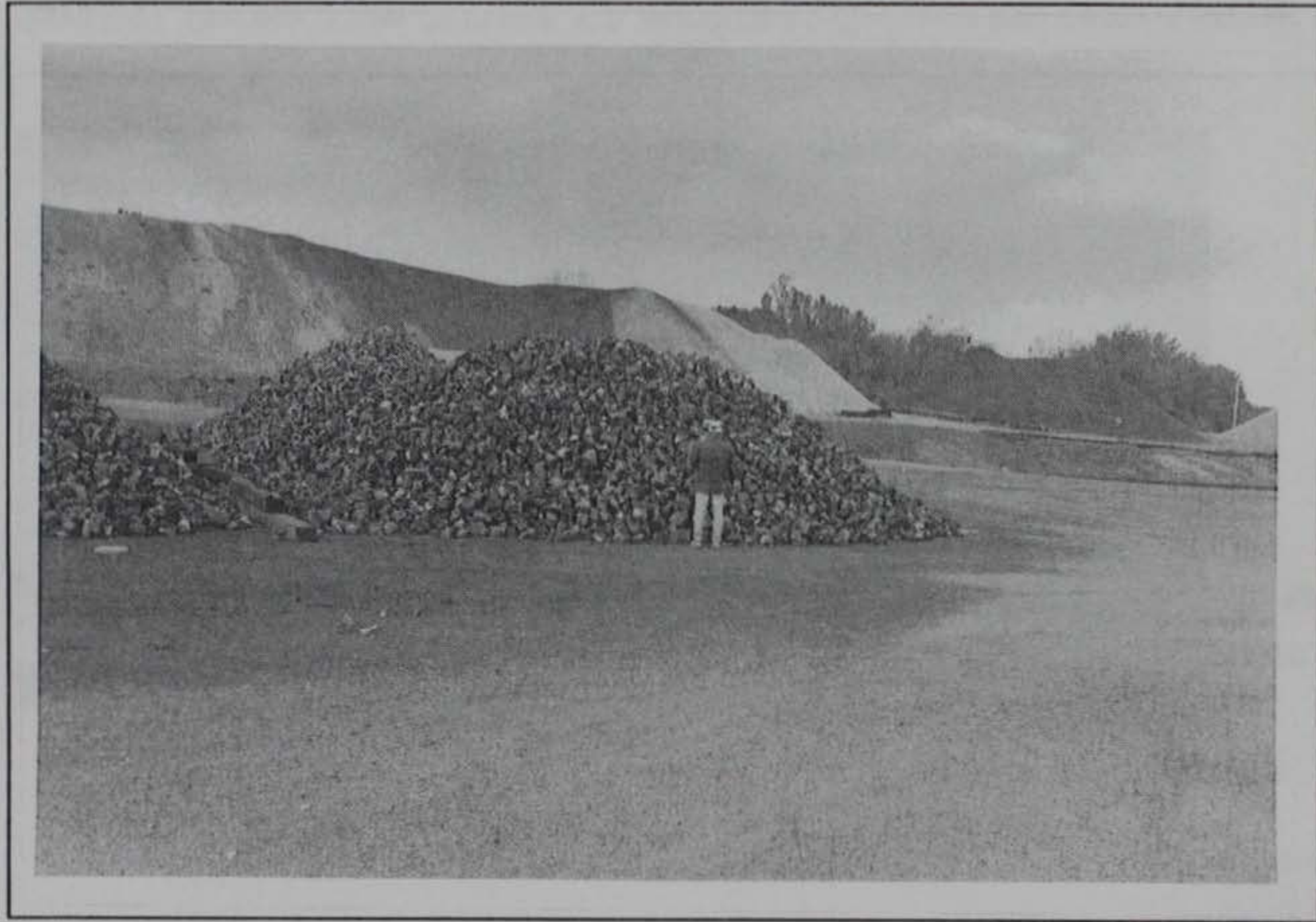
Figure C-30. Pile #6, Warren Depot, OH
