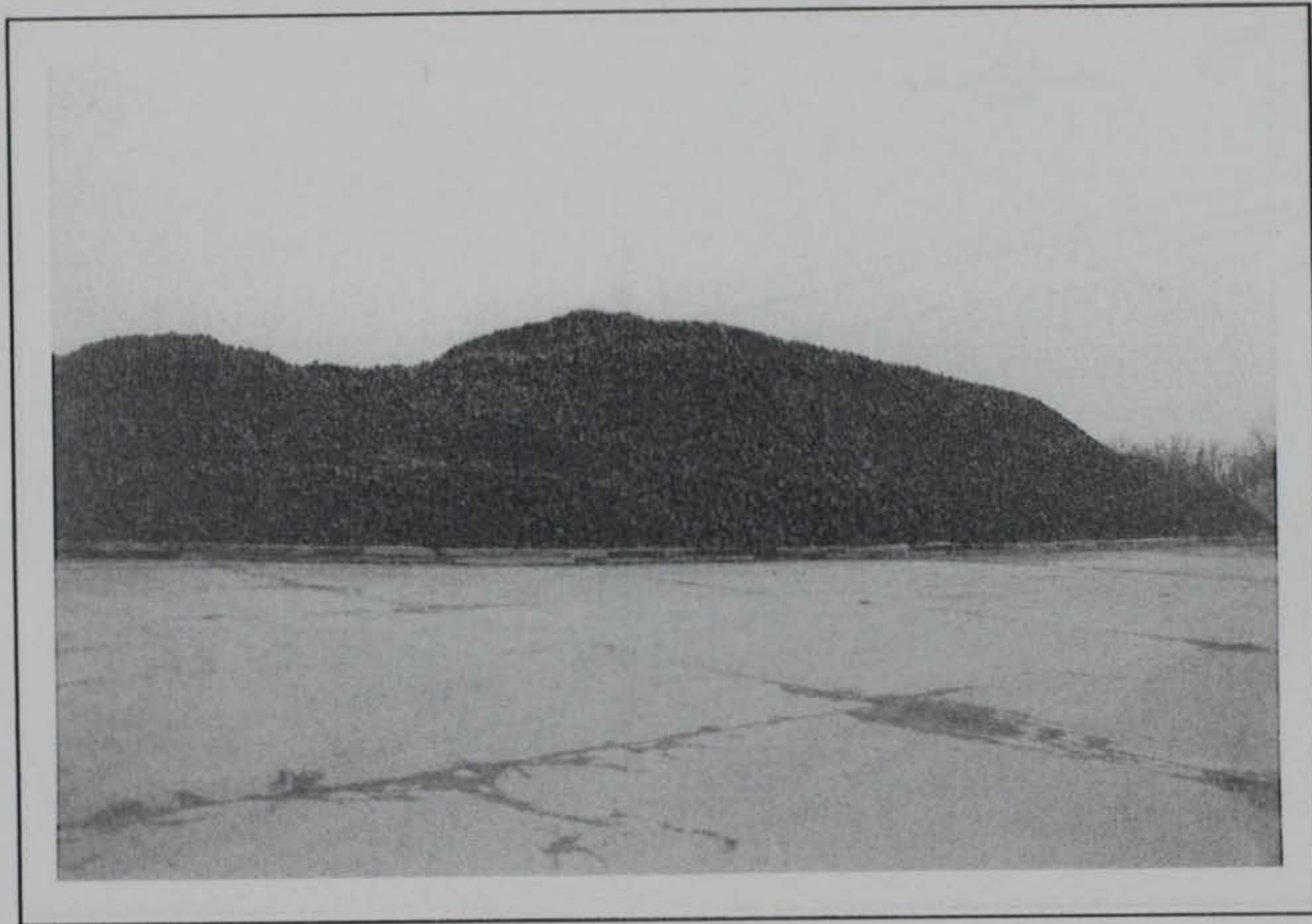
Figure D-51. Pile #27, Curtis Bay Depot, MD
