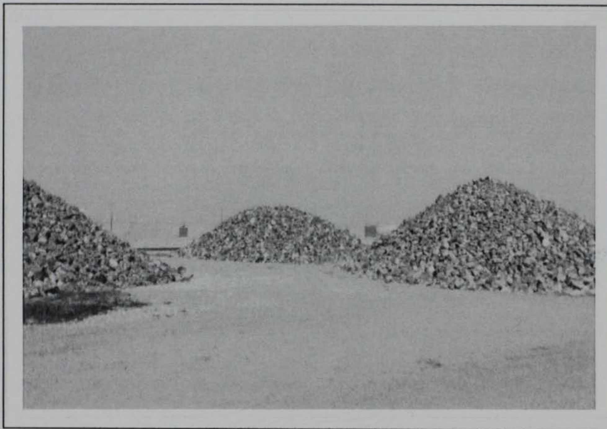
Figure B-5. Pile #13 (center back), New Haven Depot, IN
