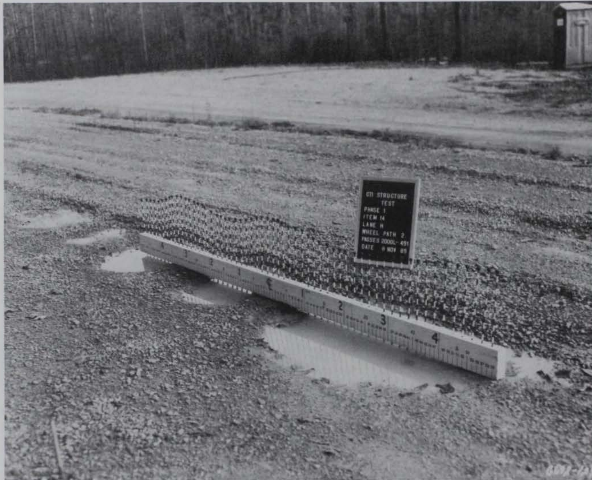
Photo 62. Item 14, high-pressure tire lane, high-severity washboarding after 491 passes during the induced failure plan
