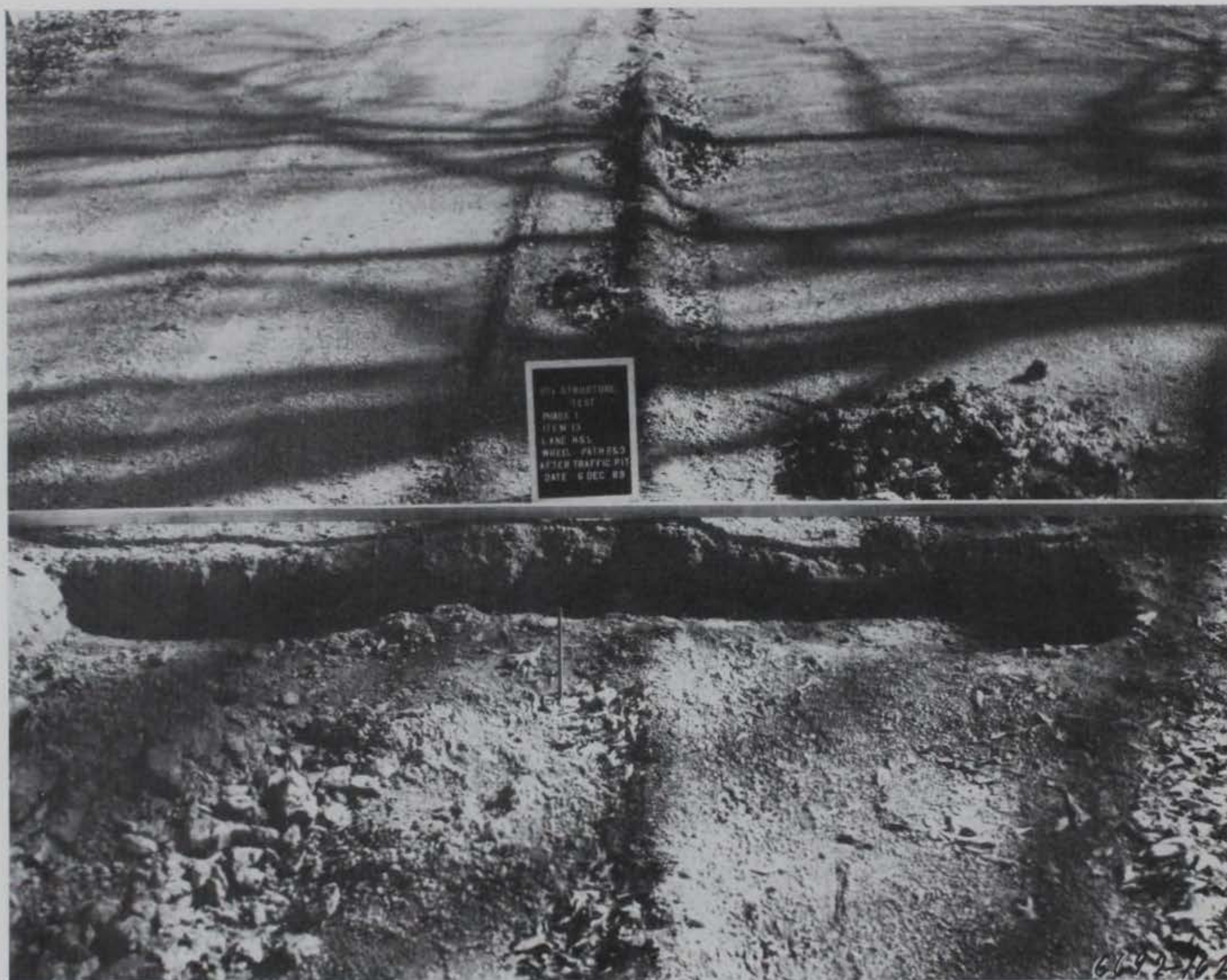
Photo 68. Item 13, general view of the post-traffic test pit
