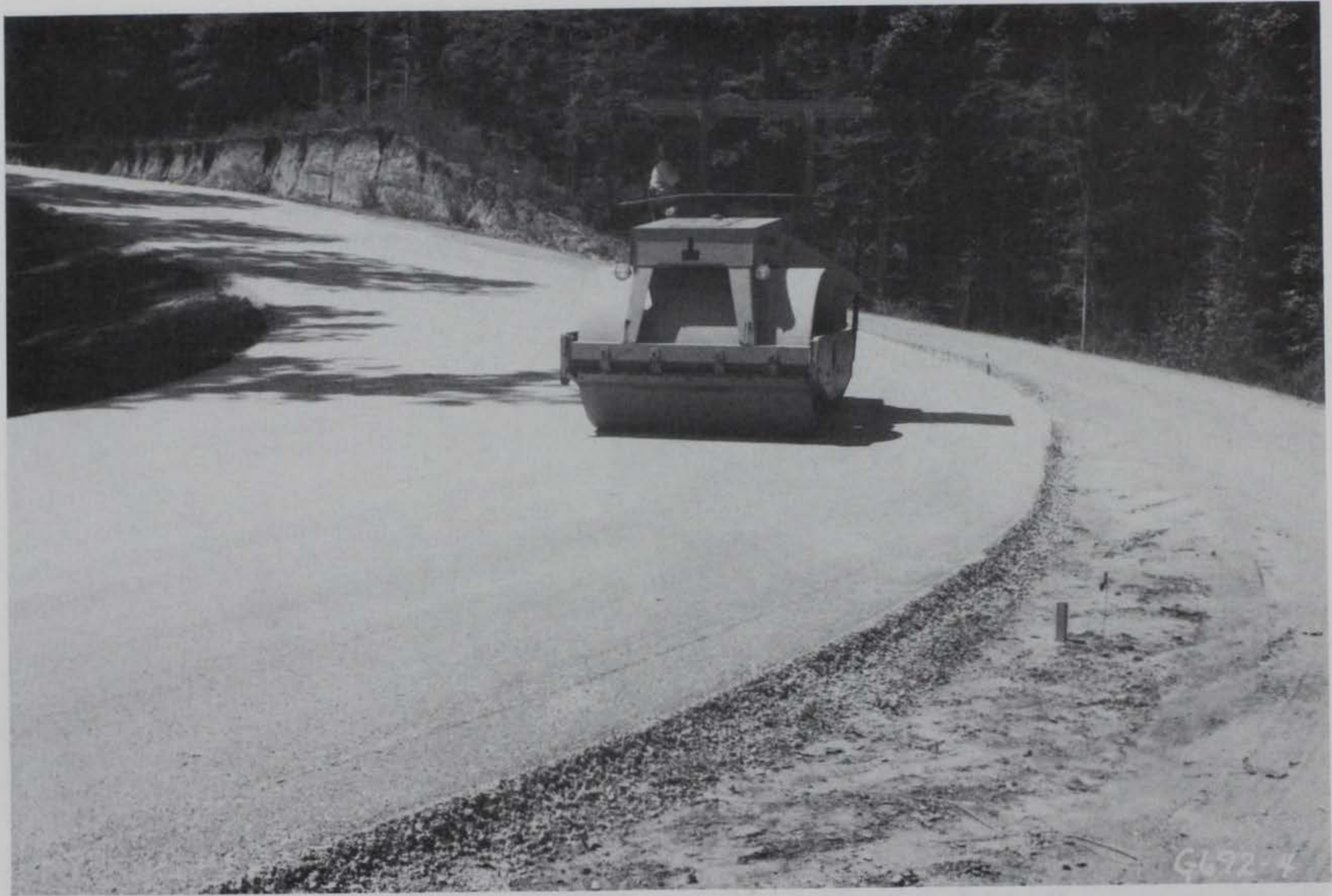
Photo 2. Compaction of the aggregate base material
