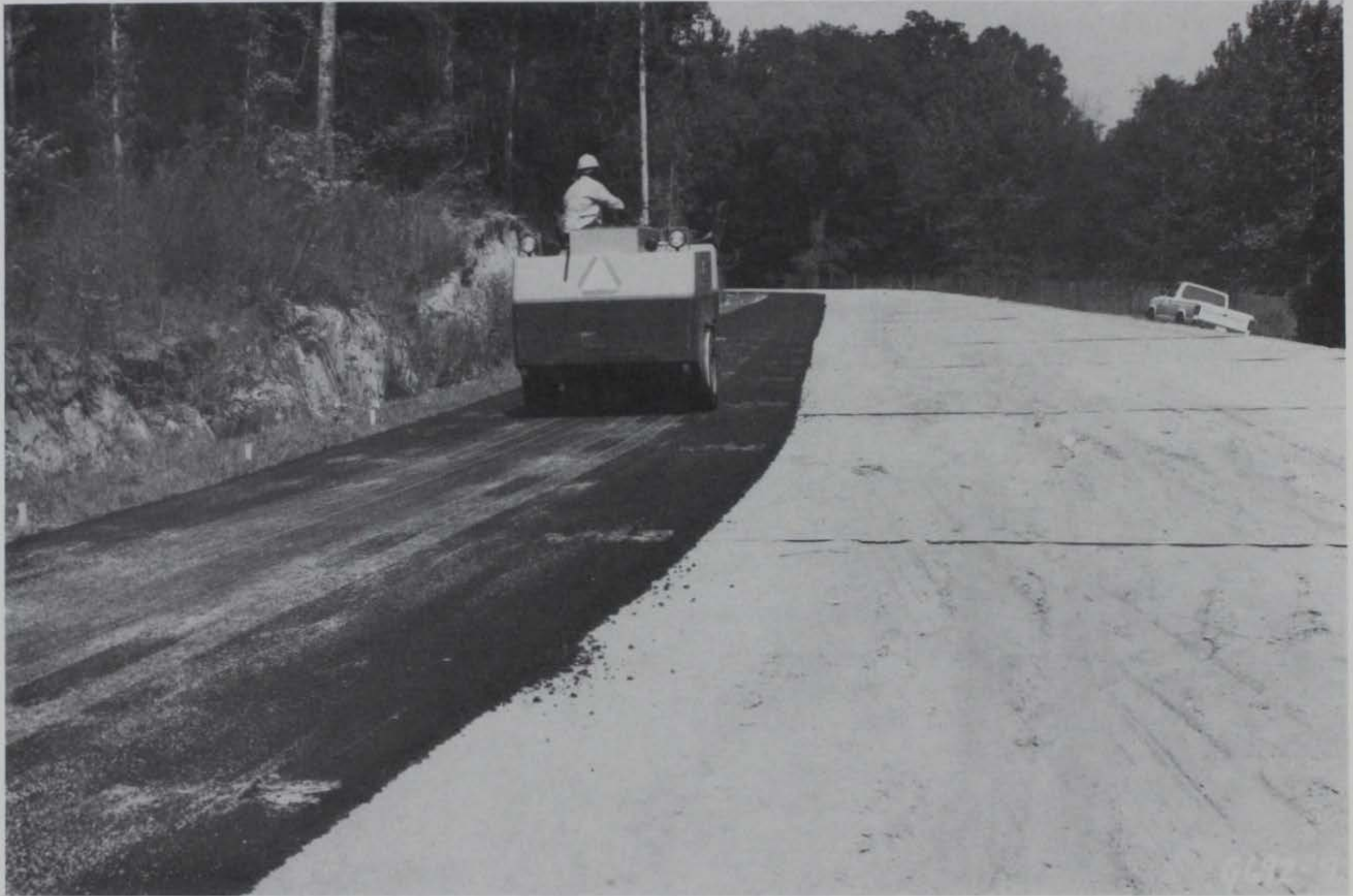
Photo 6. Compaction of the asphalt mix with a rubber-tired roller
