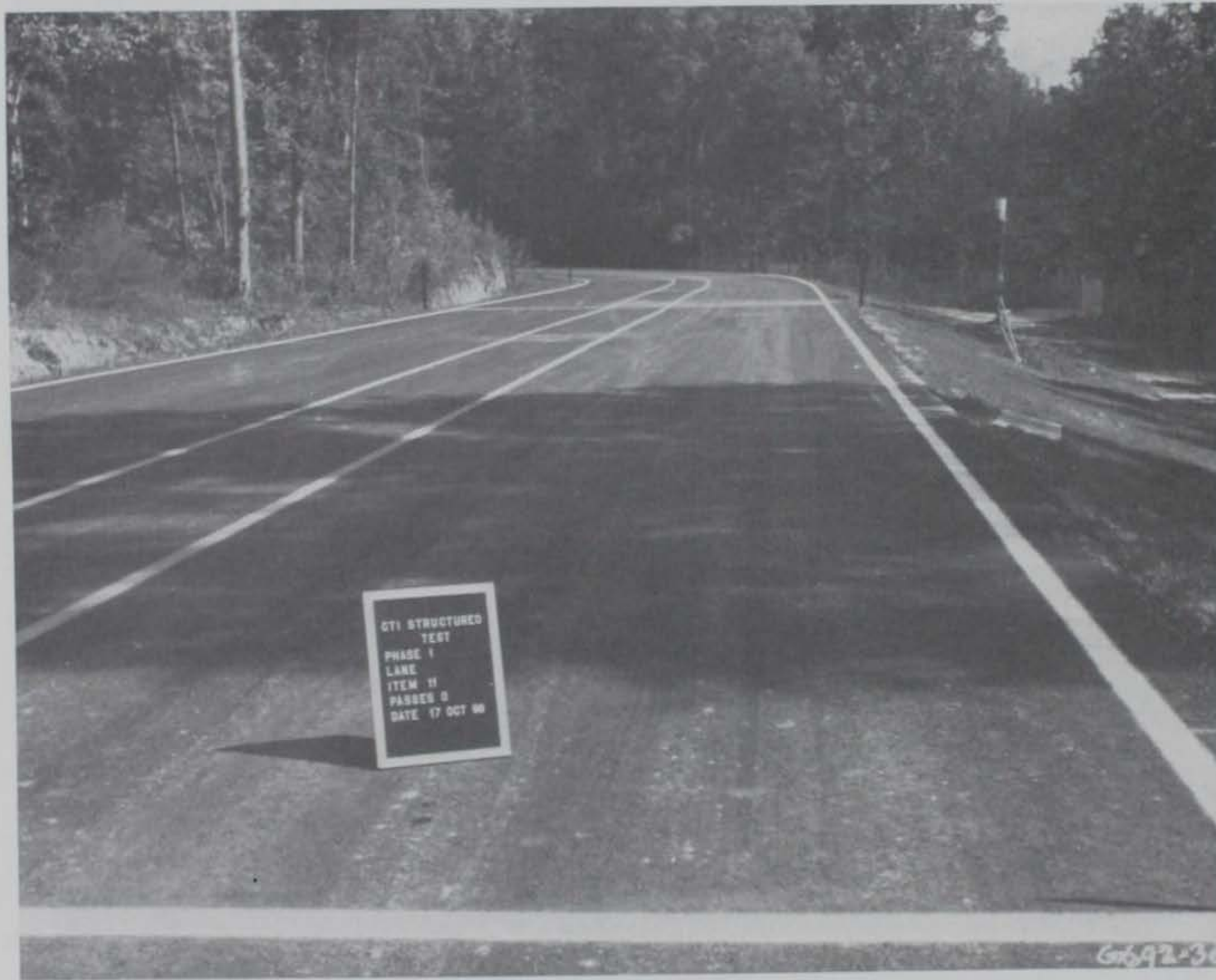
Photo 29. Item 11, general view before traffic
