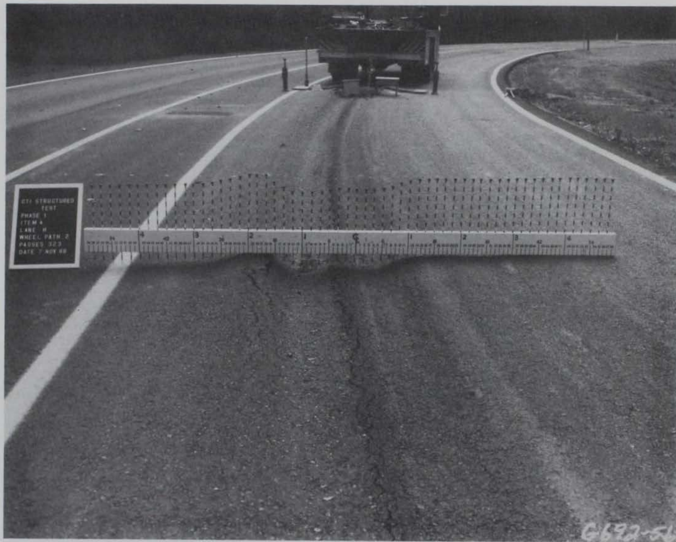
Photo 14. Item 4, wheel path 2, general view of second failure, 323 passes
