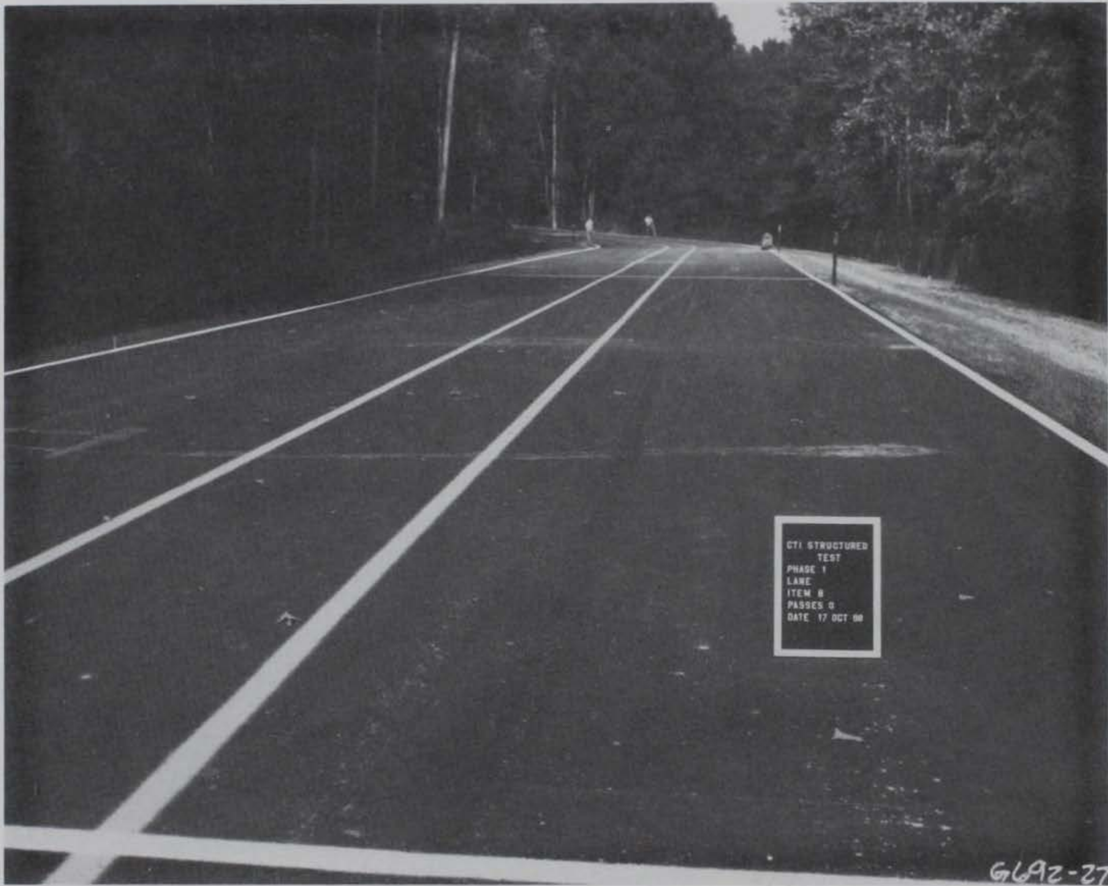
Photo 26. Item 8, general view before traffic
