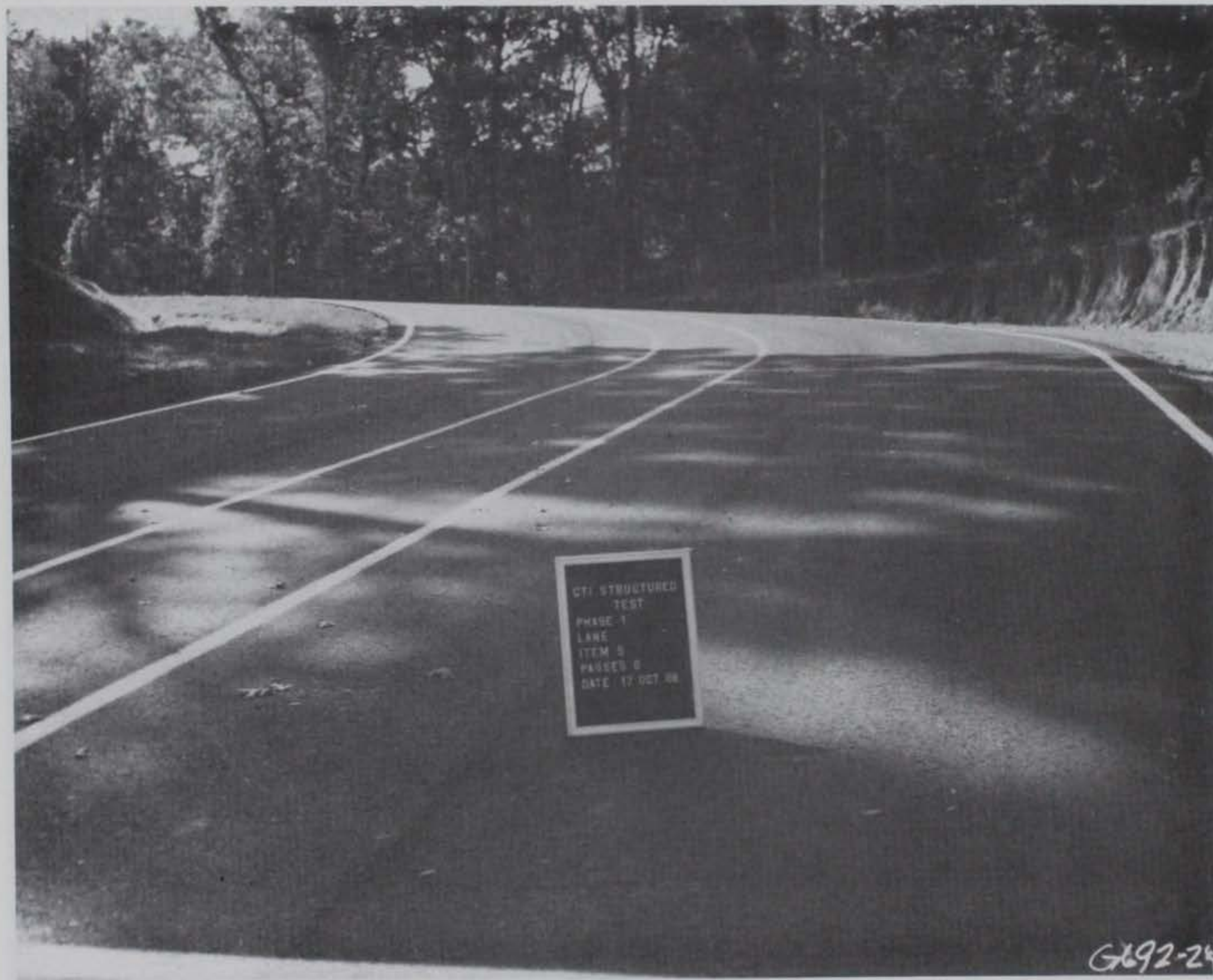
Photo 11. General view of Item 5 before traffic
