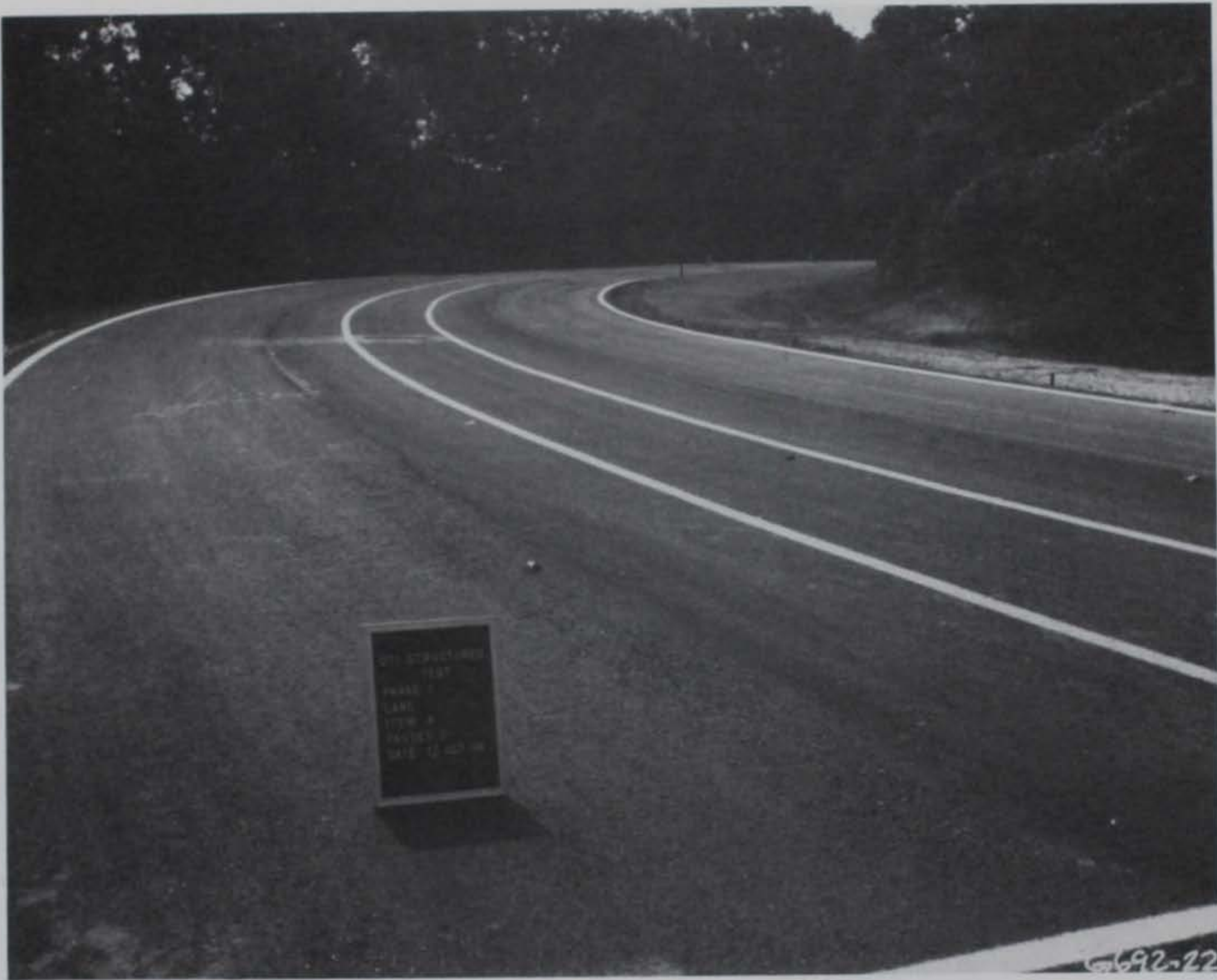
Photo 10. General view of Item 4 before traffic
