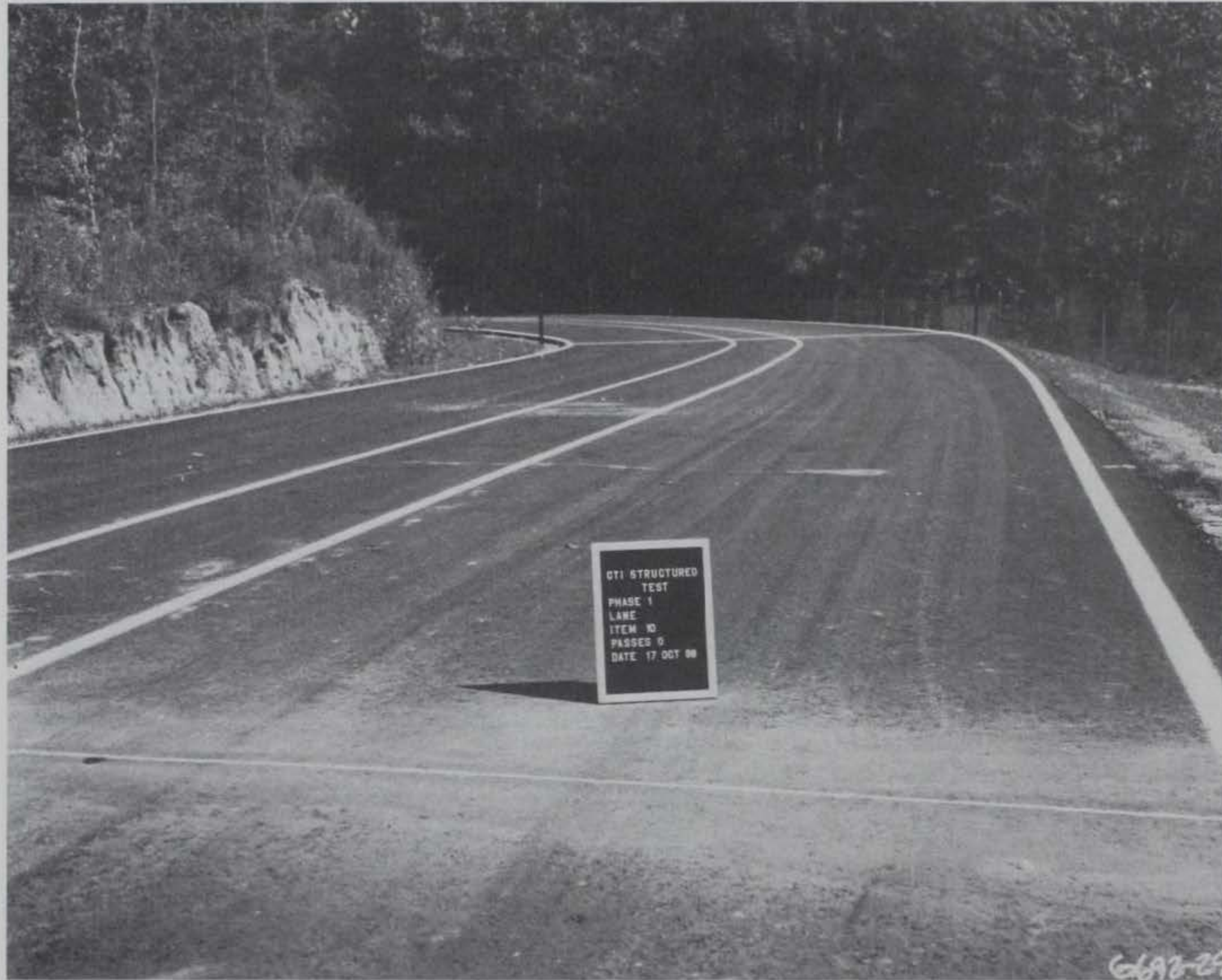
Photo 28. Item 10, general view before traffic
