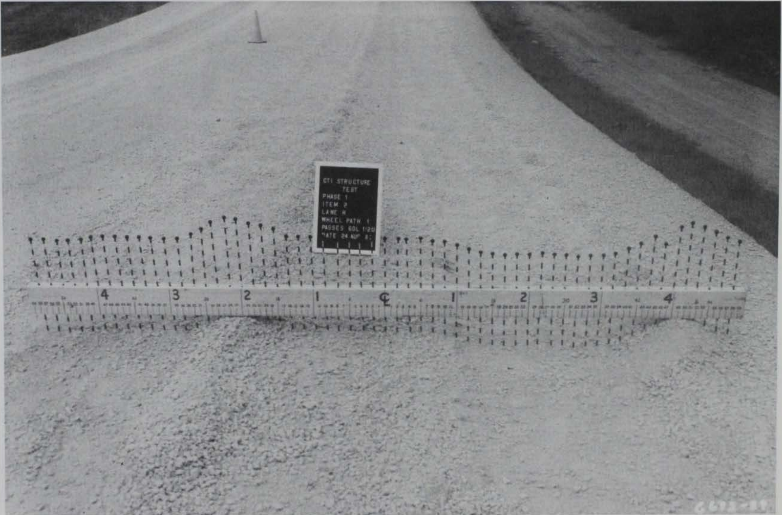
Photo 47. Item 2, high-pressure tire lane, failure after 112 unloaded passes
