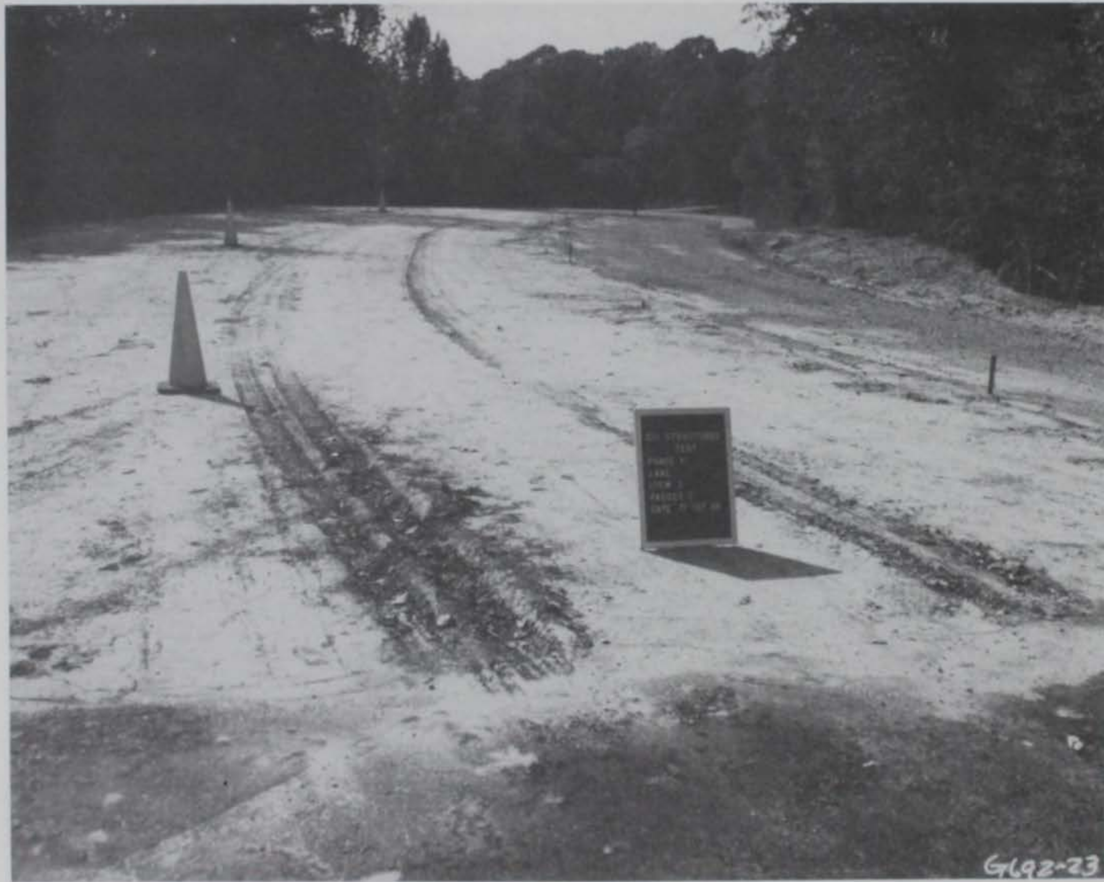
Photo 37. Item 3, general view before traffic
