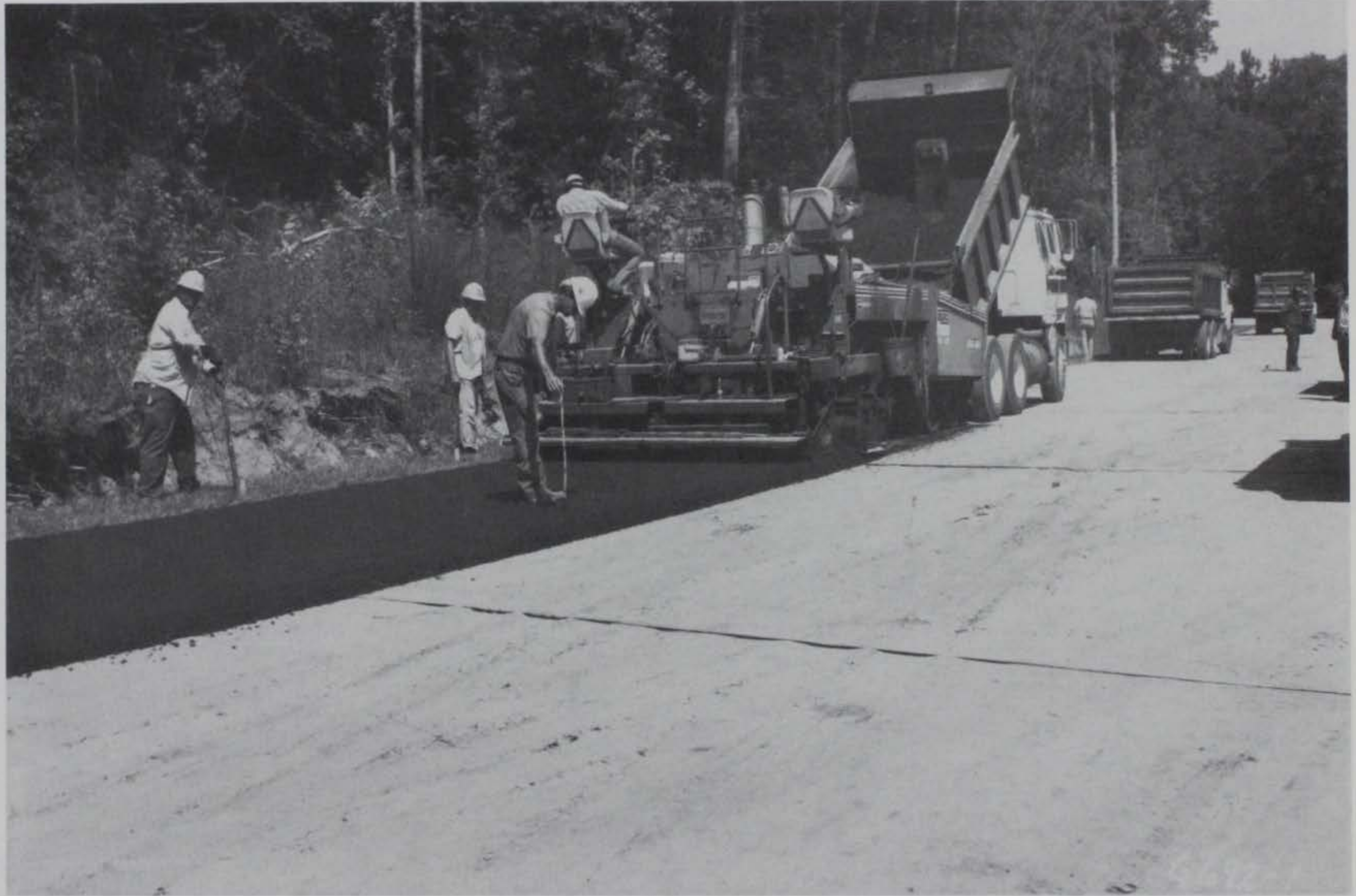
Photo 4. Placement of the asphalt concrete
