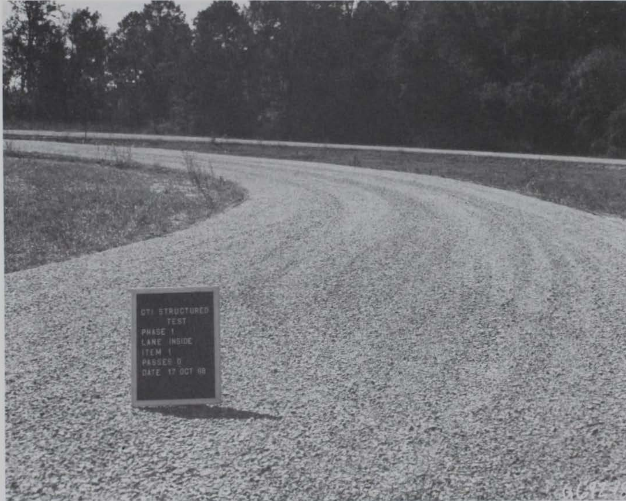
Photo 35. Item 1, low-pressure tire lane, general view before traffic
