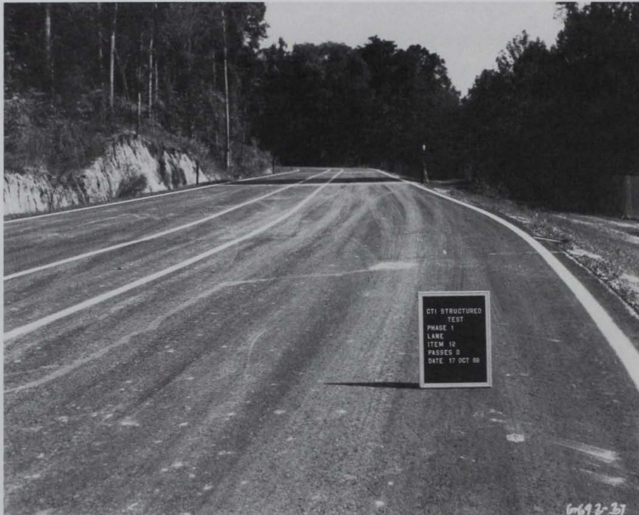
Photo 30. Item 12, general view before traffic
