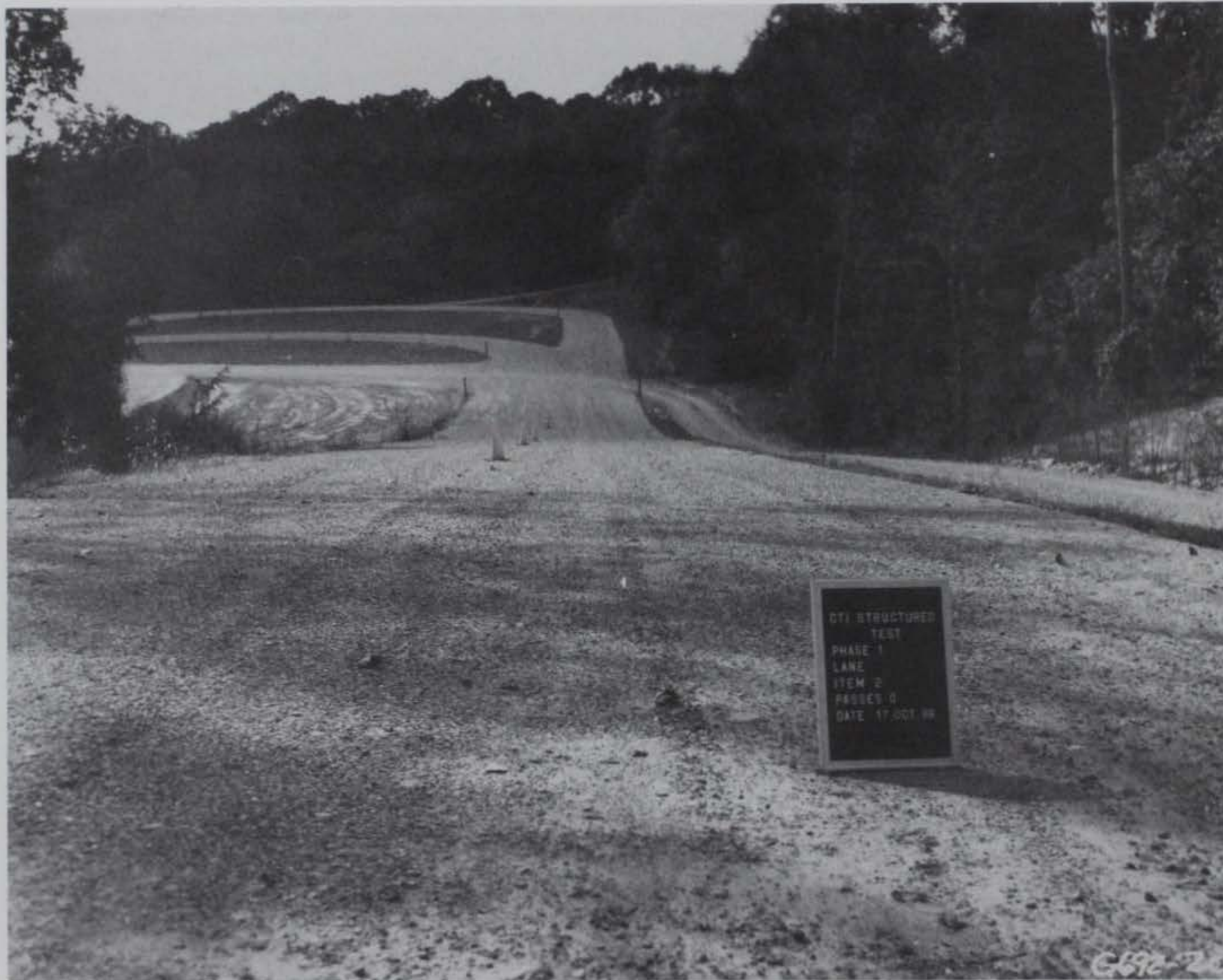
Photo 36. Item 2, general view before traffic
