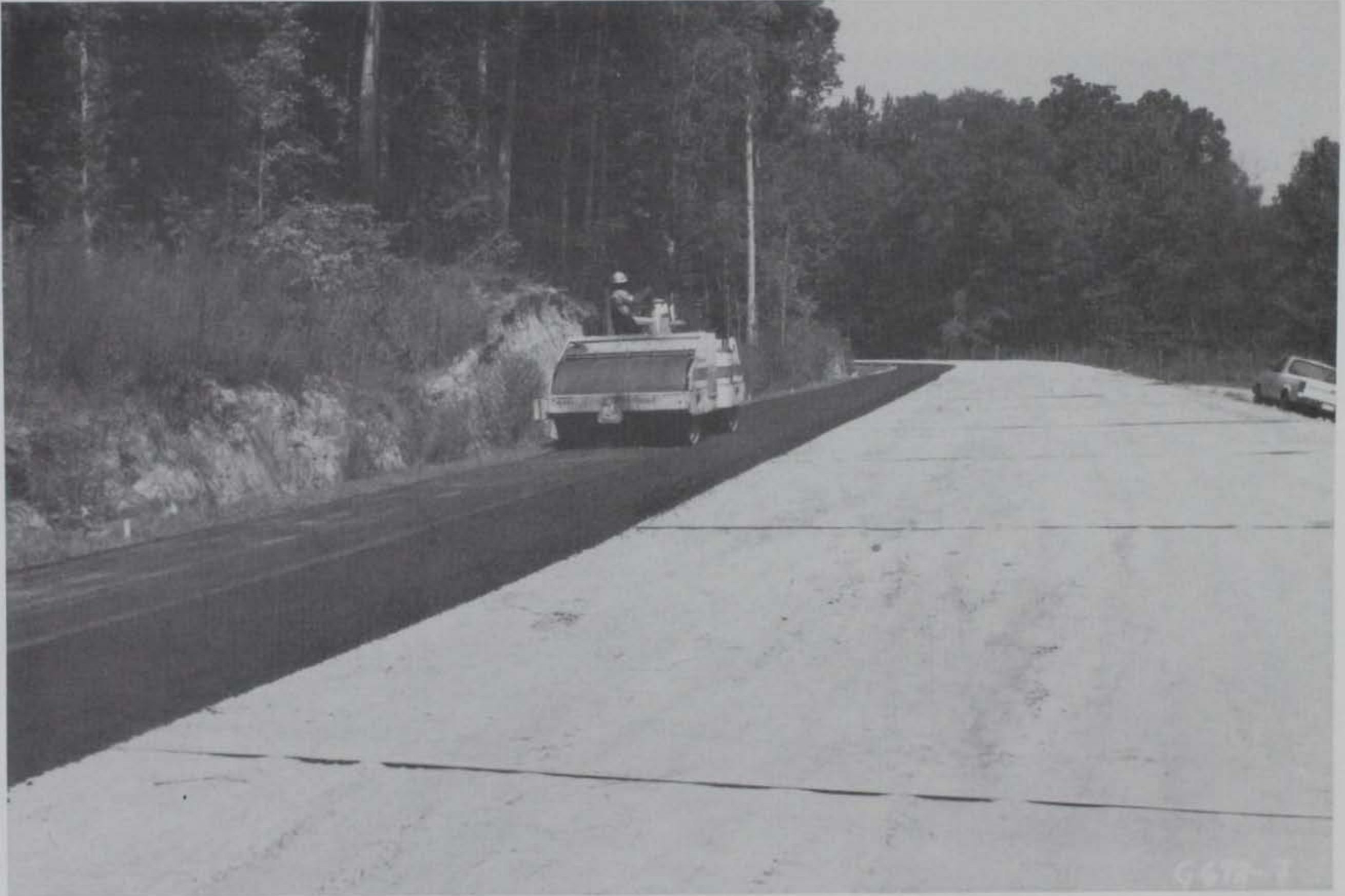
Photo 5. Breakdown rolling of the hot asphalt mix
