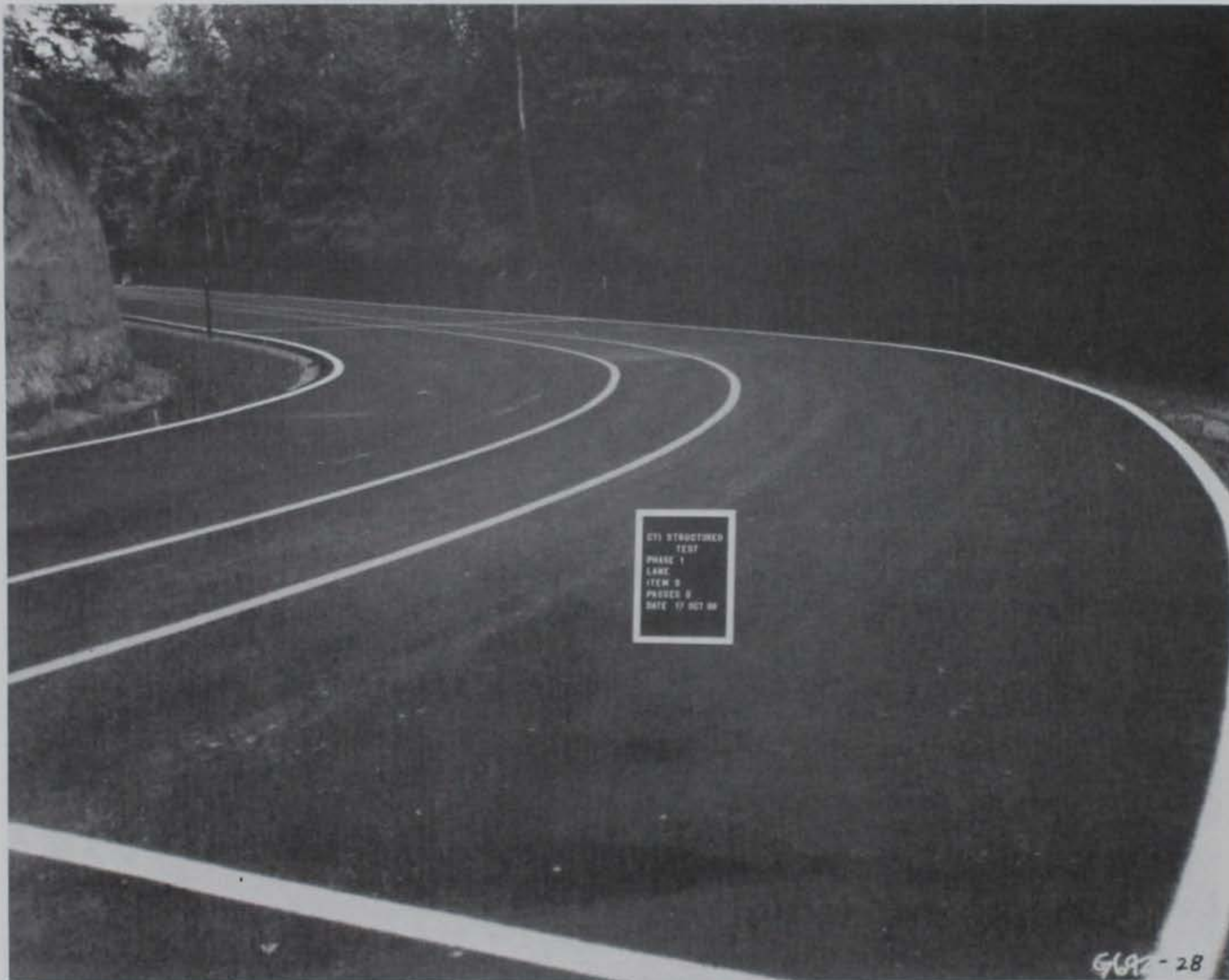
Photo 27. Item 9, general view before traffic
