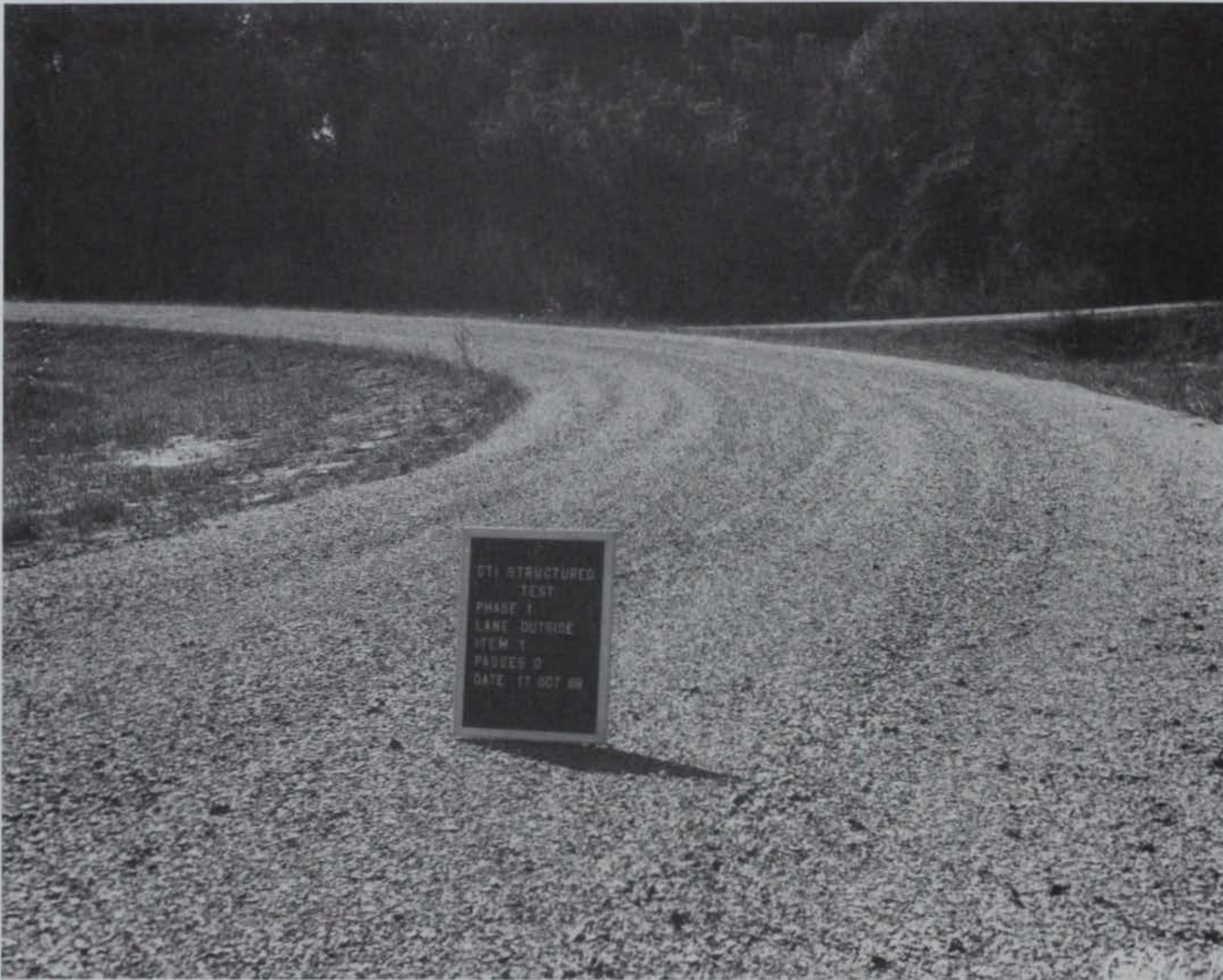
Photo 34. Item 1, high-pressure tire lane, general view before traffic
