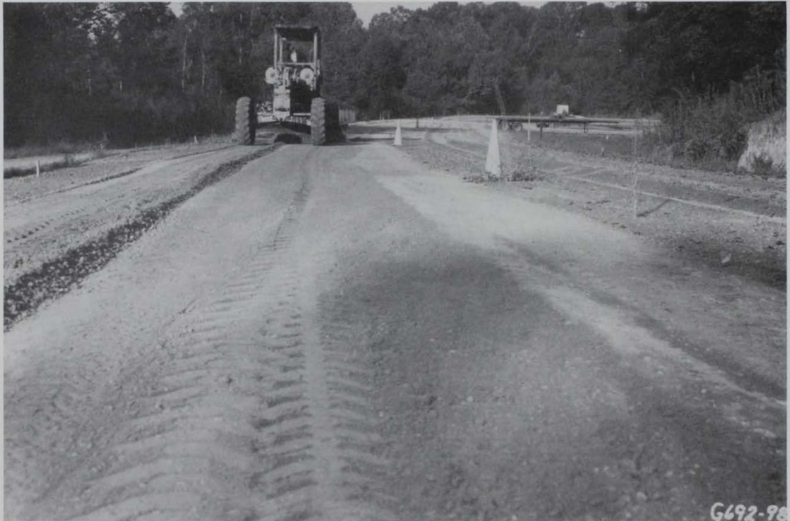
Photo 54. Grading both lanes of Items 13, 14, and 15
