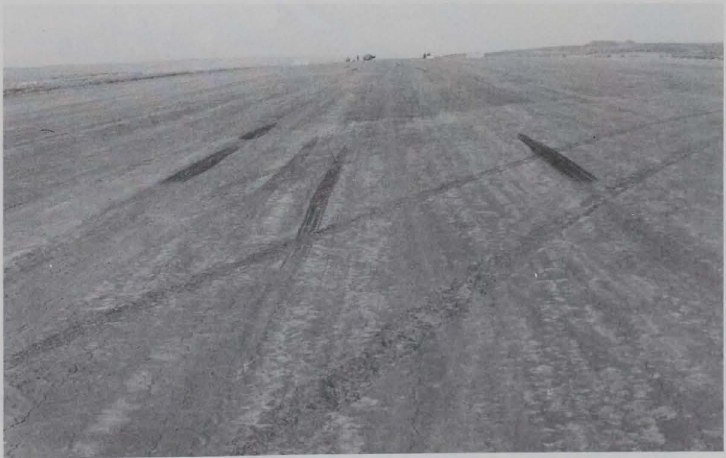
Figure 32. Black skid marks from the C-130 landing gear
