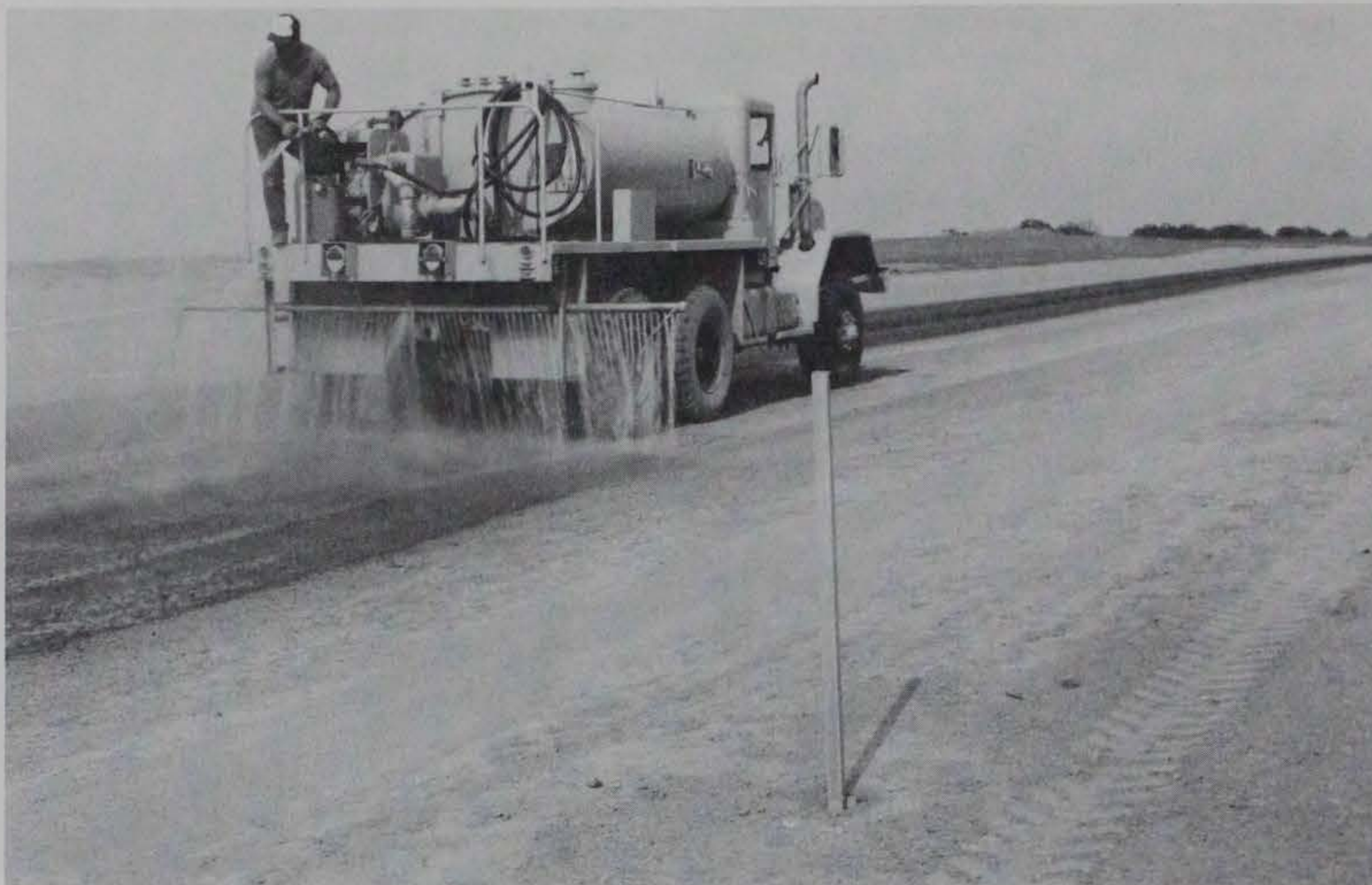
Figure 21. Prewetting the airstrip surface with a 1,000-gal water truck
