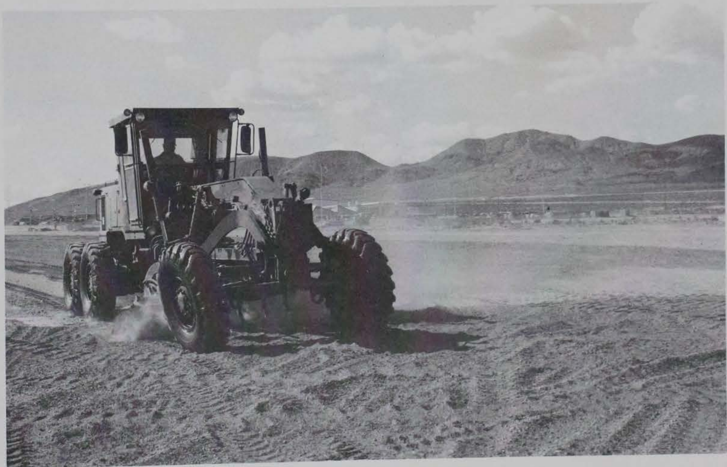
Figure 13. Motor grader removing loose excess surface material
