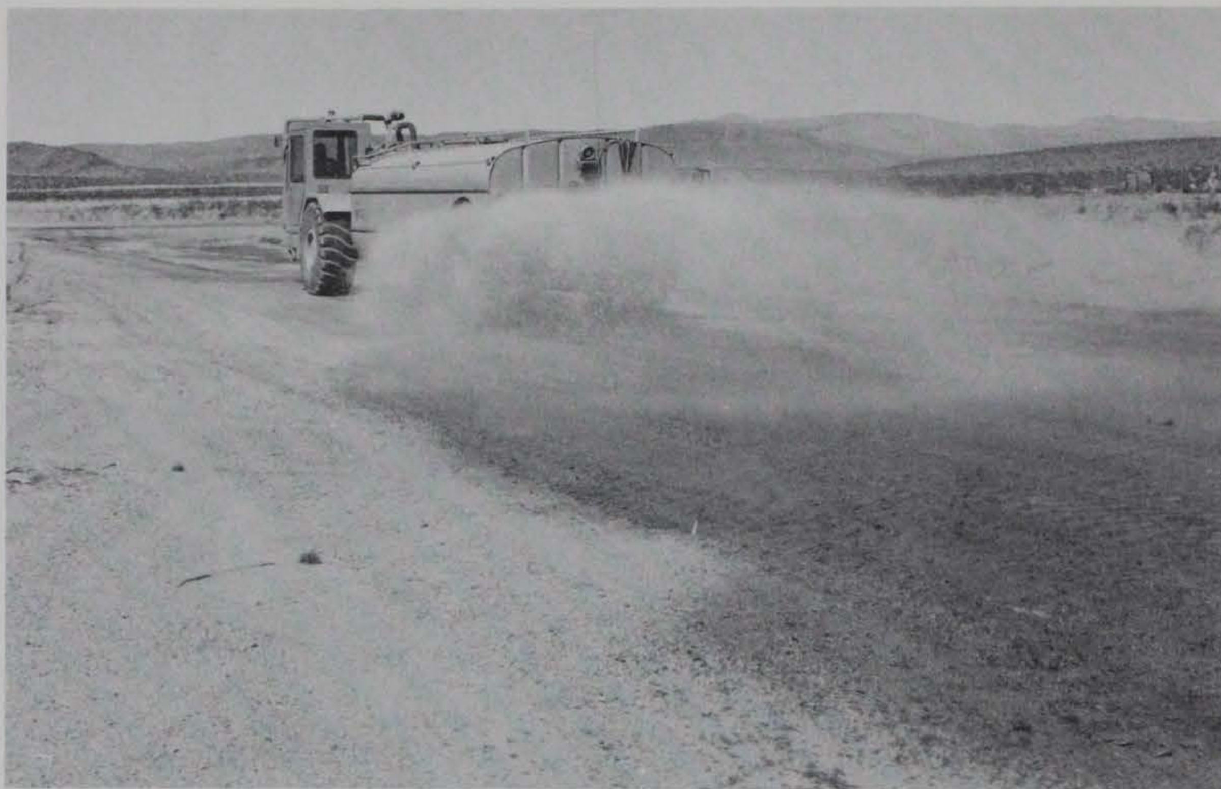
Figure 14. A 5,000-gal water truck prewetting area to be treated
