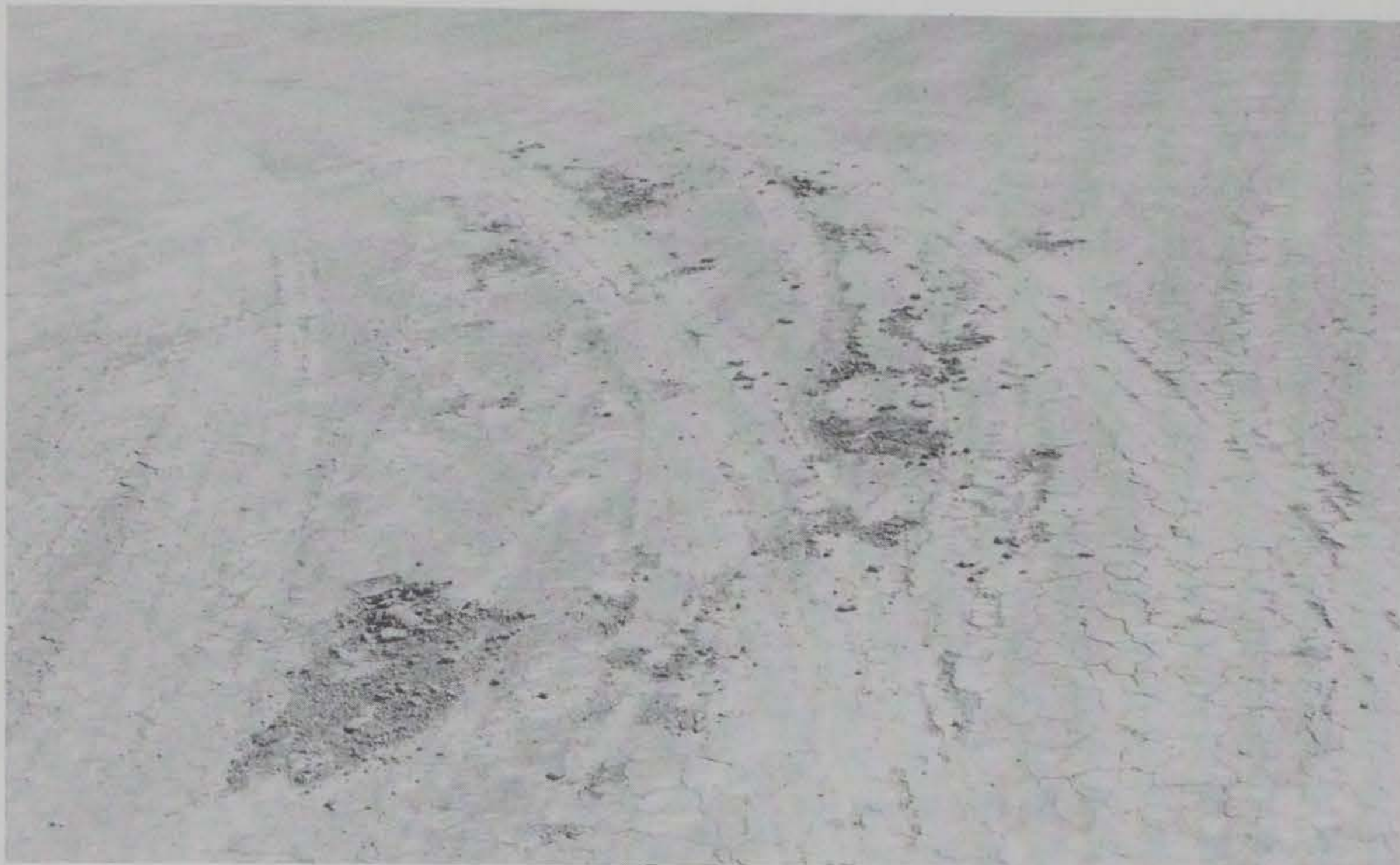
Figure 35. Nose gear ruts at the entrance to the parking apron
