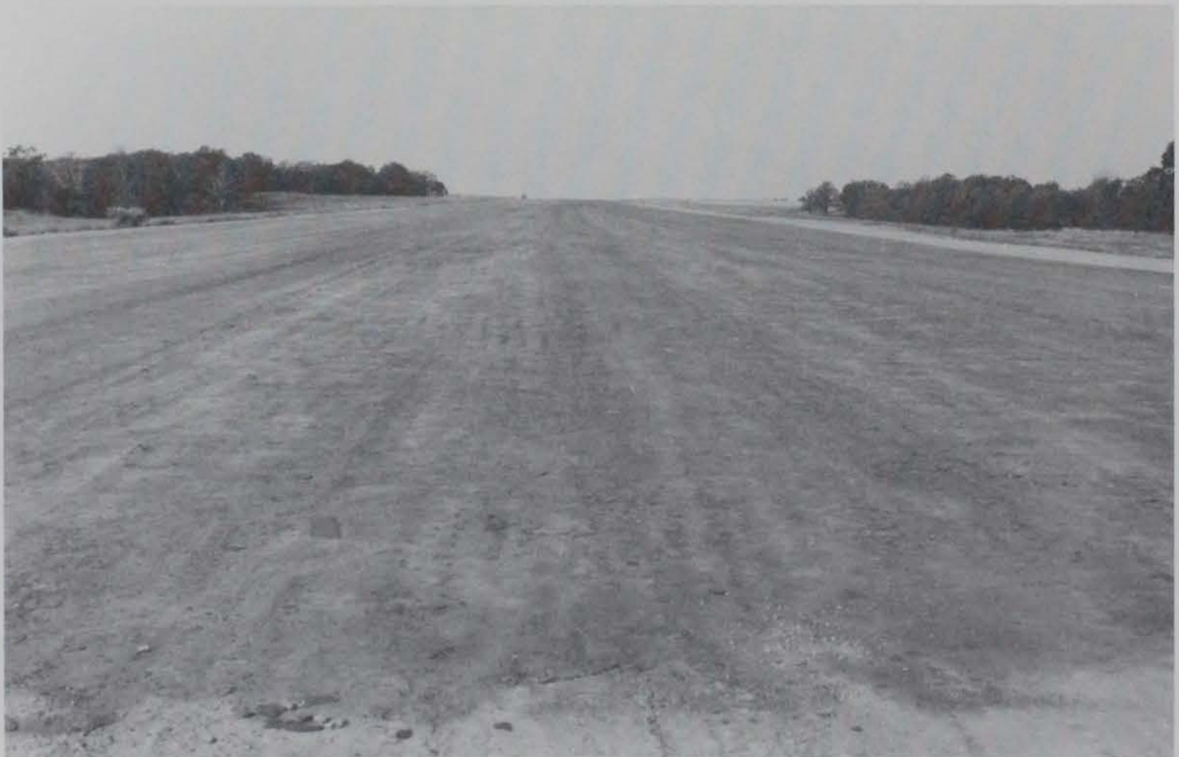
Figure 26. East end of airstrip looking west
