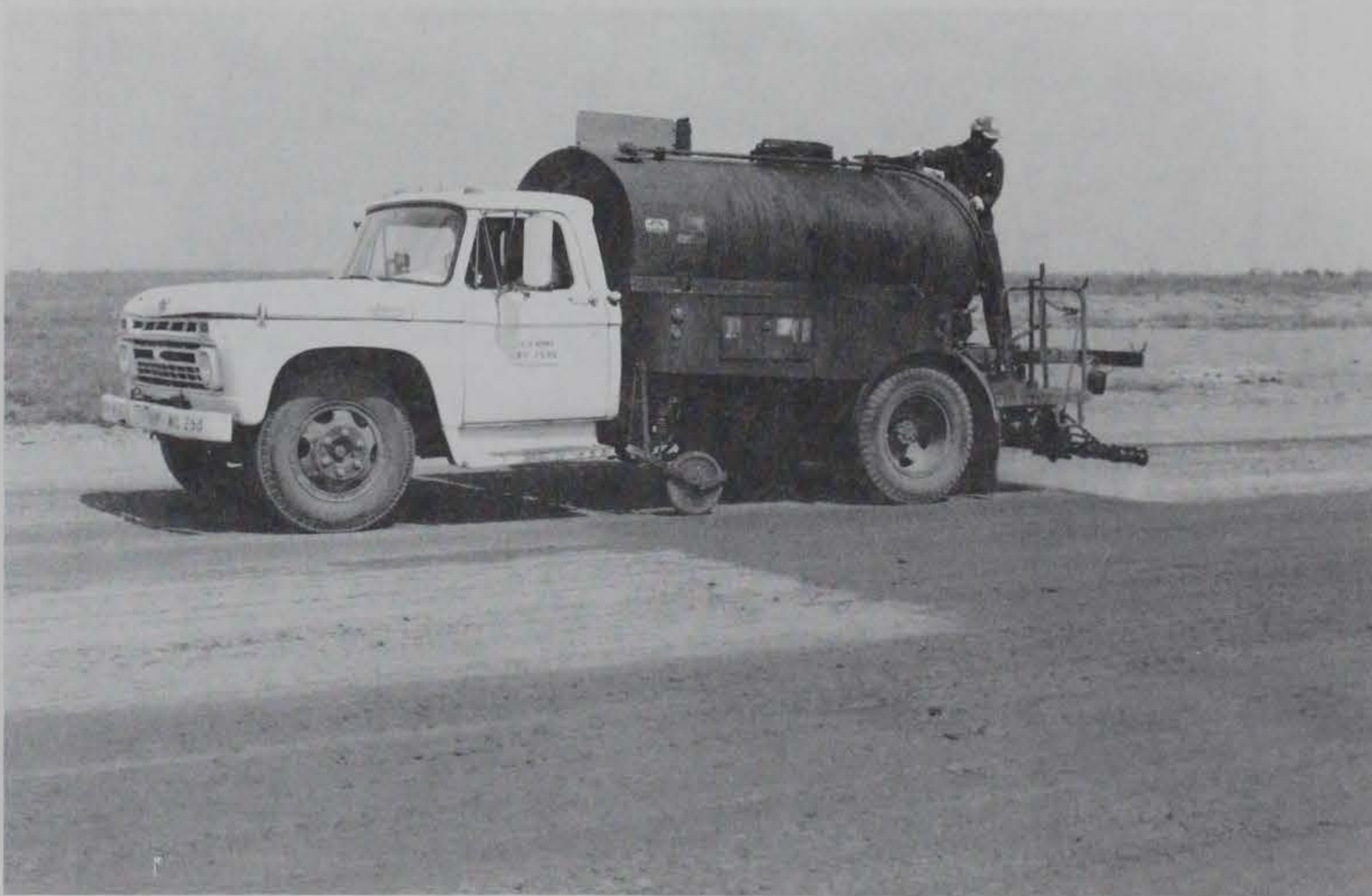
Figure 22. WES modified asphalt distributor applying MgCl_2 at Fort Chaffee
