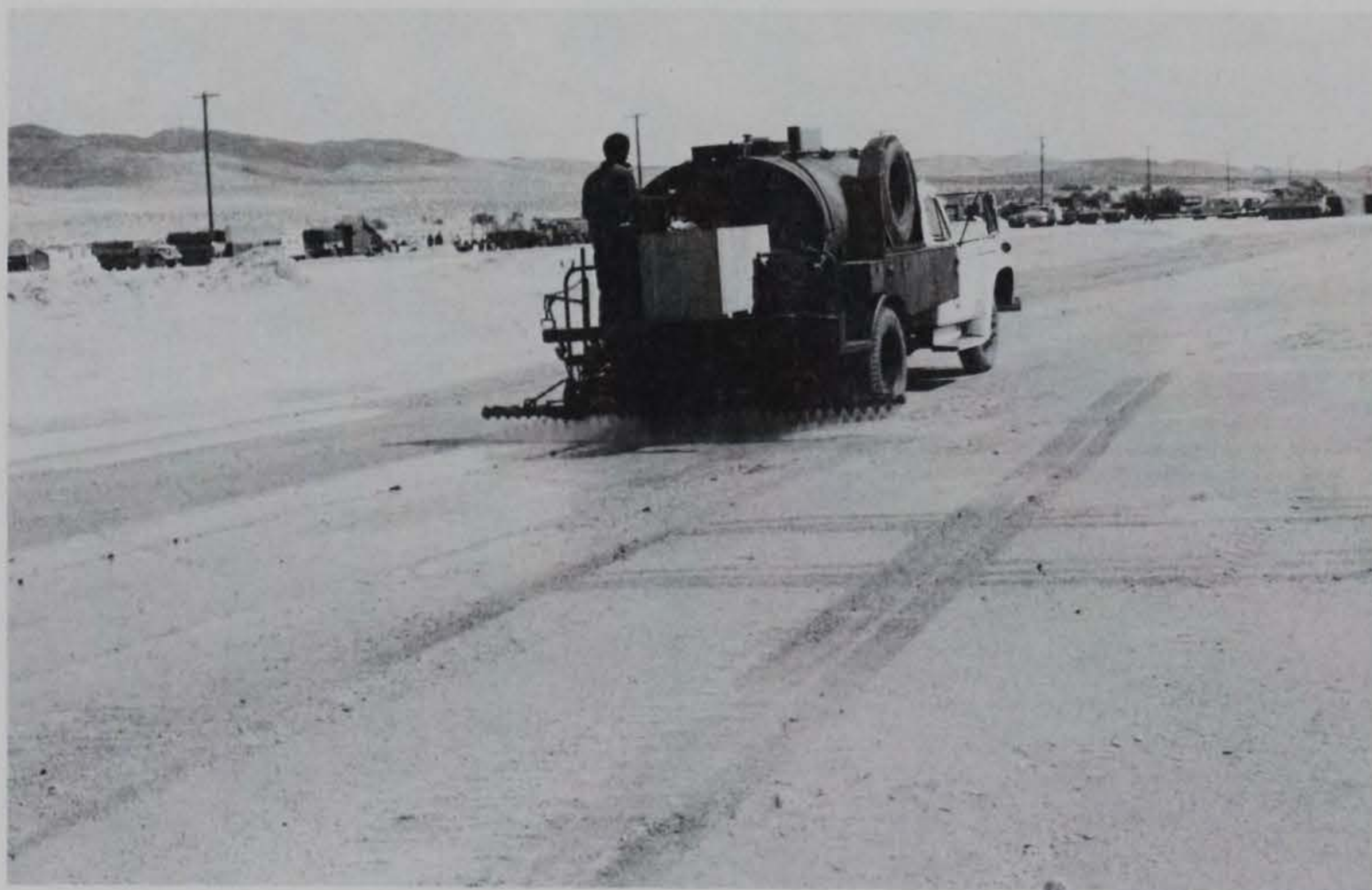
Figure 15. WES modified asphalt distributor applying MgCl_2 at Fort Irwin
