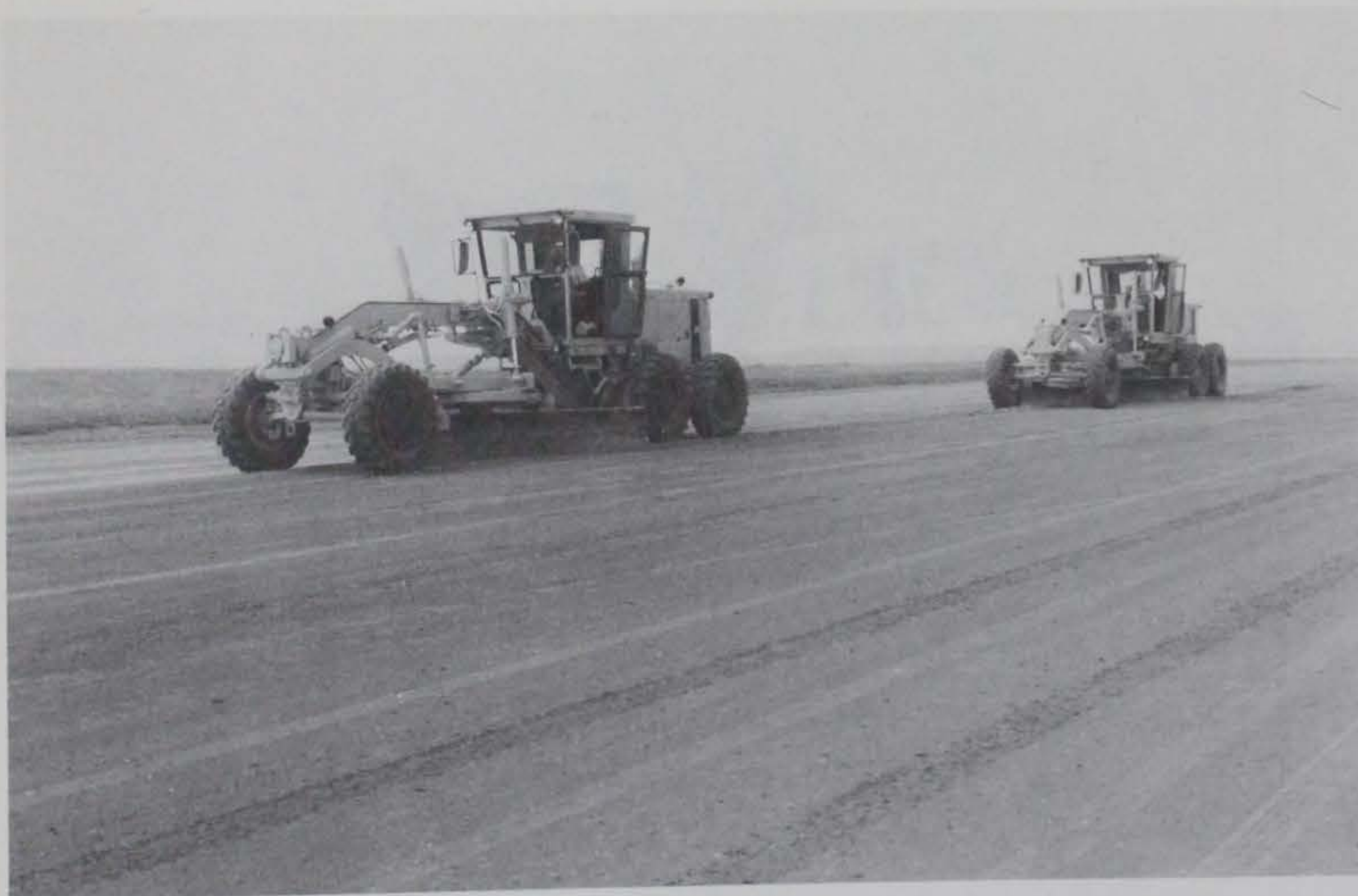
Figure 20. Motor graders operating in tandem removing excess surface material and ruts
