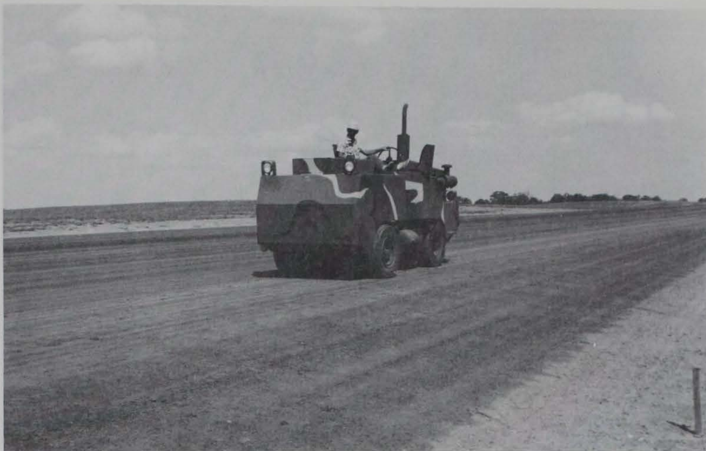
Figure 23. Pneumatic rubber-tired roller compacting the MgCl_2 treated airstrip surface
