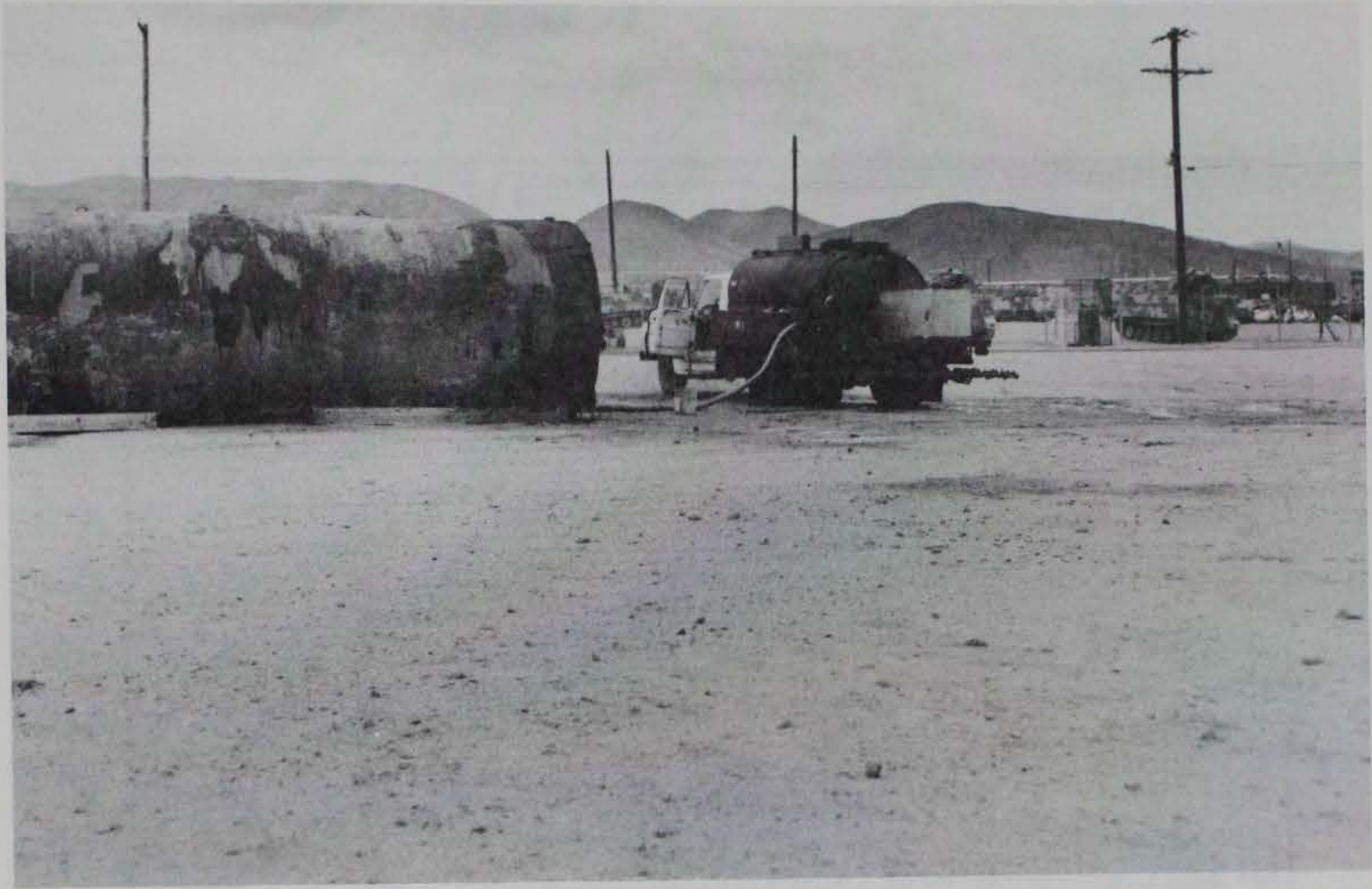
Figure 16. WES distributor loading MgCl_2 from storage tanks
