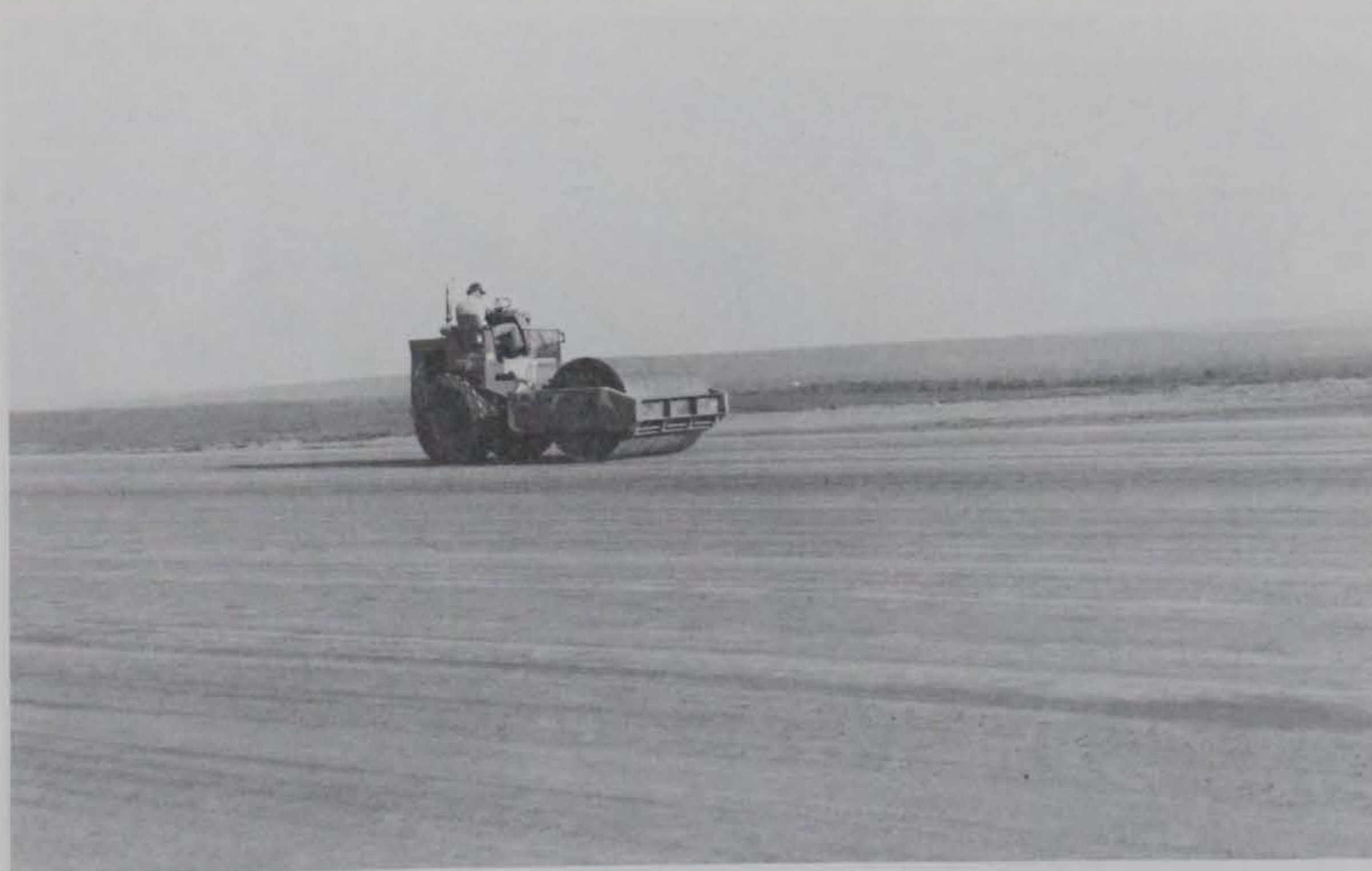
Figure 24. Steel wheel roller completing the finish rolling of the airstrip
