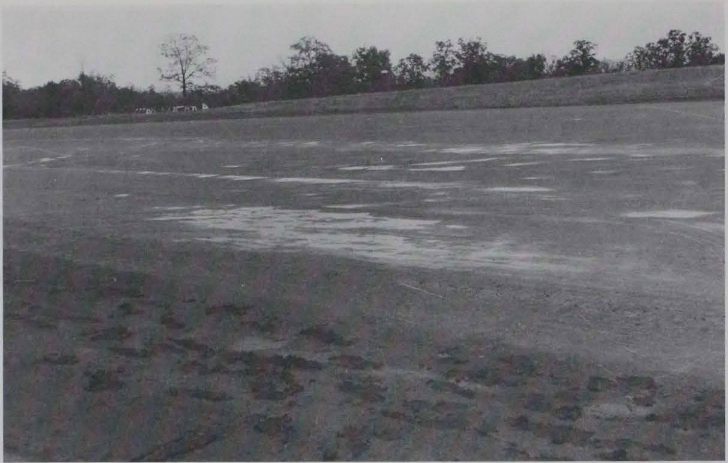
Figure 25. Airstrip surface showing surface swell and some puddling
