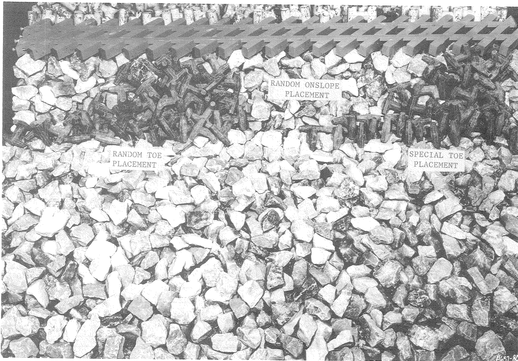
Photo A1. Comparison of random and special dolos toe construction.
