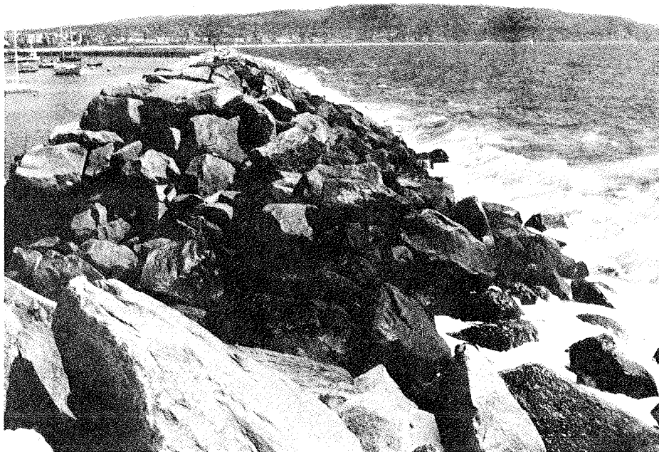
Figure 1. A rubble-mound breakwater protecting a boat harbor
