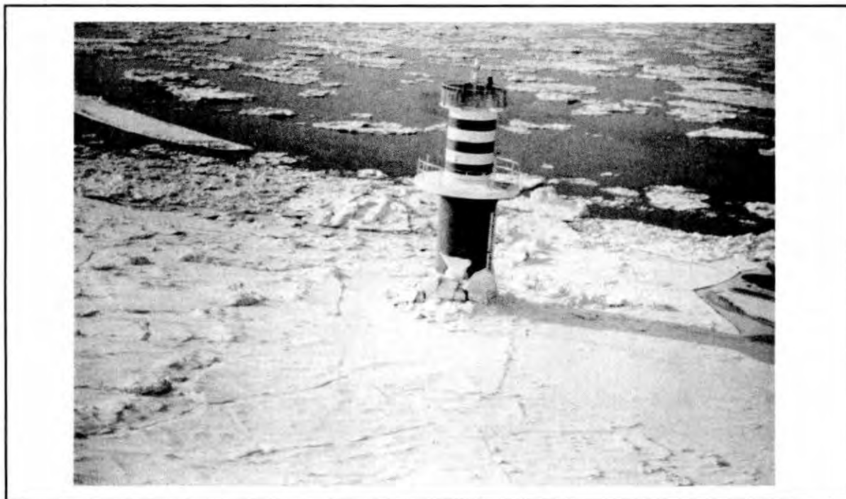
PLATE 8. INTERACTION BETWEEN THE YAMACHICHE LIGHTHOUSE AND A FIRST-YEAR ICE SHEET IN LAC ST-PIERRE IN THE ST-LAWRENCE SEAWAY. COURTESY R.FREDERKING, NRC.
