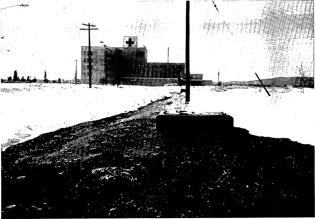
Figure 1. The ground above a buried utilidor in March at Fort Wainwright.
