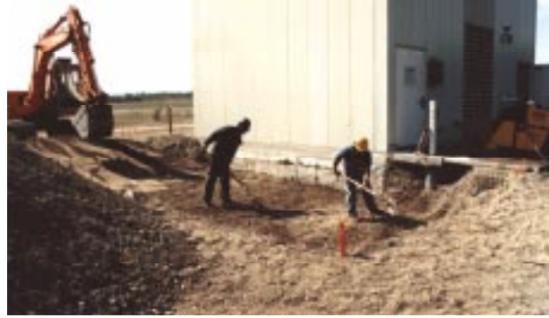
Figure 6. Excavation of foundation.
