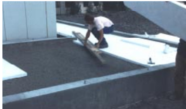
Figure 7. Floor insulation.
