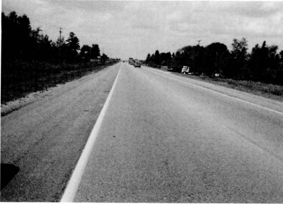
Figure 35. Typical flexible pavement section east of Acme on Route 72, Michigan.
