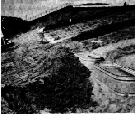
Figure 6. Installing the under-drains for the tanks.
