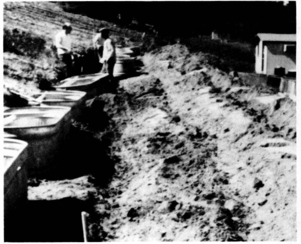
Figure 3. Removing sod from the plots.
