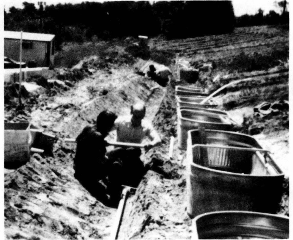
Figure 7. Placing soil around the tanks.
