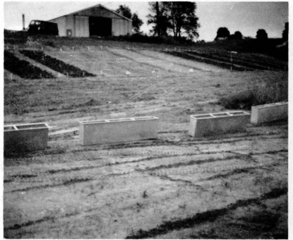
Figure 18. View of finished plots prior to the installation of the sediment tanks.
