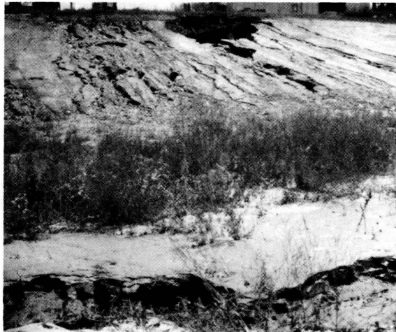
Figure 16. Overall view of damage incurred by water main break, looking southeast.
