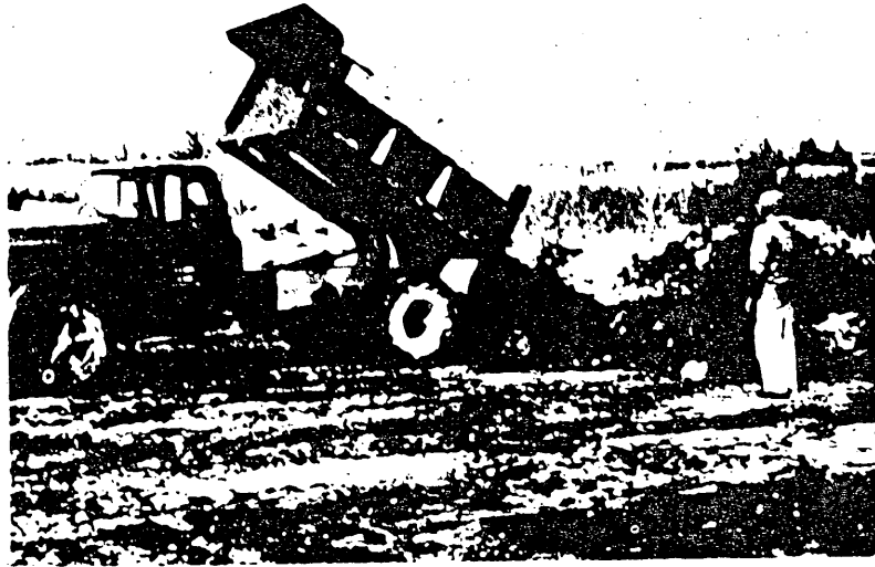
FIGURE III-3A PLACING OF FILL MATERIAL
