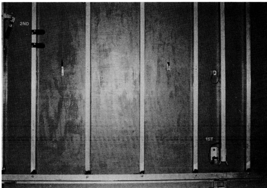
Figure 3.4.1. Support arms. Be sure to unpin the bottom of the support arms, First , before fastening the porch latches, Second .
