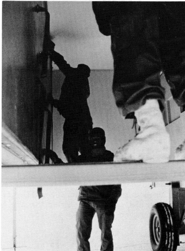
Figure 3.4.8. Walking along the beams to unhook the floor.
