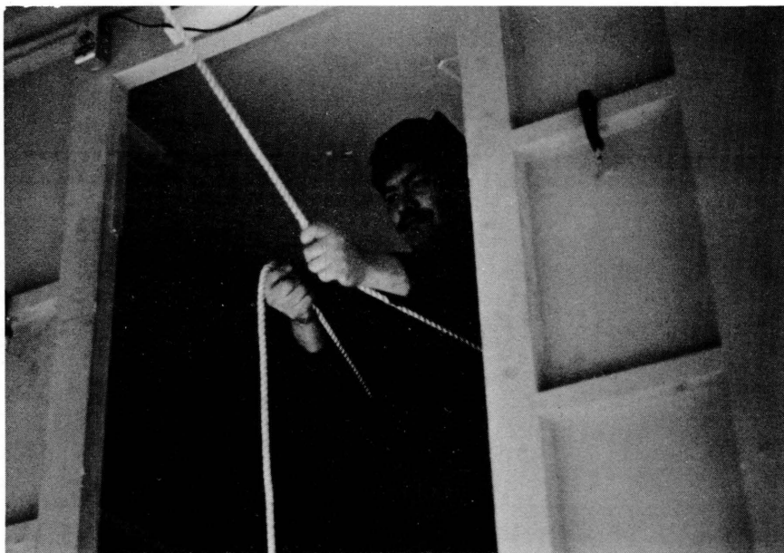
Figure 3.4.7. Snubbing the line around the waist to control the floor.
