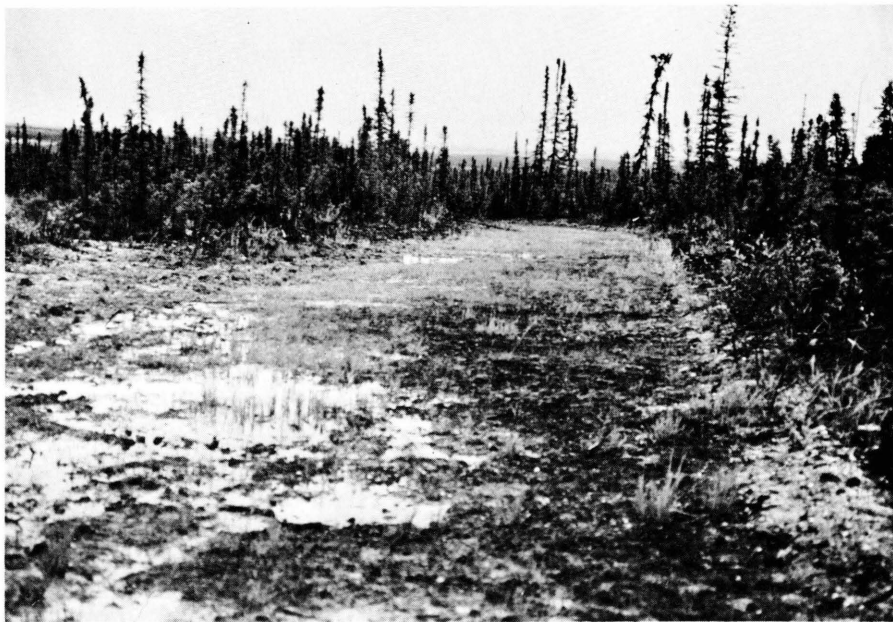
Plate 22. A.S. 81-82: Winter haul road on east side seeded, just south of No-Name Creek. Cover 10% on organic substrate and 20% on more sandy substrate.
