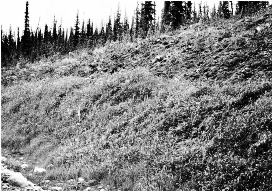
Plate 10. A.S. 107 (Station 35732): Organic mat folding over road cut. Trees were cut above the road cut to avoid shearing of the slumping organic mat.
