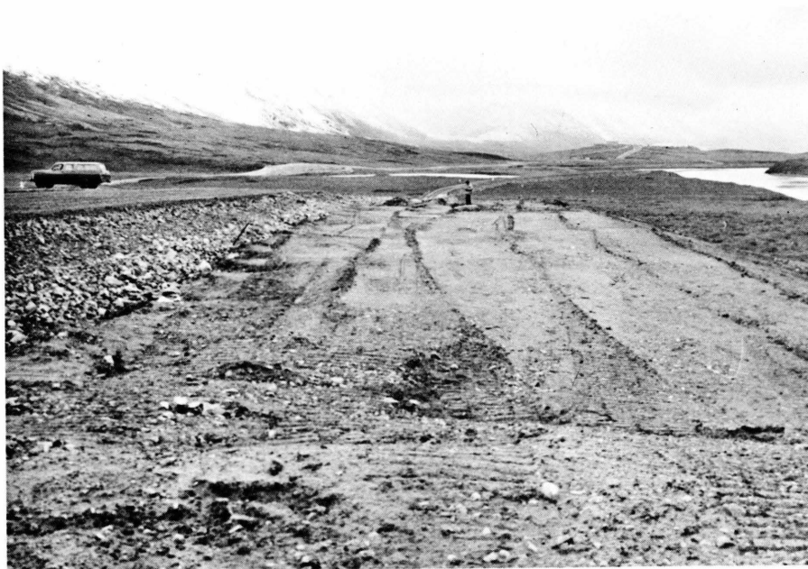
Plate 5. A.S. 114: Seeded disposal blankets along shoulder of road between Galbraith Lake access road and Atigun River cut.
