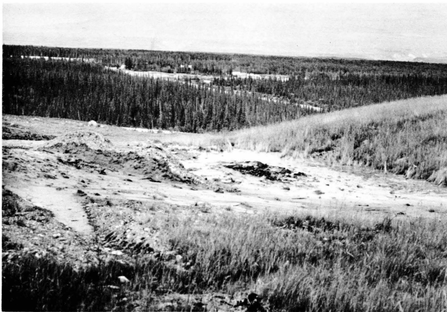
Plate 35. Material Site 17-5: Disposal materials used to cover gravel and then reseeded. Upper area had almost 100% plant cover.
