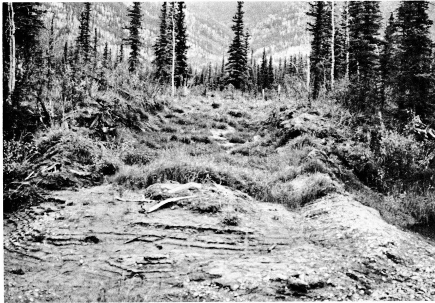
Plate 15. A.S. 100: Abandoned and bladed trail was seeded and mulched with hay just north of Middle Fork Koyukuk.
