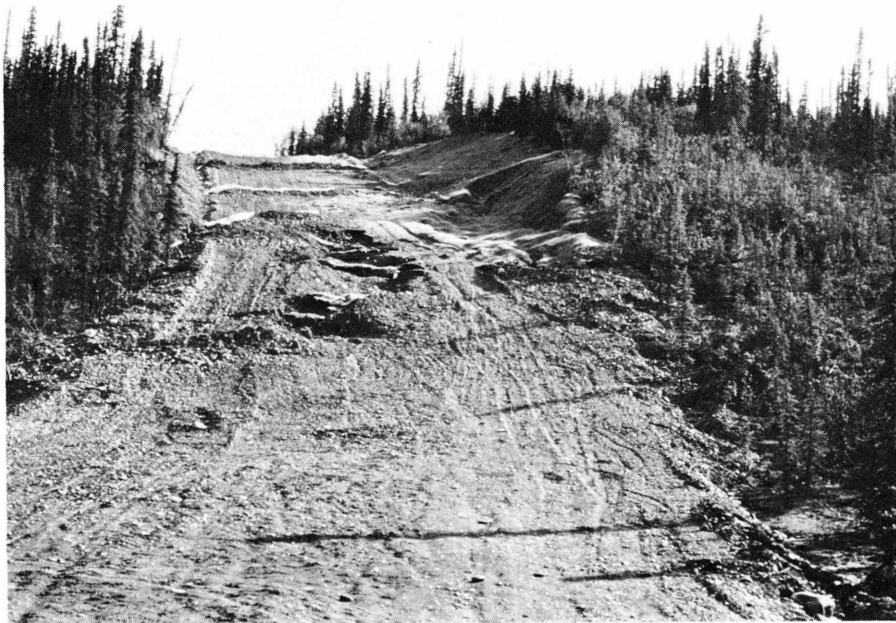
Plate 34. A.S. 18.1: Ice-rich soils exposed and eroding despite gravel overburden and thick hay mulch.
