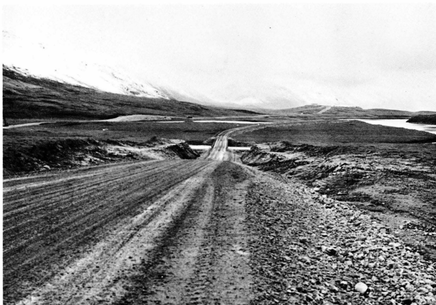
Plate 6. A.S. 114: Near vertical road cut hydroseeded and mulched on north side of Atigun River.
