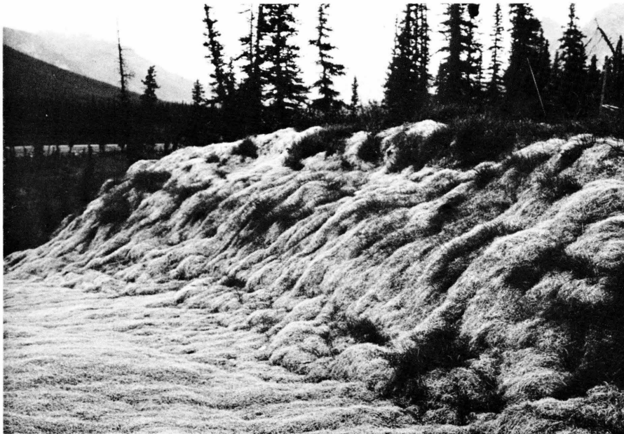
Plate 13. A.S. 102: Excelsior mats used to stabilize hand seeded cut on east side of work pad; growth mostly annuals.
