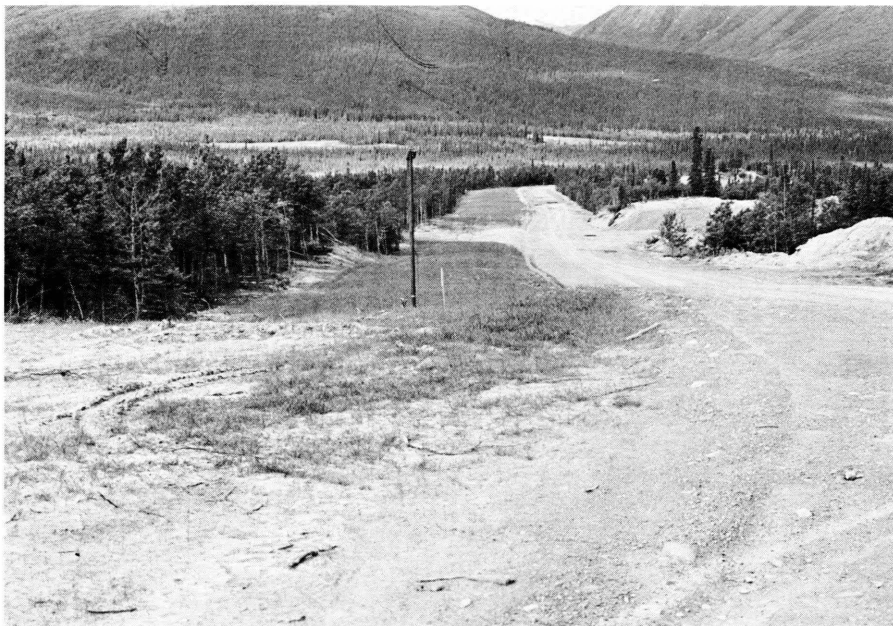
Plate 38. North of Pump Station 12: Intersection of workpad with Richardson highway. Entire width of workpad seeded over buried pipe.
