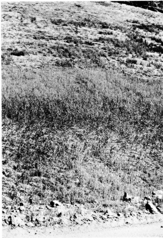
Plate 30. A.S. 48: About 1 mile north of Tanana River, road cuts in ice-rich silt, hydroseeded and hay mulched. Tractor had been run up and down the side slope to produce depressions for holding seed and moisture.
