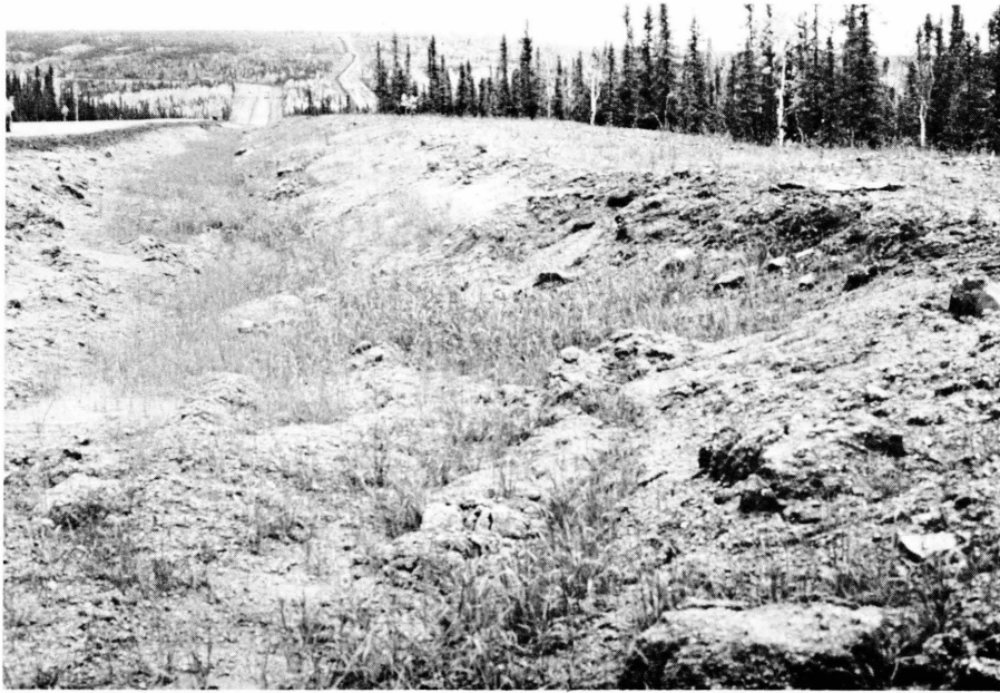
Plate 19. A.S. 90: Hydroseeding over weathered granite substrate.
