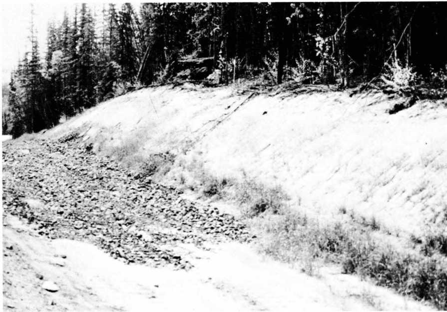
Plate 23. A.S. 80: Roadcut seeded on east side of Haul road north of 80-3.1. Germination very low on upper slope.
