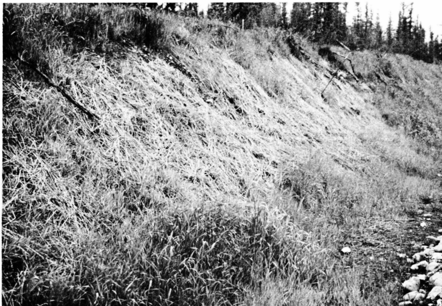
Plate 14. A.S. 101: Straw mulch and hydroseeded Haul road cut.
