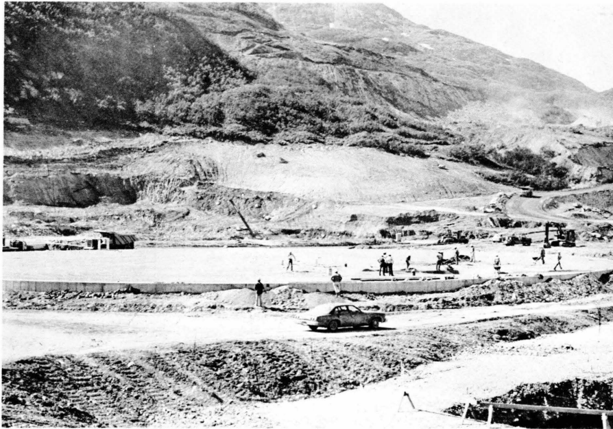
Plate 39. Valdez Terminal: Areas hydroseeded.
