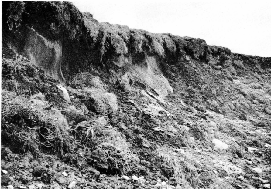
Plate 3. A.S. 122: Happy Valley road cut with ice wedge meltout and slumping.
