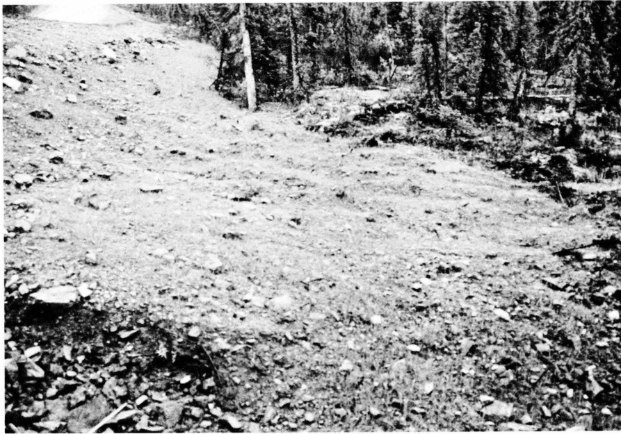
Plate 21. A.S. 84: West side of road hydroseeded with wood fiber mulch (beside a stream). Some barley and chenopods germinating from hay.
