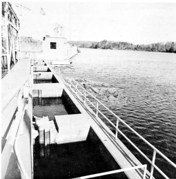
Figure 12. Gauge house and impoundment area, Wilder Dam, Wilder, Vermont.
