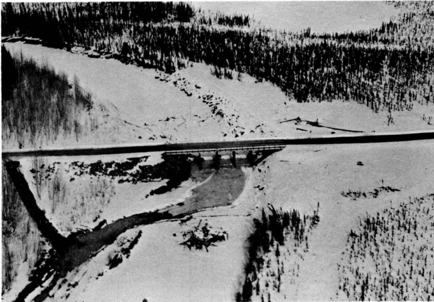
Figure 35. Hess Creek Bridge on TAPS road.
