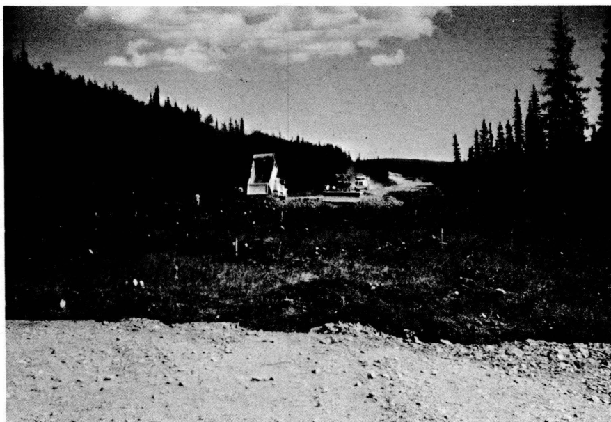
Figure 4. End dumping on Goldstream Road.
