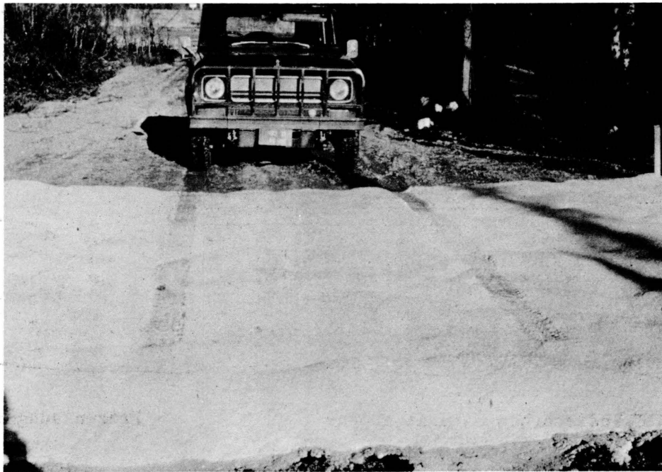
Figure 6. Foamed-in-place polyurethane (FIP).
