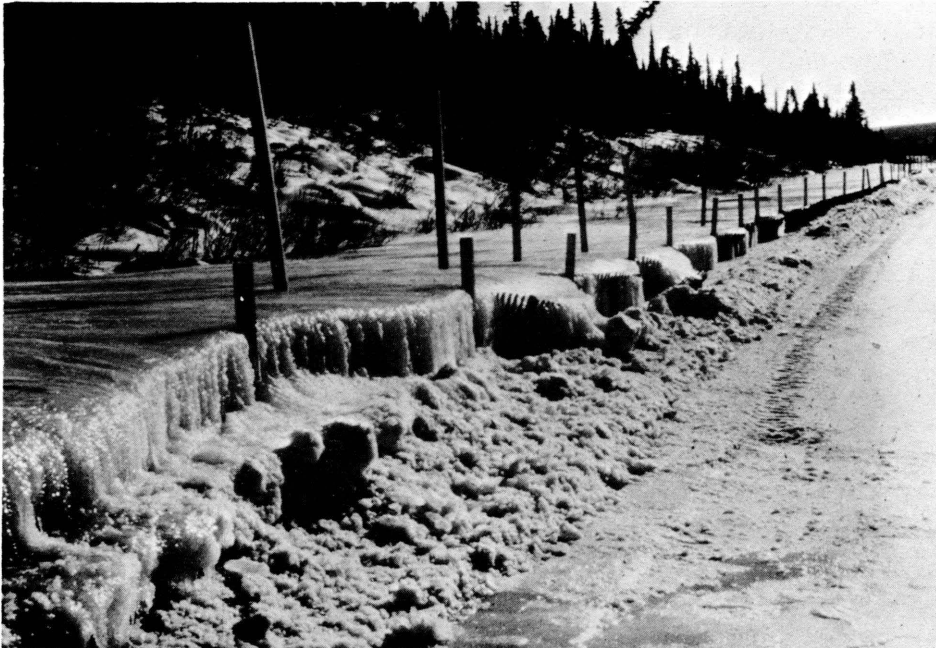
Figure 32. Fence to control icing on the Richardson Highway near Paxson, Alaska.
