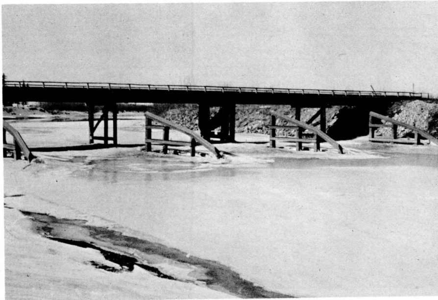
Figure 38. Ice and debris deflectors to protect bridge bents, Engineer Bridge, Fort Wainwright.
