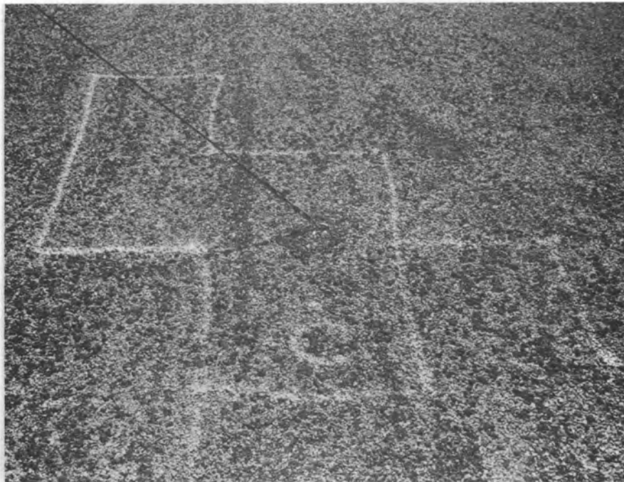
Figure 6. 1975 thermogram and 1975 photograph of wet area surrounding bolt, Building 120 (arrow points to bolt).
