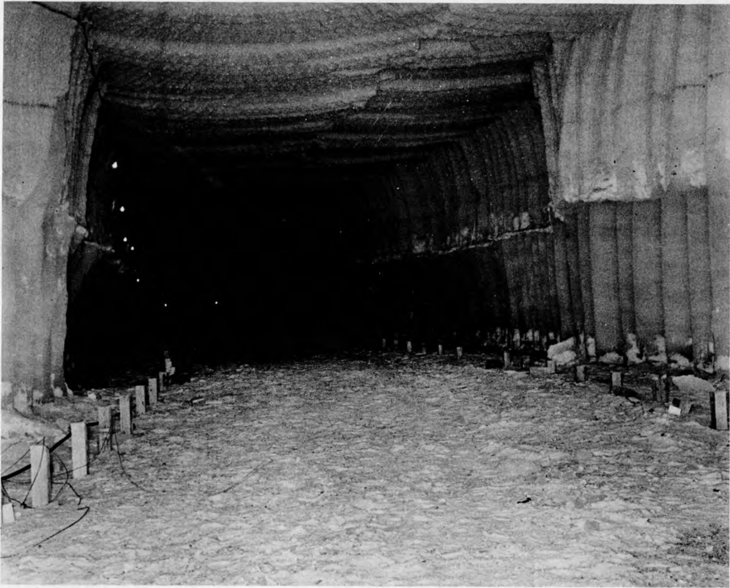
Figure 4. Underpinning frozen in place ready for erection of Mess and Latrine buildings.
