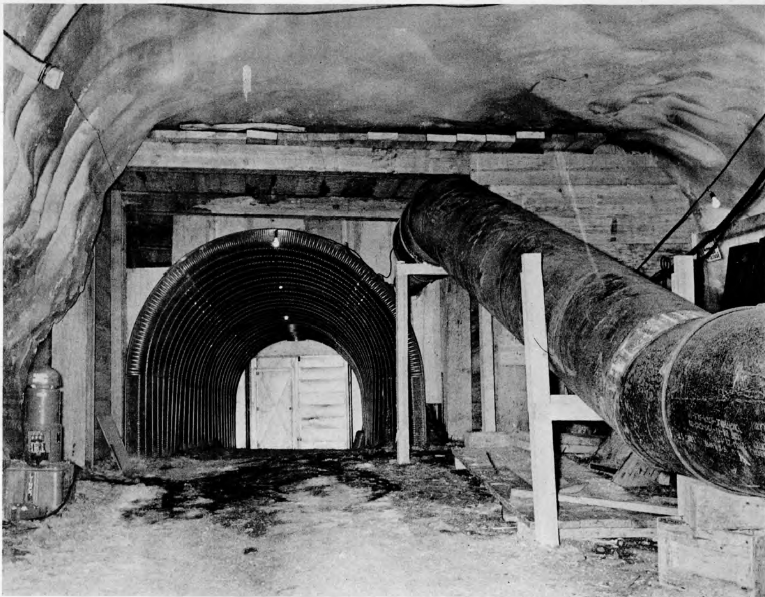
Figure 8. Interior of portal looking toward door opening, showing outer and inner portal structures and 30-in. ventilation exhaust line.
