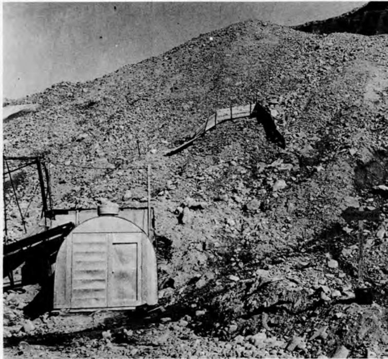
Figure 9. Portal exterior showing moraine veneer covering ice cap at this point, and ventilation exhaust. Fresh air intake is through ventilation in roof.
