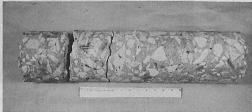
Figure 12. Concrete cores drilled from abutment
