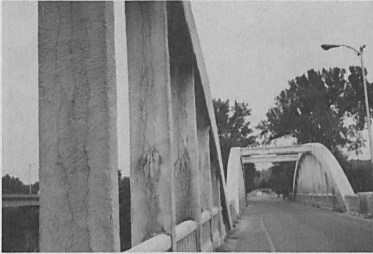
a. Overall view
