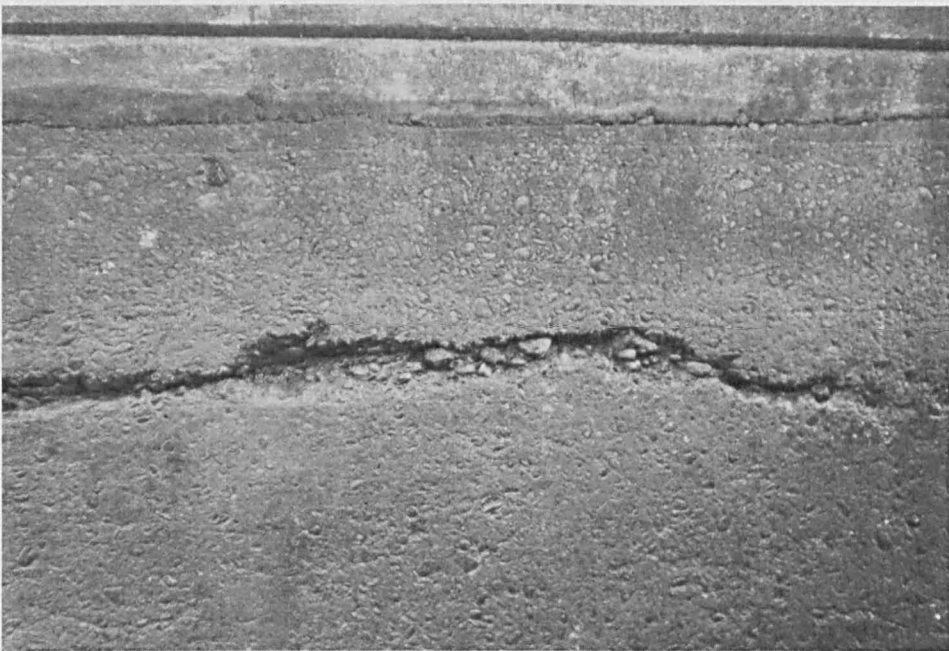
Fig. 35 Land wall, lock chamber face.
