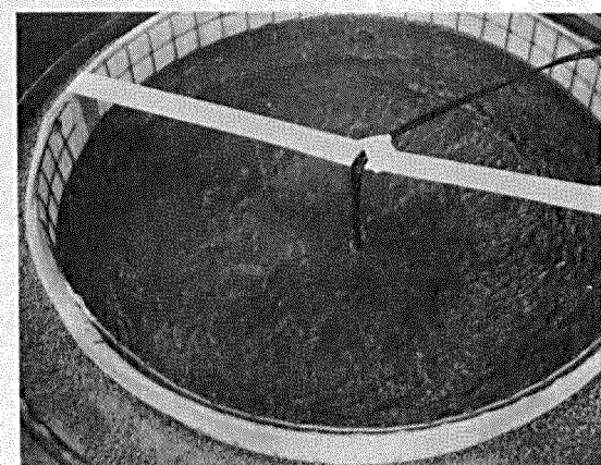
f. Thermocouple located in center of grout core
