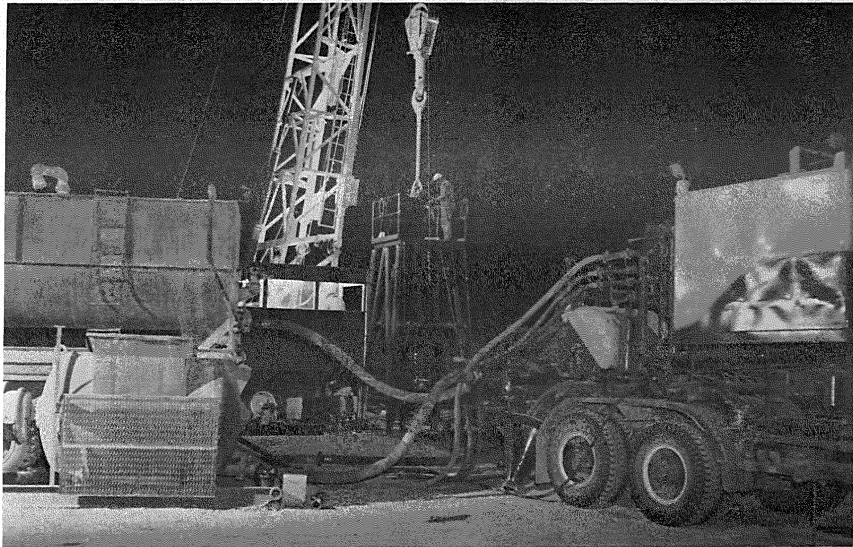
Photograph 3. Typical grouting equipment setup
