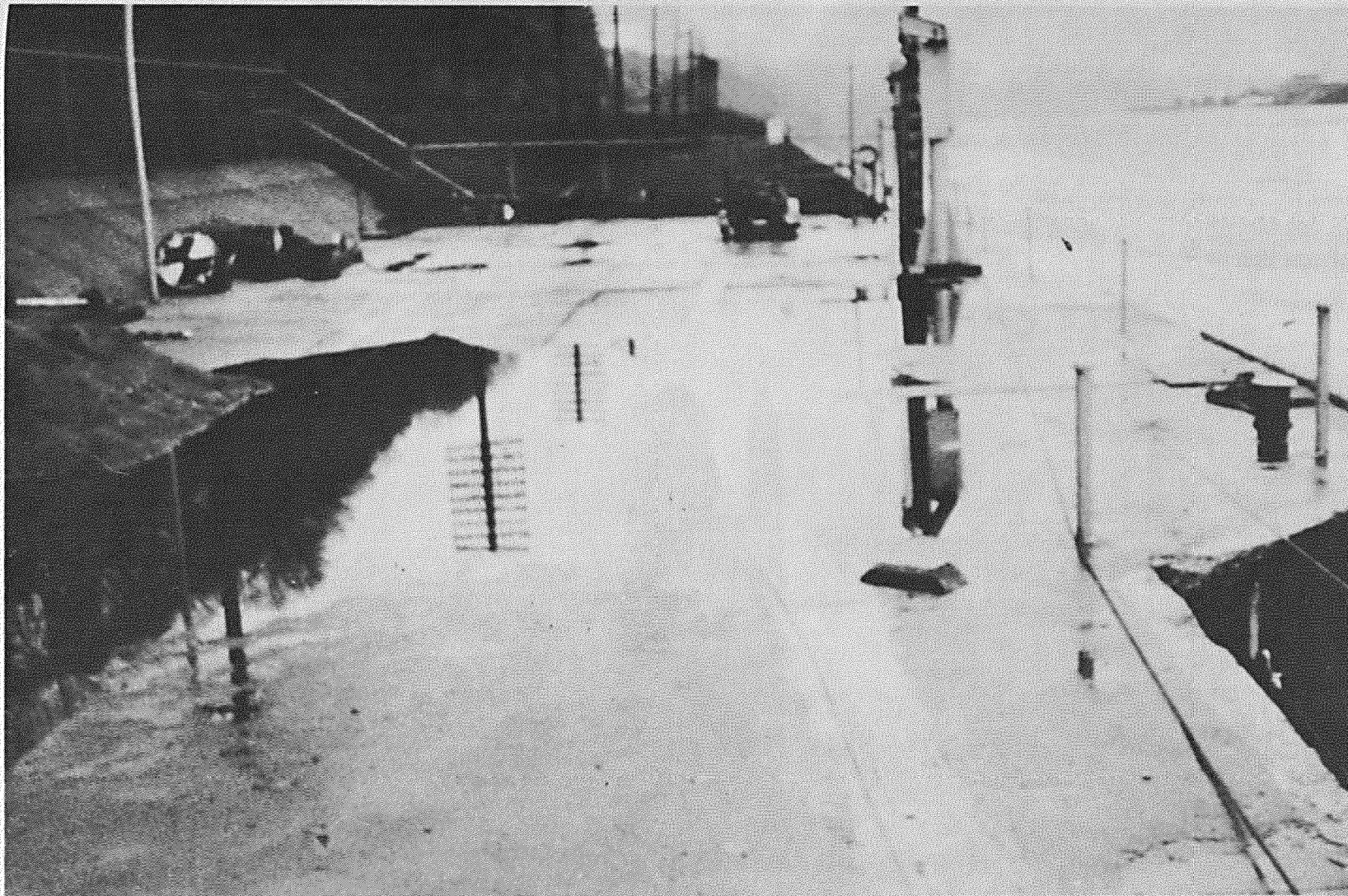
Figure 2.1 Differential settlement in the Esplanade which holds water
