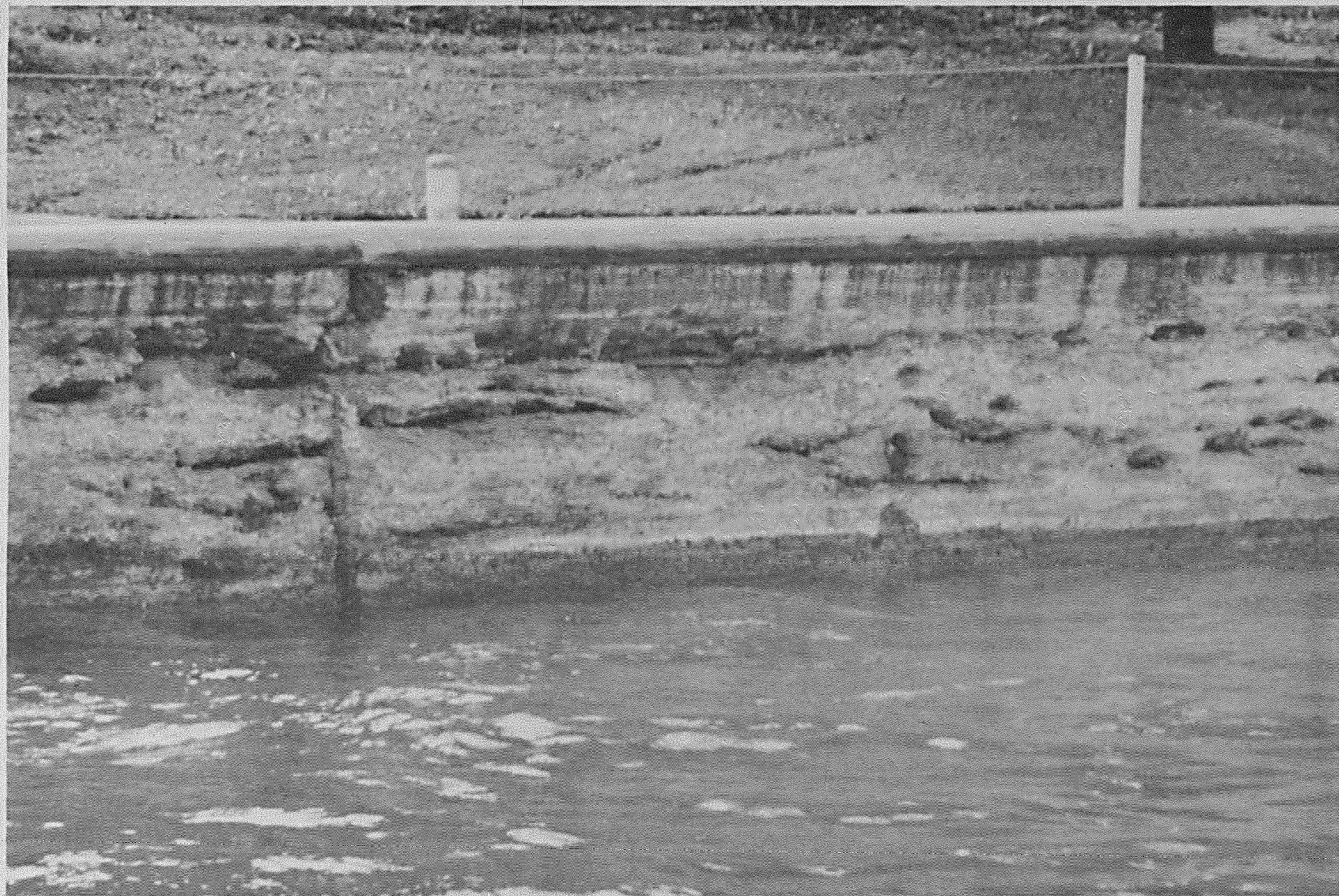
Figure 6.1. Gouged Upper Guide Wall
