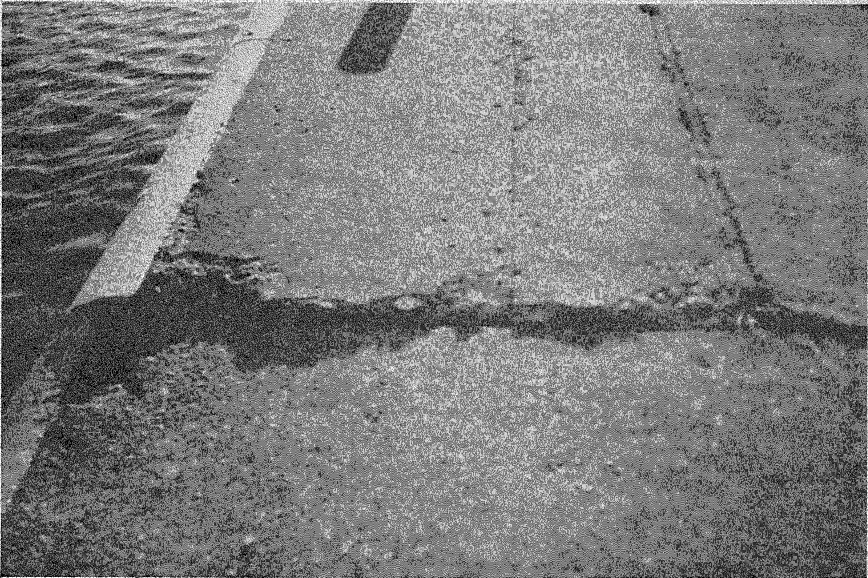
Figure 6.3. Tilted Upper Guard Wall
