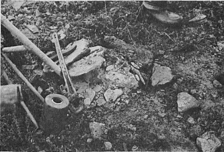
Figure III.3. Backfill Removed with 6-in.-Diameter Core Barrel (M-7).
