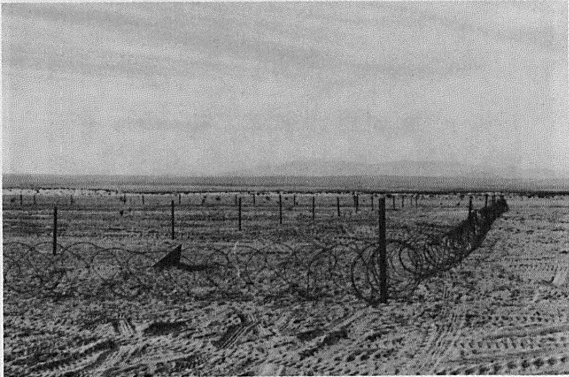
Figure 12. Barbed wire and concertina wire surrounding Site II with corner reflector.
