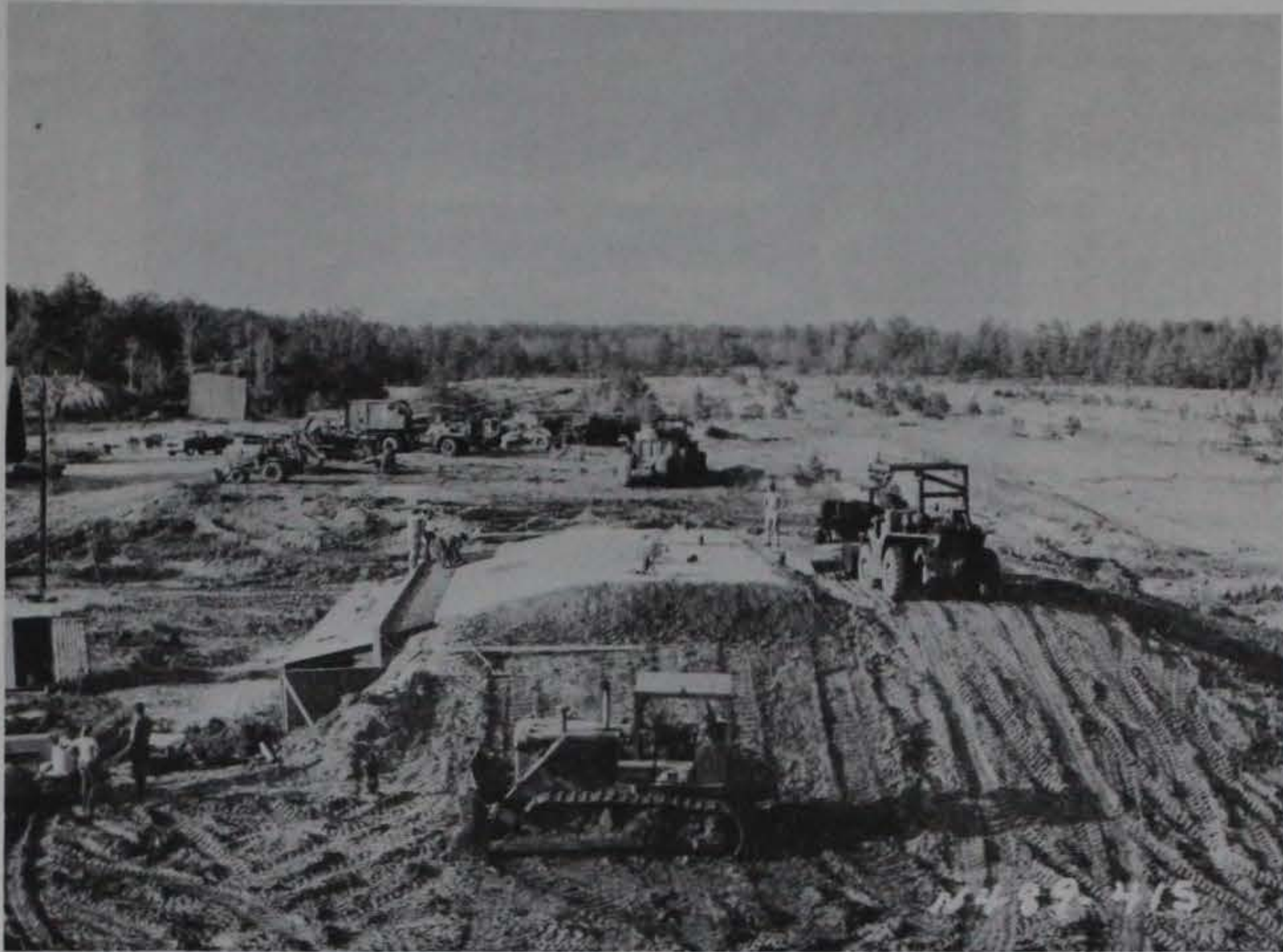
Figure 3.25. Sand layer over bays and air locks.
