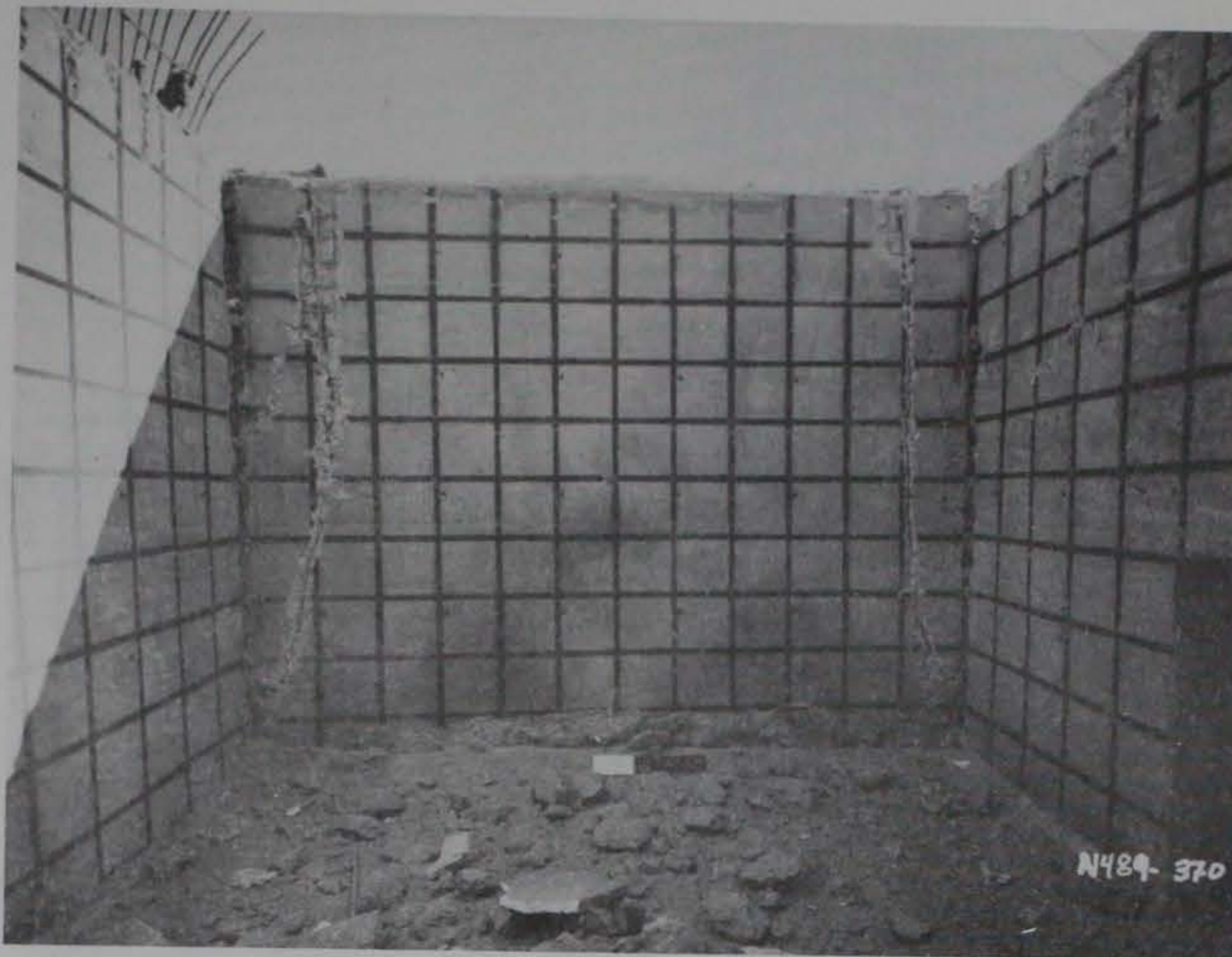
a. Overall view.
