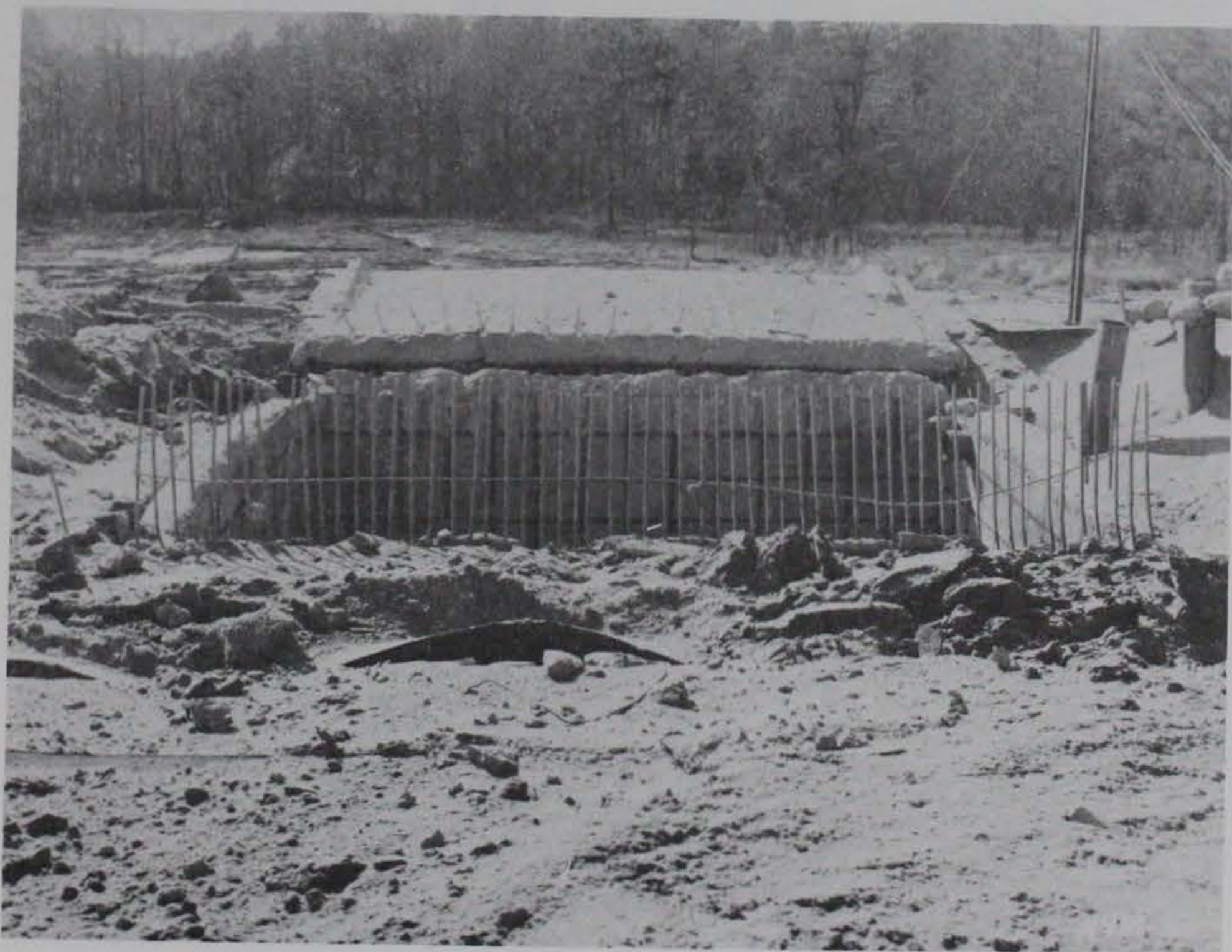
b. View facing west.
