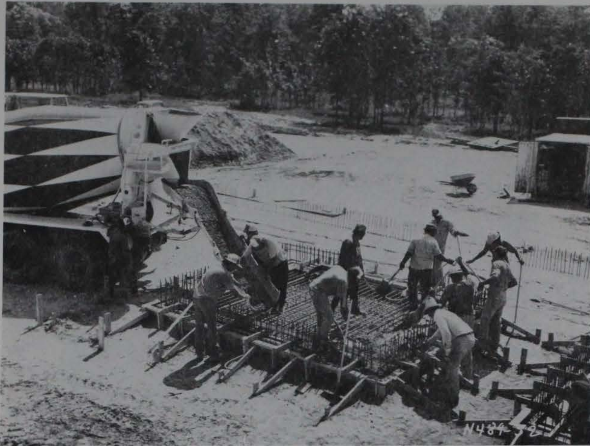
Figure 3.11. Concrete placement in bay floor.
