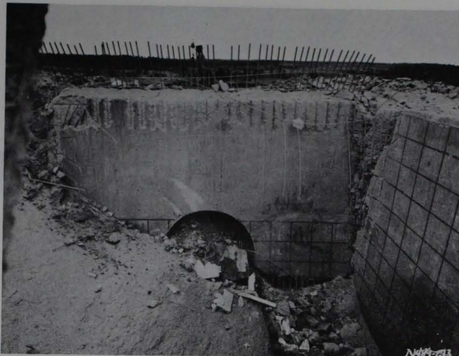
a. Overall view.
