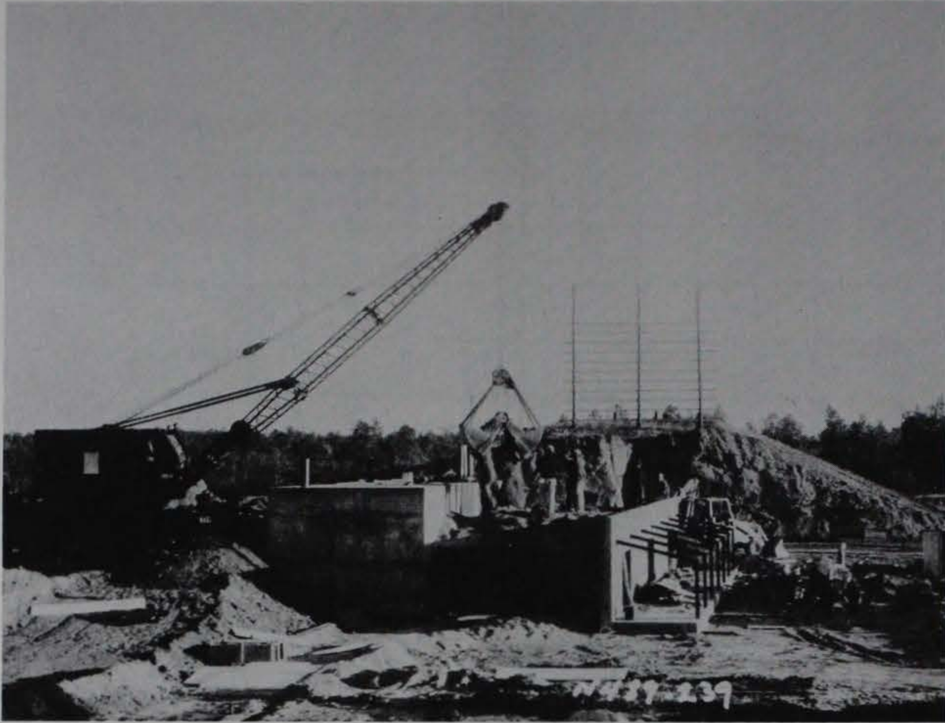
a. Placement of select sand between bays.
