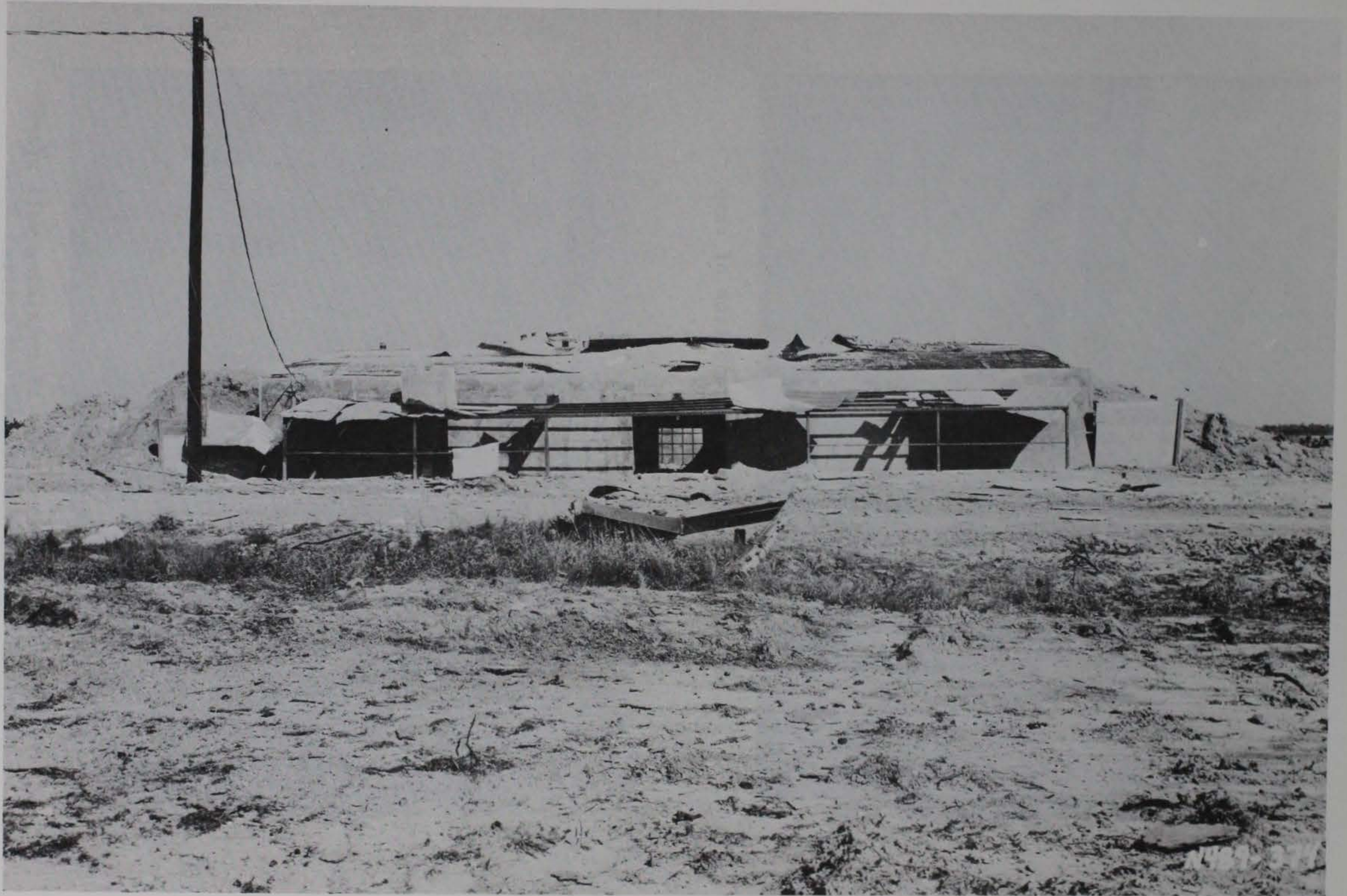
Figure 5.20. Posttest view of Phase II structure.
