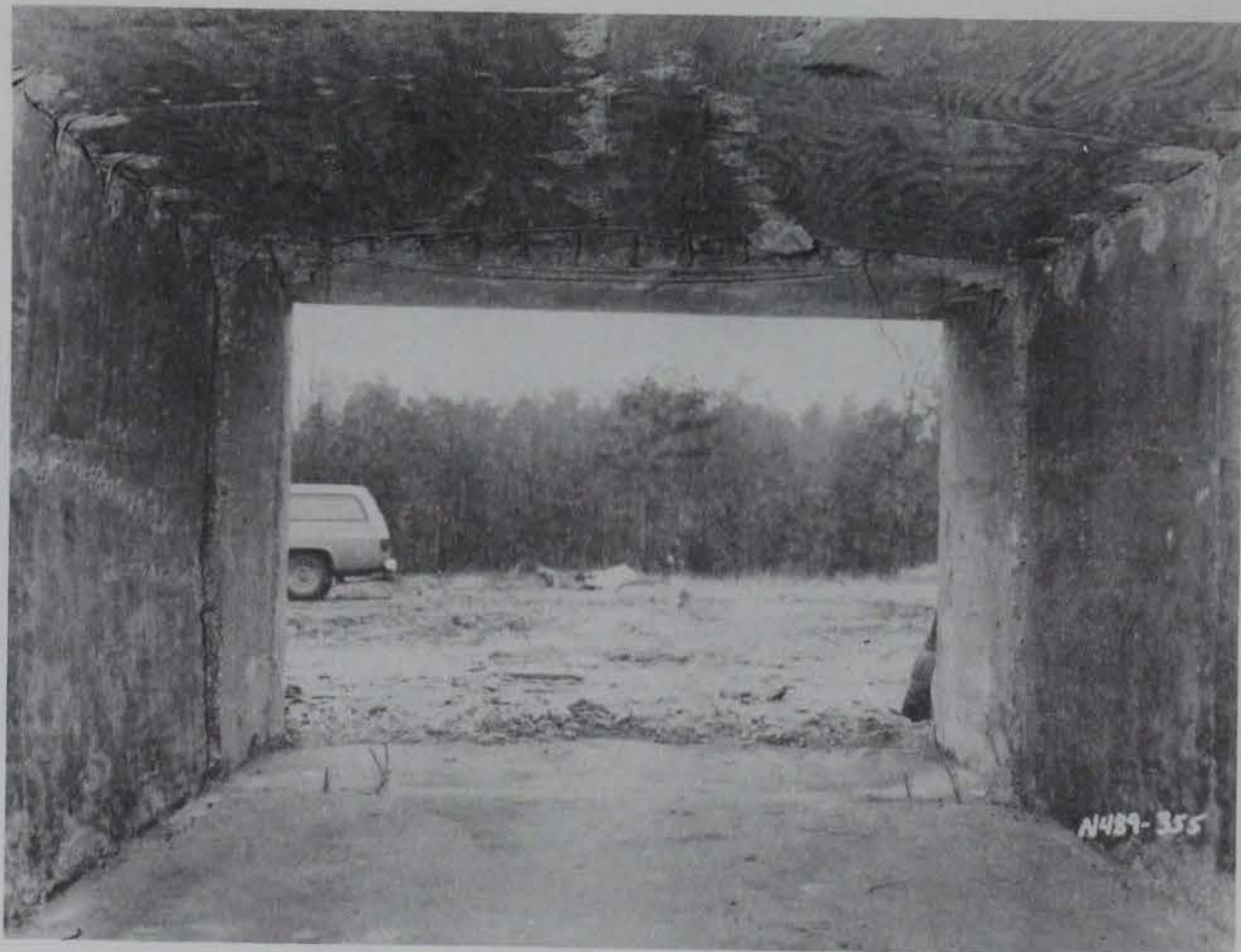
b. Internal view at door bulkhead.
