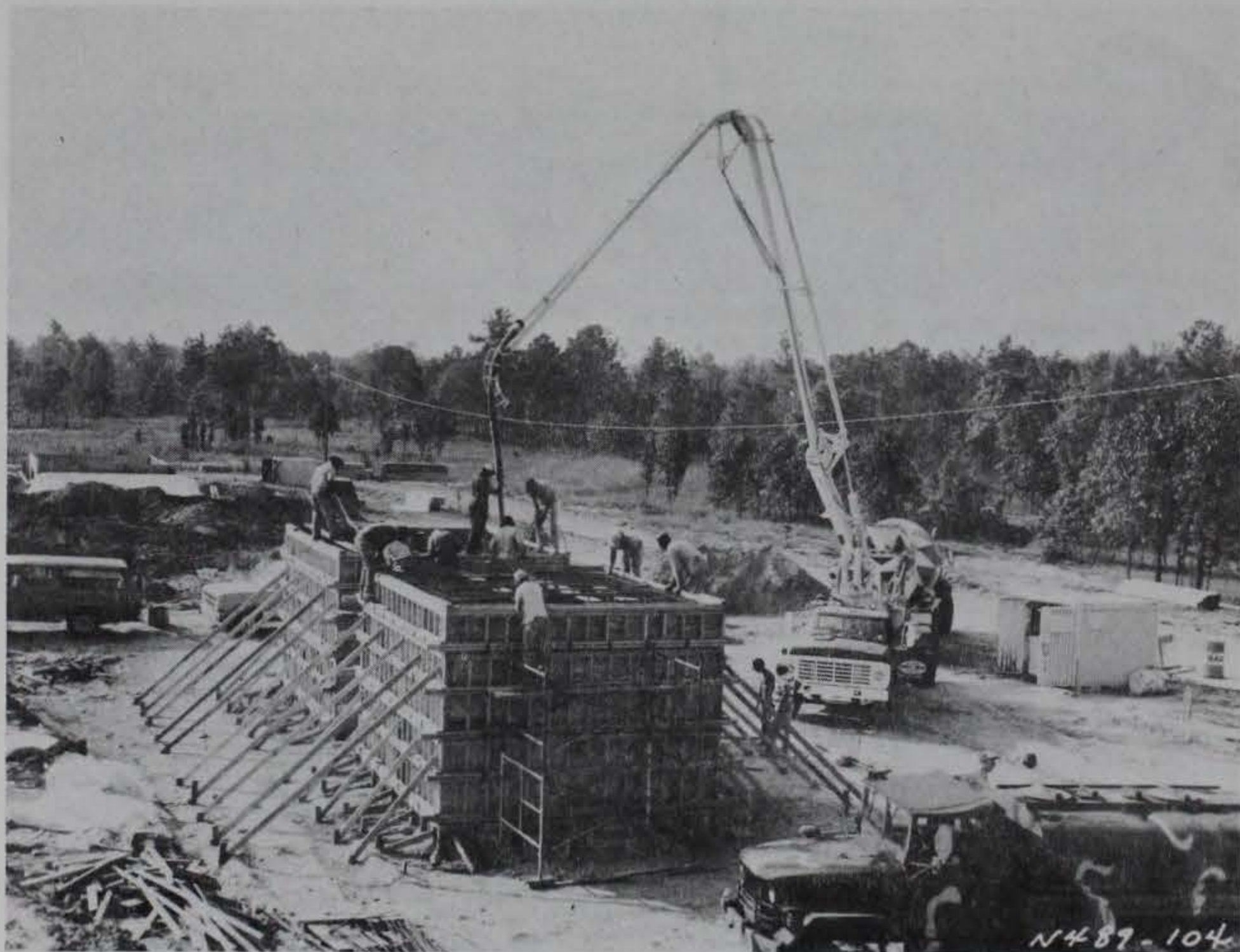
Figure 3.15. Concrete placement in bay walls.
