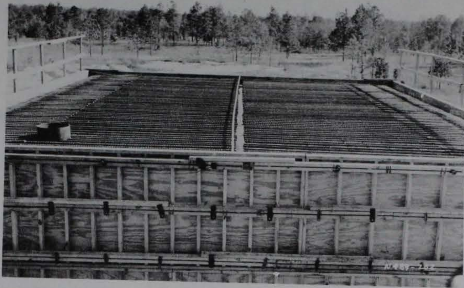
a. Overall view.
