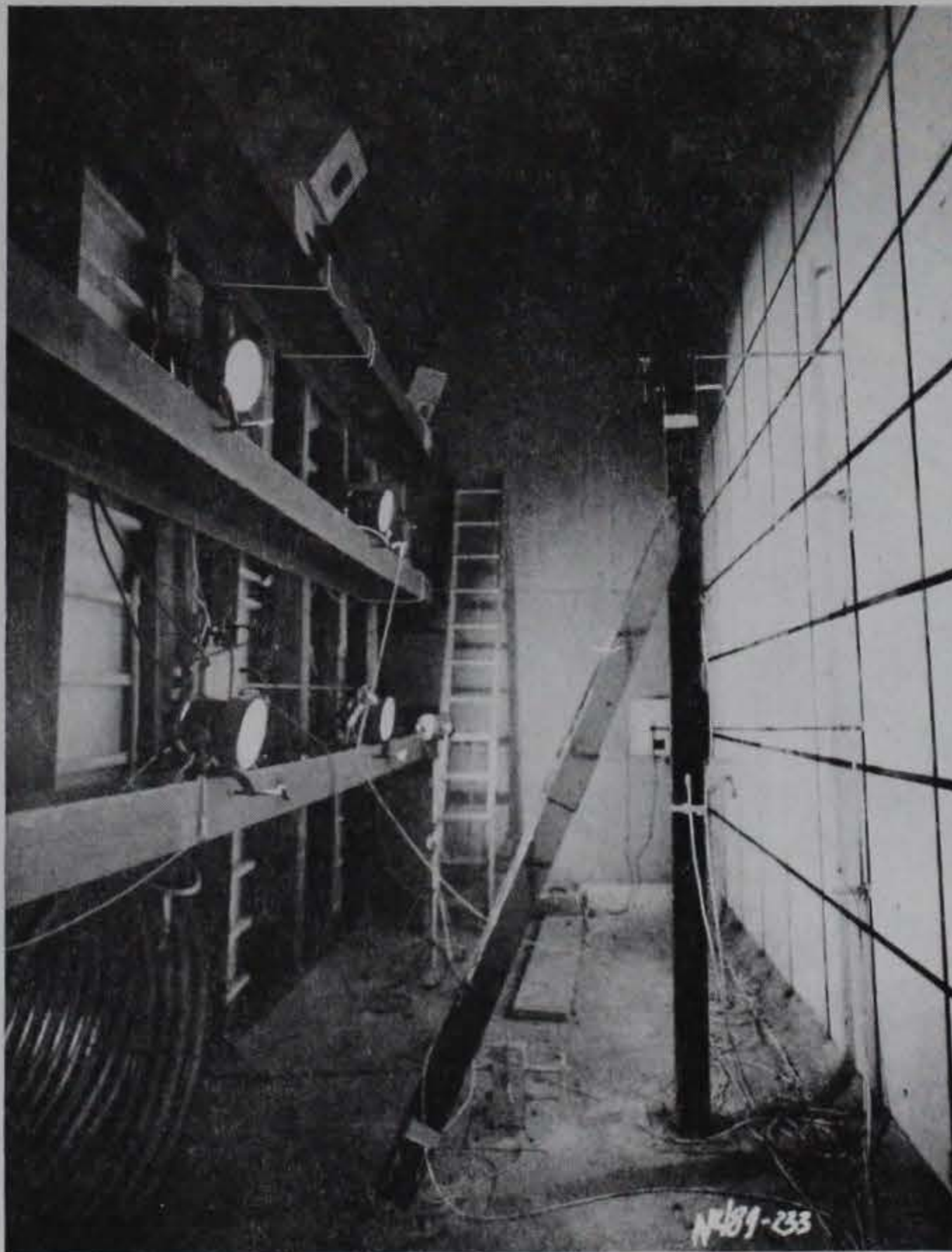
Figure 2.29. Interior of acceptor bay.
