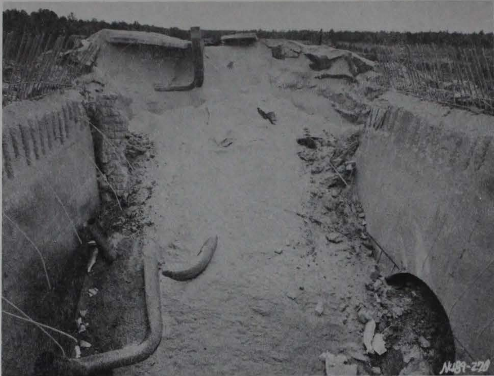
a. Before excavation.
