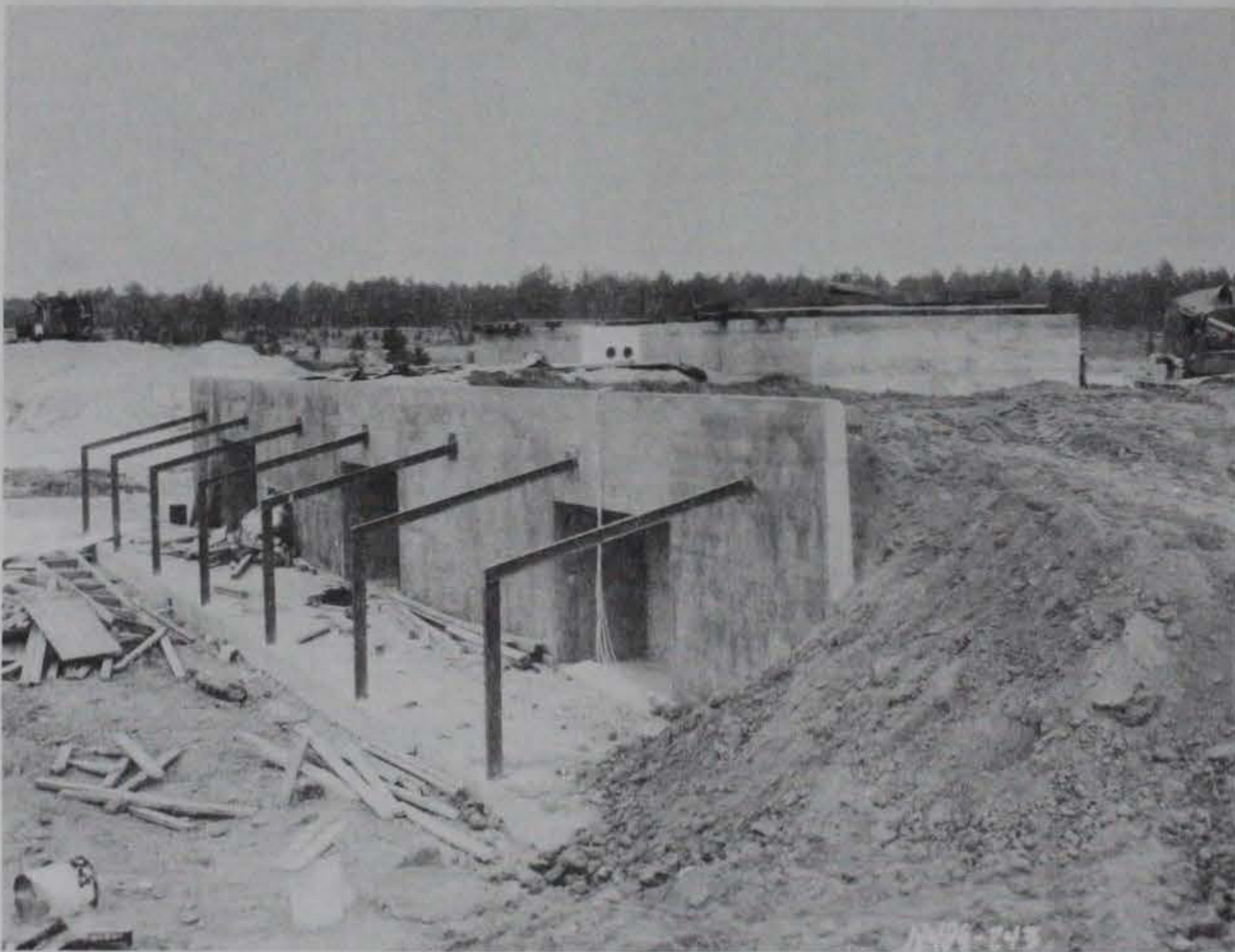
b. Native soil placed around bays.
