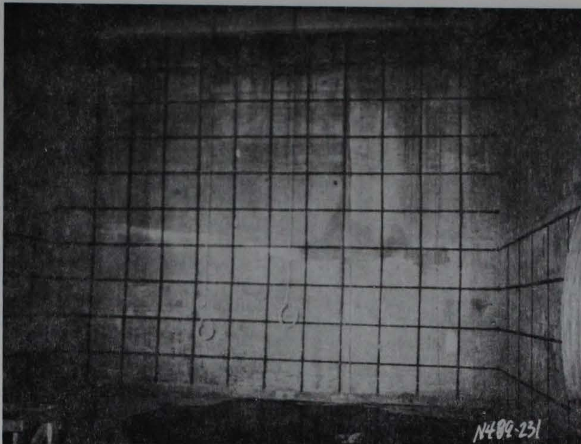
a. North wall.
