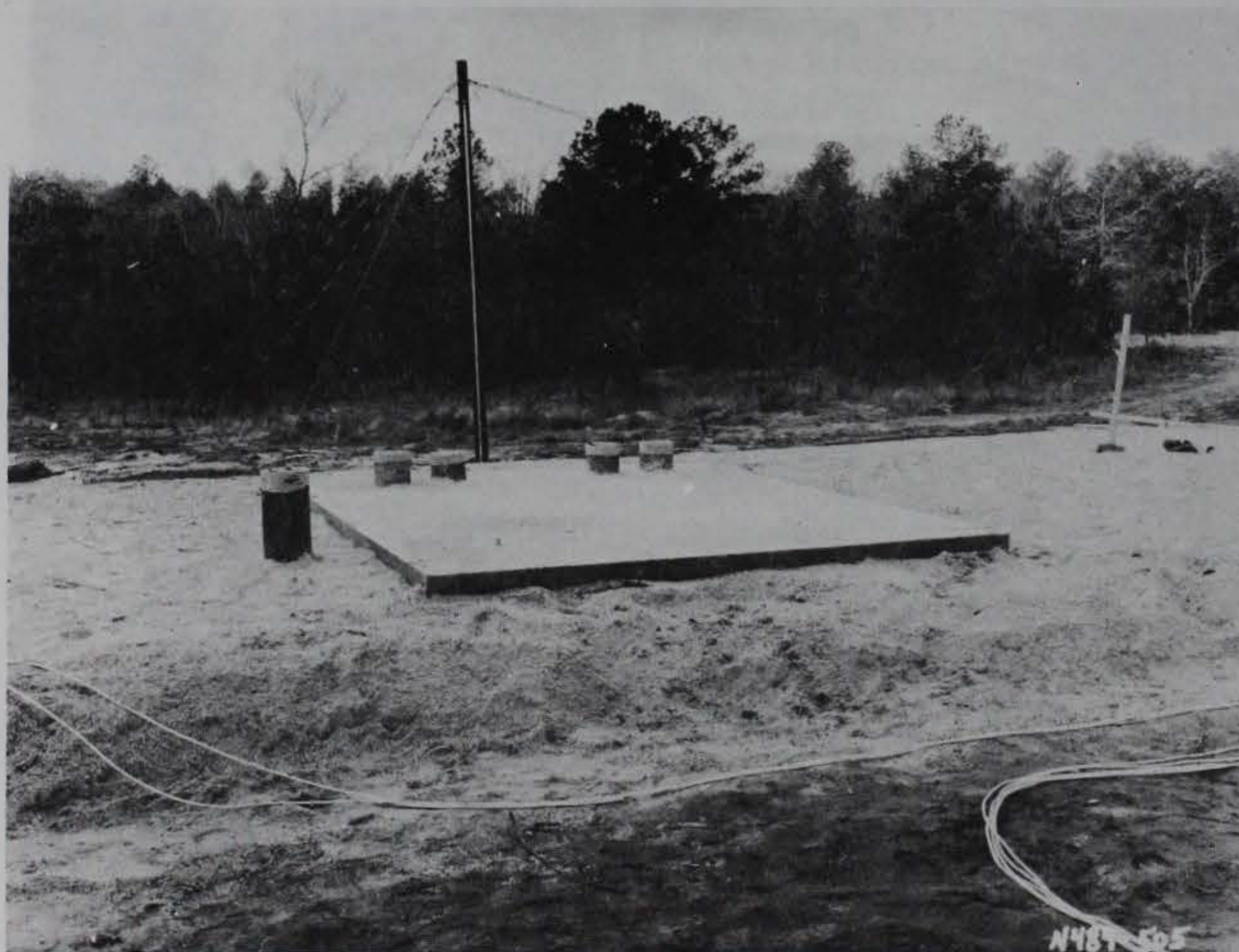
b. Completed penthouse slab.
