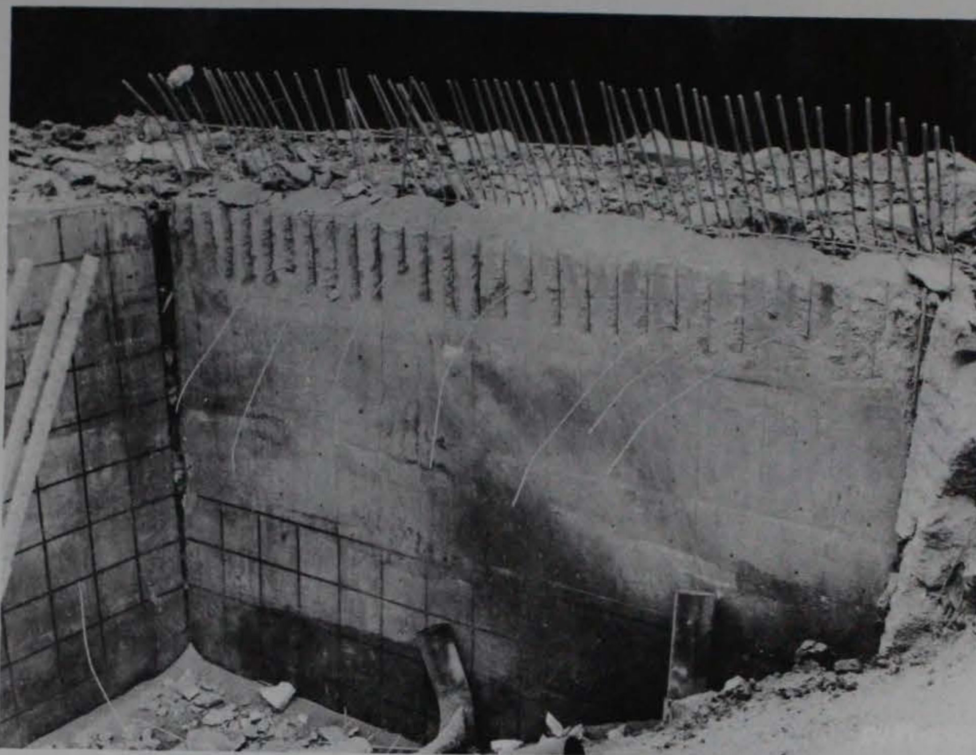
a. Overall view.
