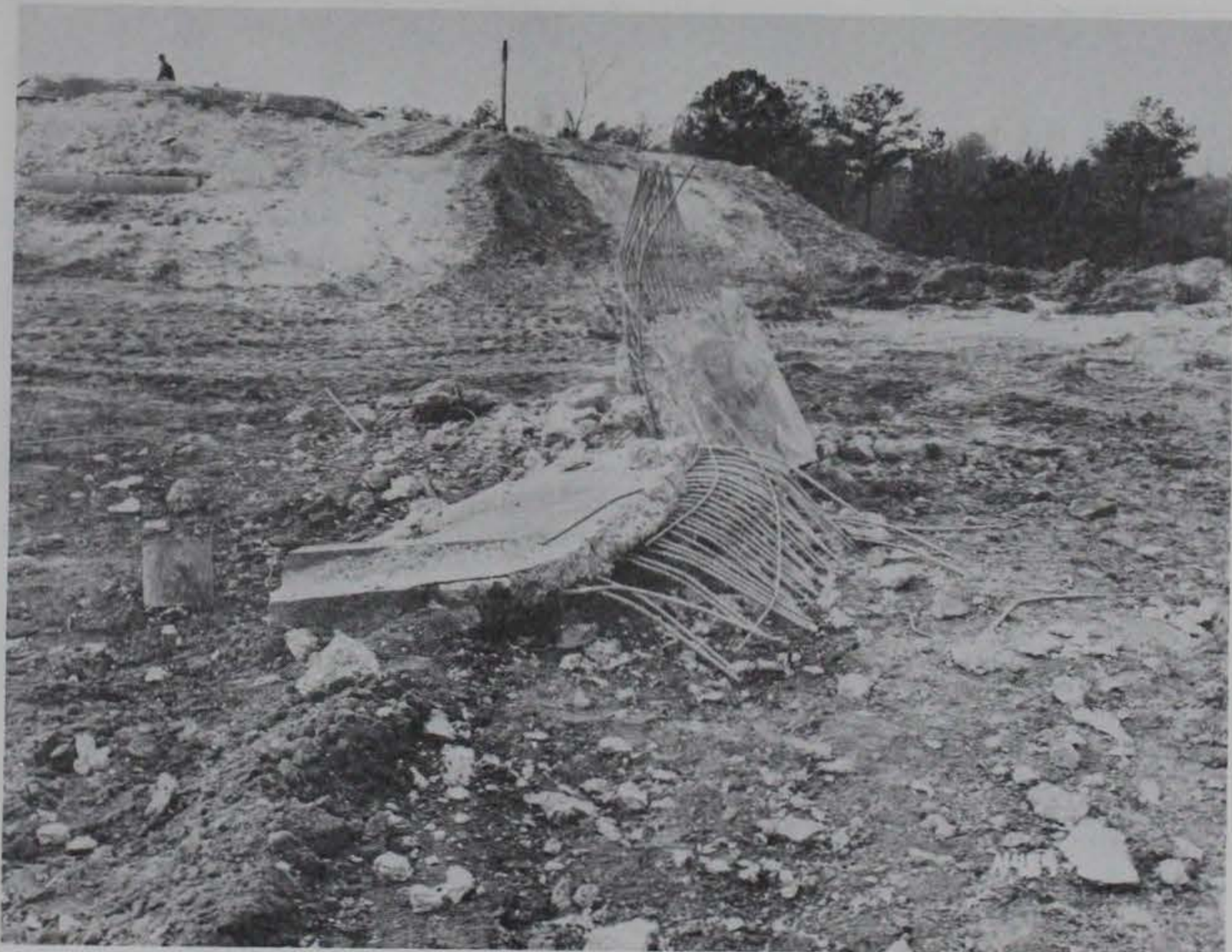
b. View facing west.
