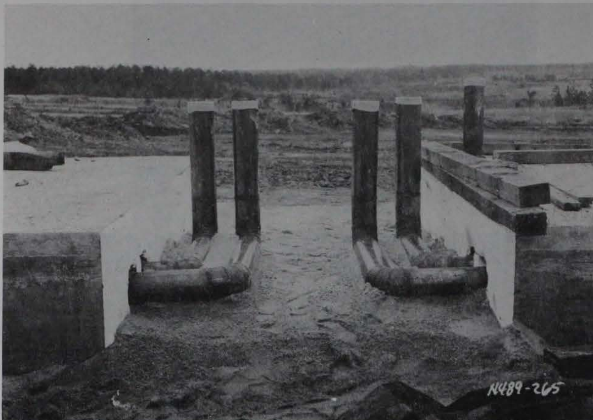
a. Installed ductwork.
